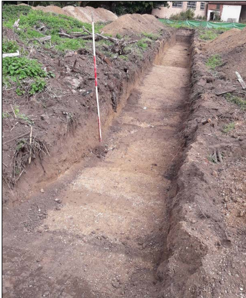
Plate 7. Trench 3, general view (camera facing northeast; 2m scale)
