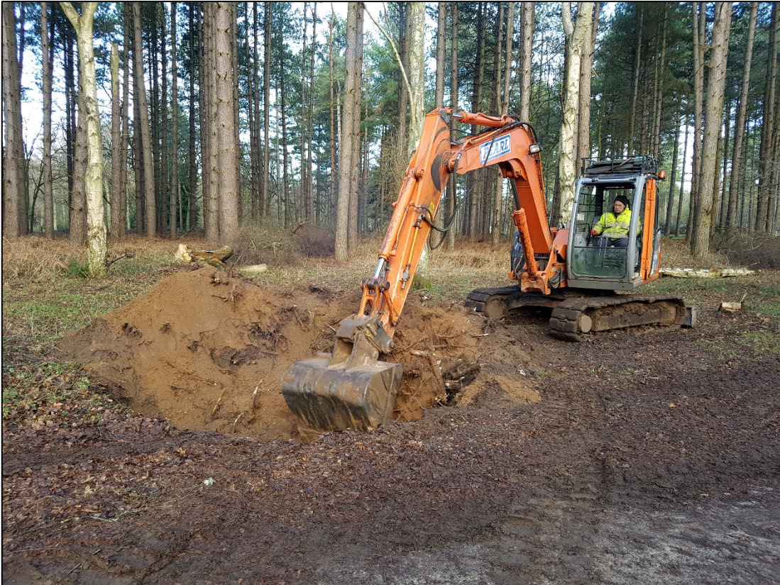
Plate 4. Tree stump removal
