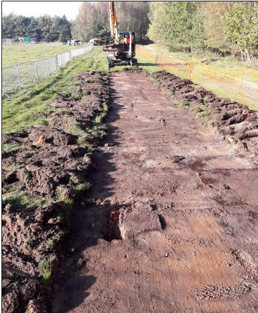
Plate 3. Soil strip in area to south of Horseshoe Pit
