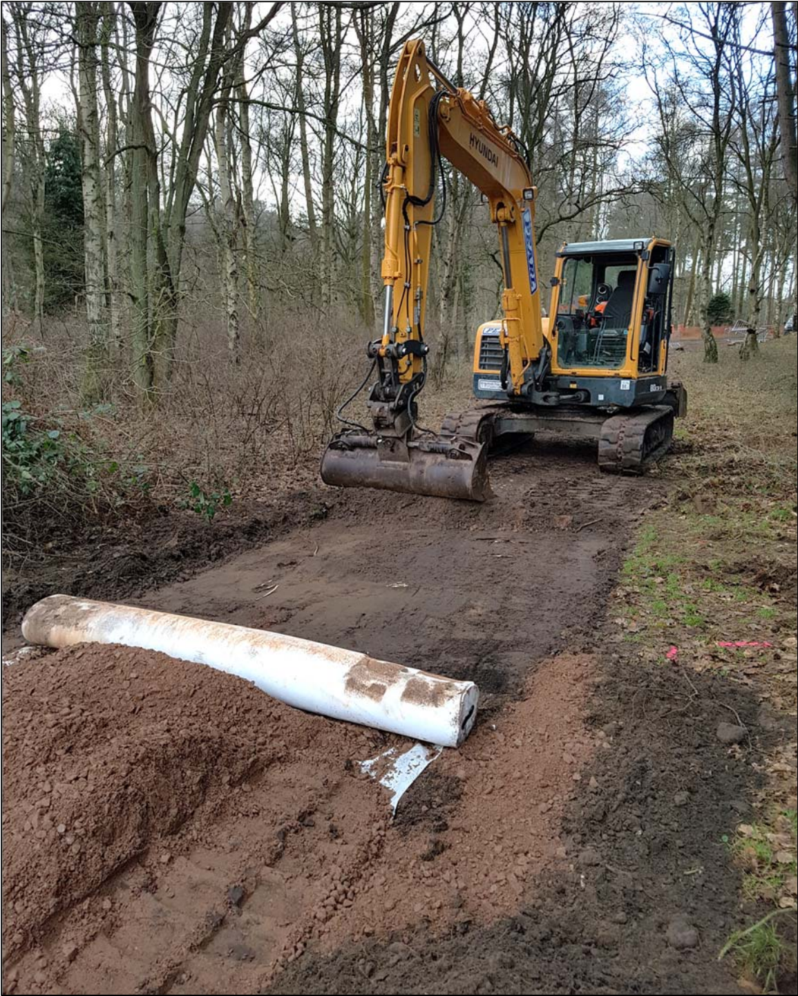
Plate 1. Typical trail construction (in area of former High Lodge Farm)
