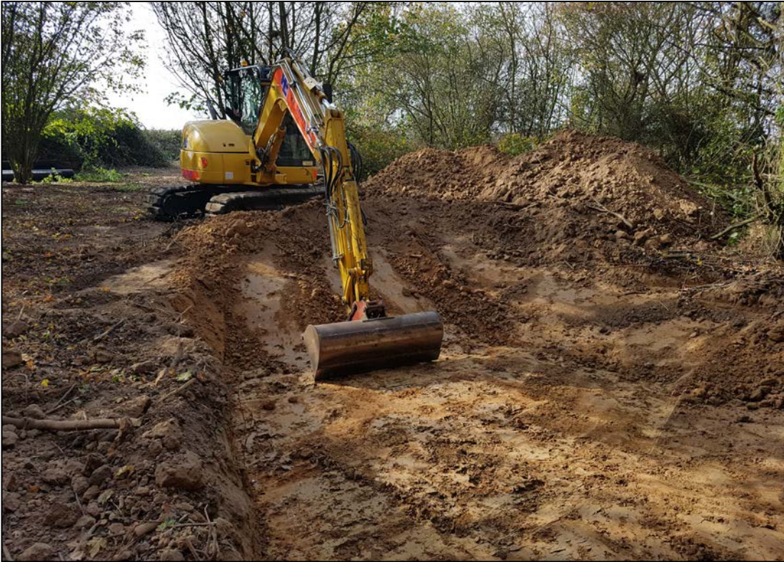
Plate 1. General view of works underway, camera facing south
