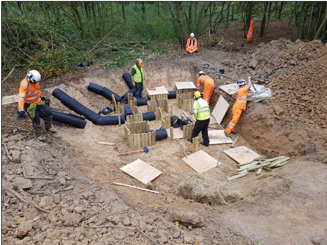
Plate 4. Construction of artificial sett underway, camera facing northeast
