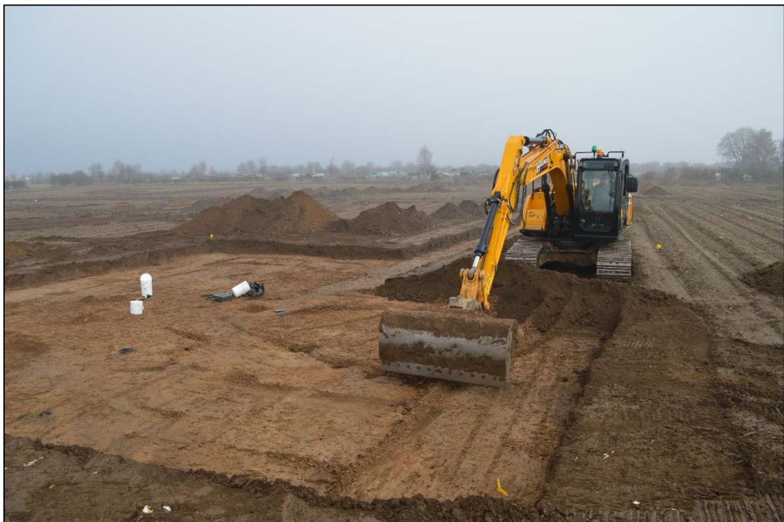
Plate 12. Machining of Area 1 (camera facing north)
