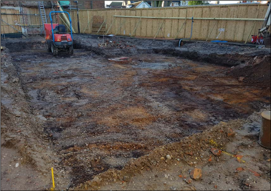
Plate 1. General view of excavated area (camera facing south)
