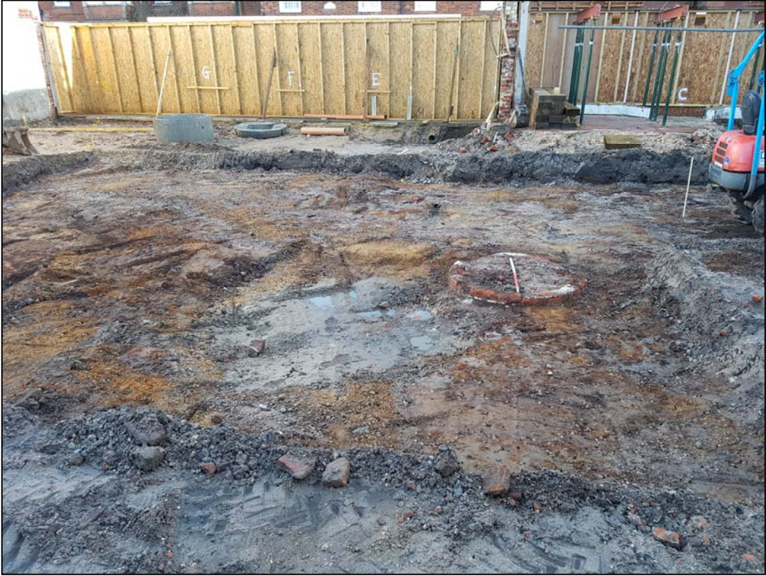
Plate 4. Pit 0004 (foreground) with Well 0003 (middle right; camera facing northeast)
