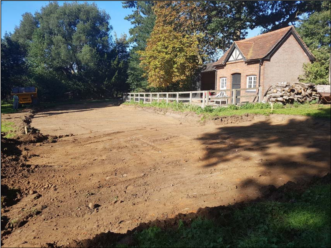
Plate 3. Area of garage and drive (camera facing W)
