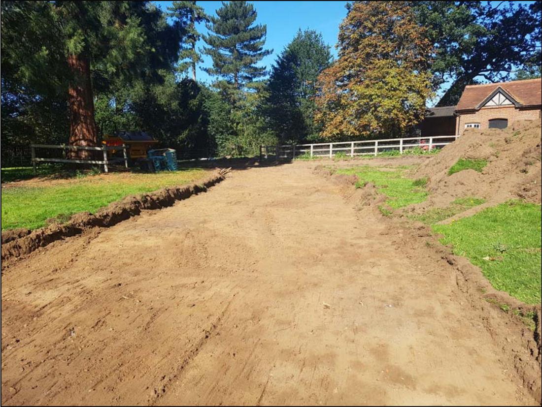
Plate 2. Contractors access between buildings (camera facing N)
