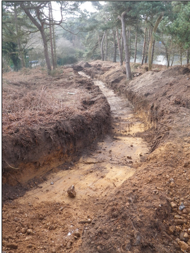
Plate 1. Monitored area facing southwest
