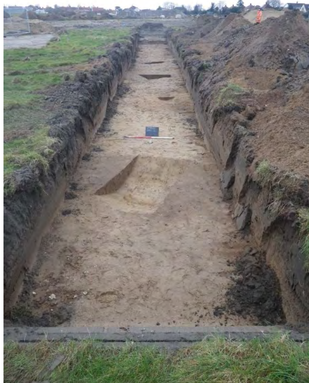
Plate 3. Trench 4, showing typical surface geology and ditches at north end of site
