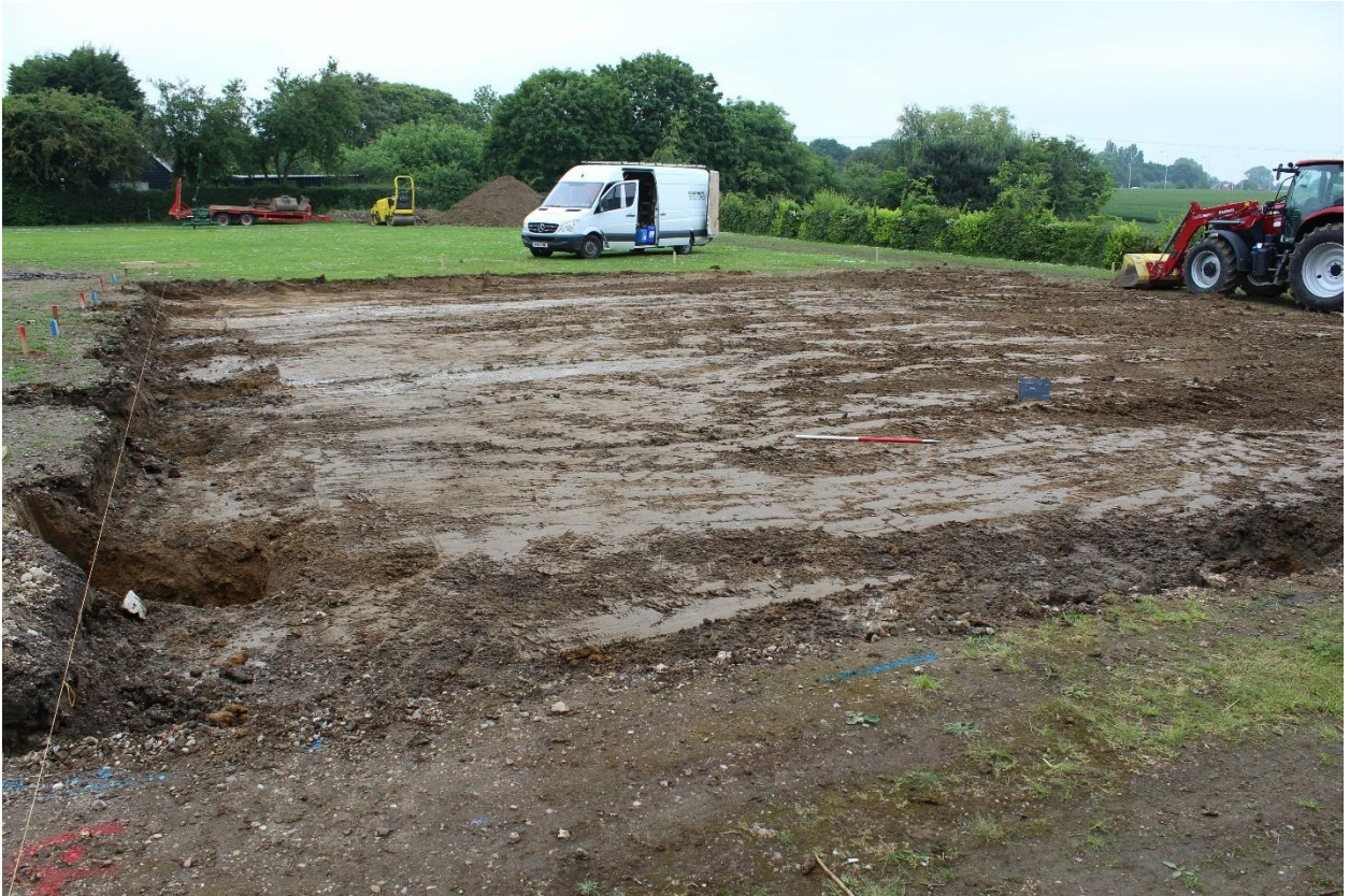
Plate 1: Site levelling, Looking north-east, 1x1m scale
