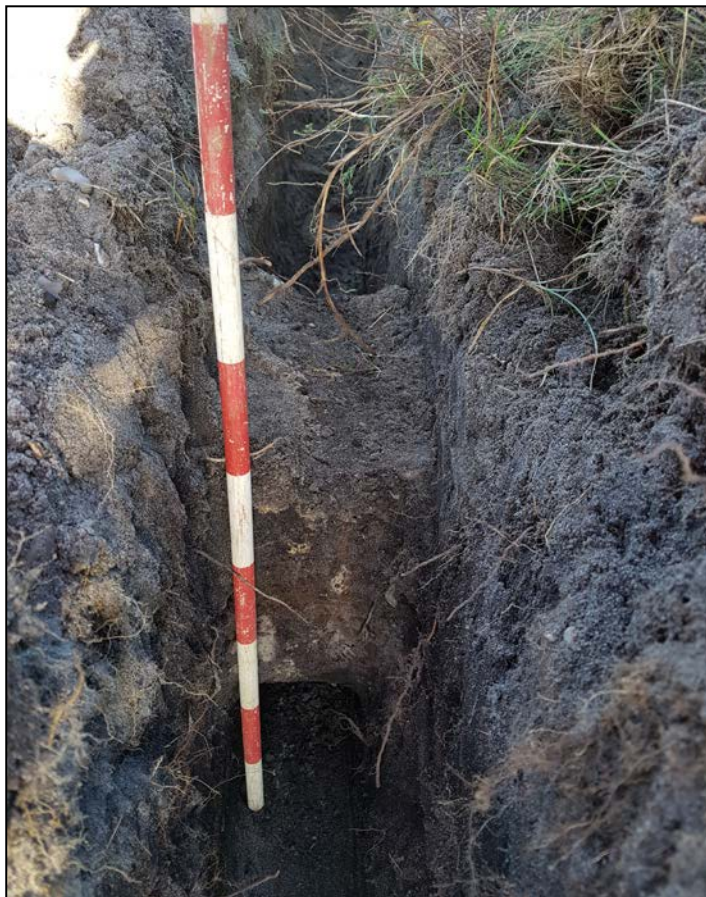
Plate 14. Item F: probable concrete footing, middle of a group of three (camera facing N)
