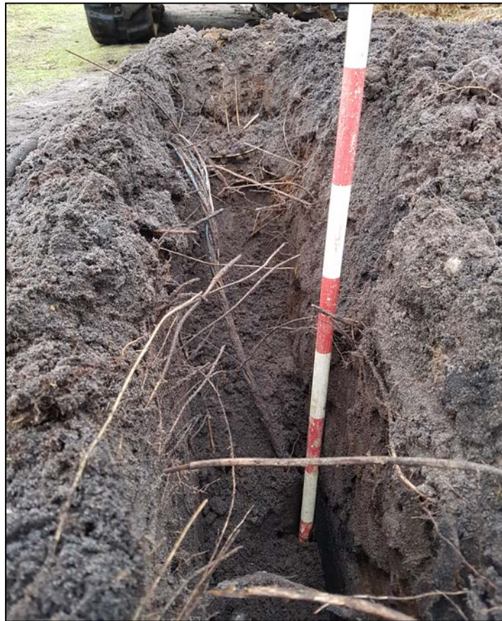
Plate 1. Item A: probable communications cable (camera facing S)
