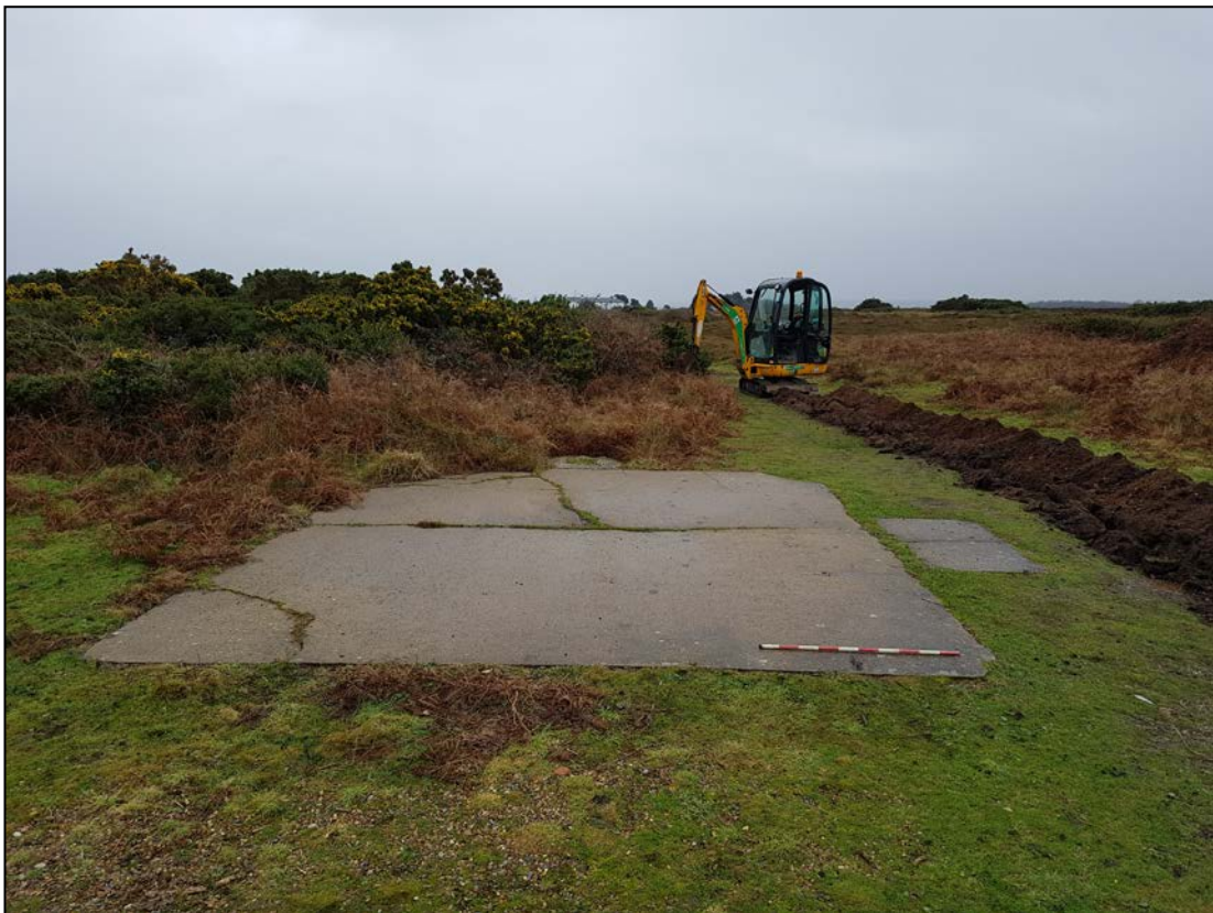
Plate 8. Base of former guard room (camera facing S)
