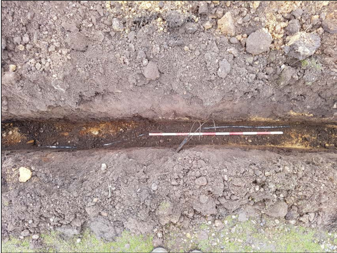
Plate 7. Item D: 'armoured' electrical cable with smaller cable crossing at higher level
