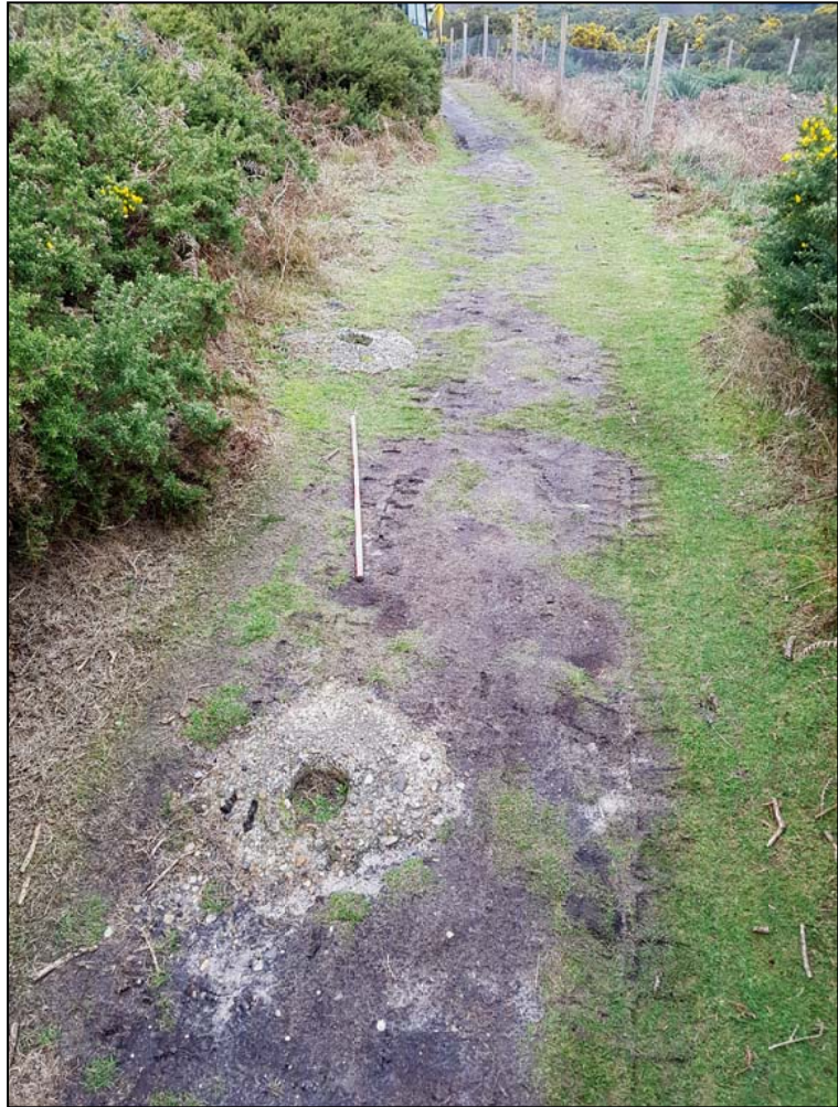
Plate 3. Item B, four concrete 'post settings' (camera facing N)
