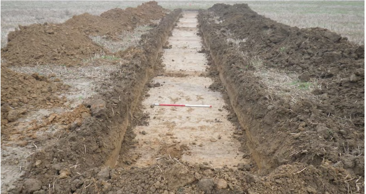
Plate 13. Trench 11, looking east, 1 x 1m scale.
