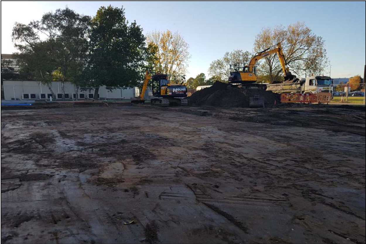
Plate 2. Stripped area close to northwest end of site
