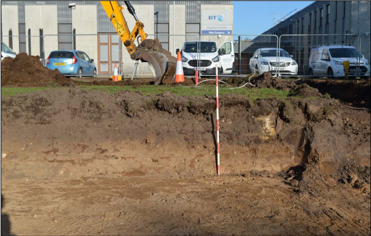
Plate 1. Cross section showing soil depths and construction level at southeast end of site
