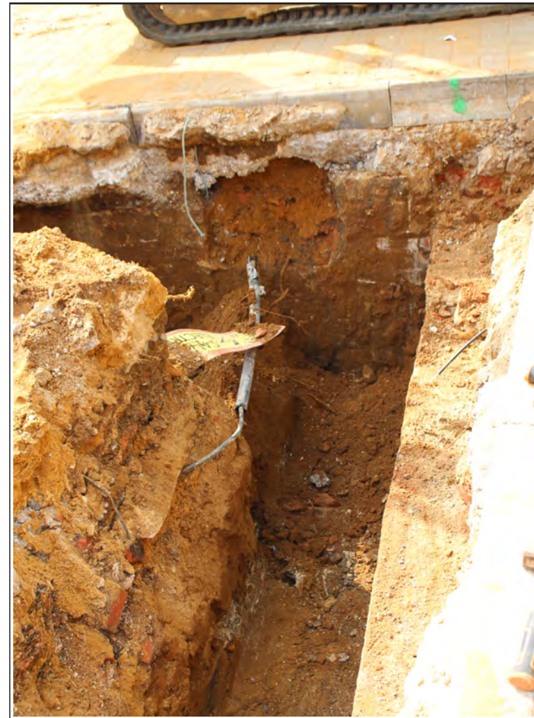
Roadside, western garden retaining wall foundation trench, N-S and E-W modern footings, looking south
