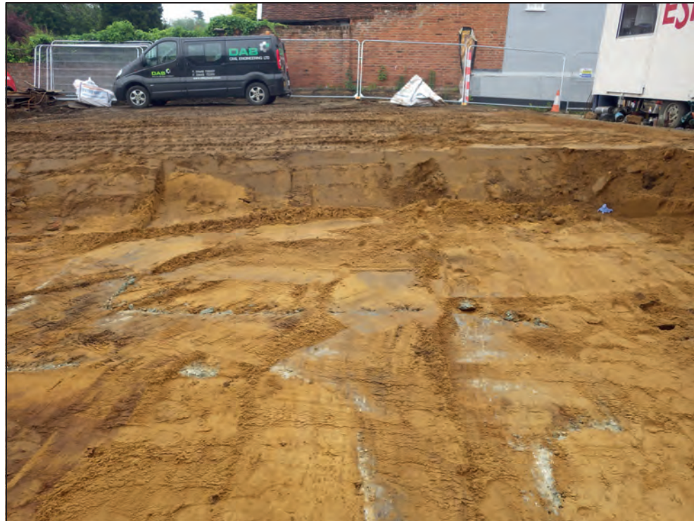
South end of footings, looking east
