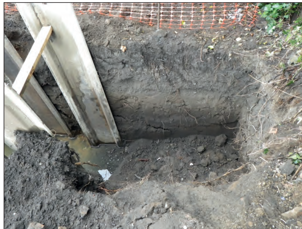
Northern retaining wall showing depth of made ground, looking north
