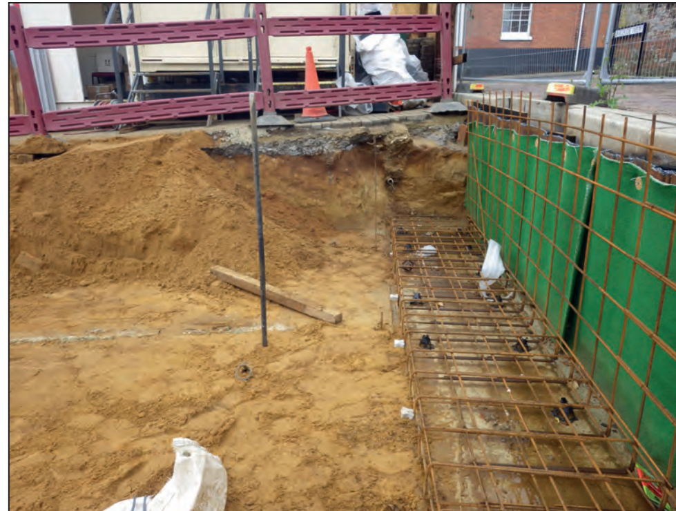
South end of footings, looking south
