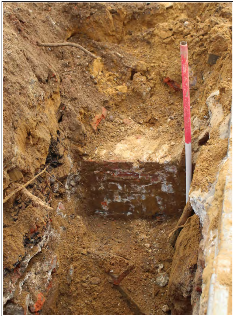
Roadside, southern garden retaining wall foundation trench, N-S modern footings, looking east
