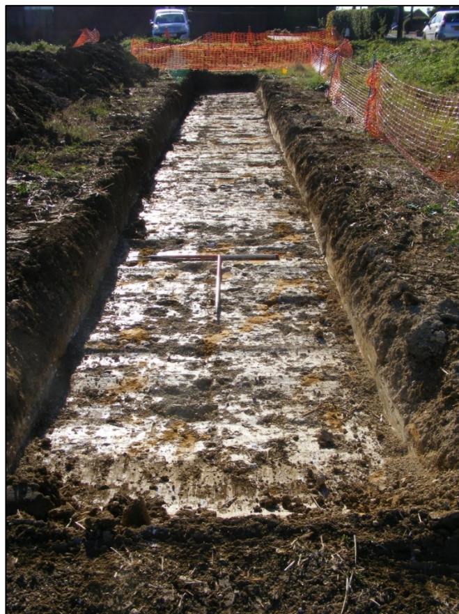
Plate 4. Trench 2, post-excitation, looking northwest (2 x 1m scale)
