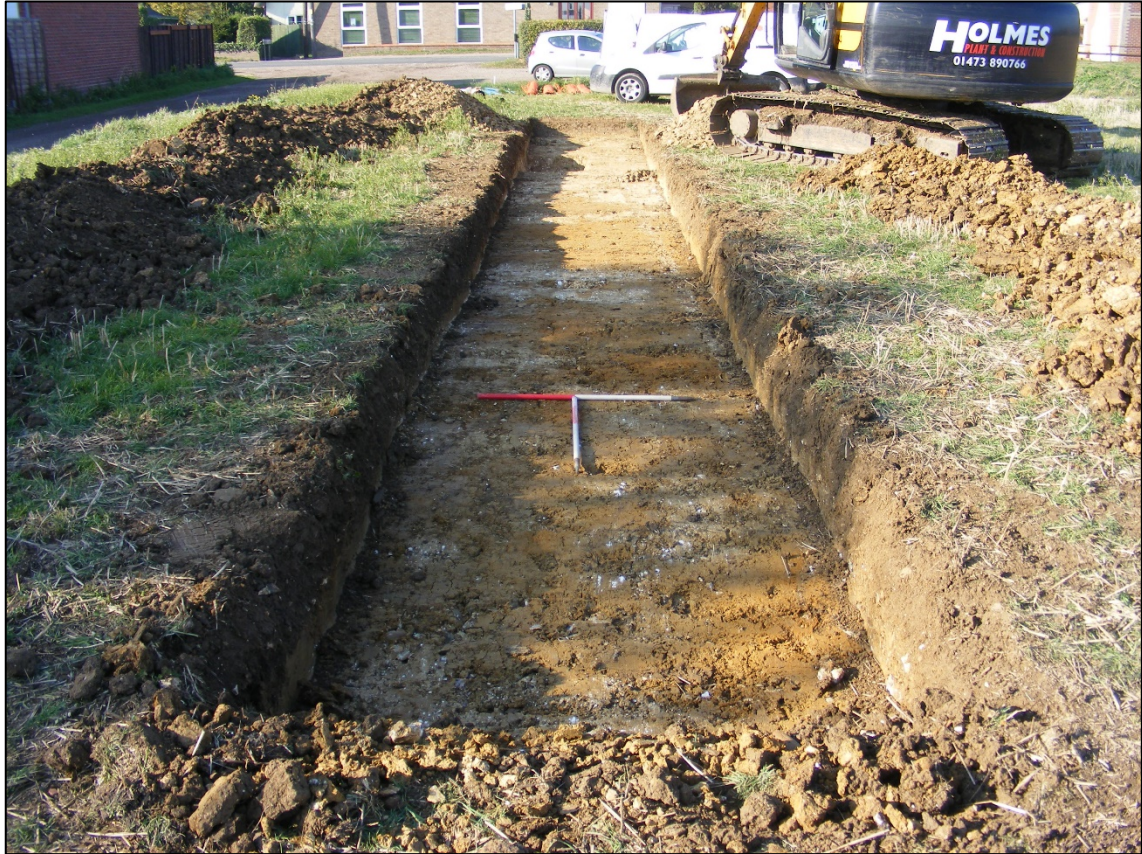
Plate 2. Trench 1, post-excavation, looking northwest (2 x 1m scales)
