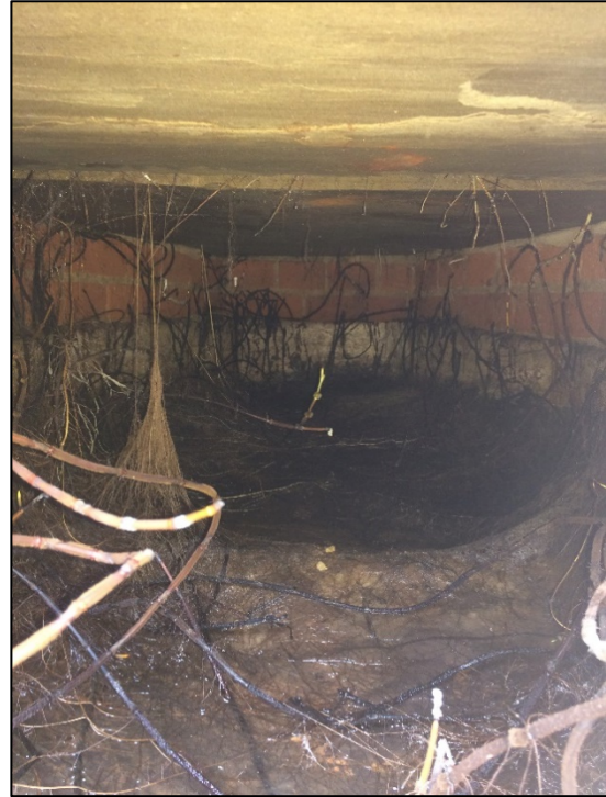
Plate 6. Looking north into brick shaft 0036
