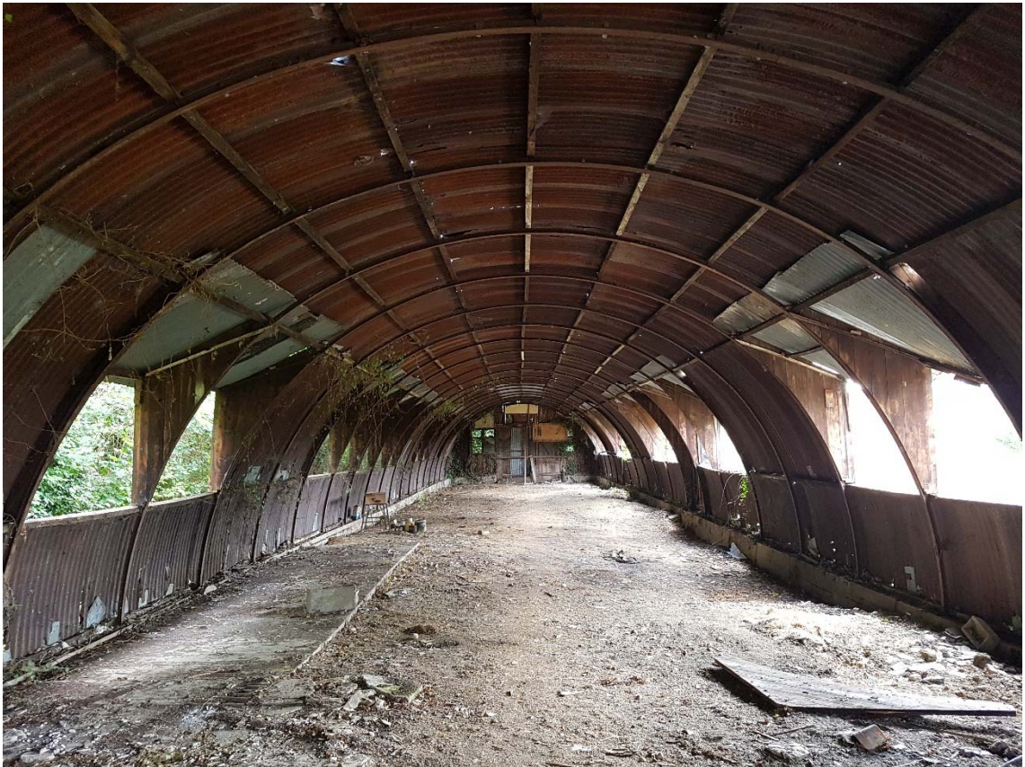
Plate 10. Hut 2, interior view towards southeast end
