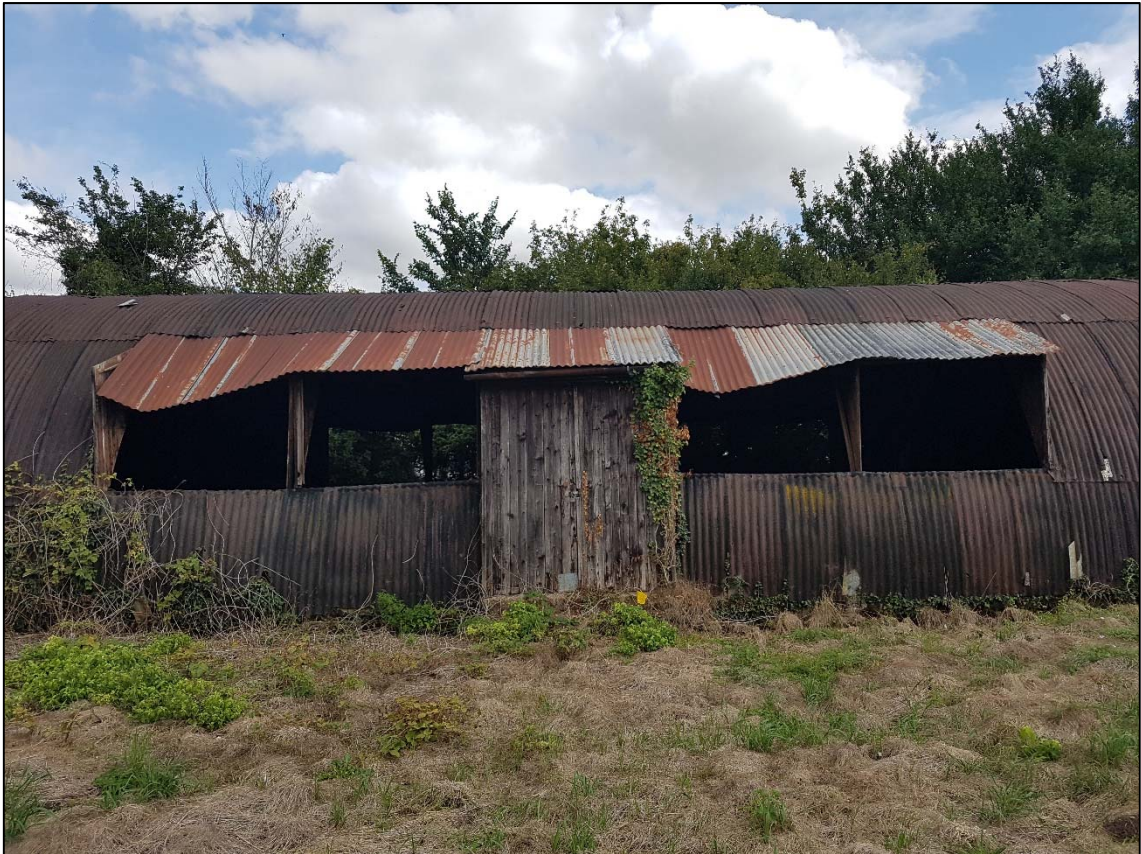
Plate 7. Hut 2 showing double doors on southwest side (camera facing northeast)
