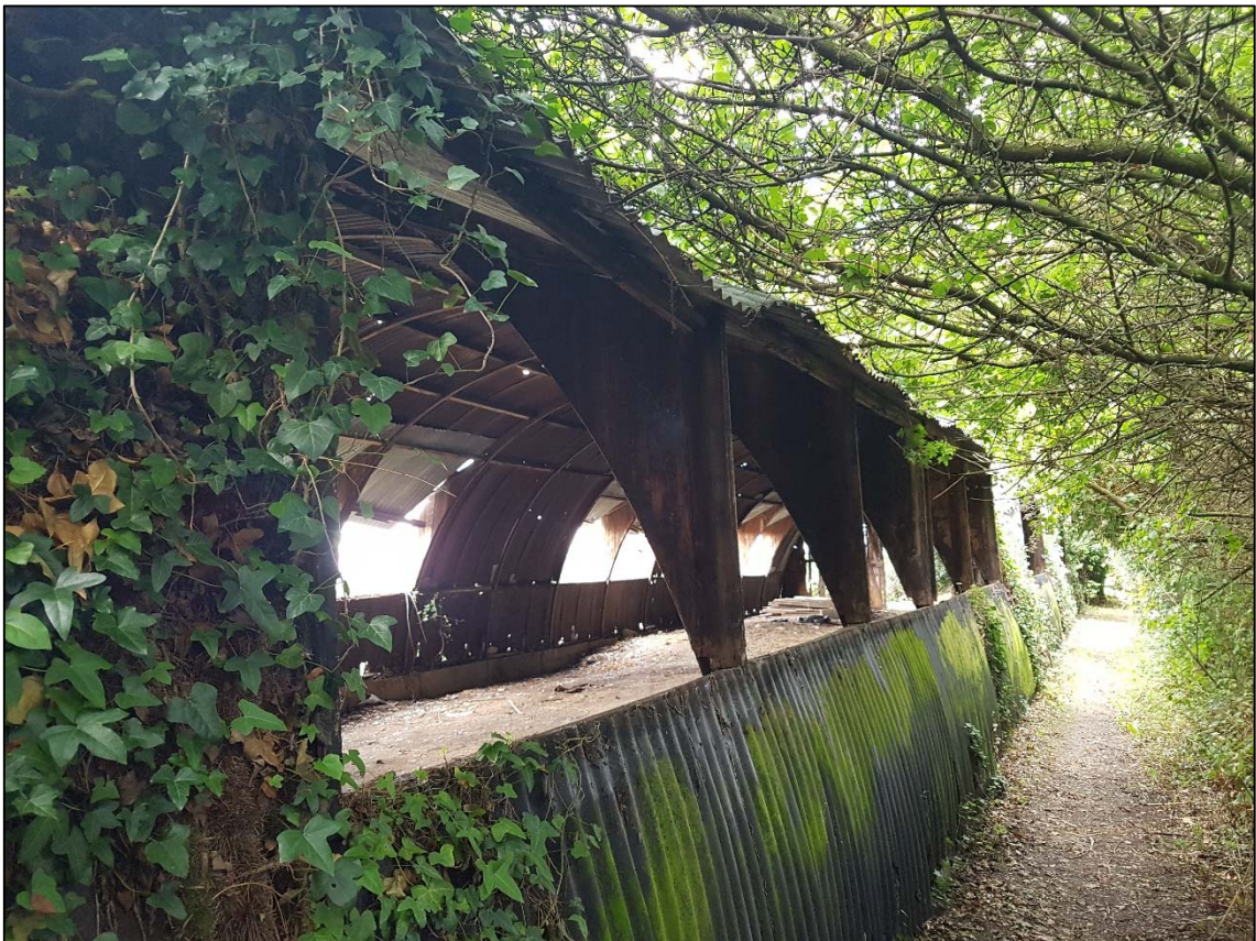
Plate 8. Hut 2 showing multiple window openings on northeast side (camera facing northwest)
