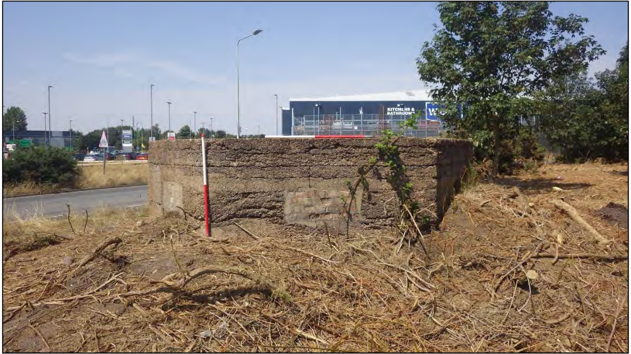
Plate 8: SE facing elevation of pillbox 0020, looking northwest
