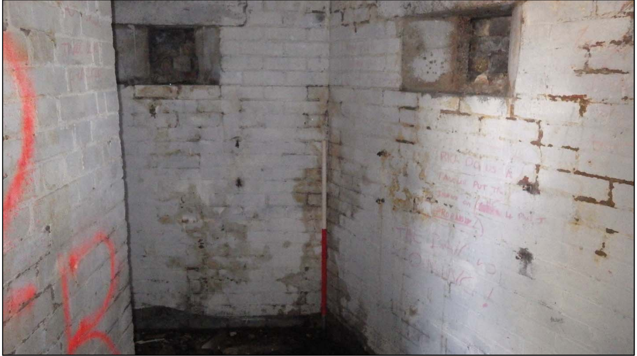
Plate 9: Internal photograph of pillbox 0020, note the original nail fixings either side and below each embrasure
