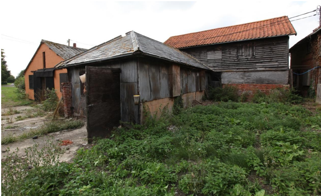
Illus. 16. The animal yard to the south-west of the barn as seen from the south-east with the detached mid-19 th century pantiled loose boxes and granary (5) in the rear and the much altered slate-roofed shelter-shed (6) in the foreground (originally open-sided to the right). The 20 th century covered cattle yard (8) is shown to the left. The narrow passage between the two loose boxes (3b and 5b) lies to the extreme right. This yard was almost certainly designed for cattle rather than horses but no relevant fixtures or fittings survive.
