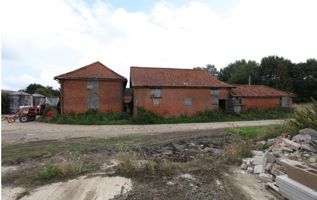
Illus. 3. The buildings from the north-west showing the mid-19 th century extension to the barn (3) on the left which contains a cart shed (3c) entered from the rear (north-east) and a loose box facing the animal yard in front of the barn (3b) along with a first-floor hay loft. The contemporary central structure (5) also contains loose boxes with a granary above, and its slightly later lean-to in the foreground provided additional grain storage with a suspended floor and ventilation arches beneath. The single storied right-hand shed (7) is a shelter-shed serving a yard in the rear (8).
