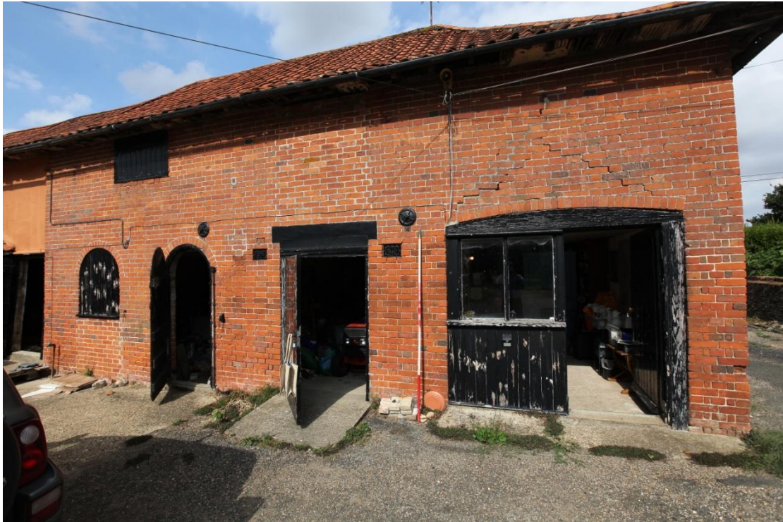
Illus. 13. The south-western facade of the coach house (2) built in the mid-19 th century as an extension to the barn. The right-hand doors opened into a vehicle shed (2a) and the large central door into a stable which retains a manger backing onto a chaff box connected by two hatches (2b). The original loading door to the first-floor granary lay above this door but has been blocked. The arched window and door to the left originated unusually as a pair of doors but appear to have opened into a single space that probably served as a tack room (2c).
