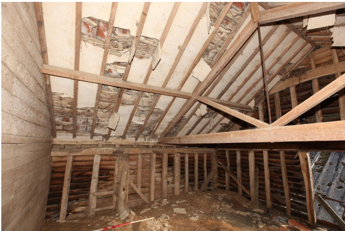
Illus. 18. The south-western compartment of the first-floor granary (5a) seen from the north-west with the gable loading hatch on the right (and the corrugated asbestos roof of the 20 th century cattle yard beyond). Note the crudely hewn inverted knee-brace supporting the floor and the original softwood roof with a vertical iron tie-rod – typical of the 1860s and 70s. The original plaster between the rafters is secured by reeds and laths and the boarded wall on the left adjoins the identical north-eastern compartment.
