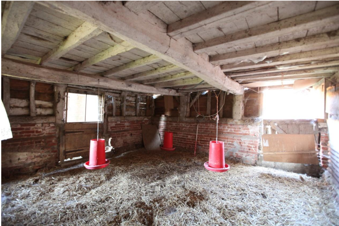
Illus. 17. The interior from the west of the north-eastern ground-floor loose box of the granary (5b) showing its re-used ceiling of partly tenoned and partly lodged joists with a hay drop to the left of the right-hand door (which opens onto the yard shown in A2.16).
