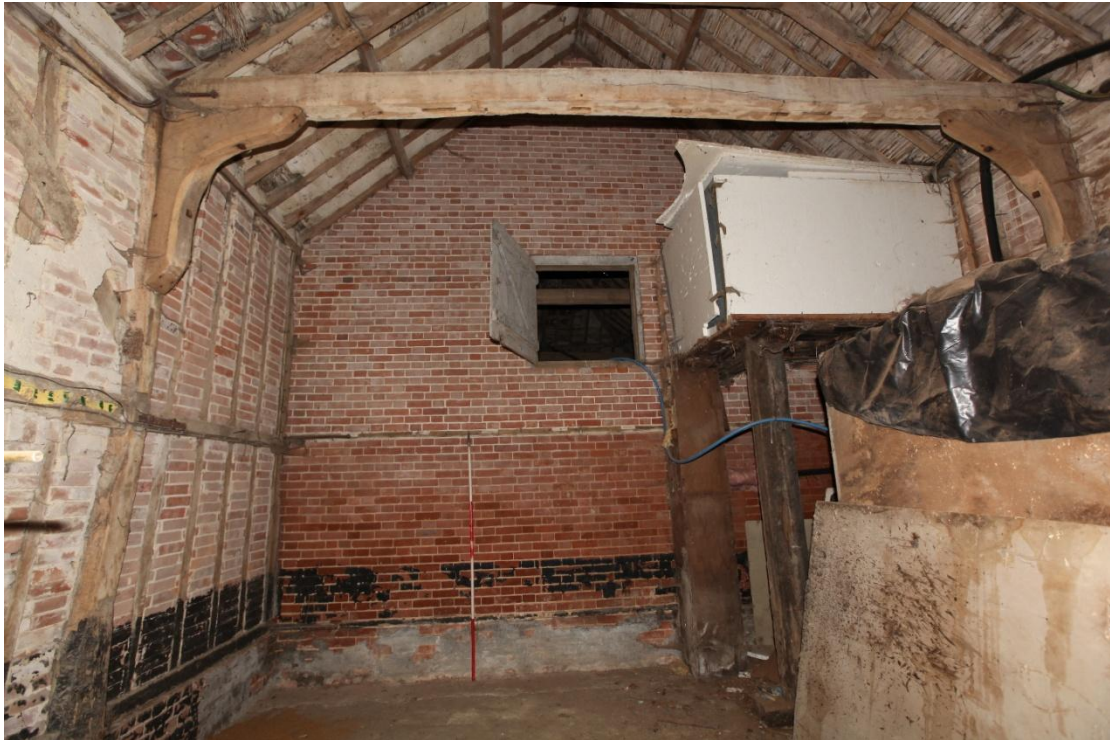
Illus. 7. The original north-western gable of the barn from its final bay (1d) showing empty mortises for a missing solid wall in its tie-beam – which is the only timber now in situ . The first-floor hatch opens into the hay loft of the brick extension shown in A2. 15.
