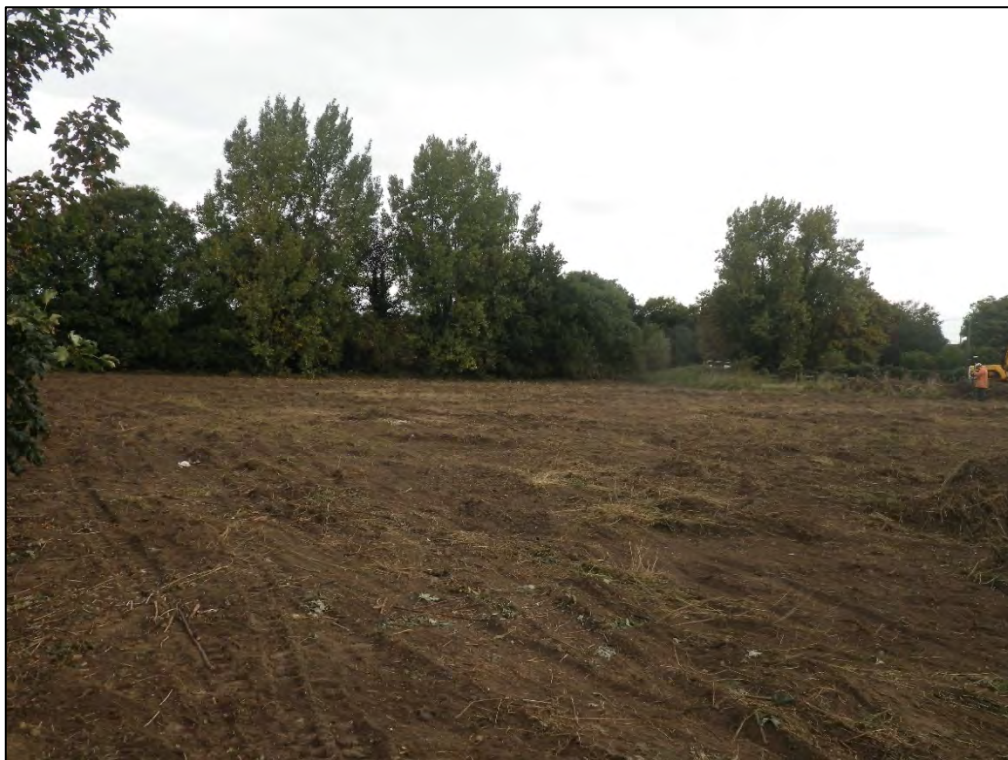
Plate 1. Site topography prior to excavation, looking NE.
