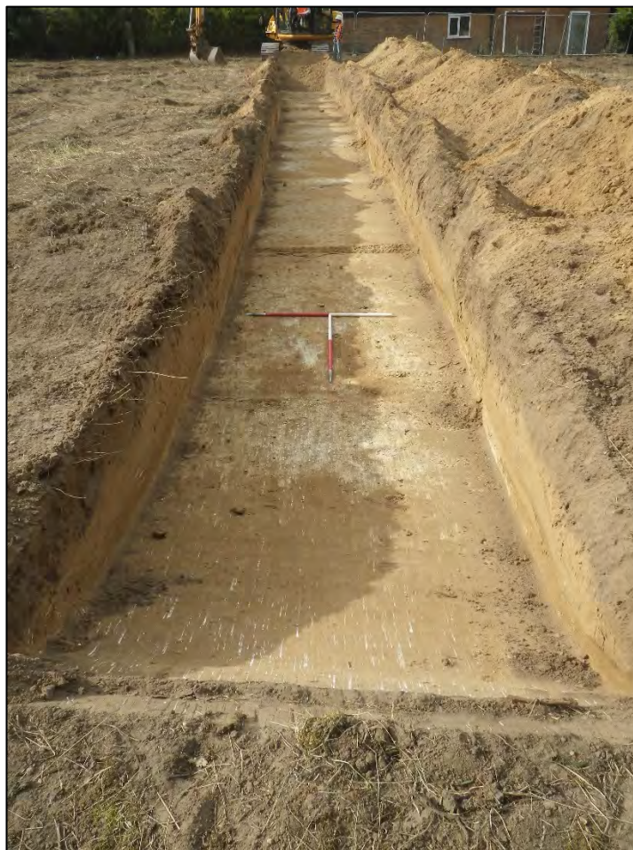
Plate 6. Trench 4, looking SE
