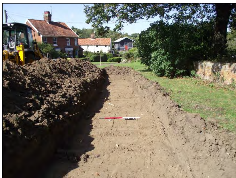
Plate 7. Excavated area recorded during watching brief, Peasenhall, looking north-north-west
