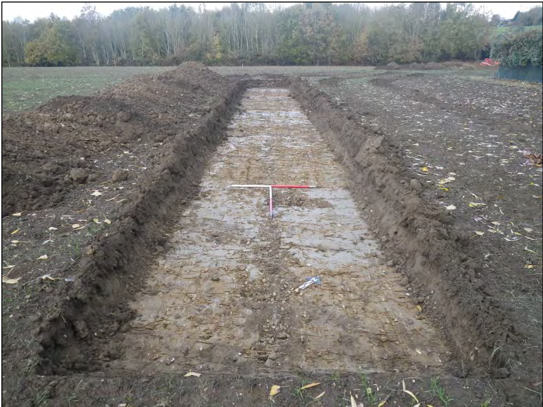
Plate 6. Trench 3, Saxmundham, looking north-west
