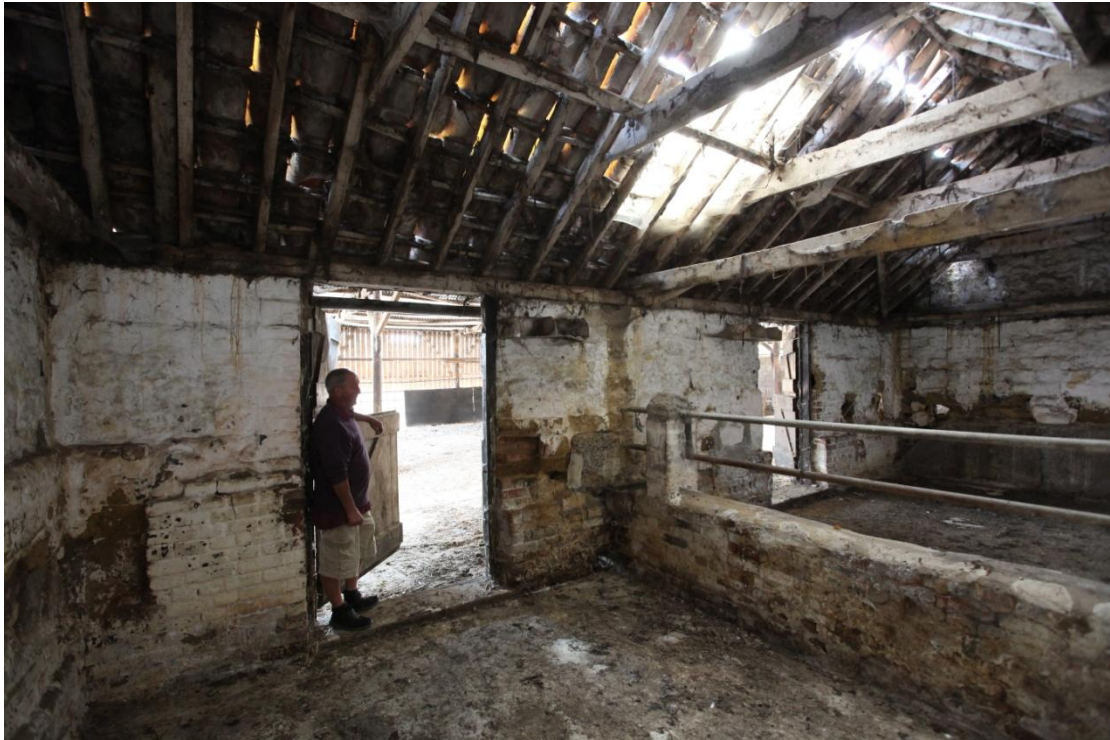
Illus. 11. The eastern internal wall of the loose box (2b) showing its whitewashed clay-lump with the scar of its probably original clay-lump internal partition in the centre. Only the brick plinth of this partition now survives. Mr Glyn Thomas and his father have operated a dairy farm here since the 1960s.
