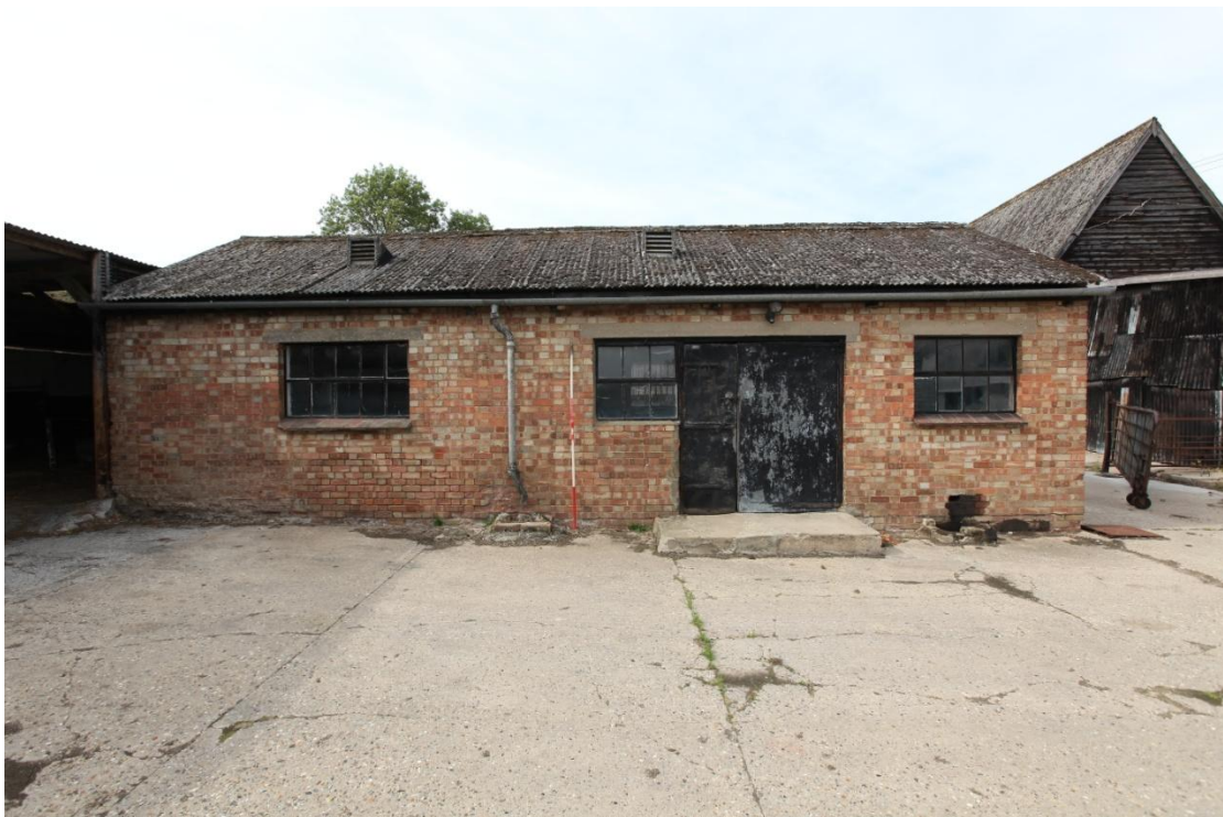
Illus. 18. The eastern facade of the 1950s Fletton-brick milking parlour (6) showing the steel entrance doors to its central compartment with the threshing barn on the right. The milking equipment from this building is now at the Museum of East Anglian Life.
