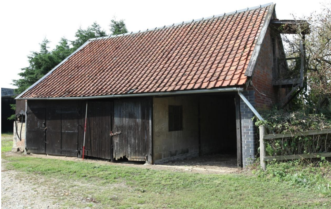
Illus. 17. The eastern facade of the pantiled late-19th century cart lodge adjoining the site entrance (5). This three-bay building was formerly open-fronted with a grain loft in its northern bay reached by an external stair against the gable to the right. The present internal partition dates only from the 20 th century with original boarding above. Note the glazed and curved bricks to both piers in typical late-19 th century fashion. This structure may well date from 1899 as suggested by a boldly cut internal inscription.
