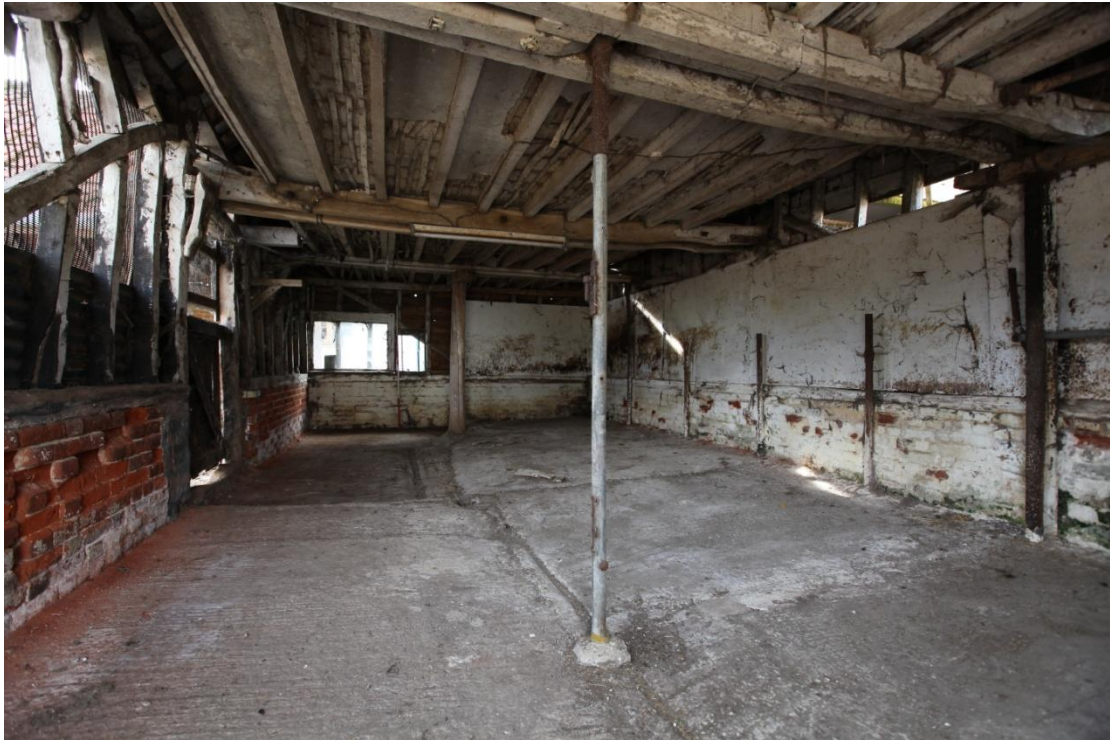
Illus. 13. The interior of the stable (3) from the north. This space has been used for cattle in recent years but a section of original brick floor with an axial drain survives in the rear to the left with the remains of a chaff box on the right. The ceiling joists retain original plaster secured by laths nailed to the loft boards and are tenoned to the principal joists – but the latter are sandwiched between later bolted reinforcing rails.
