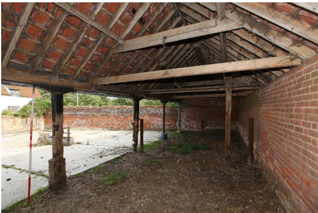
Illus. 16. The interior from the west of the stable's shelter-shed (4) showing its original arcade posts and softwood clasped-purlin roof with nailed collars. The eastern gable in the rear was built against the earlier brick wall of the horse yard on the left.
