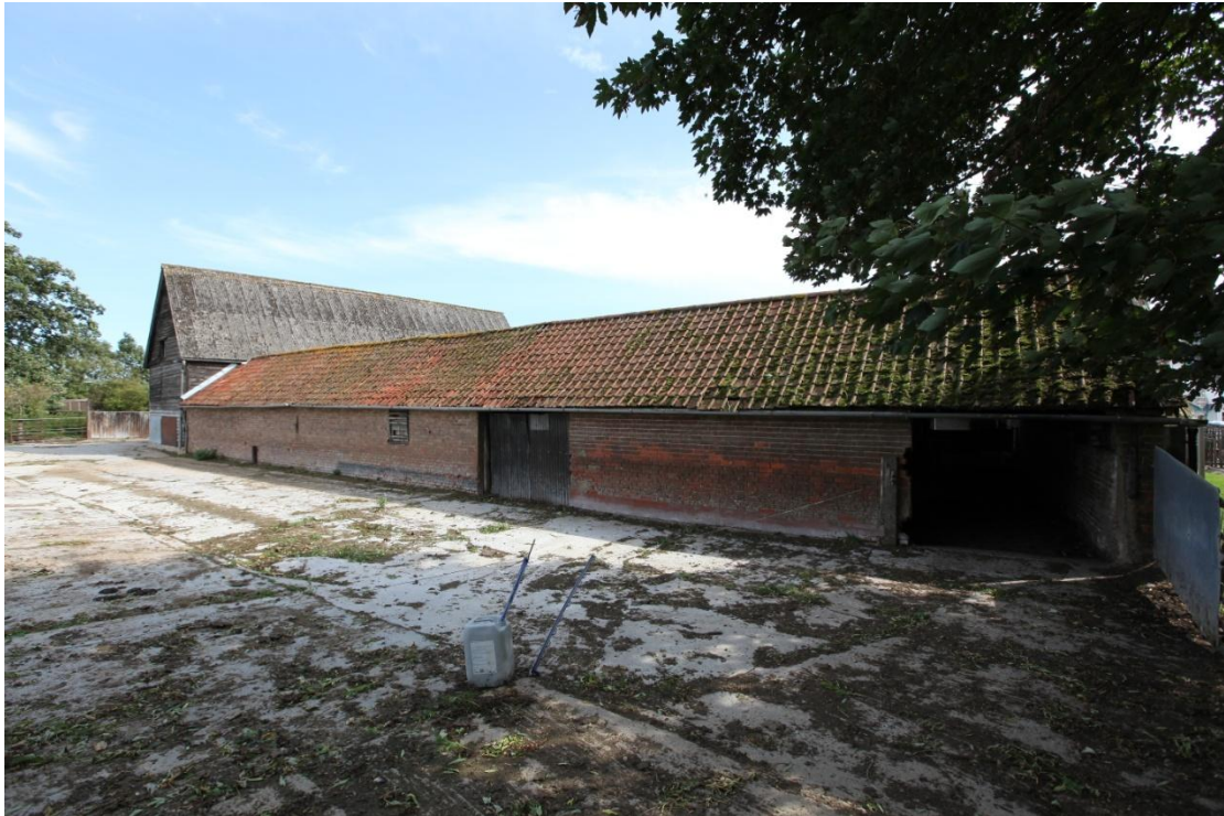
Illus. 9. The barn and the mid-19 th century shelter-shed (2) from the cattle assembly yard showing the latter's two inserted doorways. The central doorway divides original 19 th century red brick on the right from the wall of the central loose box (2b) and northern shelter-shed (2a) that was rebuilt in Fletton brick in the 20 th century.
