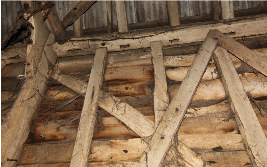
Illus. 7. A detail of the barn's southern wall (in the penultimate eastern bay to the left in A2. 6) showing the empty mortises and 16 th century style edge-halved and bridled scarf joint in the roof plate above. The inverted V braces on the right are 20 th century additions but the trenched external braces are original to the fabric. These are highly unusual in a 19 th century barn and have also been re-used; they are now lapped and nailed to the studs but terminate in pegged tenons from their former lives.
