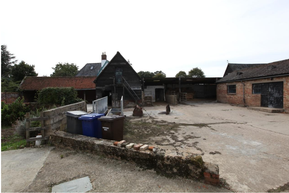
Illus. 3. The southern range of farm buildings seen from the house to the north showing the 1950s Fletton-brick milking parlour (6) on the right and the stable (3) in the centre with the shelter-shed of a horse yard adjoining on the left (4). The external stair to the granary above the stable is an early-20 th century replacement but retains the traditional narrow steps intended to help labourers carrying heavy sacks.
