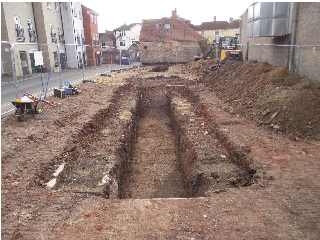
Plate 1. View of Trench 2, looking south towards Gainsborough's House Museum, (the straight-sided feature 0004 can be seen in the foreground).
