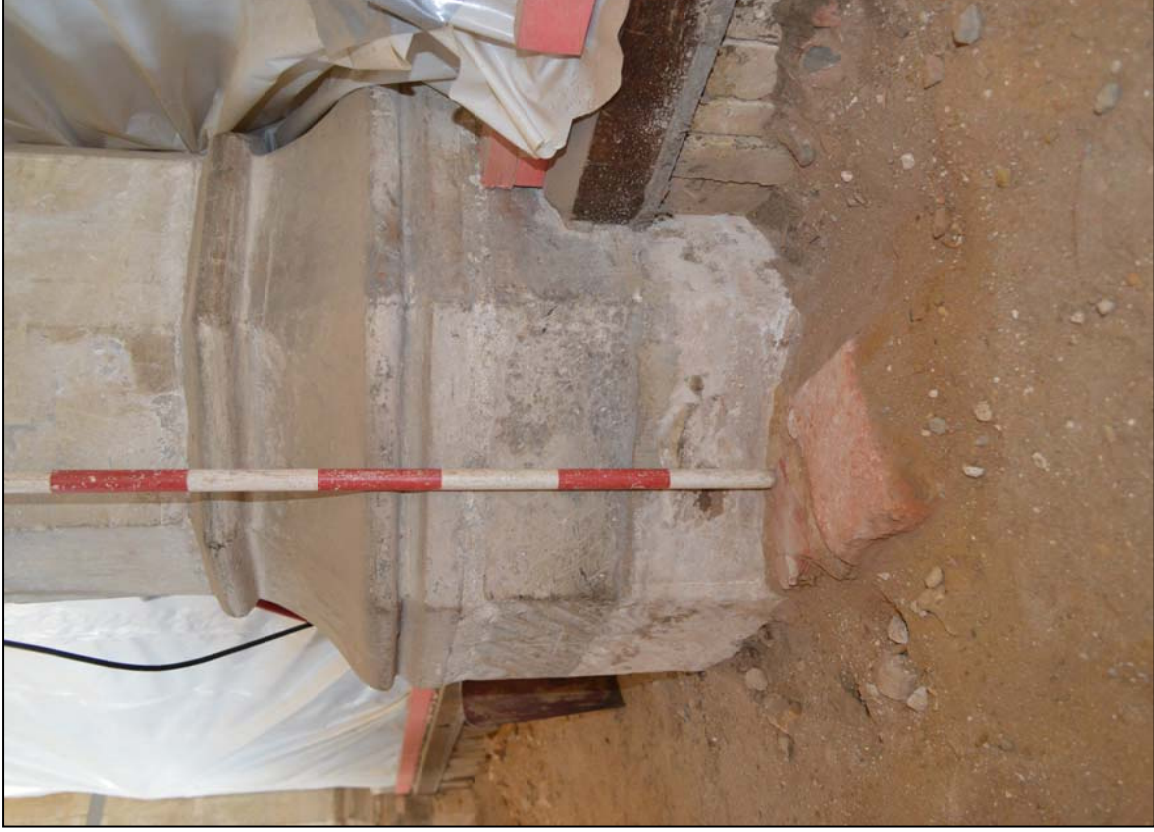
Plate 11. Surviving brick floor (0024), south aisle, camera facing NW
