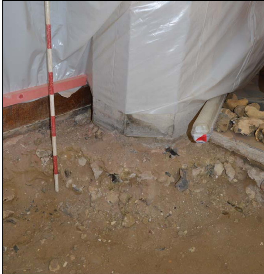
Plate 8. Flint and mortar foundation (0007), camera facing northeast
