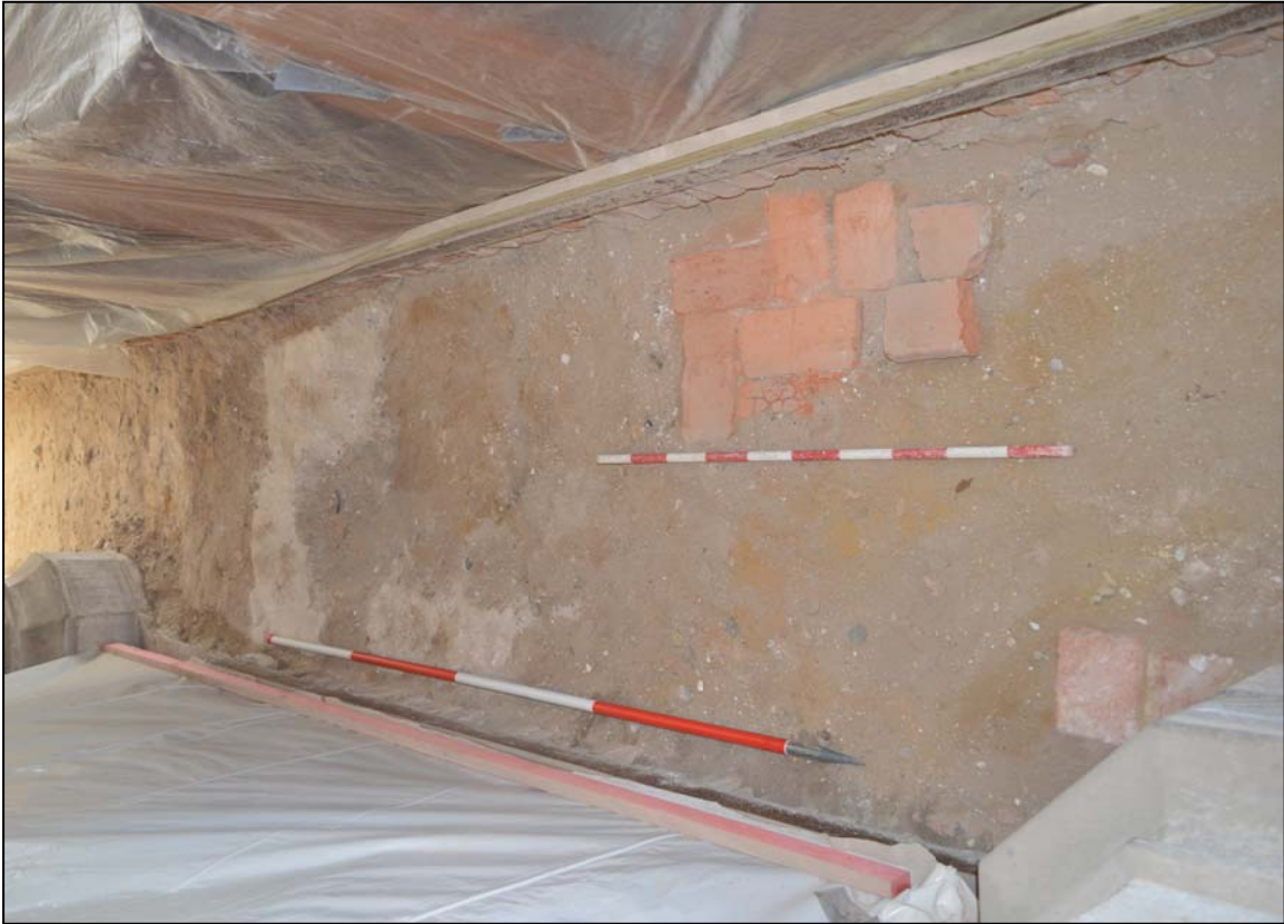
Plate 10. Surviving brick floor (0024), south aisle, camera facing east
