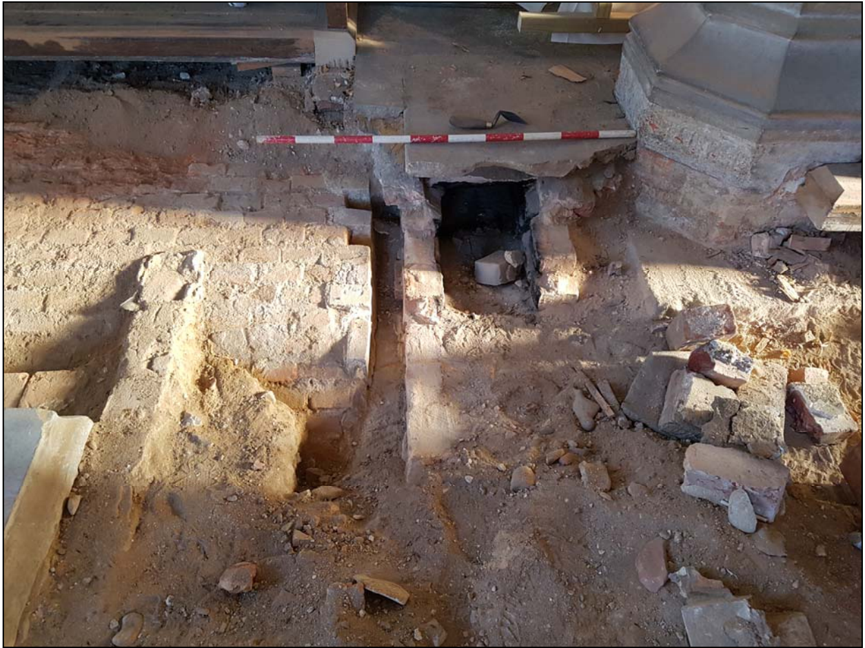
Plate 26. Repair to vault 0028 after insertion of heating duct to the right, camera facing east
