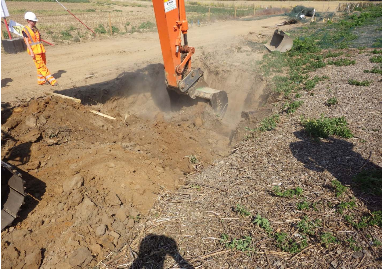
Plate 5. Sett C during works, looking south-west
