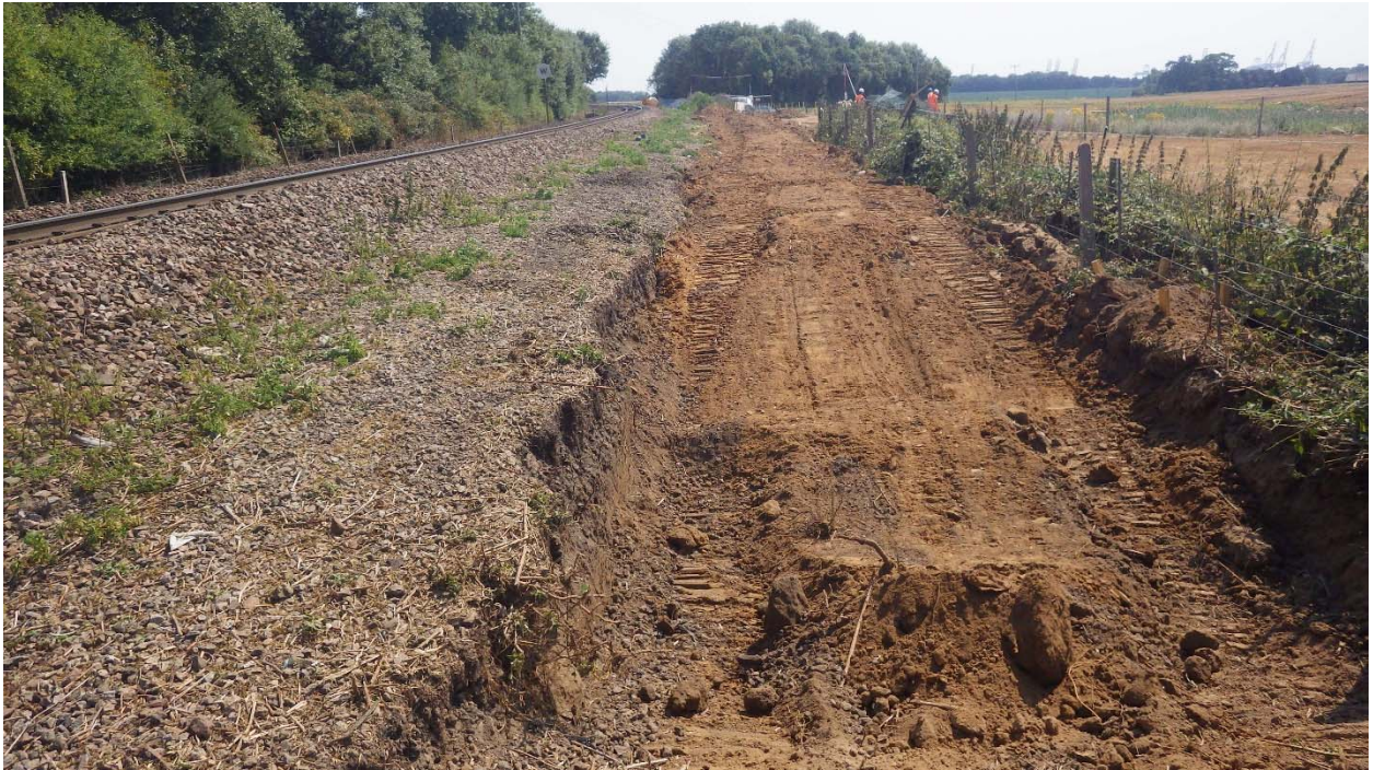
Plate 6. Sett C completed, looking east
