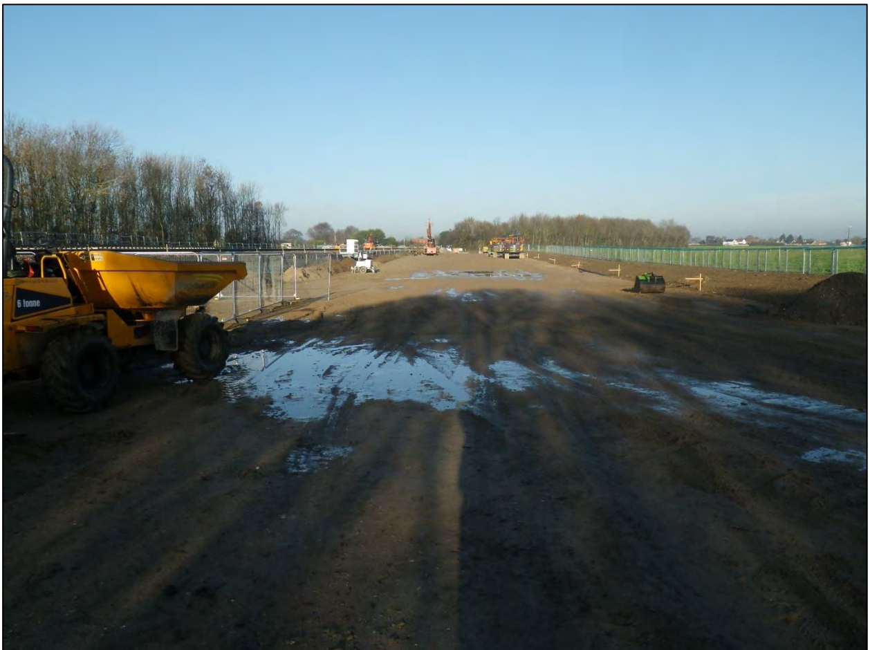
Plate 1. Concrete crush on site, looking north-west
