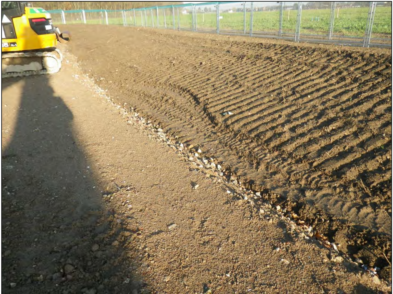
Plate 2. Concrete crush, showing topsoil windrow, looking north
