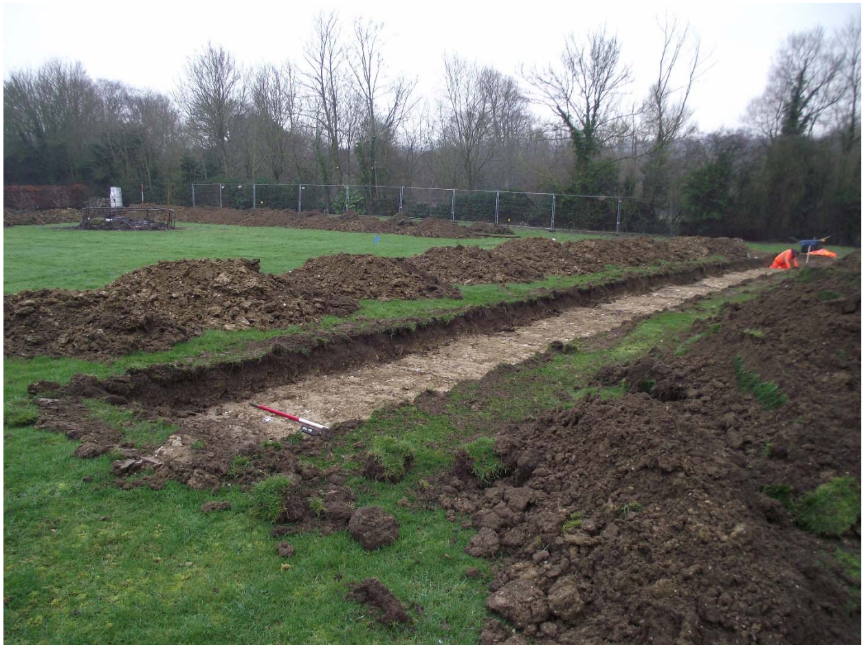
Plate 3. View from Trench 1 looking south across site.
