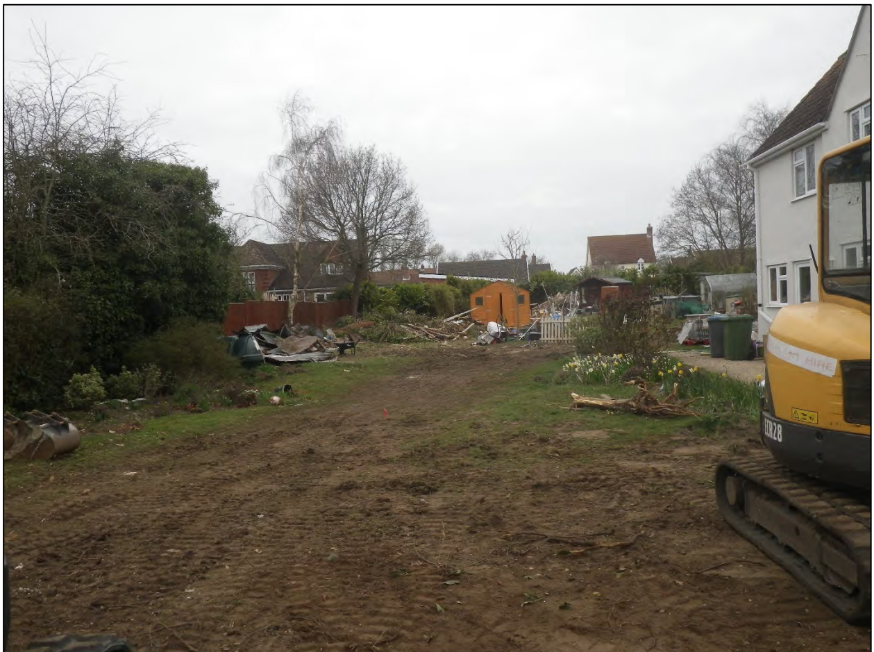
Plate 1. The site prior to the excavation of the two trial trenches
