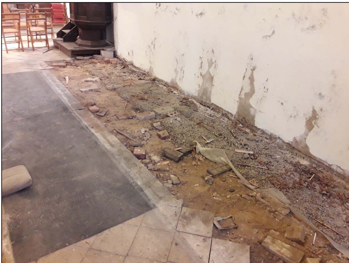
Plate 2. Area C prior to ground level reduction, showing concrete layer against the south wall of the church and ledger slabs set in the nave floor. Looking SE.
