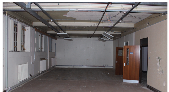
View of 1970s office in eastern portion of ground floor
