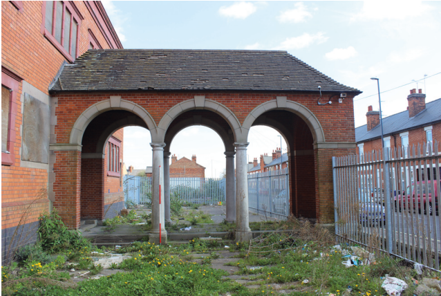
View of 1928 Loggia from south
