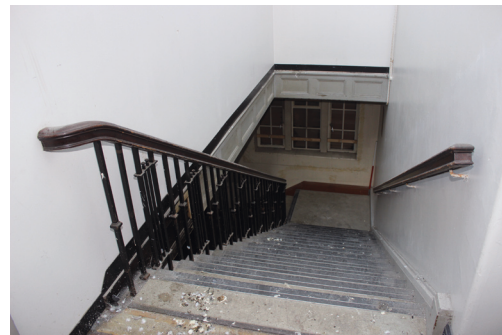
View of first floor infill/extension to 1912 stair
