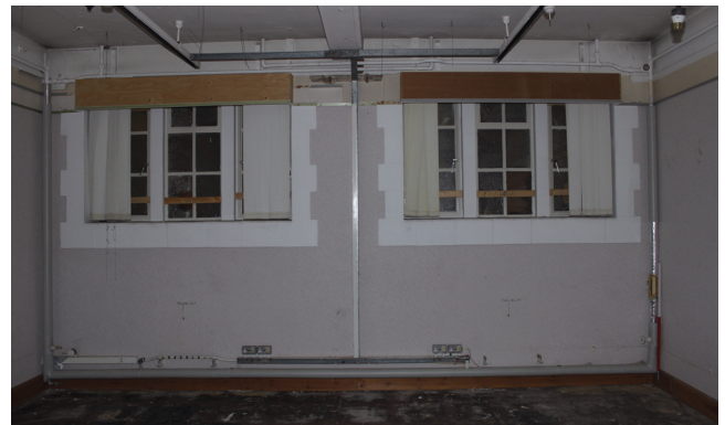
View of ground floor room in east portion of north wing
