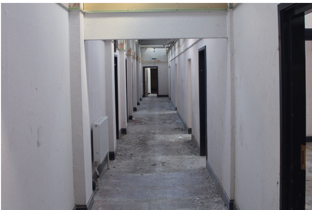
View of first floor corridor in north wing
