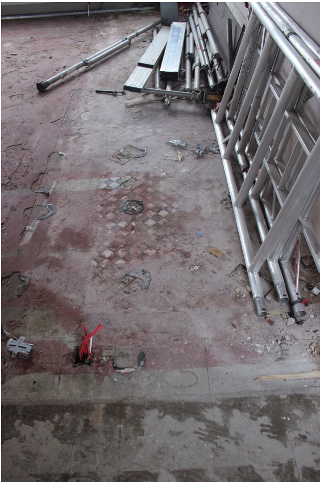
Tiled floor on the first floor adjacent to the north stair
