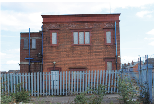
View of south elevation
