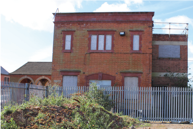
View of north elevation
