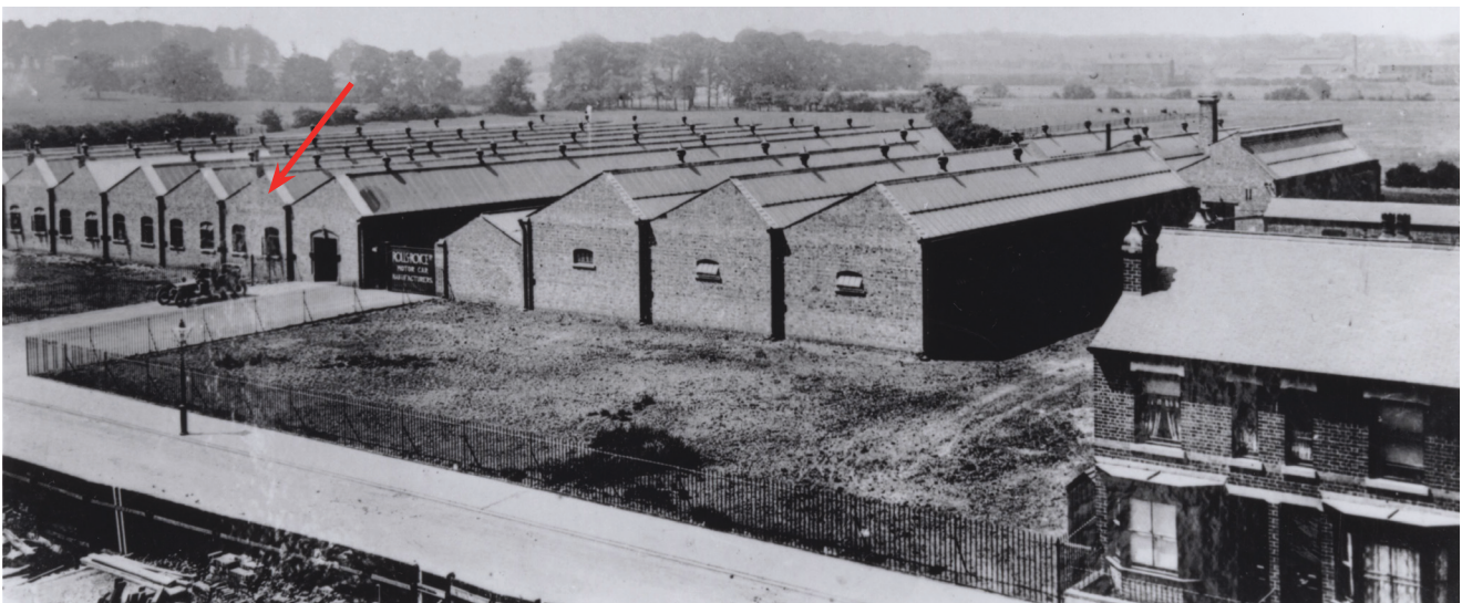
The factory photographed in 1908 with Nightingale Road in the foreground. The location of the remains of the gable wall are highlighted. (Courtesy Sir Henry Royce Memorial Foundation)
