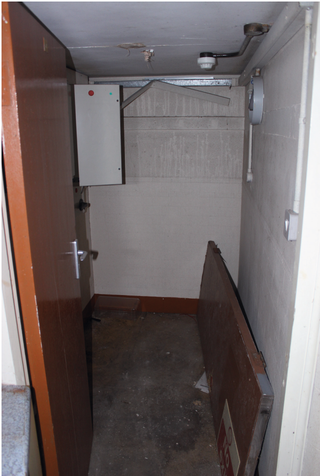
View of second floor cupboard
