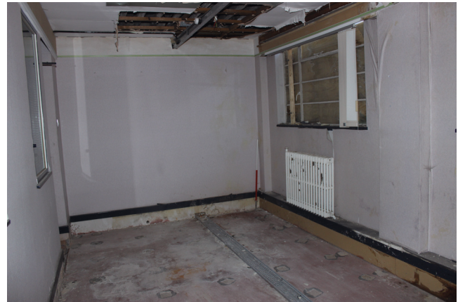
View of office in west portion of building; 1960s/1970s construction
