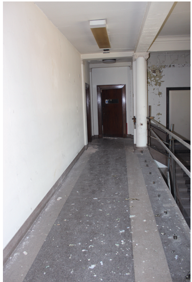
View of first floor landing
