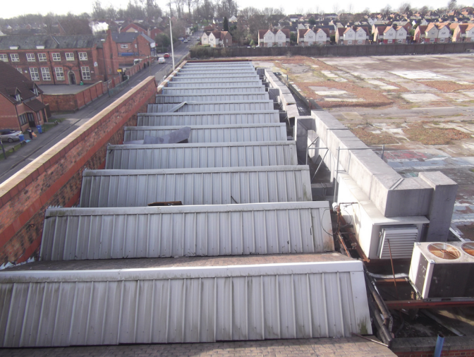
View of roof over south wing, photograph taken in 2013
