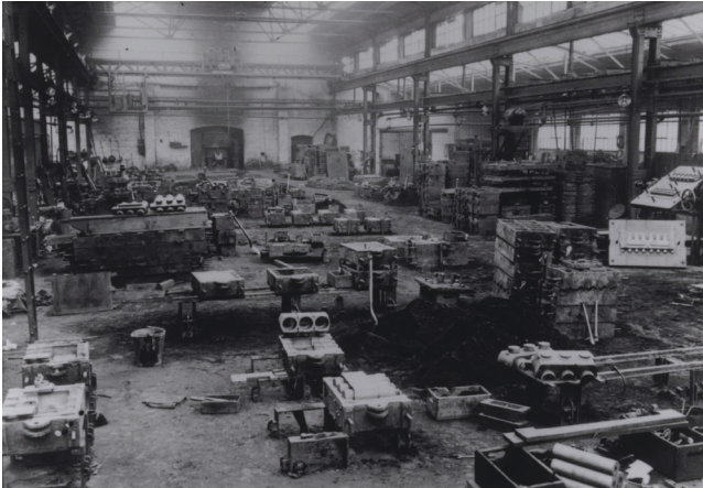
The foundry in the main works, c.1913. (Courtesy Sir Henry Royce Memorial Foundation)
