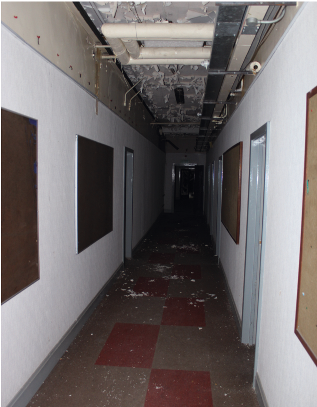
View of ground floor central corridor in north wing
