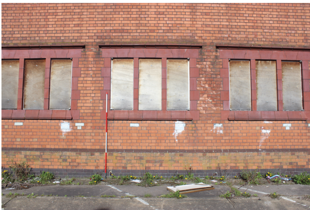
Detail of east elevation, 1912 masonry and windows
