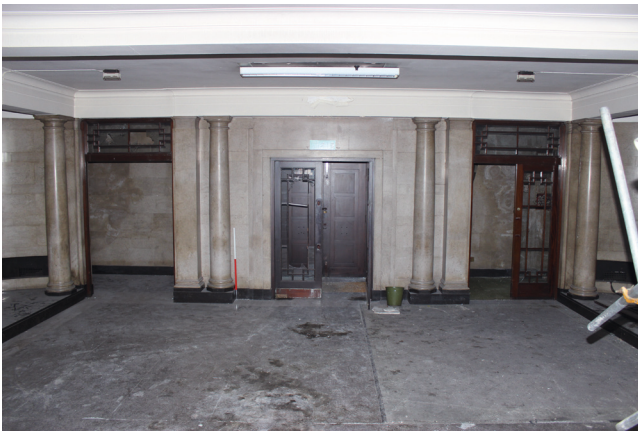
View of entrance to the main hall, flanked by entrances to ante-rooms
