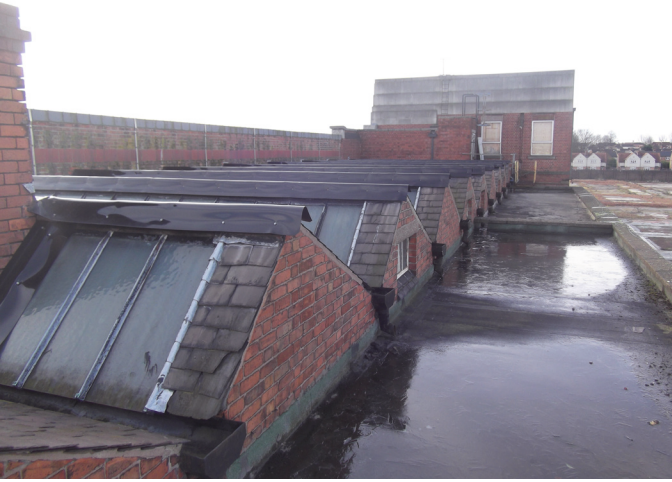
View of roof over north wing, photograph taken in 2013
