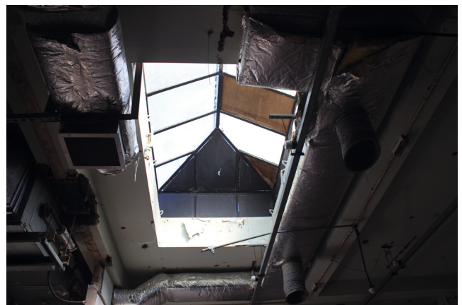
View of second floor roof lantern
