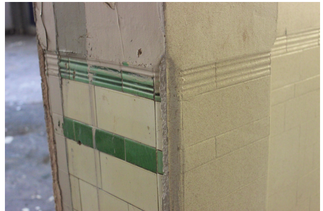
Detail of stair tiles
