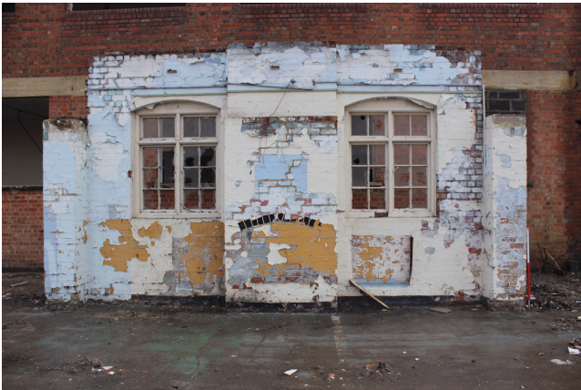
General view of gable remains from west
