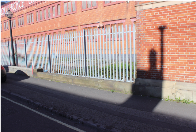
View of reused railing footings from loggia
