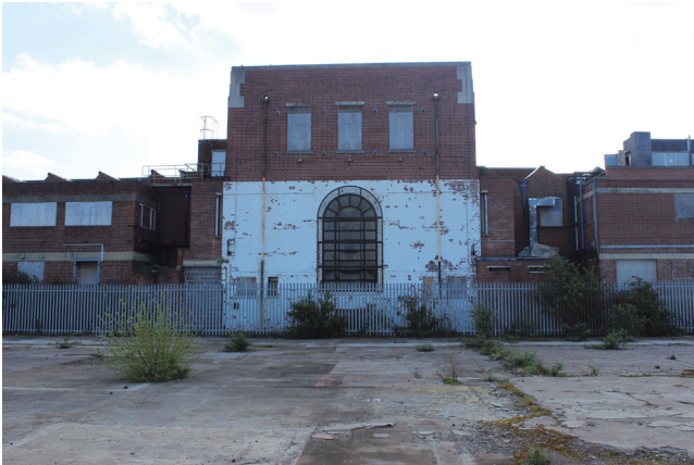
View of central block of west elevation
