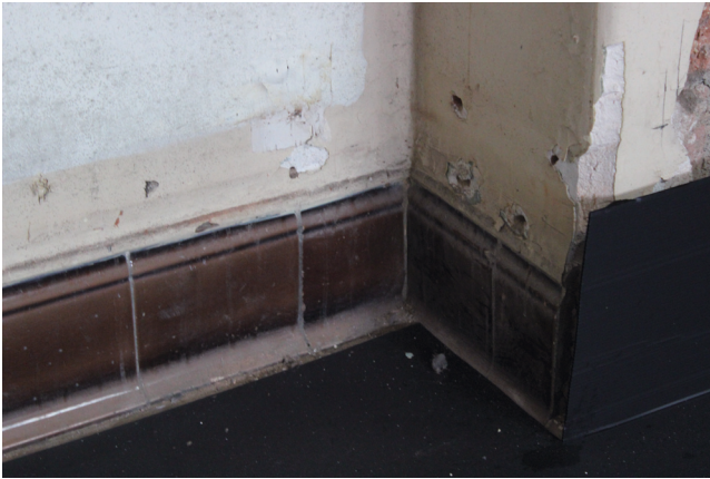
Detail of skirting tile
