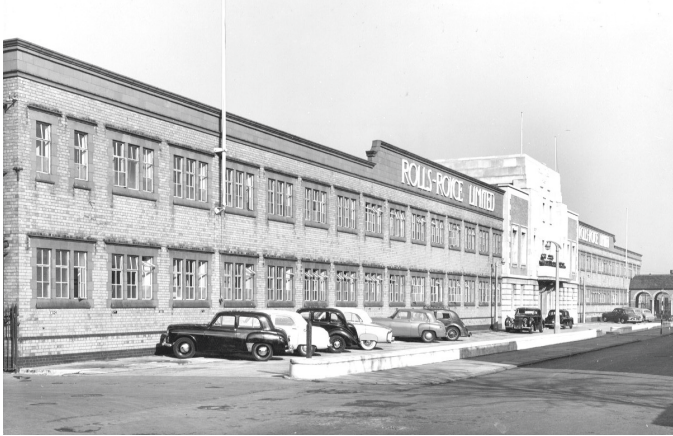
View of Marble Hall, 1950s (Courtesy Rolls-Royce Heritage Trust)
