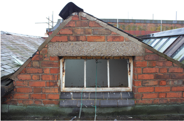
Detail of window in gable of saw-tooth profile roof
