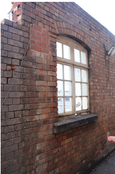
View of east side of gable wall
