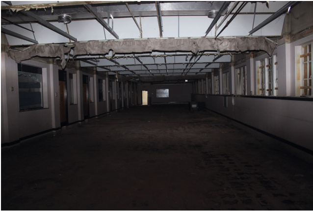
View of first floor east side of building
