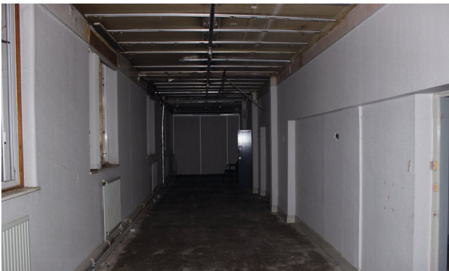
View of ground floor room in west portion of north wing
