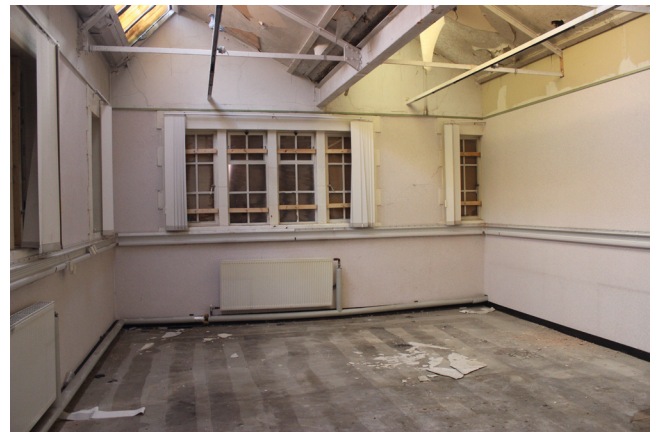
View of first floor room on east side of corridor
