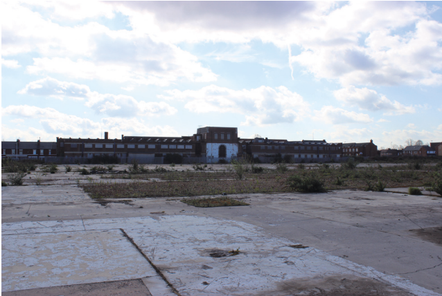
View of west elevation
