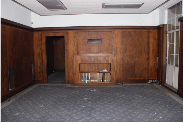
View of south panelled room and fire surround
