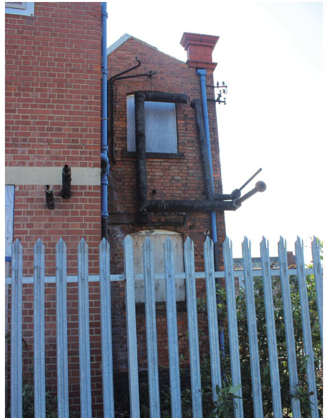
View of south extent of west elevation showing 1912 windows
