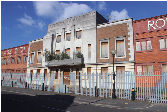
View of 1938 central block from east
