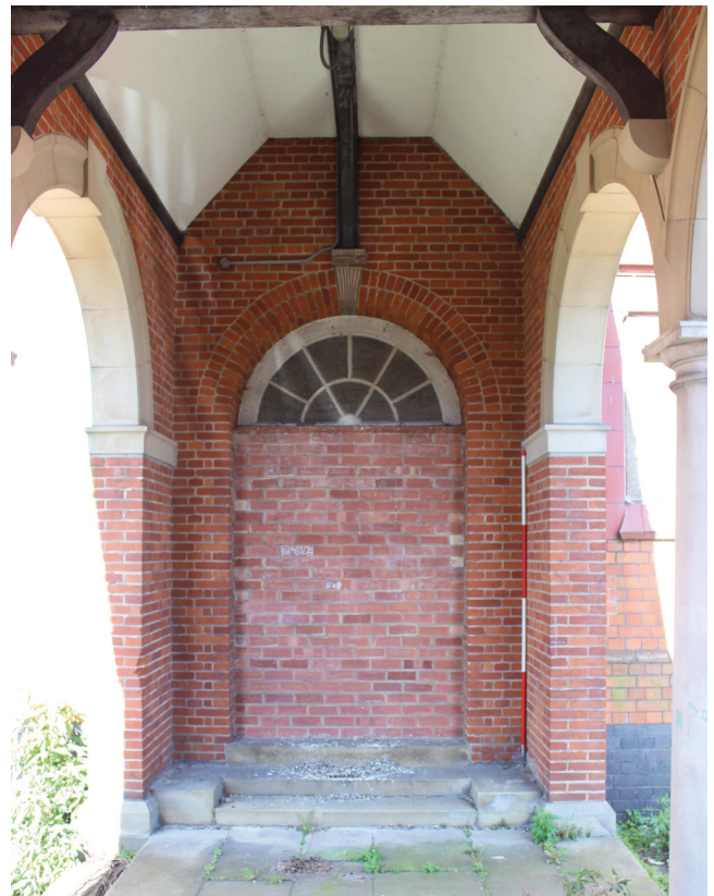
Detail of fanlight above block door to main building
