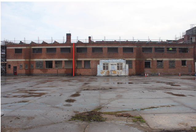
Detail of 1960s/1970s extension with break in masonry highlighted
