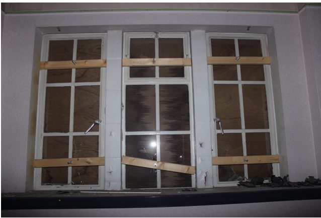
View of first floor window in east elevation
