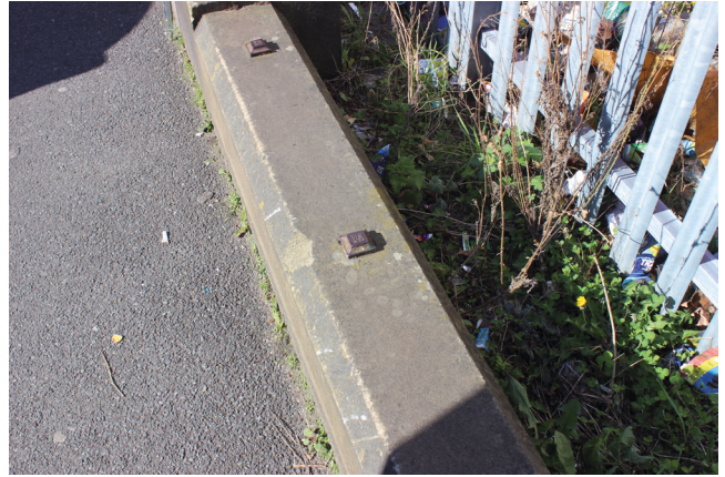
Detail of reused railing footings from loggia
