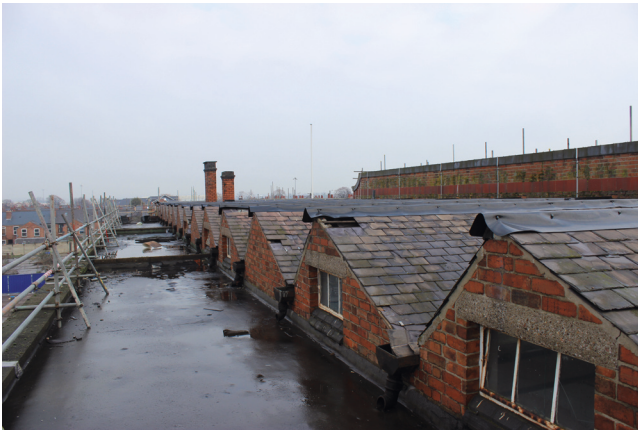
General view of roof above north wing
