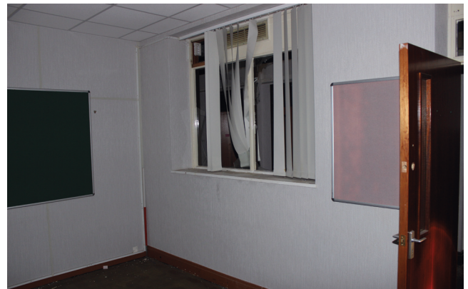
View of 1970s office in western portion of ground floor
