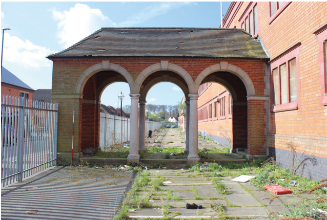
View of 1928 Loggia from north
