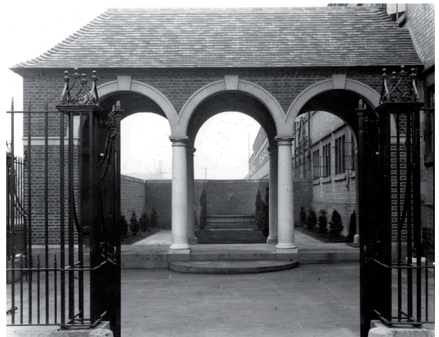
View of loggia, memorial garden and entrance gate. (Source unknown)
