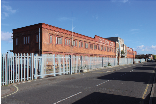
View of east elevation from south
