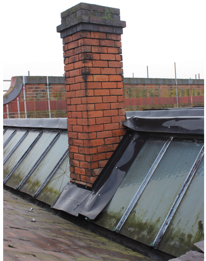
Detail of chimney
