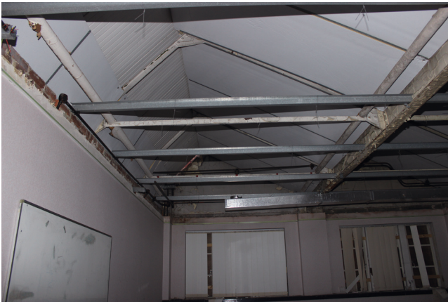
View of roof trusses in east portion of building
