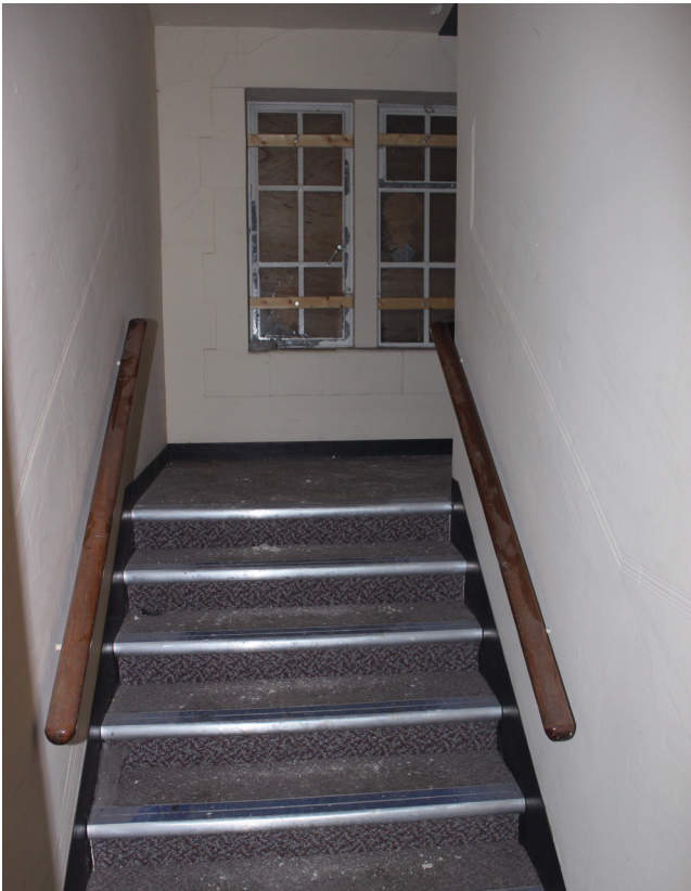
View of stair at south end of building
