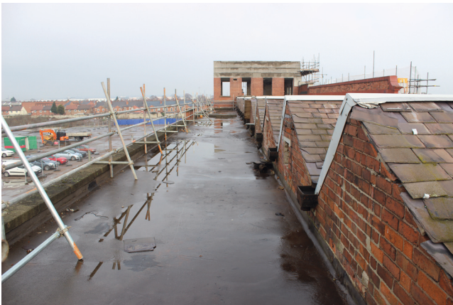
General view of roof above south wing
