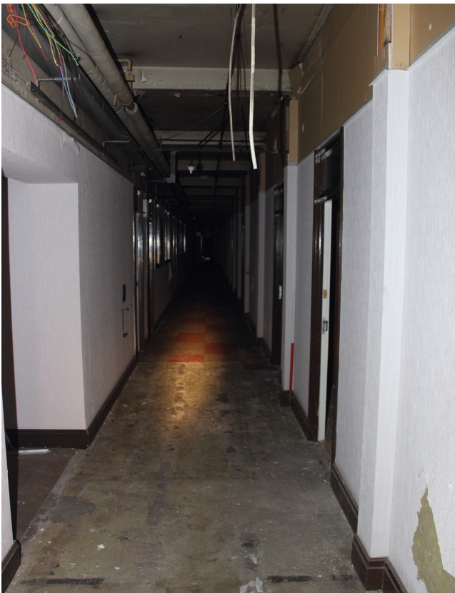
View of ground floor corridor in south wing
