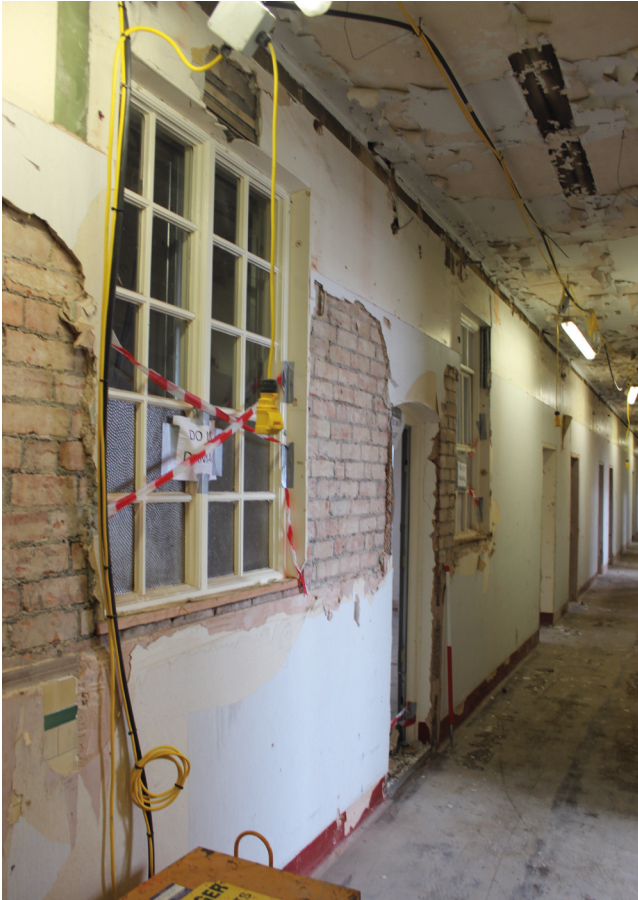
View of sash window in ground floor north corridor
