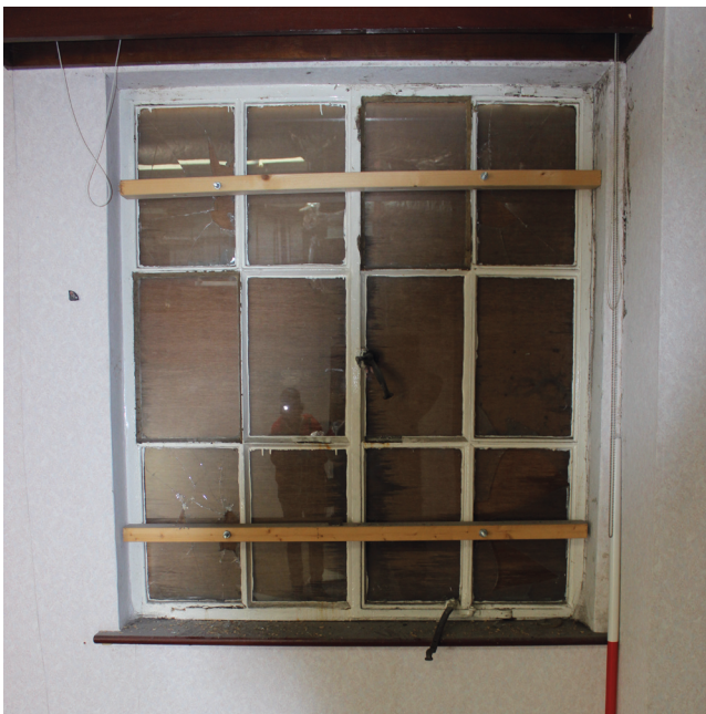
View of second floor window in east elevation
