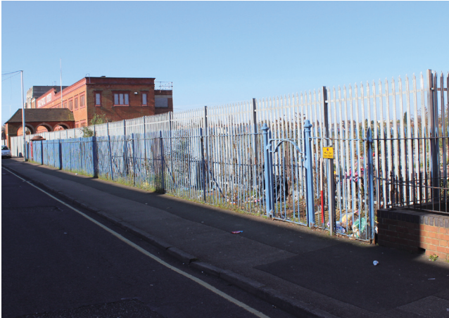
View of c.1908 railing on Nightingale Road
