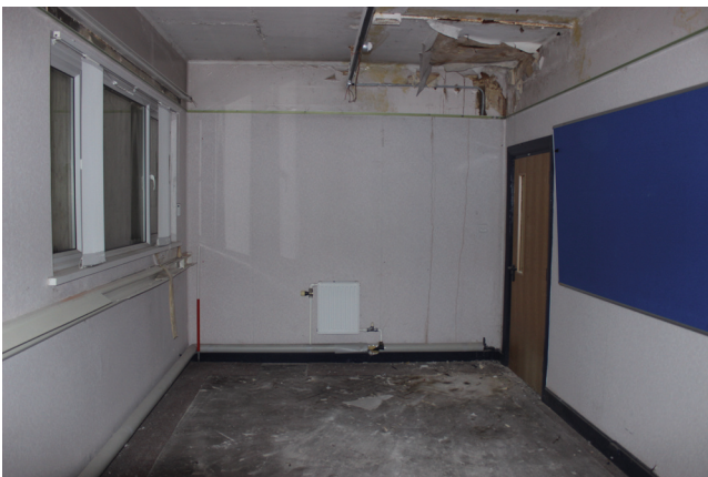
View of first floor room on west side of corridor
