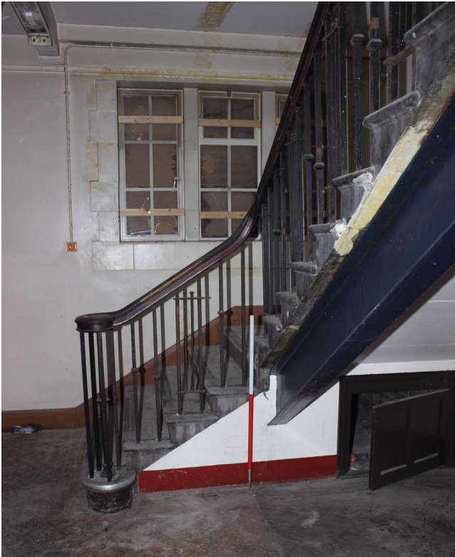
View of 1912 stair at north end of building
