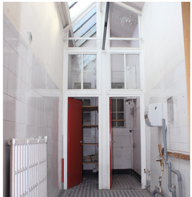
View of first floor toilets
