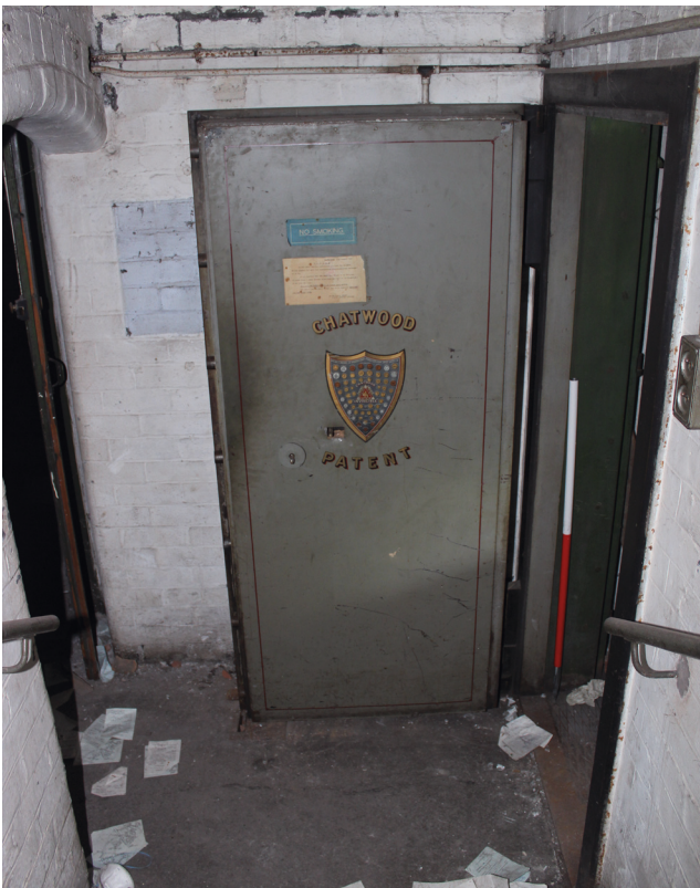
View of safe door to north basement room
