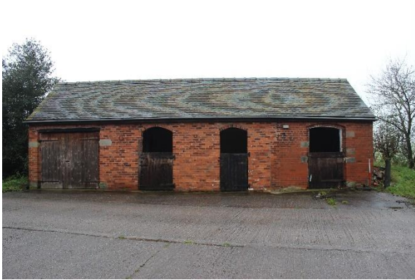
Figure 33: View of east elevation
