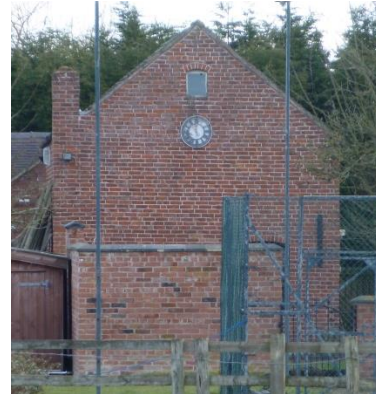
Photo 6: Bramshall Villa/ Park House - outbuilding detail
