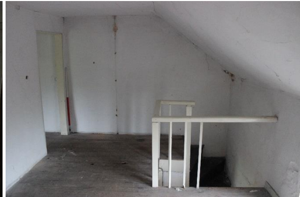
Figure 22: View of attic floor
