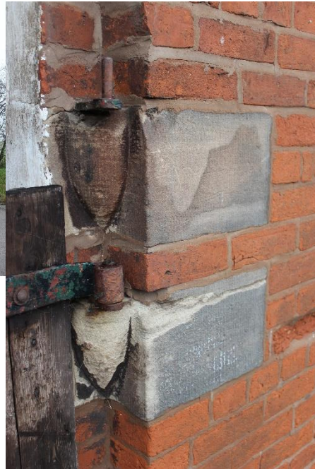
Figure 34: Detail of door hinges and stone quoins
