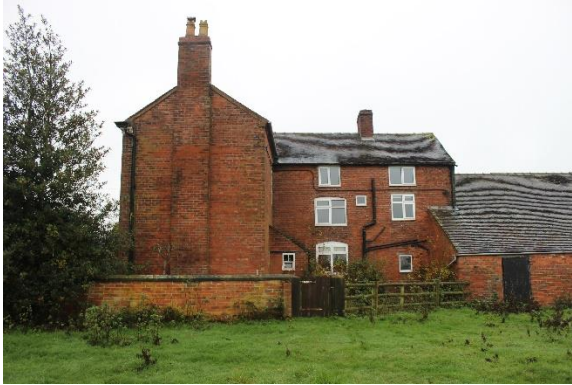
Figure 11: View of east gable
