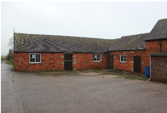
Figure 31: View of south elevation
