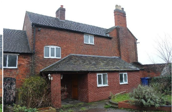
Figure 18: View of west elevation
