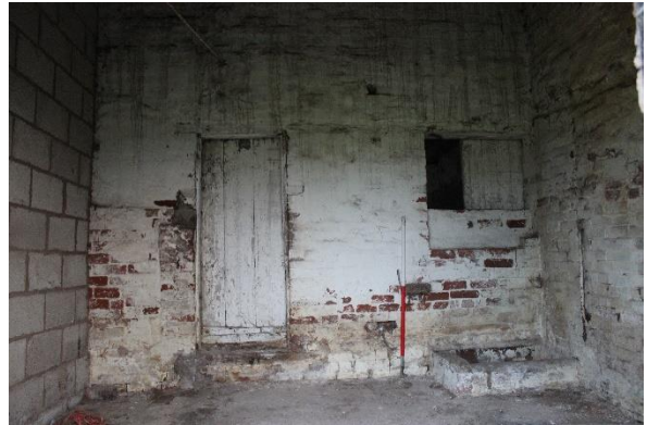
Figure 28: View of room in east bay
