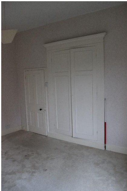
Figure 15: View of first floor room, west side
