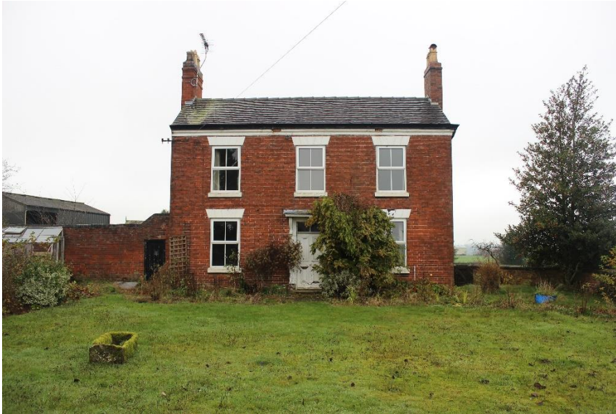
Figure 10: View of front (south) elevation
