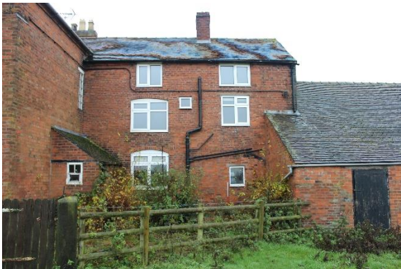
Figure 17: View of east elevation
