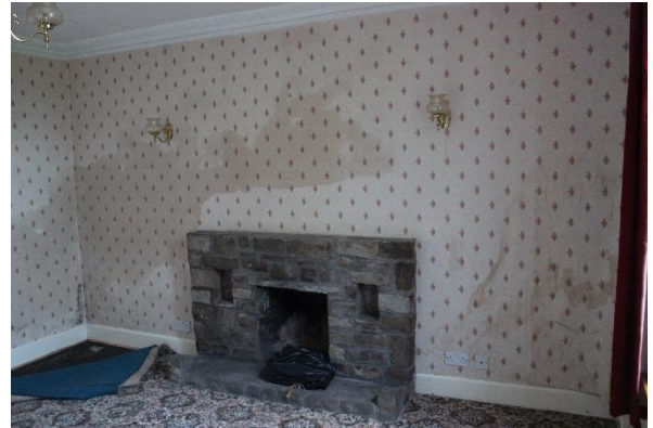
Figure 14: View of ground floor room, east side
