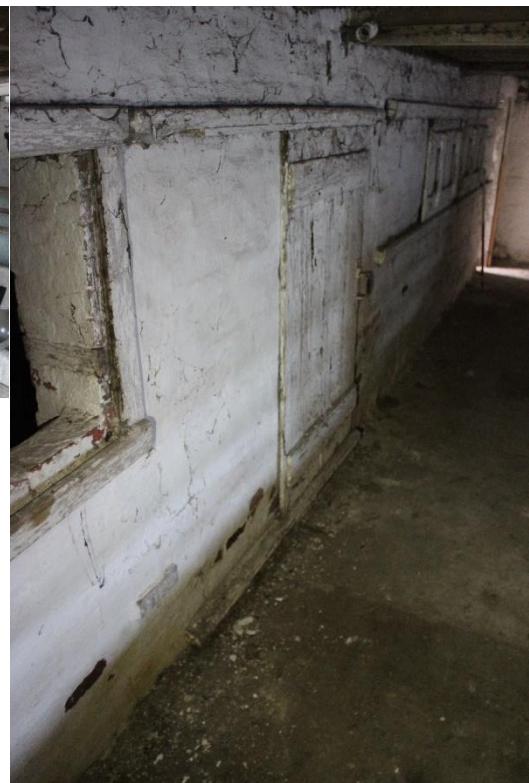
Figure 26: View of sliding windows and doors in east wall
