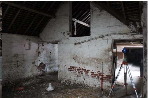
Figure 30: View of south bay of cowshed with former loft access
