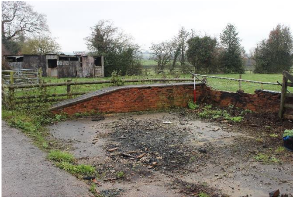
Figure 39: View of ramp to the north of the yard
