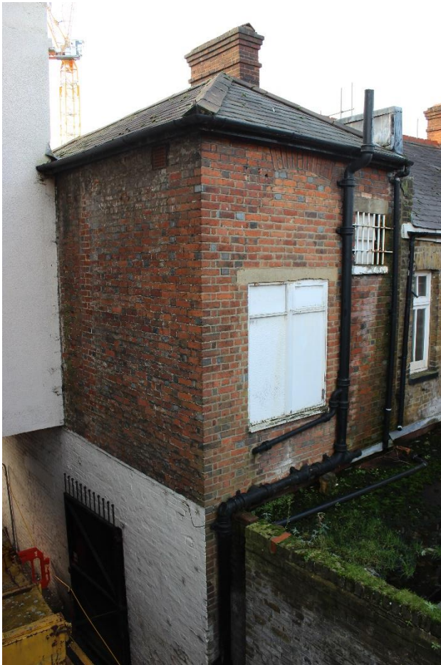
Figure 27: Number 45: View of rear elevation
