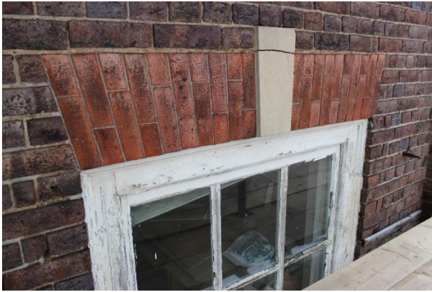
Figure 18: Number 39-41a: View of first floor window head
