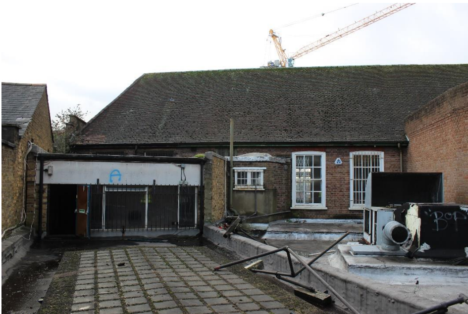
Figure 19: Number 39-41a: View of rear elevation
