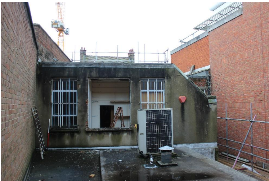
Figure 15: Number 37: View of rear elevation
