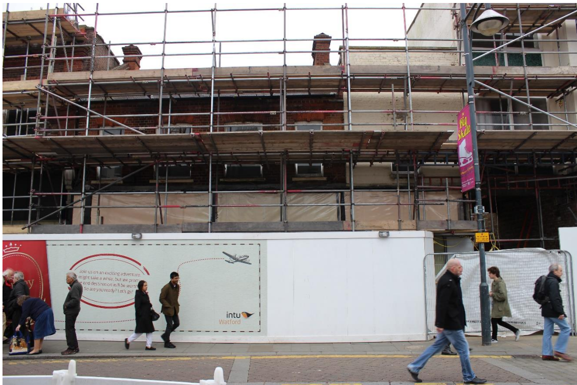
Figure 20: View of Number 45 High Street façade
