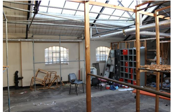
Figure 30: Industrial range: View of first floor
