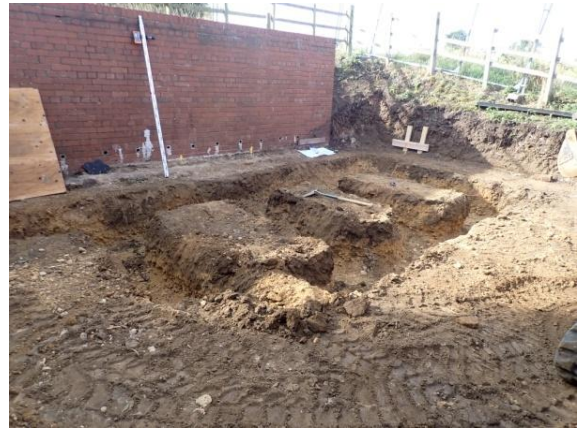
Plate 53: Excavation of the foundations, from the north-east
