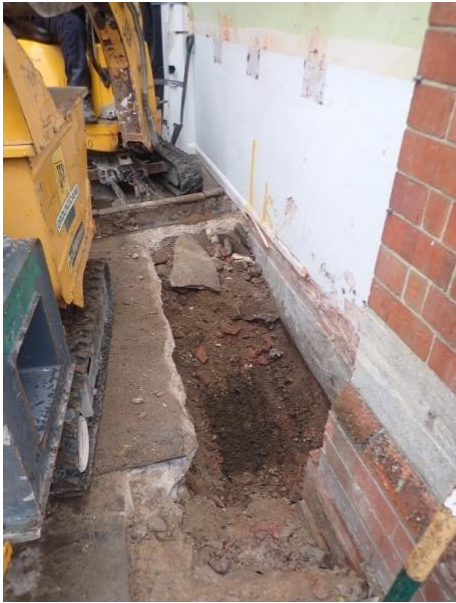
Plate 117: Excavation of the foundations, from the north
