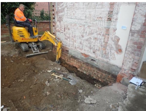
Plate 85: Excavation of the foundations, from the north-west
