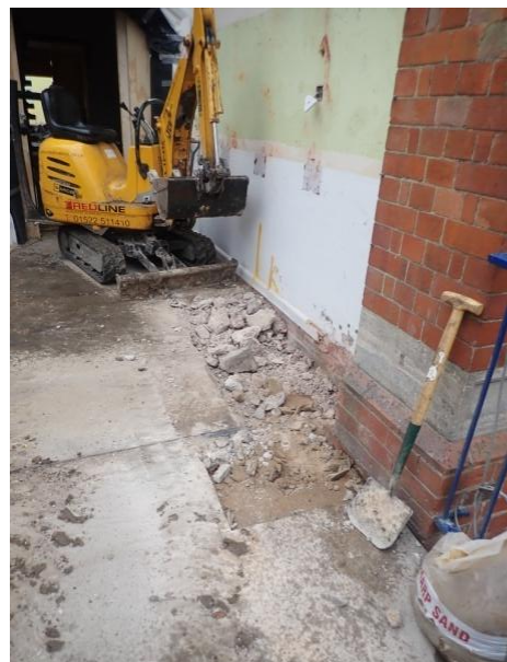
Plate 115: Excavation of the foundations, from the north
