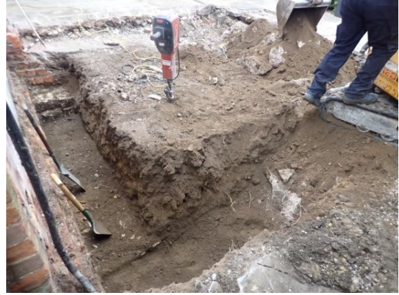
Plate 95: Excavation of the foundations, from the east
