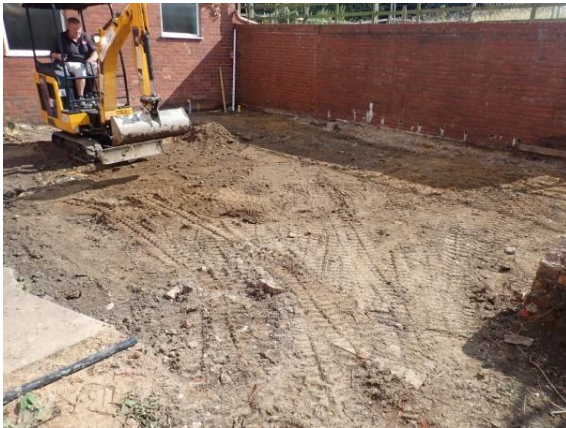
Plate 26: Initial ground reduction, from the north-west
