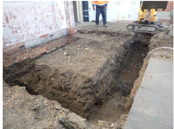
Plate 128: Excavation of the foundations, from the east
