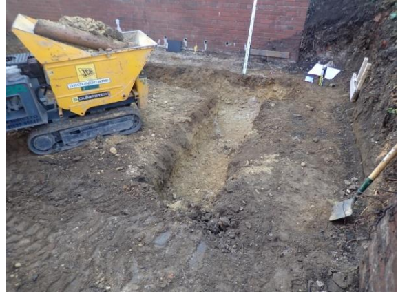
Plate 40: Excavation of the foundations, from the north
