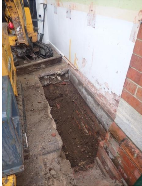
Plate 119: Excavation of the foundations, from the north
