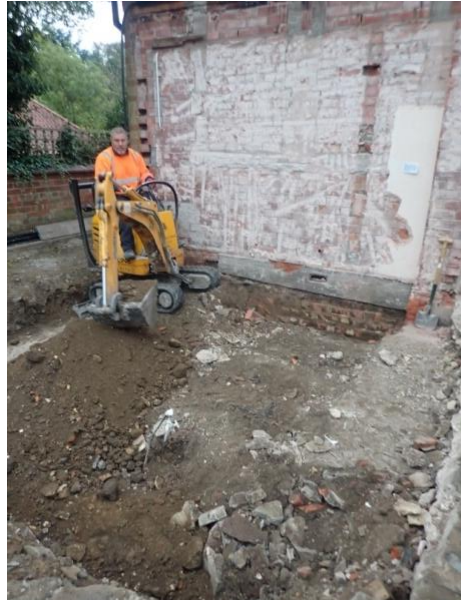
Plate 81: Excavation of the foundations, from the north
