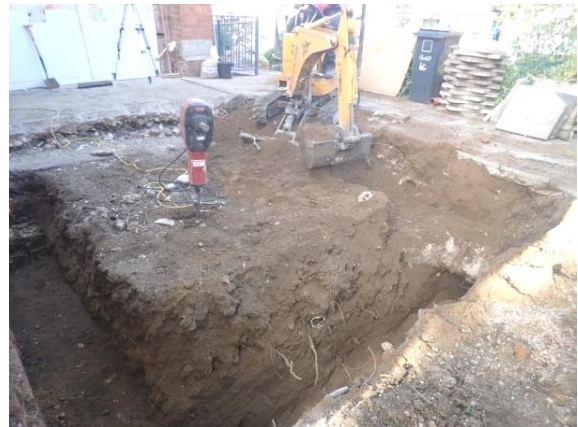
Plate 102: Excavation of the foundations, from the east
