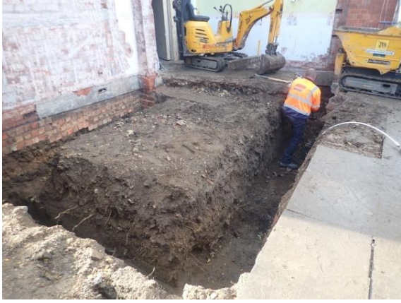
Plate 130: Excavation of the foundations, from the east
