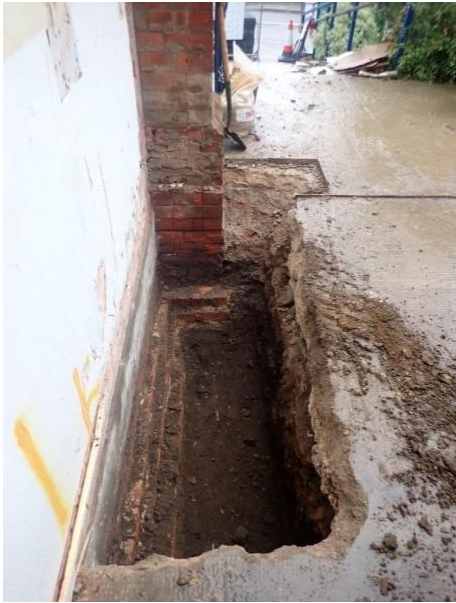
Plate 121: Excavation of the foundations, from the south
