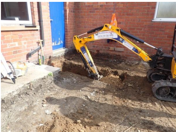
Plate 57: Excavation of the foundations, from the west
