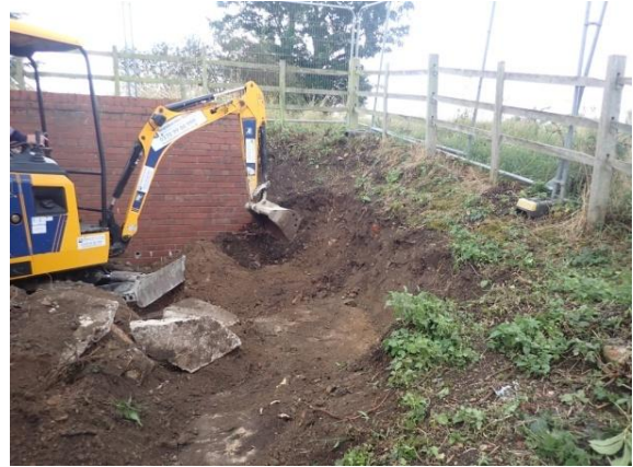
Plate 4: Initial ground reduction, from the north
