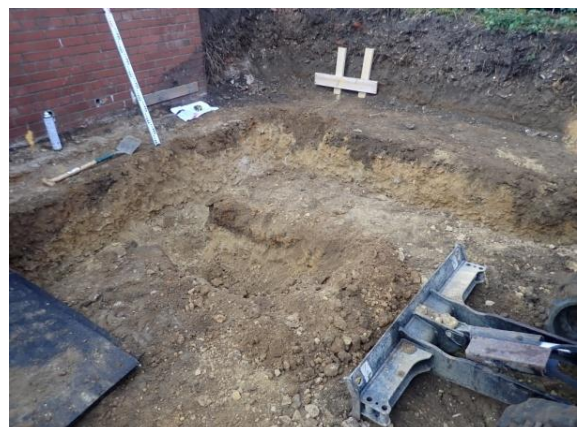
Plate 42: Excavation of the foundations, from the east
