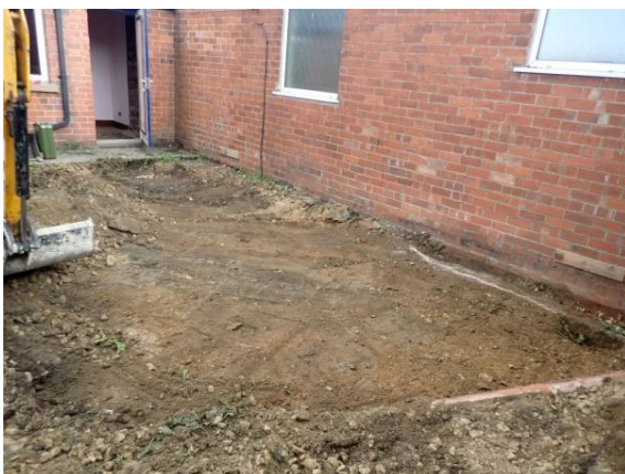
Plate 15: Initial ground reduction, from the south
