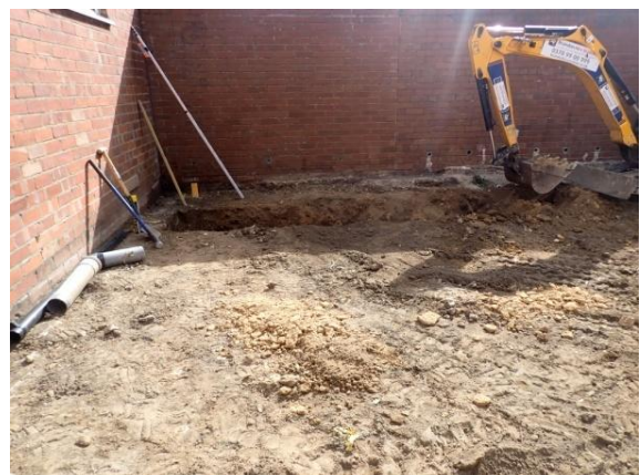
Plate 30: Excavation of the foundations, from the north
