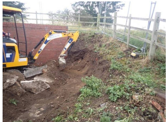
Plate 5: Initial ground reduction, from the north
