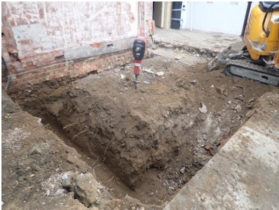
Plate 105: Excavation of the foundations, from the north-east
