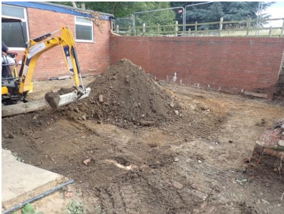
Plate 20: Initial ground reduction, from the north-west
