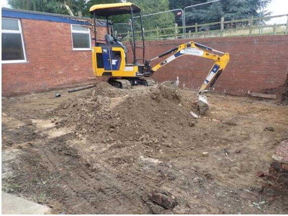
Plate 19: Initial ground reduction, from the north-west
