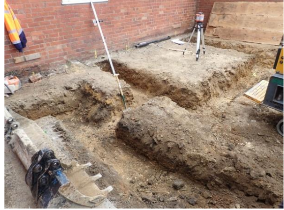
Plate 64: Excavation of the foundations, from the north-west
