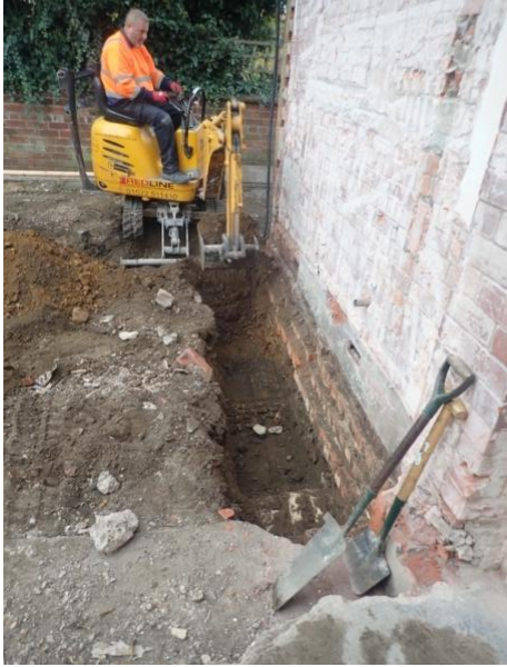
Plate 83: Excavation of the foundations, from the west
