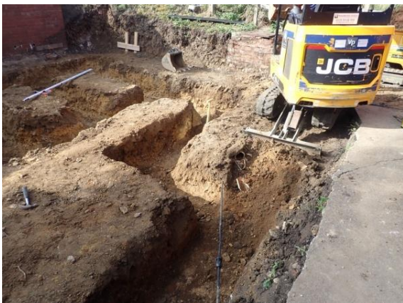
Plate 69: Excavation of the foundations, from the east
