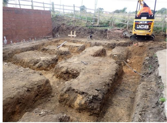
Plate 70: Excavation of the foundations, from the east
