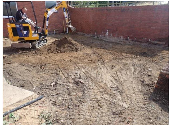
Plate 23: Initial ground reduction, from the north-west
