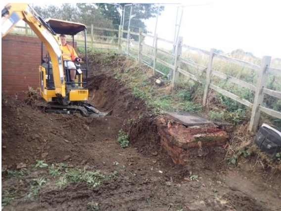
Plate 9: Initial ground reduction, from the north
