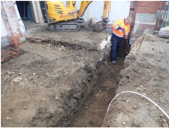
Plate 131: Excavation of the foundations, from the east
