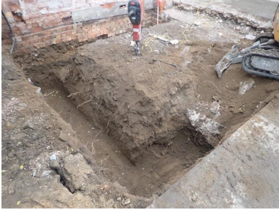
Plate 104: Excavation of the foundations, from the east
