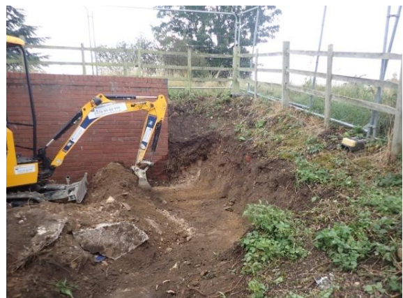
Plate 6: Initial ground reduction, from the north
