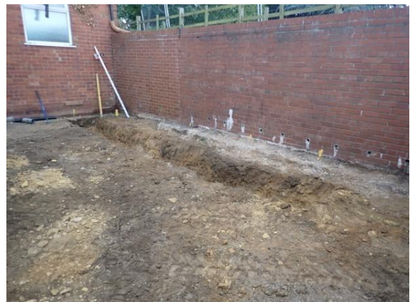
Plate 36: Excavation of the foundations, from the north-west
