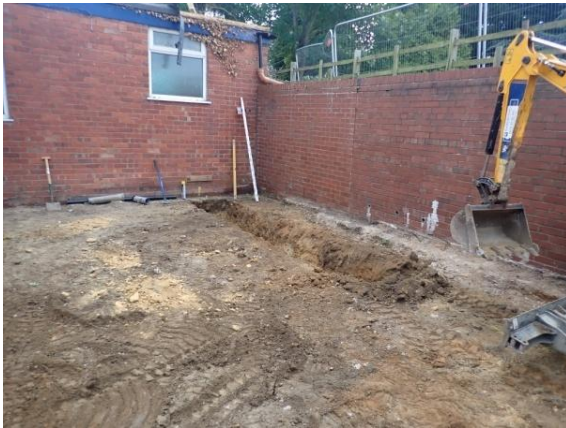
Plate 32: Excavation of the foundations, from the north-west
