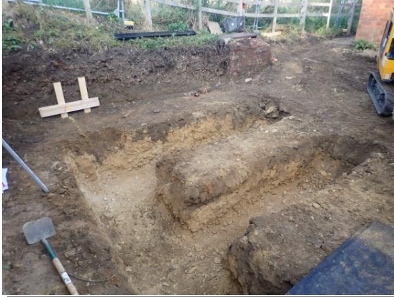
Plate 43: Excavation of the foundations, from the east
