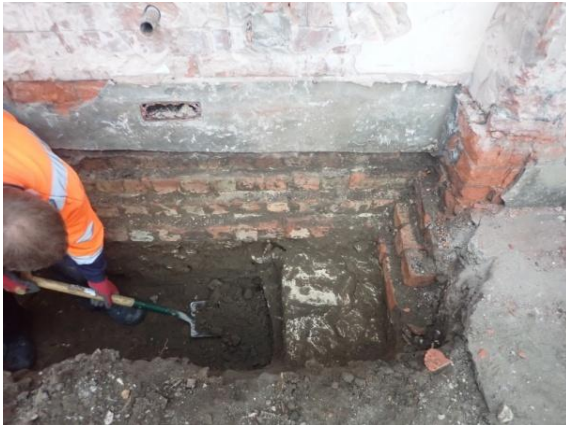
Plate 84: Excavation of the foundations, from the north
