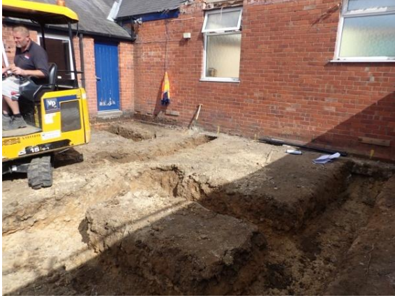
Plate 61: Excavation of the foundations, from the south-west
