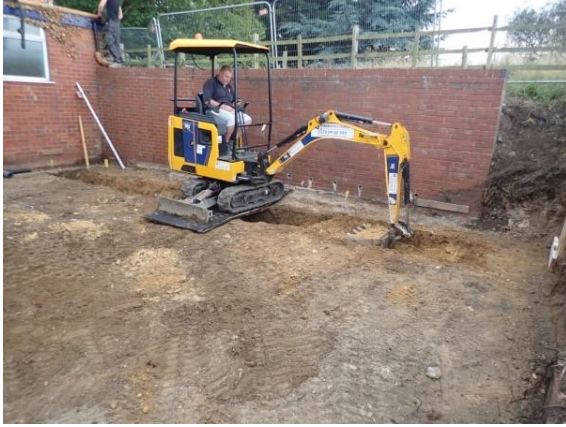
Plate 37: Excavation of the foundations, from the north
