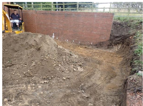
Plate 18: Initial ground reduction, from the north
