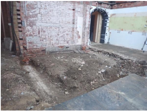
Plate 74: Pre-groundworks, from the north-east
