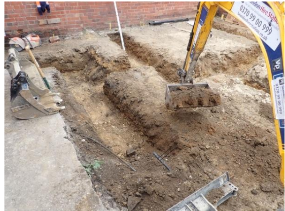
Plate 65: Excavation of the foundations, from the west
