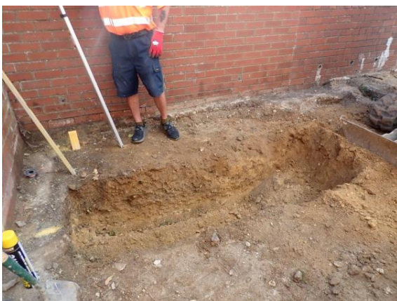
Plate 27: Excavation of the foundations, from the north
