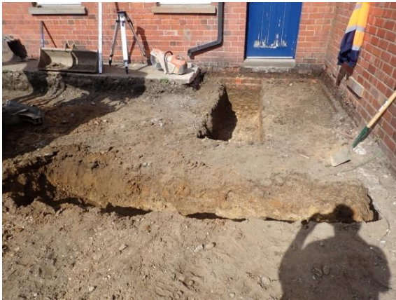
Plate 62: Excavation of the foundations, from the south
