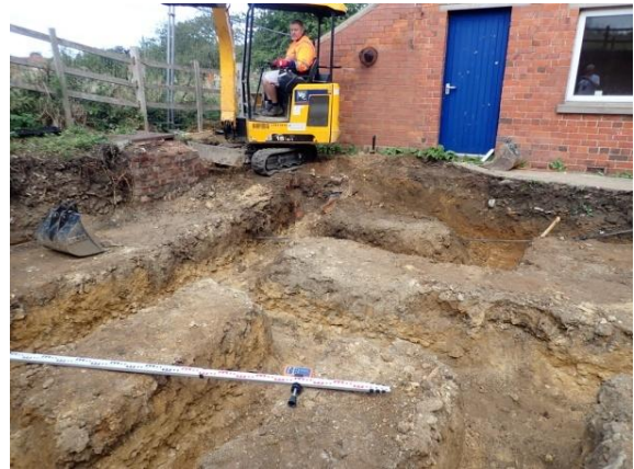
Plate 71: Excavation of the foundations, from the south
