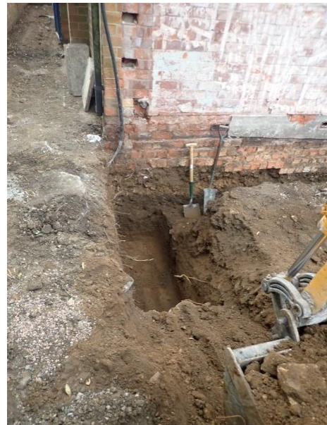
Plate 96: Excavation of the foundations, from the north
