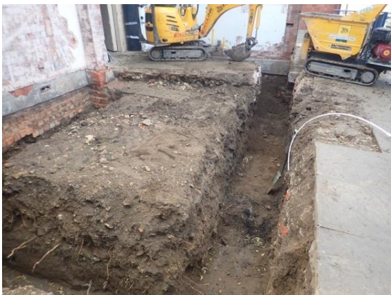
Plate 132: Excavation of the foundations, from the east
