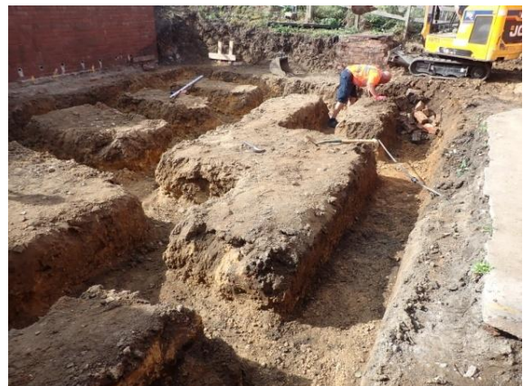
Plate 72: Excavation of the foundations, from the east
