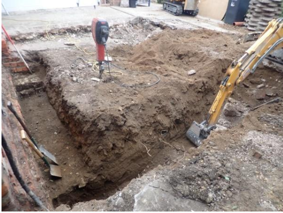
Plate 98: Excavation of the foundations, from the east
