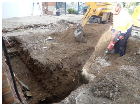
Plate 97: Excavation of the foundations, from the east
