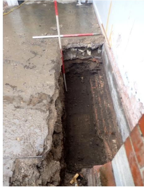
Plate 122: Excavation of the foundations, from the north
