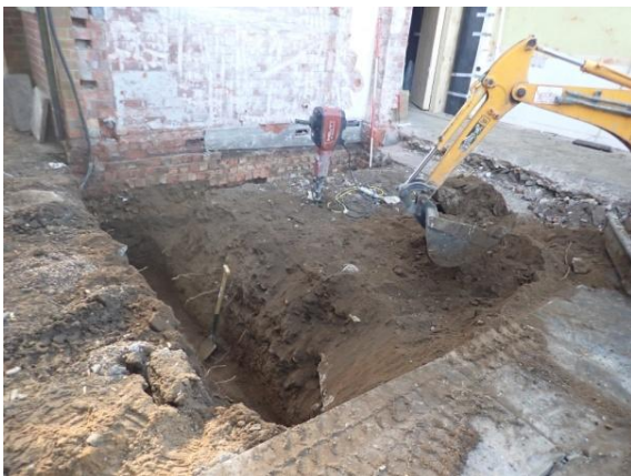
Plate 100: Excavation of the foundations, from the north
