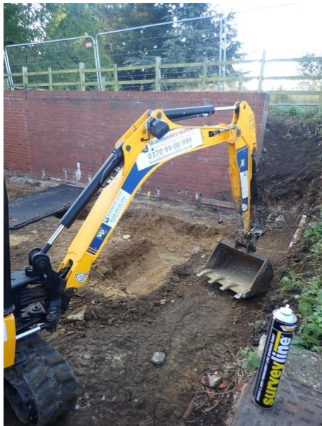
Plate 38: Excavation of the foundations, from the north
