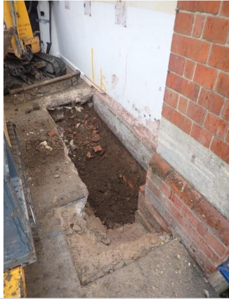
Plate 118: Excavation of the foundations, from the north
