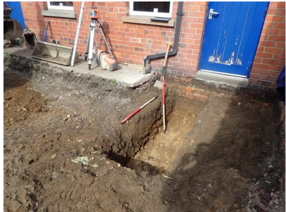
Plate 59: Excavation of the foundations, from the south
