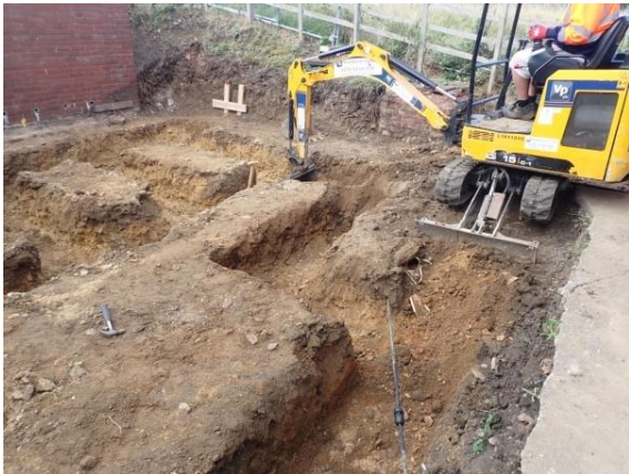
Plate 68: Excavation of the foundations, from the east
