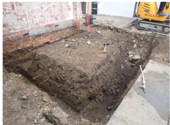
Plate 109: Excavation of the foundations, from the north-east
