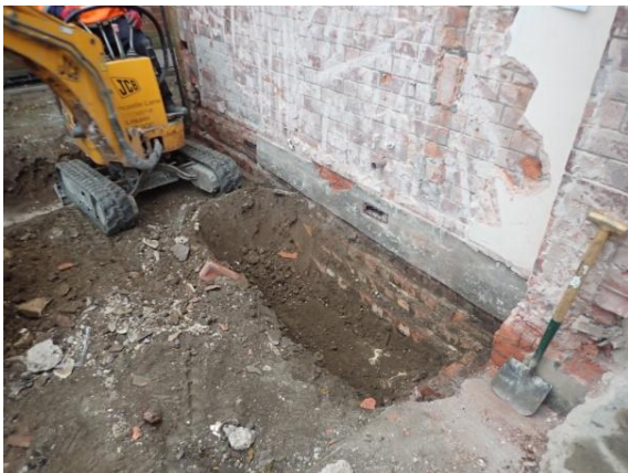
Plate 80: Excavation of the foundations, from the north-west
