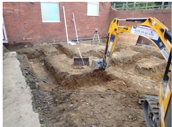
Plate 66: Excavation of the foundations, from the west
