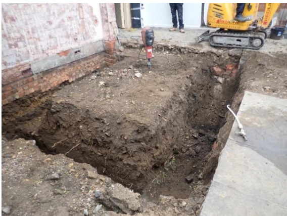
Plate 112: Excavation of the foundations, from the east
