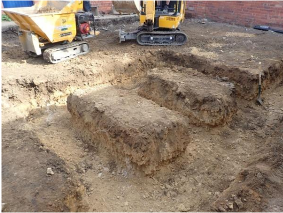
Plate 49: Excavation of the foundations, from the south-west
