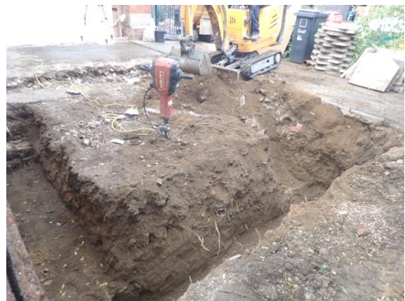
Plate 103: Excavation of the foundations, from the east
