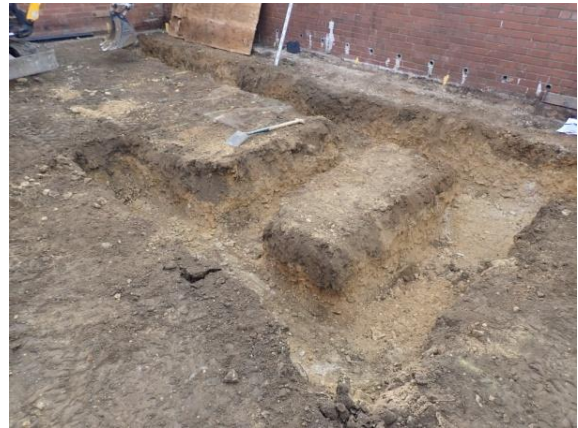
Plate 47: Excavation of the foundations, from the north-west
