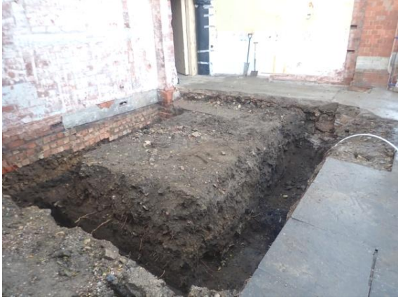
Plate 124: Excavation of the foundations, from the east
