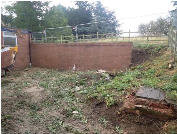
Plate 2: Pre-groundworks, from the north-west
