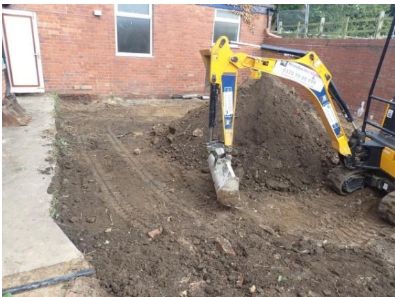
Plate 21: Initial ground reduction, from the west
