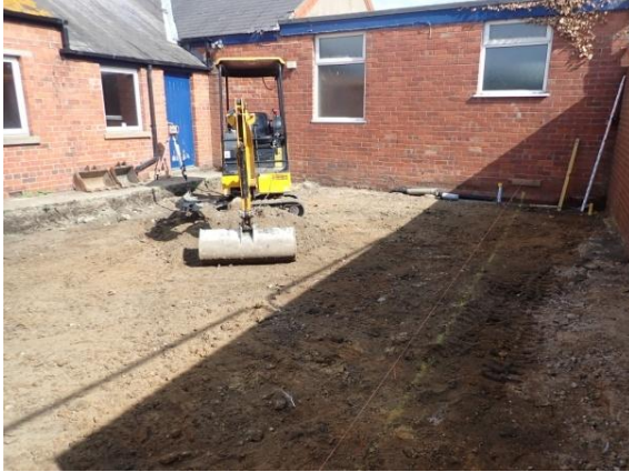
Plate 25: Initial ground reduction, from the west
