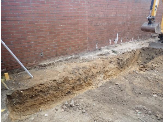
Plate 31: Excavation of the foundations, from the north
