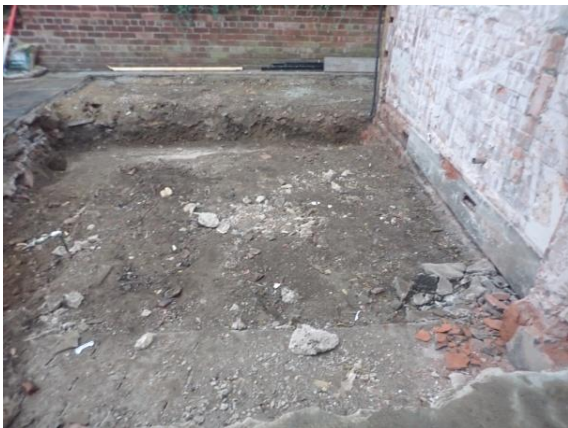
Plate 79: Pre-groundworks, from the west
