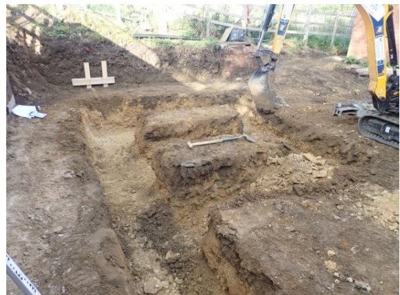
Plate 48: Excavation of the foundations, from the east
