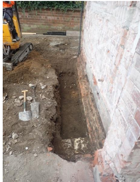
Plate 87: Excavation of the foundations, from the west
