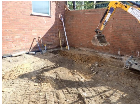
Plate 29: Excavation of the foundations, from the north-west
