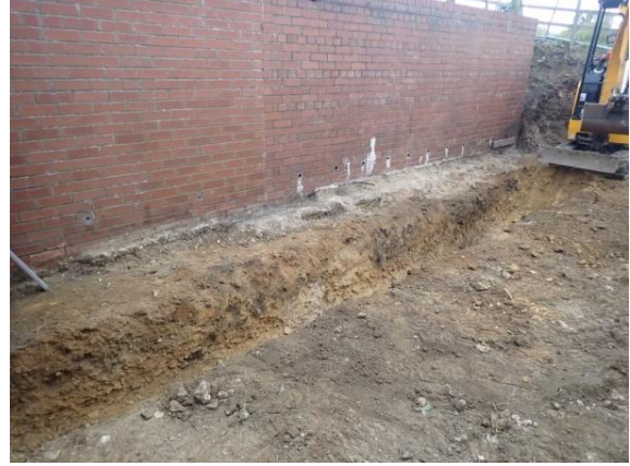
Plate 34: Excavation of the foundations, from the north-east
