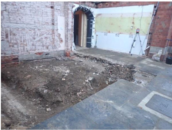
Plate 75: Pre-groundworks, from the north-east
