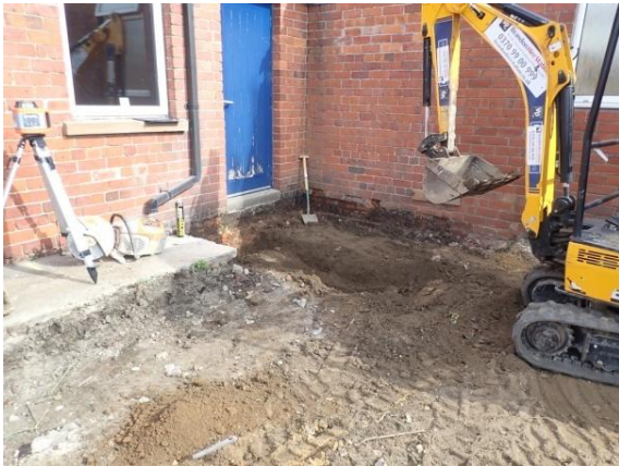
Plate 56: Excavation of the foundations, from the west
