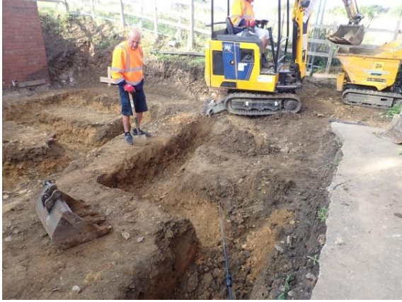
Plate 67: Excavation of the foundations, from the east
