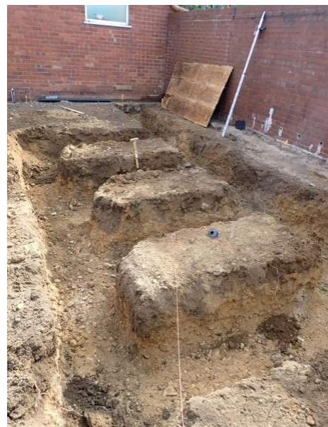
Plate 54: Excavation of the foundations, from the west
