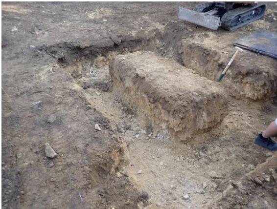
Plate 44: Excavation of the foundations, from the south
