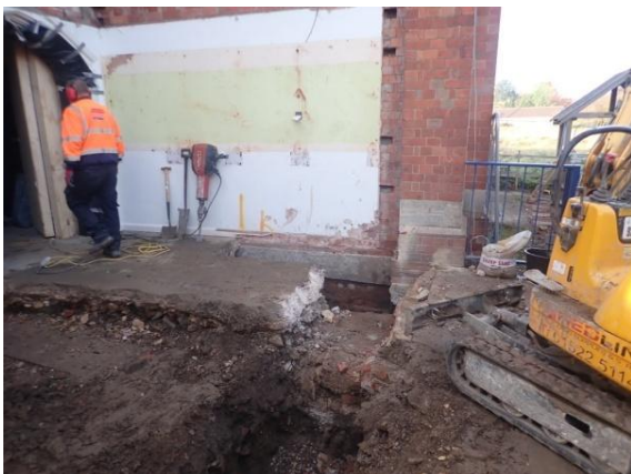
Plate 126: Excavation of the foundations, from the east
