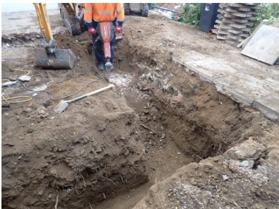
Plate 106: Excavation of the foundations, from the east
