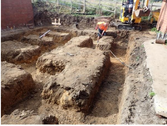
Plate 73: Excavation of the foundations, from the east
