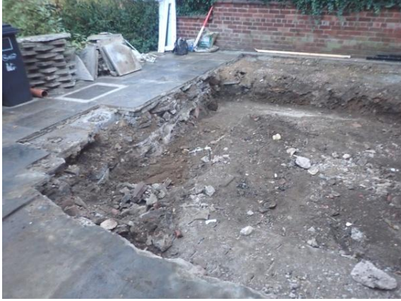
Plate 78: Pre-groundworks, from the west
