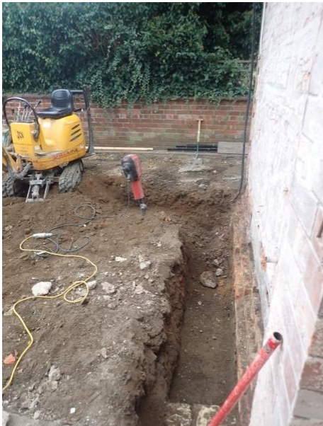
Plate 94: Excavation of the foundations, from the west
