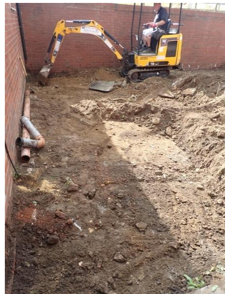
Plate 17: Initial ground reduction, from the north
