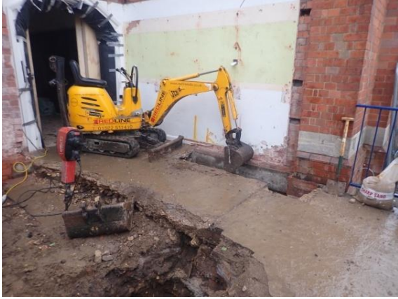
Plate 120: Excavation of the foundations, from the east
