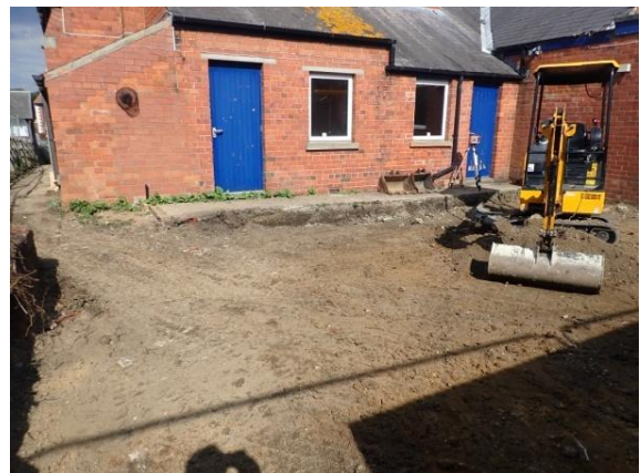
Plate 24: Initial ground reduction, from the north-west
