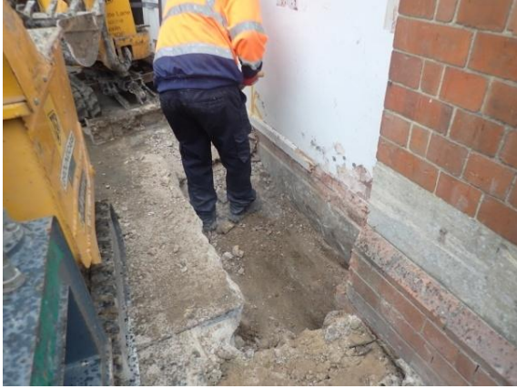
Plate 116: Excavation of the foundations, from the north
