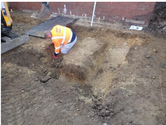
Plate 45: Excavation of the foundations, from the north
