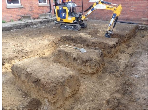
Plate 52: Excavation of the foundations, from the south-west
