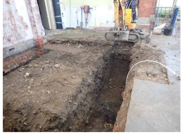
Plate 127: Excavation of the foundations, from the east
