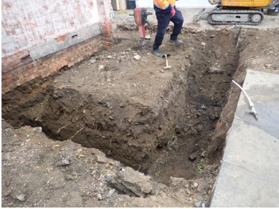
Plate 110: Excavation of the foundations, from the east
