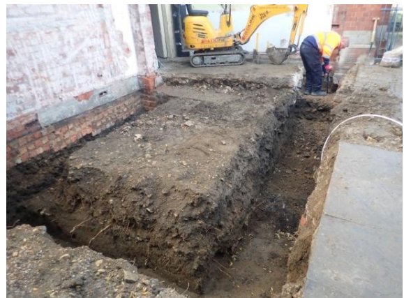
Plate 129: Excavation of the foundations, from the east
