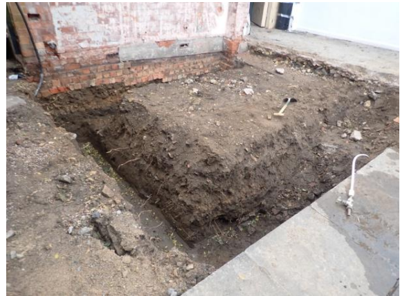
Plate 108: Excavation of the foundations, from the north-east
