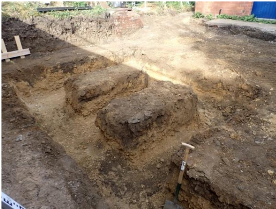
Plate 50: Excavation of the foundations, from the south-east
