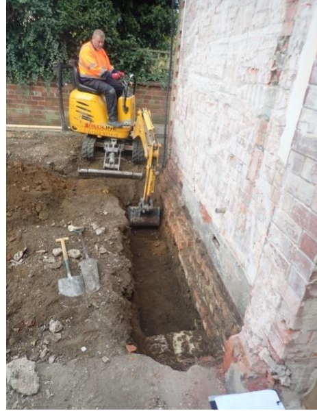
Plate 86: Excavation of the foundations, from the west
