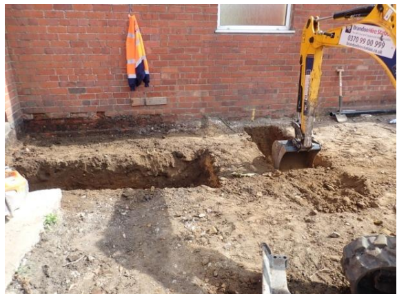
Plate 60: Excavation of the foundations, from the west
