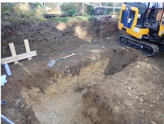
Plate 39: Excavation of the foundations, from the east
