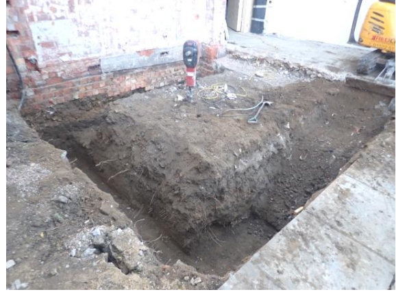
Plate 107: Excavation of the foundations, from the north-east
