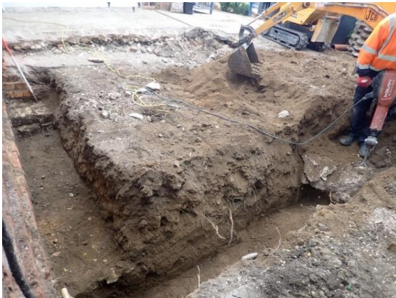
Plate 99: Excavation of the foundations, from the east
