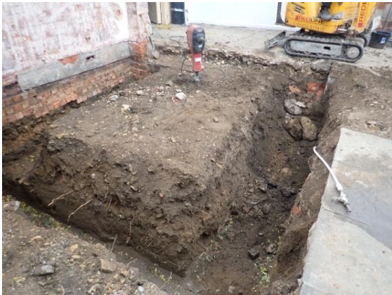
Plate 111: Excavation of the foundations, from the east
