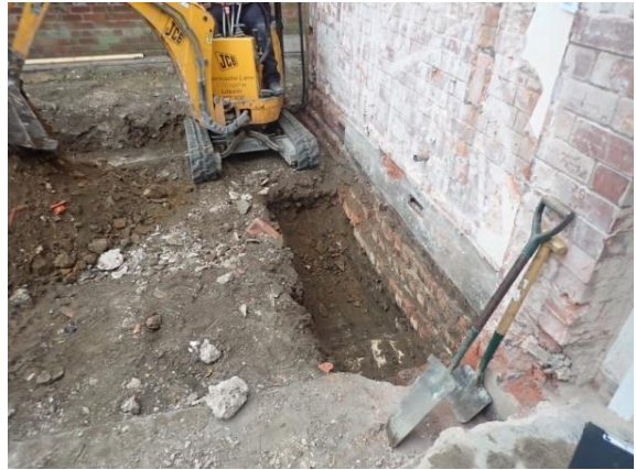
Plate 82: Excavation of the foundations, from the west
