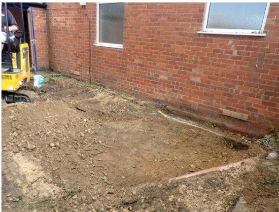
Plate 14: Initial ground reduction, from the south
