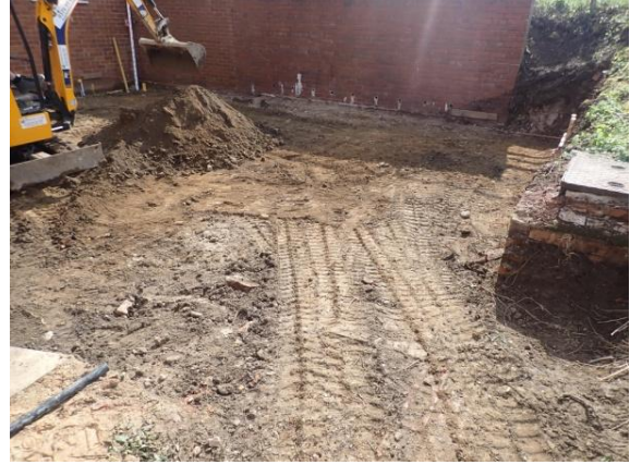
Plate 22: Initial ground reduction, from the north-west
