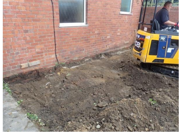
Plate 16: Initial ground reduction, from the south
