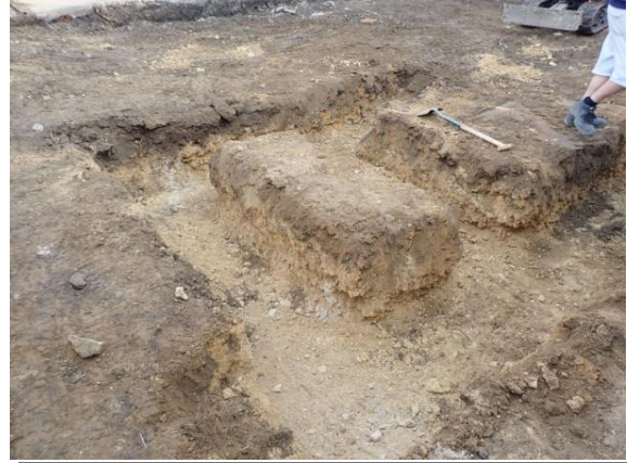
Plate 46: Excavation of the foundations, from the south
