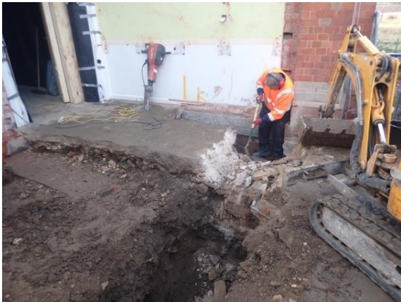
Plate 125: Excavation of the foundations, from the east
