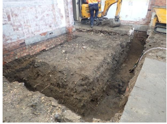
Plate 133: Excavation of the foundations, from the east
