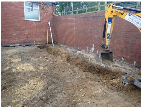
Plate 33: Excavation of the foundations, from the north-west
