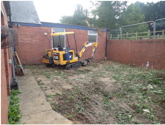
Plate 1: Pre-groundworks, from the west
