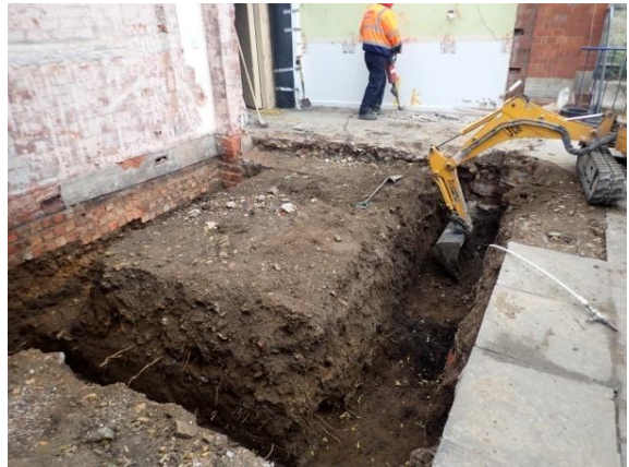
Plate 114: Excavation of the foundations, from the east
