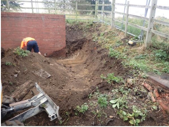
Plate 7: Initial ground reduction, from the north
