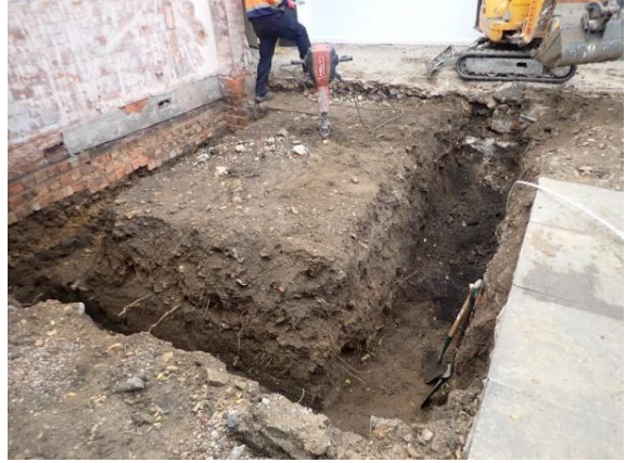
Plate 113: Excavation of the foundations, from the east
