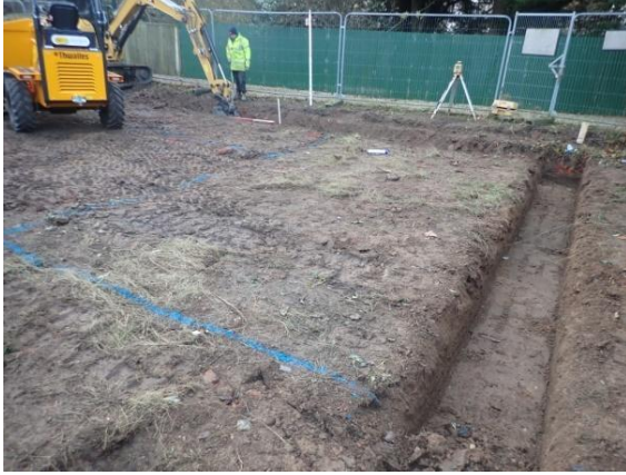
Plate 18: Excavation of the foundations, from the north
