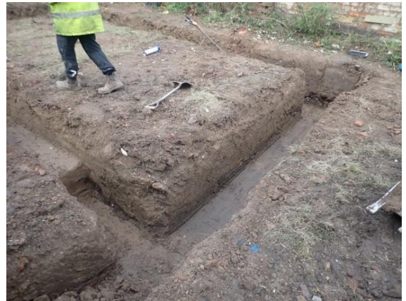
Plate 38: Excavation of the foundations, from the north-east
