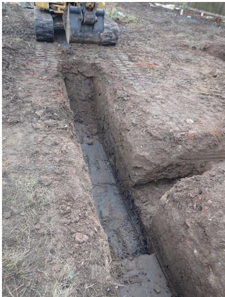
Plate 41: Excavation of the foundations, from the west
