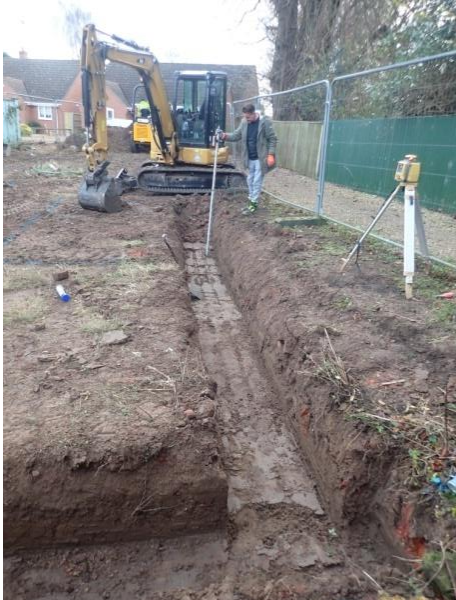
Plate 15: Excavation of the foundations, from the west
