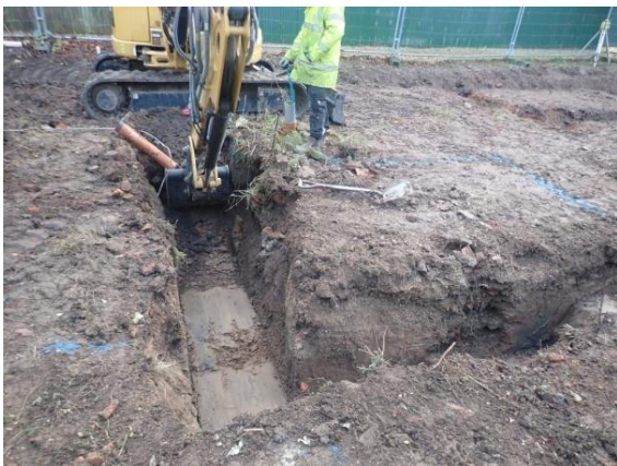
Plate 52: Excavation of the foundations, from the north
