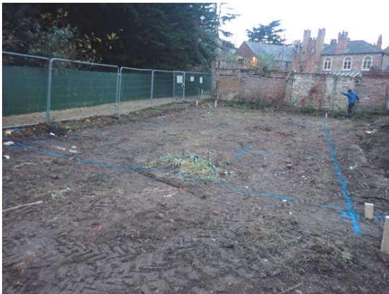
Plate 2: Pre-groundworks, from the east
