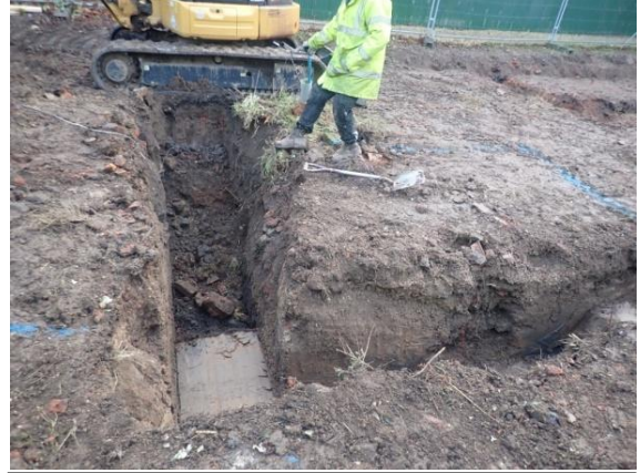
Plate 53: Excavation of the foundations, from the north
