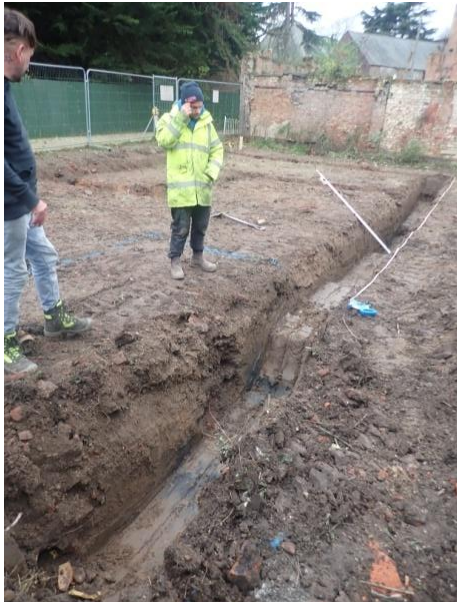
Plate 46: Excavation of the foundations, from the east
