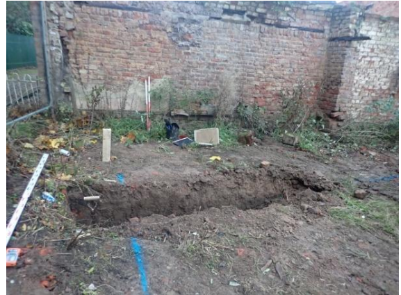
Plate 4: Excavation of the foundations, from the east
