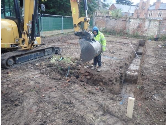
Plate 50: Excavation of the foundations, from the east
