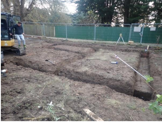
Plate 40: Excavation of the foundations, from the north
