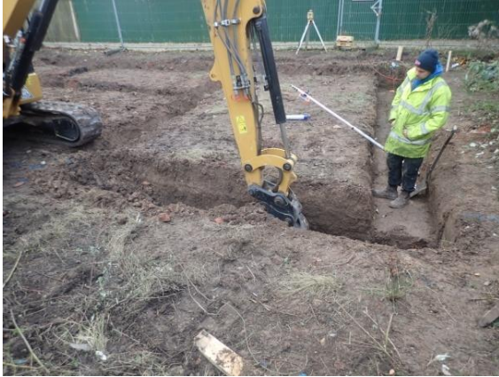
Plate 34: Excavation of the foundations, from the north
