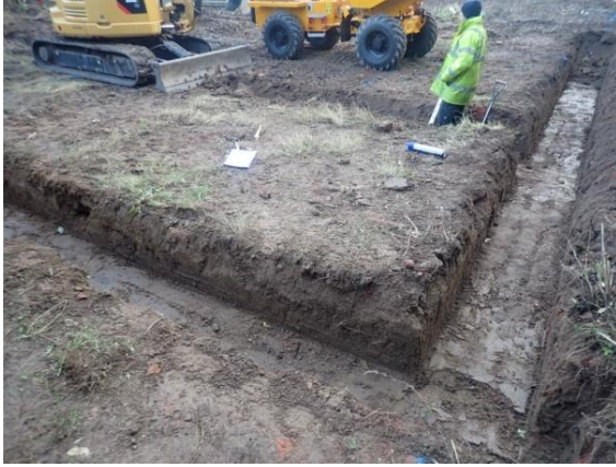
Plate 23: Excavation of the foundations, from the west
