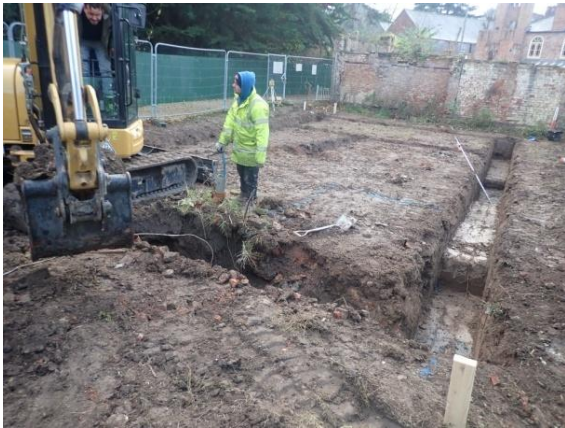
Plate 51: Excavation of the foundations, from the east
