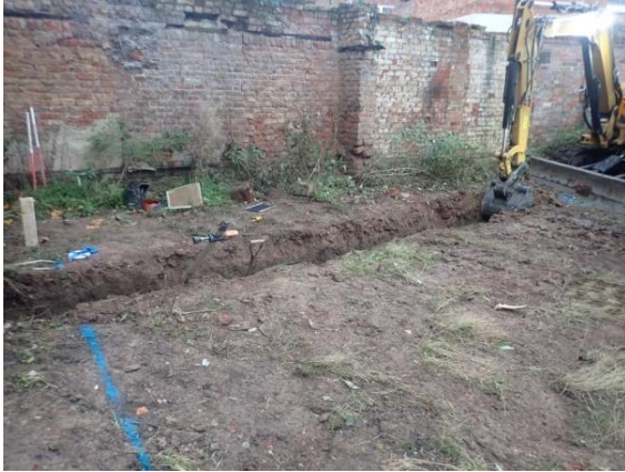
Plate 7: Excavation of the foundations, from the east
