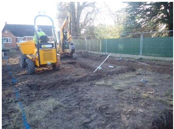
Plate 28: Excavation of the foundations, from the west
