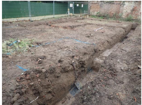
Plate 48: Excavation of the foundations, from the north-east
