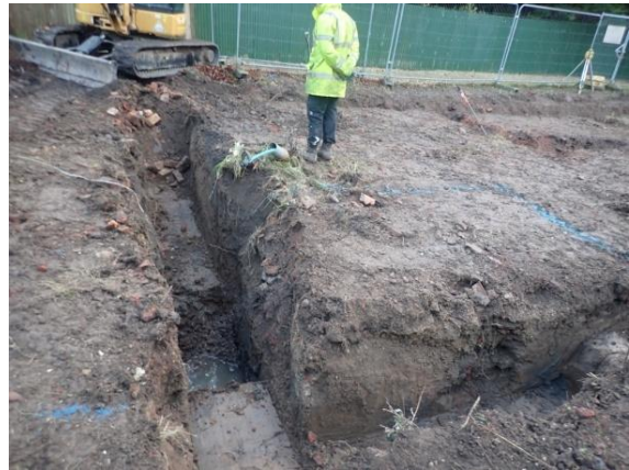
Plate 60: Excavation of the foundations, from the north
