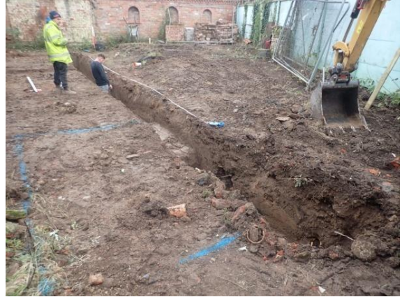
Plate 47: Excavation of the foundations, from the east
