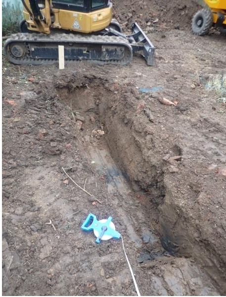
Plate 45: Excavation of the foundations, from the west
