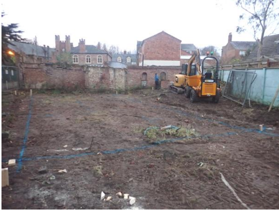
Plate 1: Pre-groundworks, from the east
