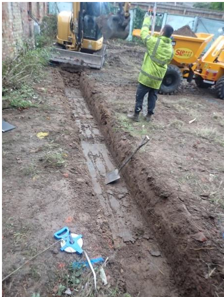
Plate 8: Excavation of the foundations, from the south
