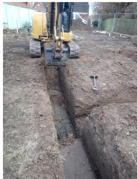
Plate 39: Excavation of the foundations, from the west
