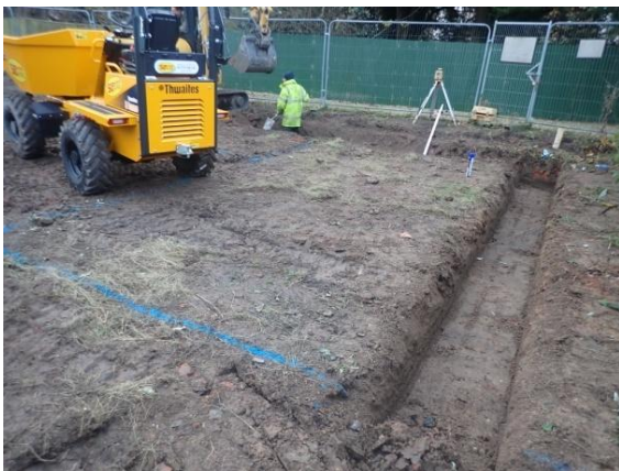
Plate 14: Excavation of the foundations, from the north
