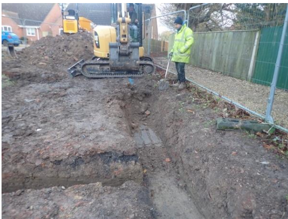
Plate 58: Excavation of the foundations, from the west
