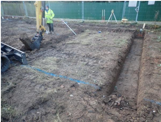
Plate 24: Excavation of the foundations, from the north
