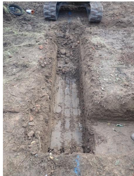
Plate 33: Excavation of the foundations, from the west
