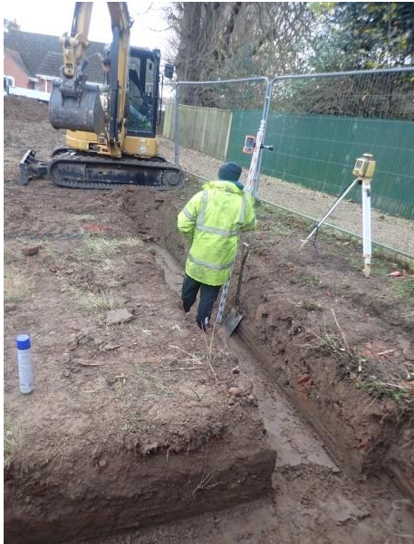
Plate 13: Excavation of the foundations, from the west
