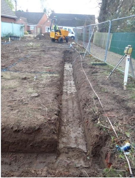
Plate 20: Excavation of the foundations, from the west
