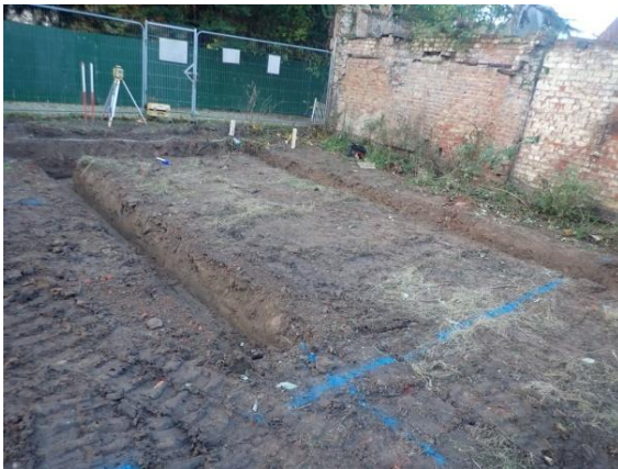
Plate 25: Excavation of the foundations, from the north
