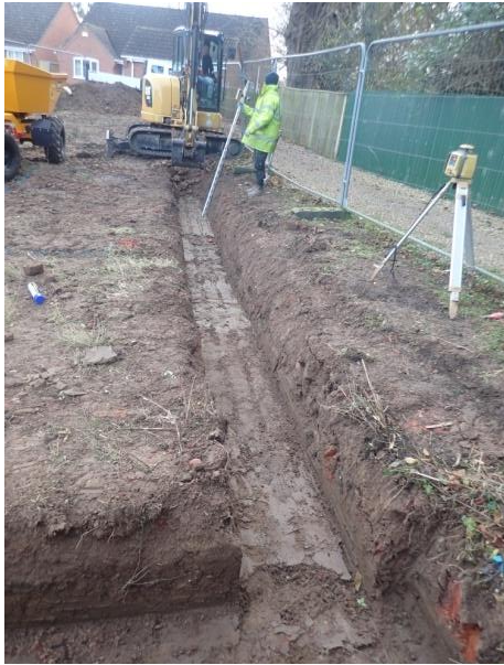
Plate 19: Excavation of the foundations, from the west
