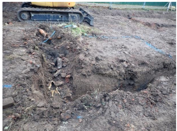
Plate 49: Excavation of the foundations, from the north
