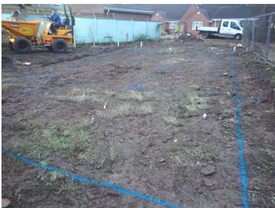
Plate 3: Pre-groundworks, from the west
