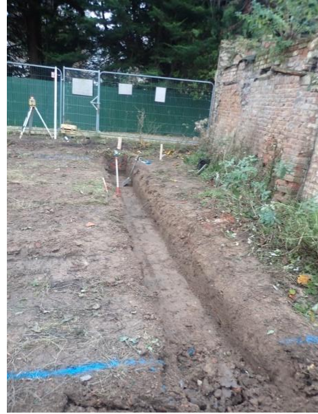
Plate 10: Excavation of the foundations, from the north
