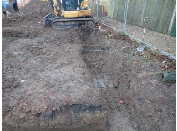
Plate 59: Excavation of the foundations, from the west
