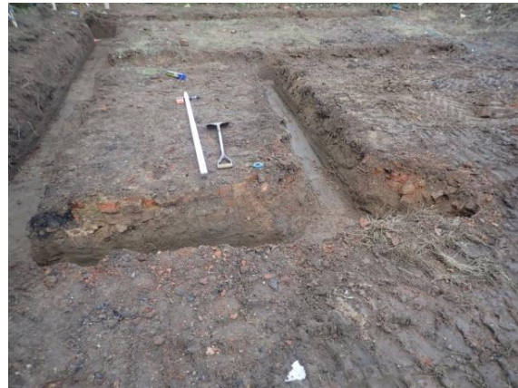
Plate 32: Excavation of the foundations, from the south
