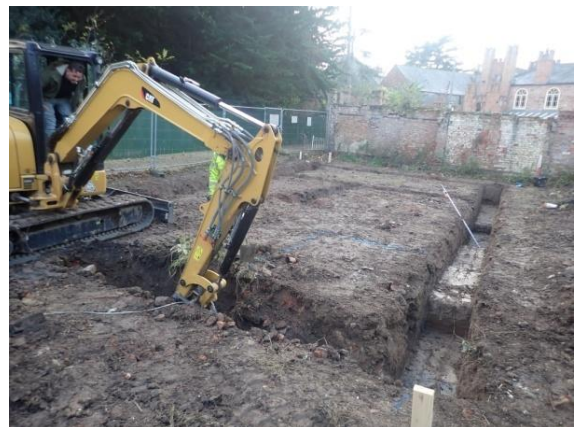
Plate 55: Excavation of the foundations, from the east
