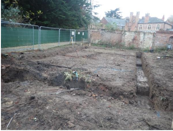
Plate 62: Excavation of the foundations, from the east
