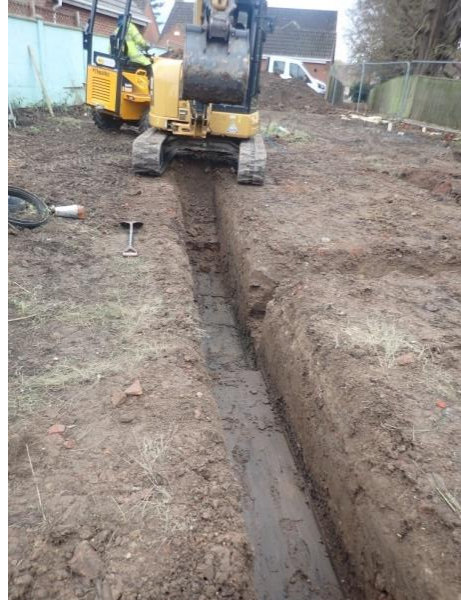
Plate 42: Excavation of the foundations, from the west
