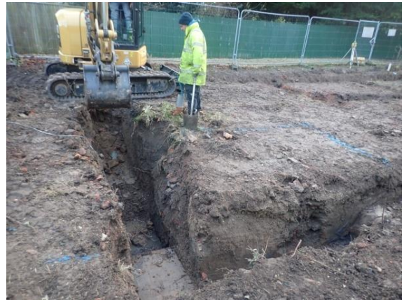
Plate 54: Excavation of the foundations, from the north
