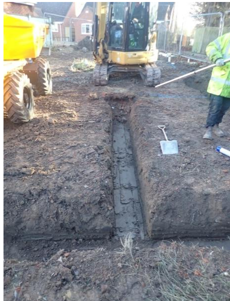
Plate 27: Excavation of the foundations, from the west
