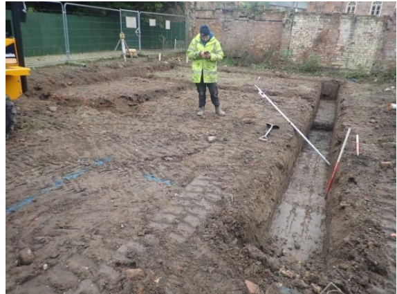
Plate 43: Excavation of the foundations, from the east
