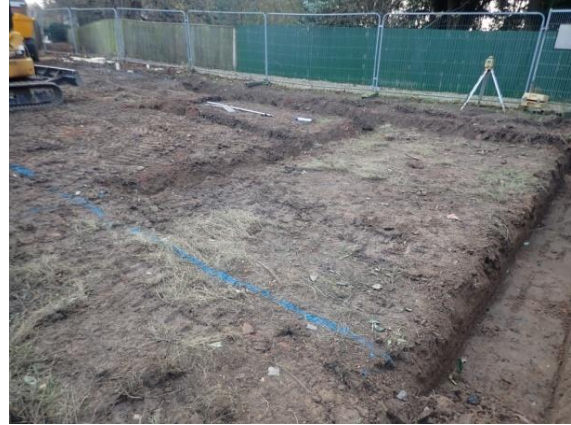
Plate 31: Excavation of the foundations, from the north
