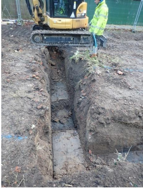
Plate 56: Excavation of the foundations, from the north
