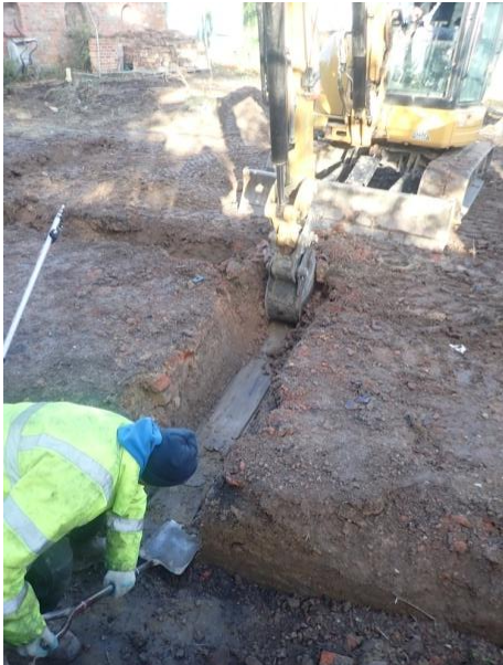
Plate 30: Excavation of the foundations, from the south
