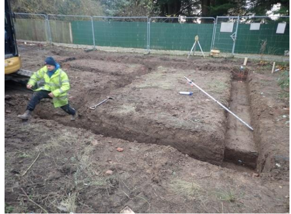
Plate 37: Excavation of the foundations, from the west
