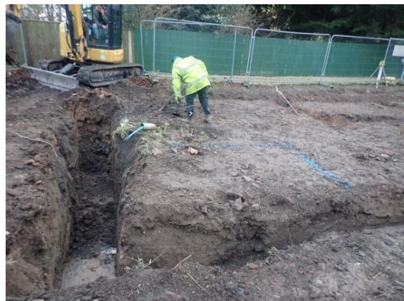
Plate 61: Excavation of the foundations, from the north
