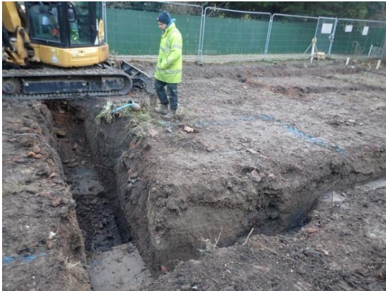
Plate 57: Excavation of the foundations, from the north
