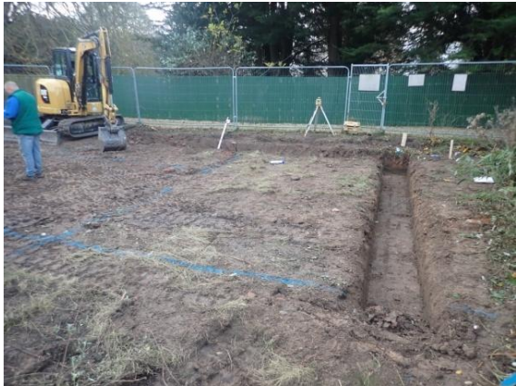
Plate 16: Excavation of the foundations, from the north
