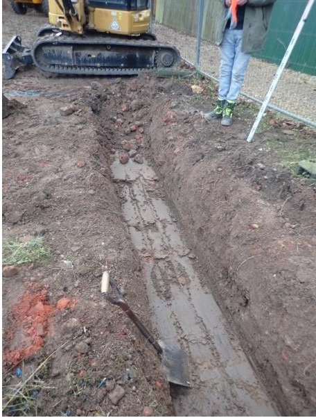
Plate 29: Excavation of the foundations, from the west
