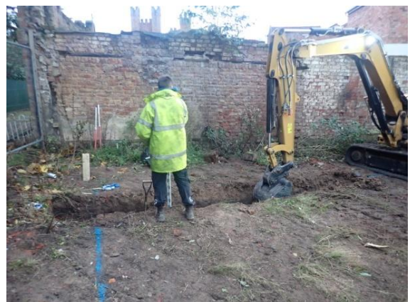
Plate 6: Excavation of the foundations, from the east
