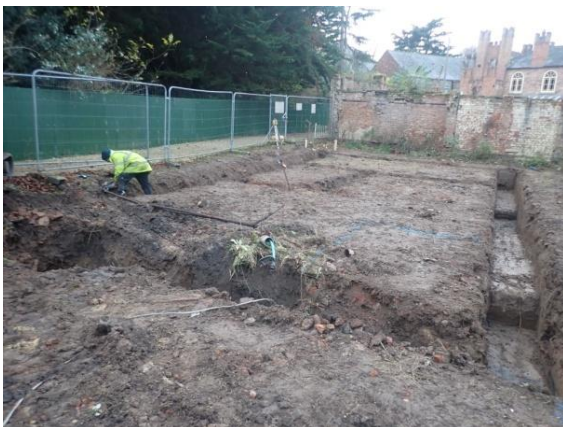
Plate 64: Excavation of the foundations, from the west
