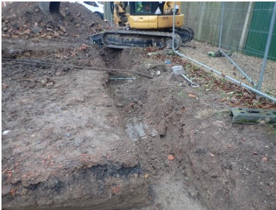
Plate 63: Excavation of the foundations, from the west
