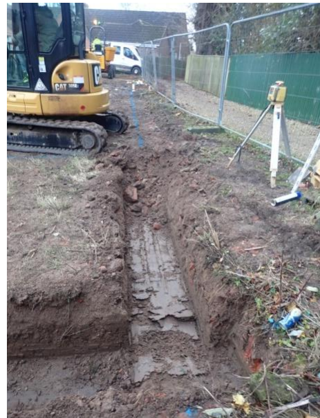
Plate 11: Excavation of the foundations, from the west
