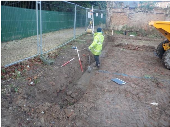
Plate 21: Excavation of the foundations, from the east
