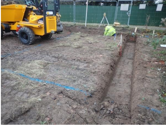
Plate 12: Excavation of the foundations, from the north
