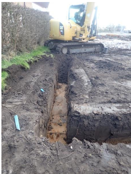
Plate 149: Excavation of the foundations, from the north
