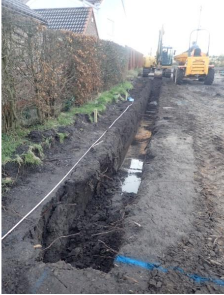
Plate 51: Excavation of the foundations, from the south
