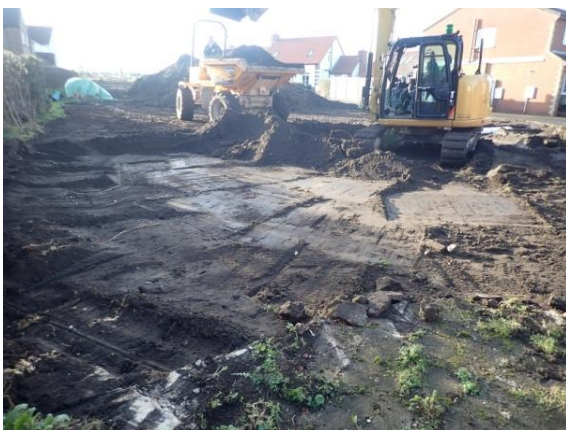
Plate 39: Further ground reduction, from the east
