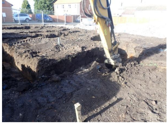
Plate 139: Excavation of the foundations, from the south-east
