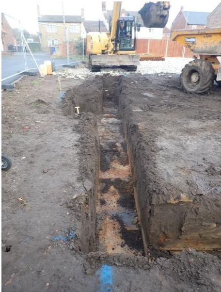
Plate 116: Excavation of the foundations, from the south
