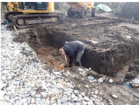
Plate 122: Excavation of the foundations, from the north-west
