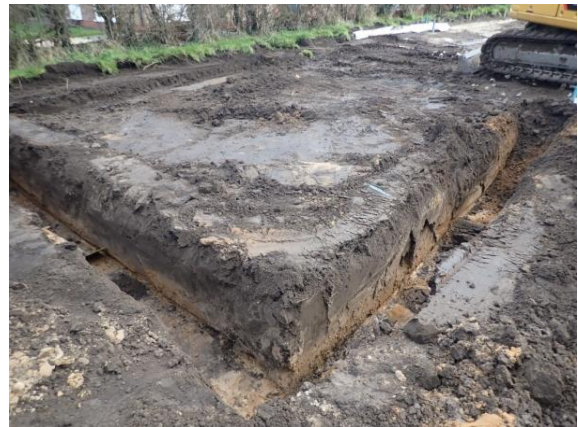
Plate 151: Excavation of the foundations, from the north-west
