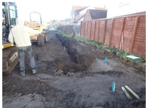
Plate 60: Excavation of the foundations, from the south
