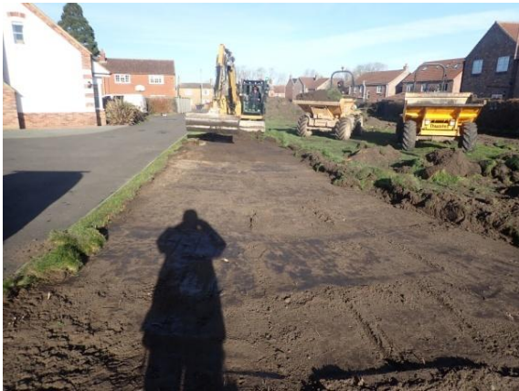
Plate 14: Initial ground reduction, from the south
