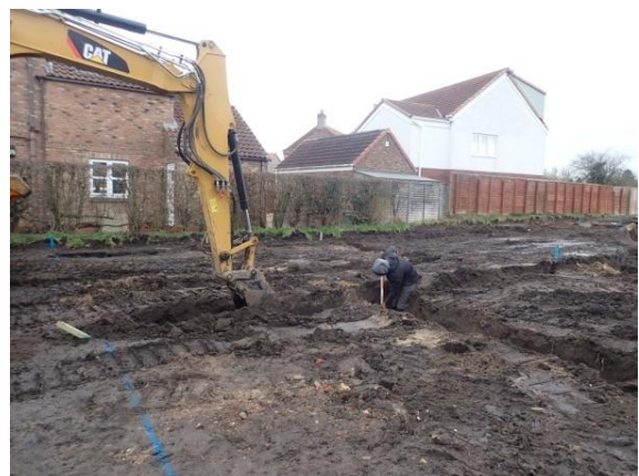
Plate 90: Excavation of the foundations, from the north-west
