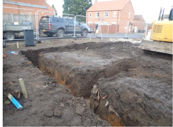
Plate 117: Excavation of the foundations, from the south-east
