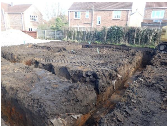
Plate 138: Excavation of the foundations, from the west
