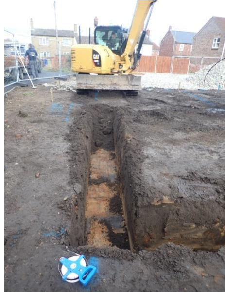
Plate 113: Excavation of the foundations, from the south
