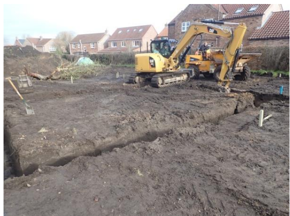
Plate 84: Excavation of the foundations, from the south-west
