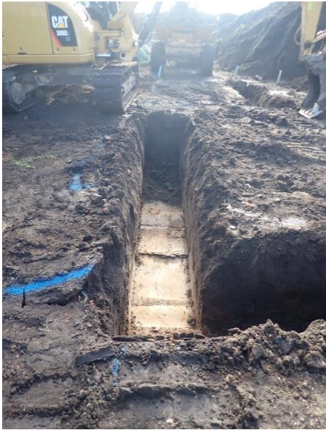
Plate 137: Excavation of the foundations, from the north
