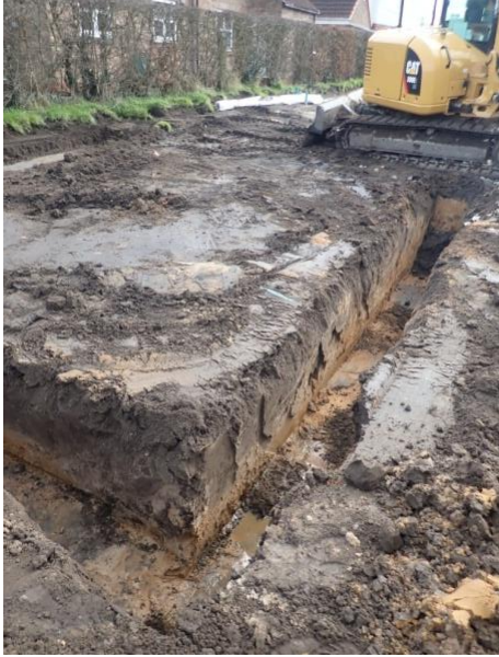
Plate 152: Excavation of the foundations, from the north
