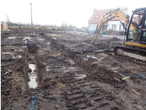
Plate 93: Excavation of the foundations, from the north
