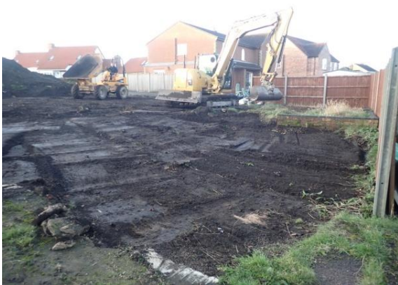
Plate 33: Initial ground reduction, from the south-east
