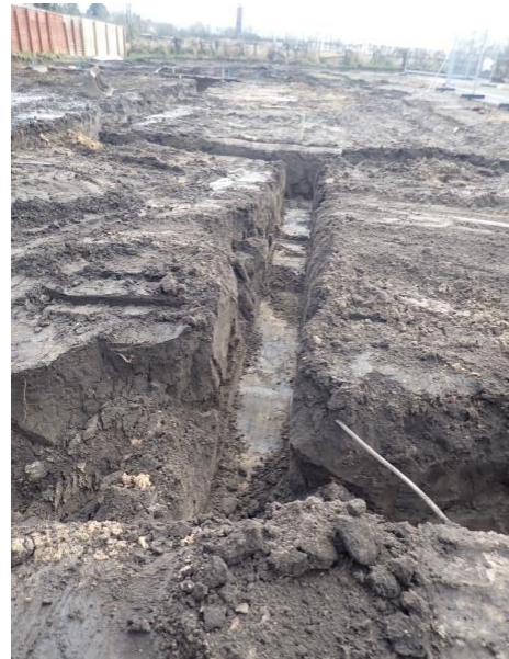
Plate 96: Excavation of the foundations, from the north
