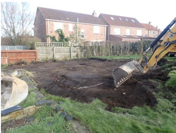
Plate 21: Initial ground reduction, from the west
