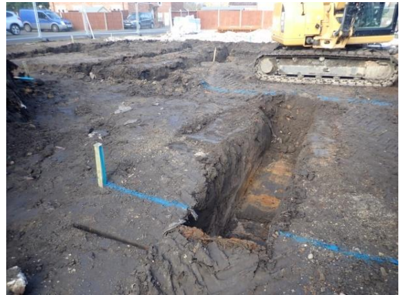
Plate 134: Excavation of the foundations, from the south
