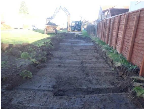
Plate 8: Initial ground reduction, from the south
