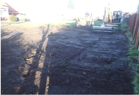
Plate 7: Initial ground reduction, from the south
