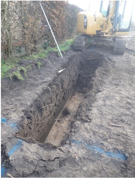
Plate 44: Excavation of the foundations, from the north
