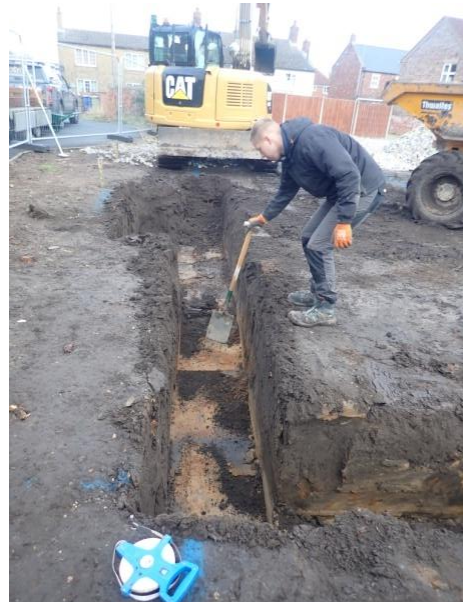
Plate 114: Excavation of the foundations, from the south
