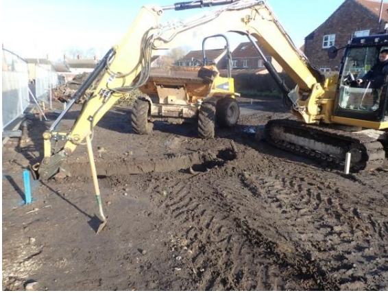
Plate 73: Excavation of the foundations, from the south
