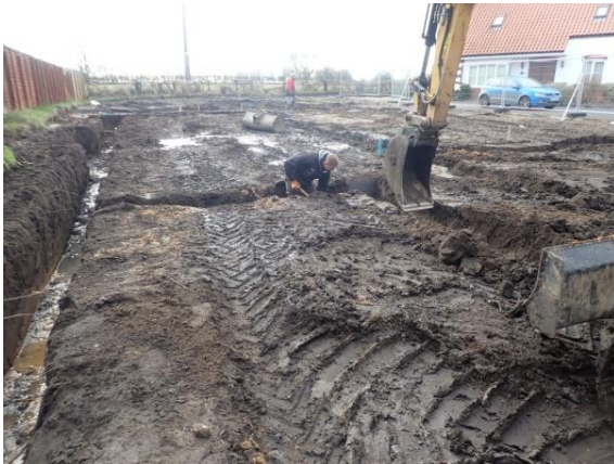
Plate 86: Excavation of the foundations, from the north
