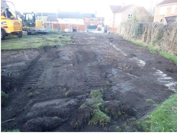
Plate 25: Initial ground reduction, from the south
