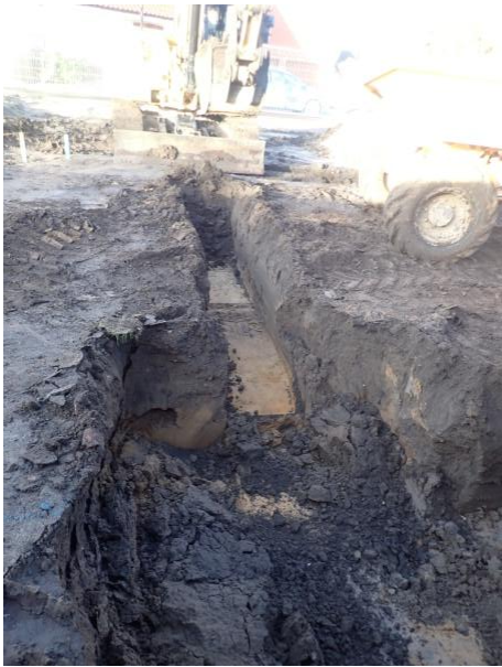
Plate 62: Excavation of the foundations, from the east
