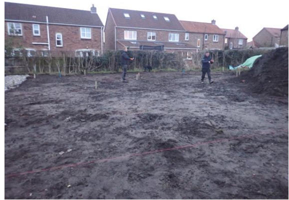
Plate 105: Set out foundations, from the west
