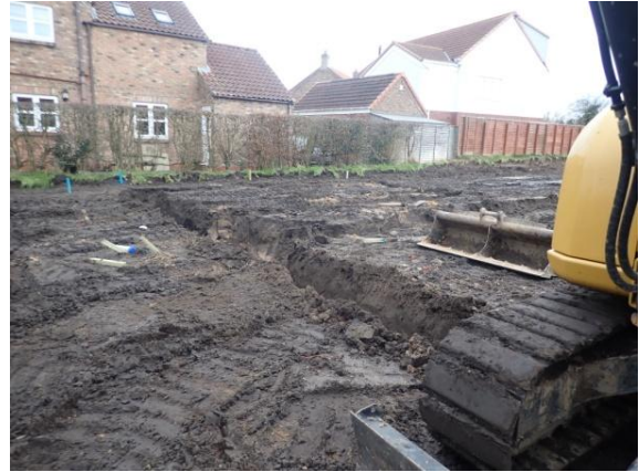
Plate 100: Excavation of the foundations, from the west
