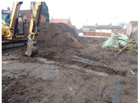
Plate 145: Excavation of the foundations, from the south
