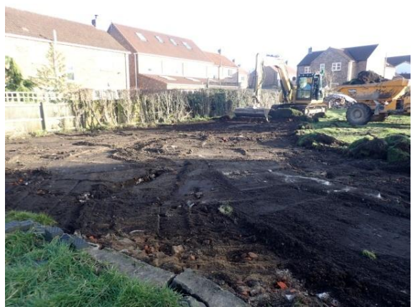
Plate 23: Initial ground reduction, from the north-west
