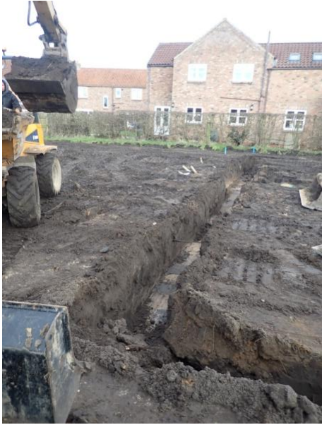
Plate 102: Excavation of the foundations, from the west
