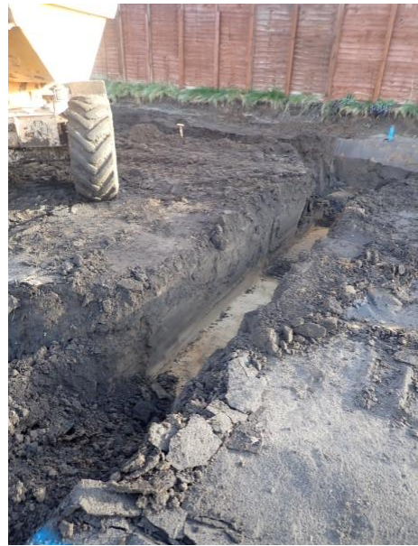
Plate 65: Excavation of the foundations, from the south-west
