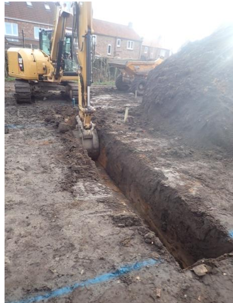
Plate 110: Excavation of the foundations, from the west
