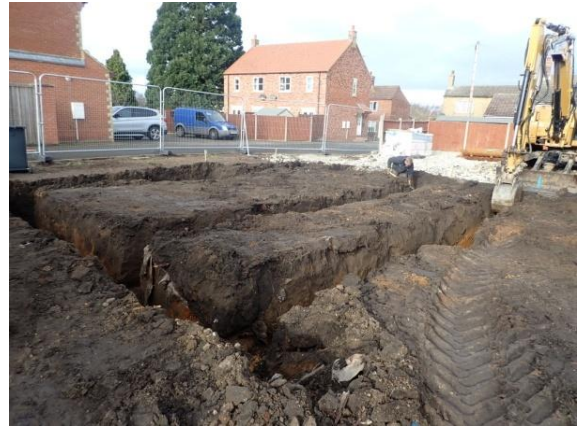
Plate 124: Excavation of the foundations, from the south-west
