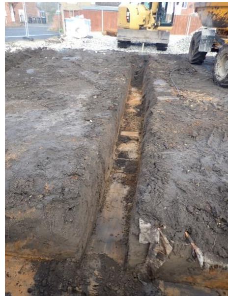
Plate 118: Excavation of the foundations, from the south
