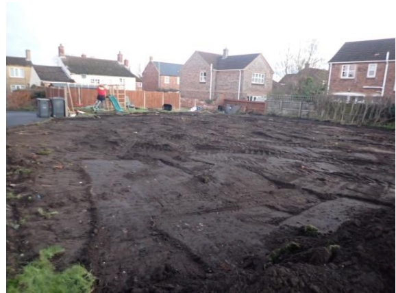
Plate 29: Initial ground reduction, from the south
