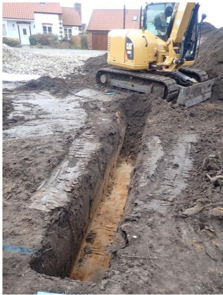
Plate 143: Excavation of the foundations, from the east
