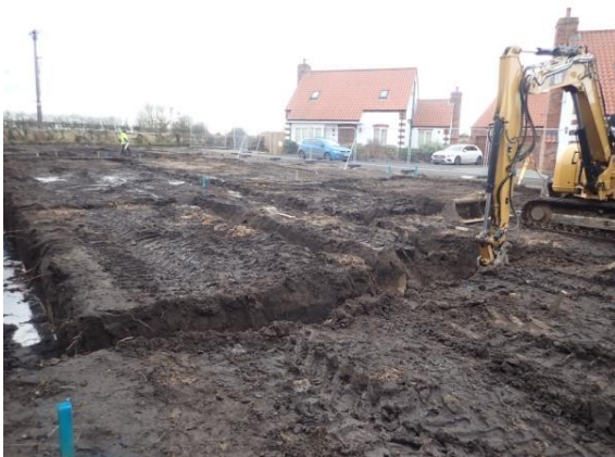
Plate 99: Excavation of the foundations, from the north
