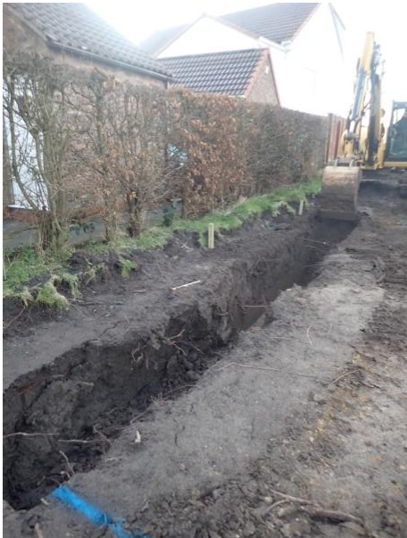
Plate 48: Excavation of the foundations, from the south
