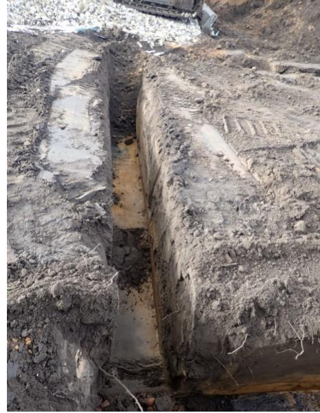
Plate 154: Excavation of the foundations, from the east
