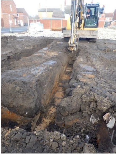
Plate 120: Excavation of the foundations, from the south
