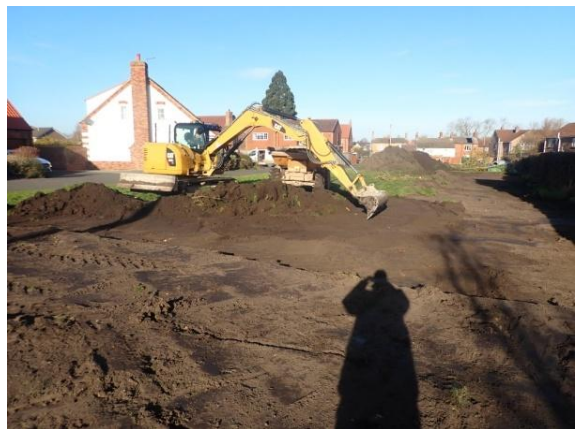
Plate 12: Initial ground reduction, from the south
