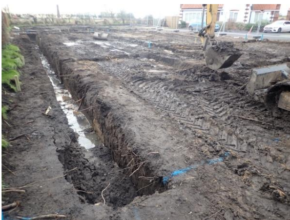
Plate 87: Excavation of the foundations, from the north
