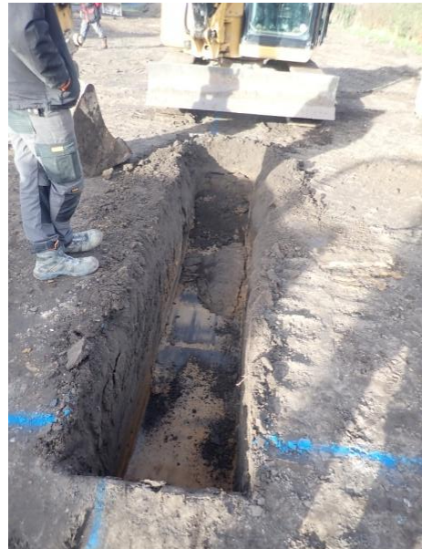
Plate 46: Excavation of the foundations, from the south
