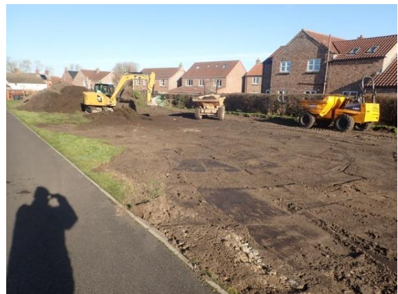
Plate 18: Initial ground reduction, from the south
