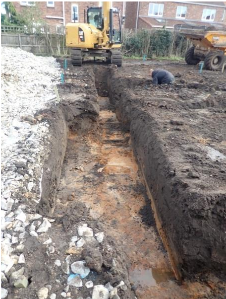
Plate 126: Excavation of the foundations, from the west
