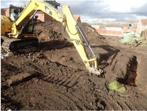
Plate 153: Excavation of the foundations, from the south
