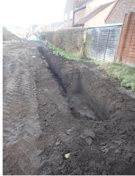
Plate 53: Excavation of the foundations, from the south
