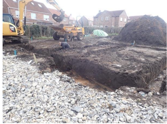
Plate 127: Excavation of the foundations, from the north-west
