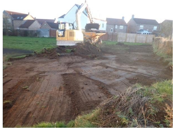
Plate 4: Initial ground reduction, from the west
