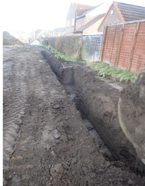
Plate 54: Excavation of the foundations, from the south
