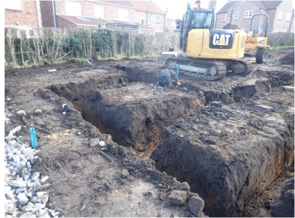
Plate 133: Excavation of the foundations, from the north-west
