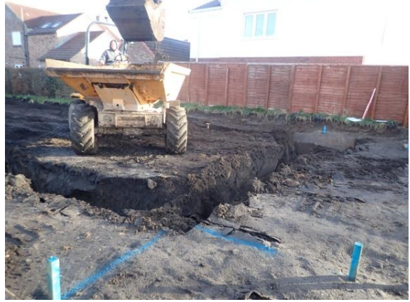
Plate 64: Excavation of the foundations, from the south-west
