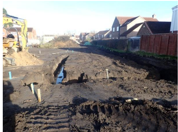
Plate 71: Excavation of the foundations, from the east
