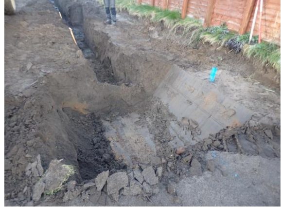
Plate 58: Excavation of the foundations, from the south
