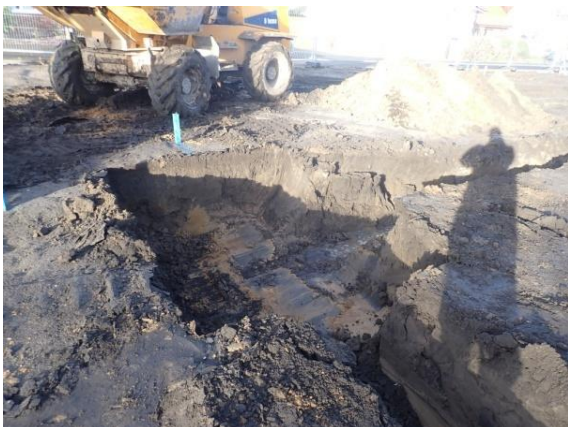
Plate 69: Excavation of the foundations, from the east
