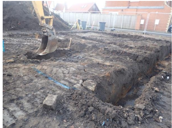
Plate 128: Excavation of the foundations, from the south-east
