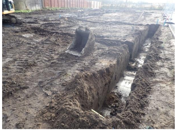
Plate 82: Excavation of the foundations, from the north
