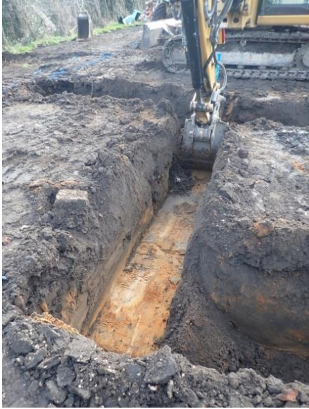
Plate 130: Excavation of the foundations, from the north
