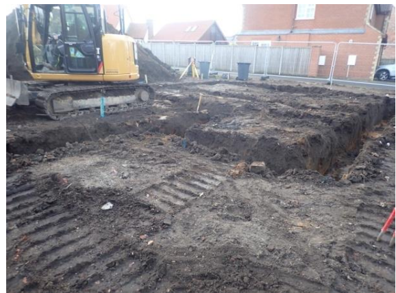
Plate 129: Excavation of the foundations, from the south-east
