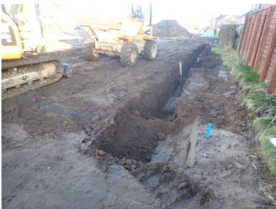
Plate 57: Excavation of the foundations, from the south
