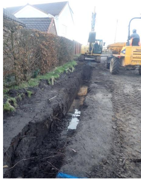
Plate 49: Excavation of the foundations, from the north
