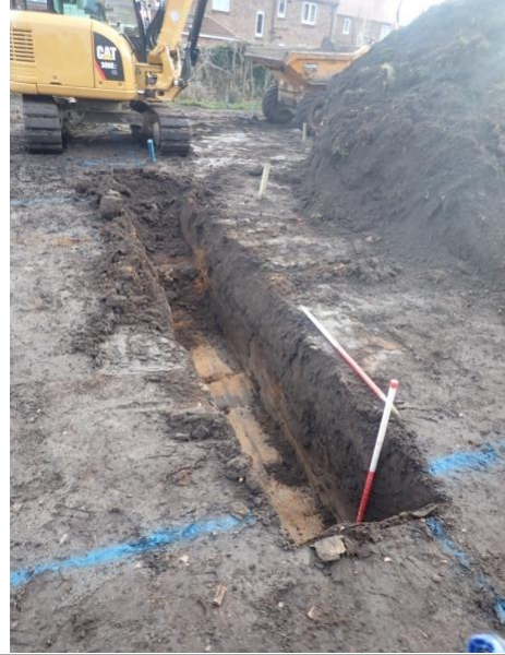
Plate 109: Excavation of the foundations, from the west
