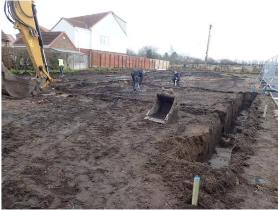
Plate 91: Excavation of the foundations, from the north
