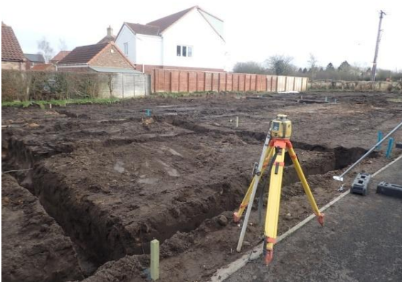
Plate 104: Excavation of the foundations, from the north-west
