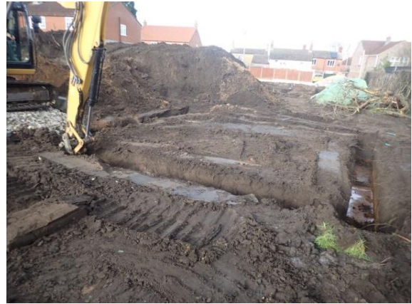
Plate 155 Excavation of the foundations, from the south
