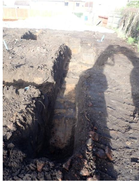
Plate 140: Excavation of the foundations, from the south
