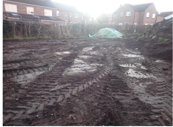
Plate 28: Initial ground reduction, from the north-west
