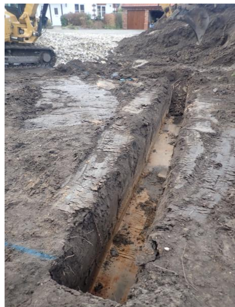
Plate 146: Excavation of the foundations, from the east
