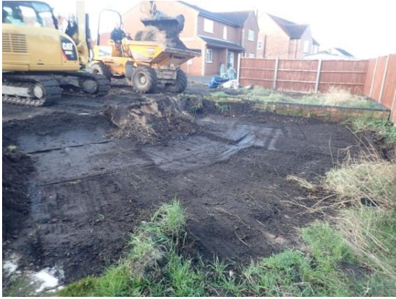
Plate 31: Initial ground reduction, from the south-east
