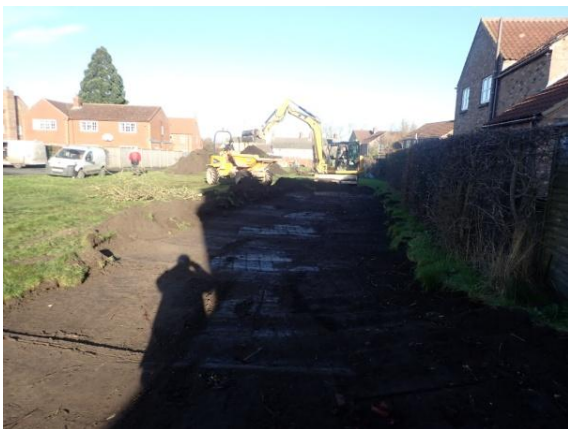
Plate 9: Initial ground reduction, from the south
