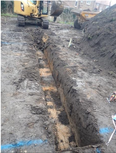
Plate 112: Excavation of the foundations, from the west
