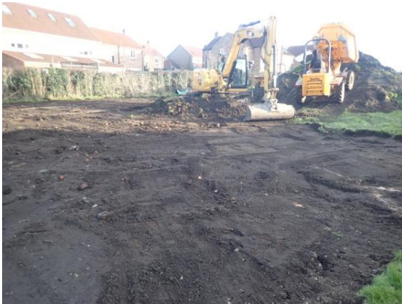
Plate 26: Initial ground reduction, from the south
