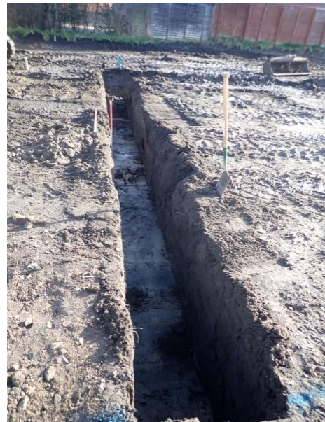
Plate 77: Excavation of the foundations, from the west
