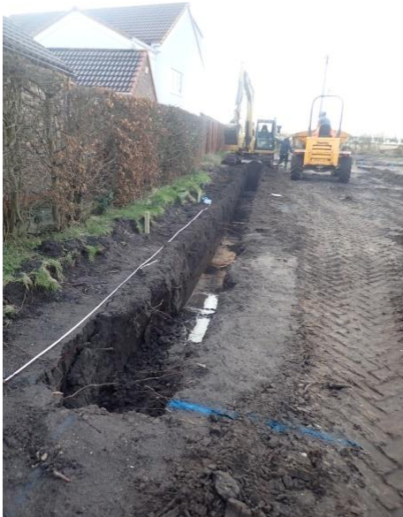
Plate 52: Excavation of the foundations, from the north
