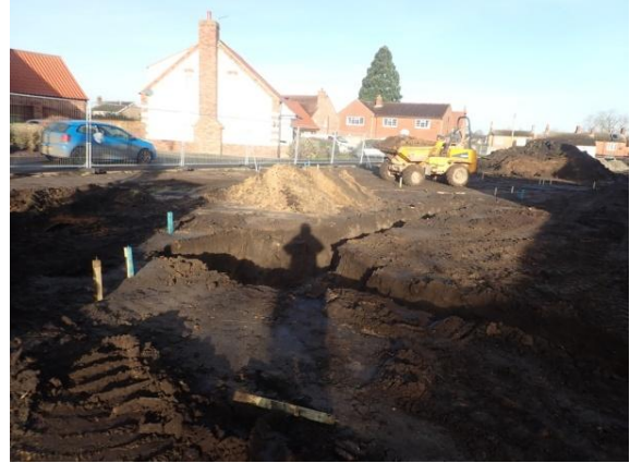
Plate 70: Excavation of the foundations, from the east
