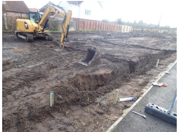
Plate 83: Excavation of the foundations, from the north-west
