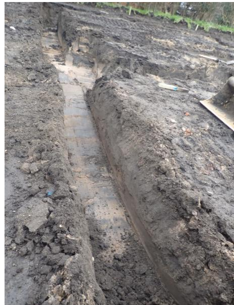
Plate 101: Excavation of the foundations, from the west
