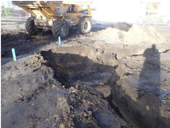
Plate 68: Excavation of the foundations, from the east
