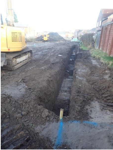
Plate 55: Excavation of the foundations, from the south
