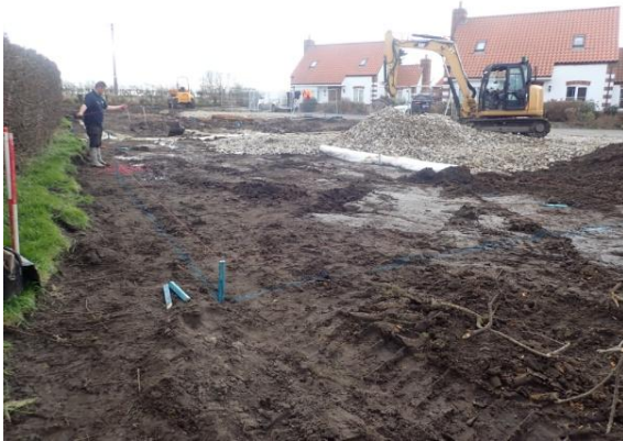
Plate 142: Set out foundations, from the south
