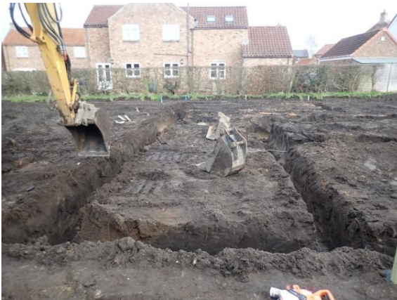
Plate 103: Excavation of the foundations, from the west
