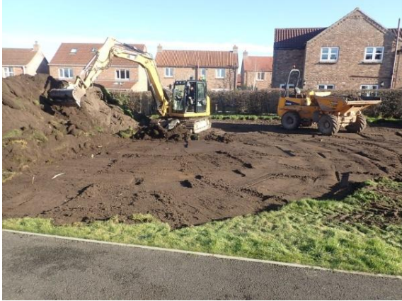
Plate 19: Initial ground reduction, from the west
