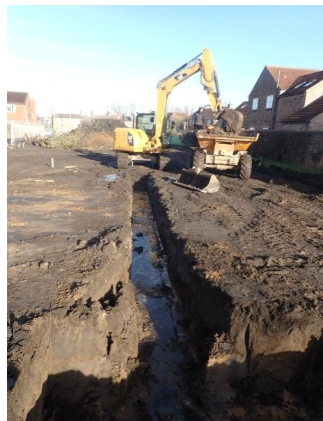
Plate 72: Excavation of the foundations, from the south
