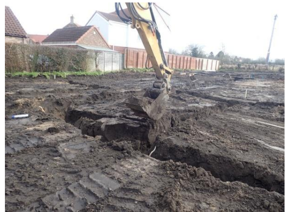
Plate 95: Excavation of the foundations, from the north-west
