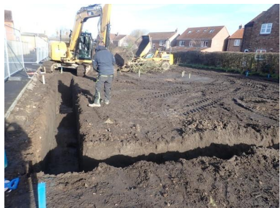
Plate 78: Excavation of the foundations, from the south
