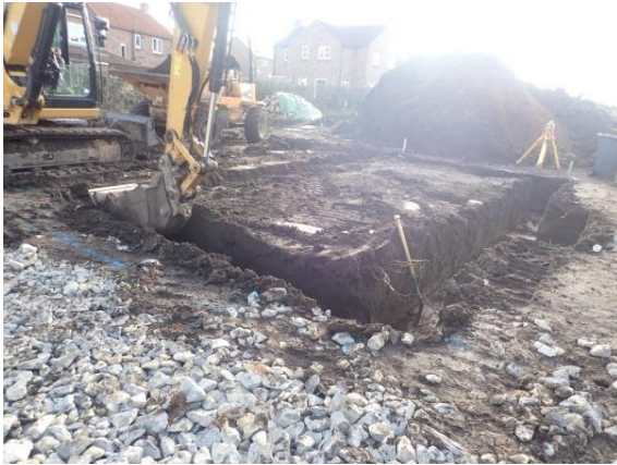
Plate 121: Excavation of the foundations, from the north-west
