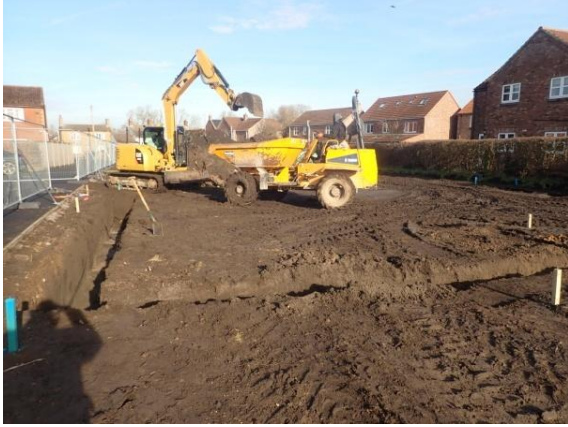
Plate 79: Excavation of the foundations, from the south
