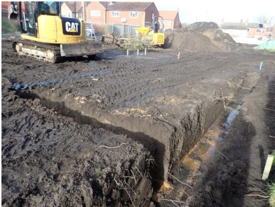
Plate 80: Excavation of the foundations, from the south
