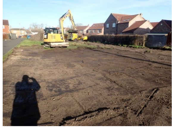
Plate 16: Initial ground reduction, from the south
