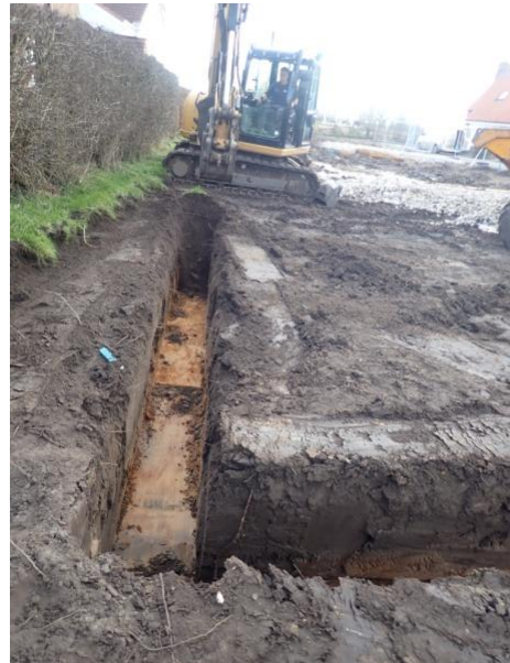
Plate 150: Excavation of the foundations, from the north
