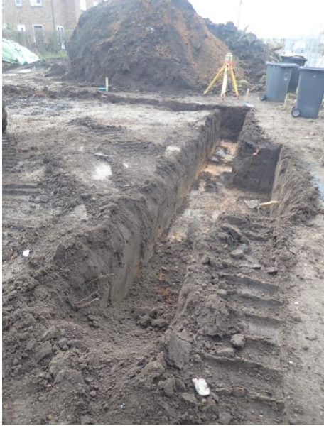
Plate 115: Excavation of the foundations, from the north
