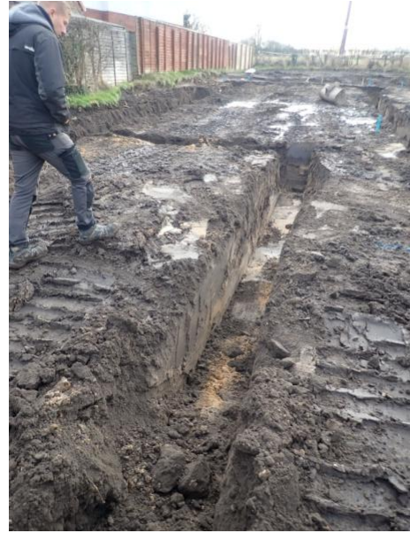
Plate 88: Excavation of the foundations, from the north
