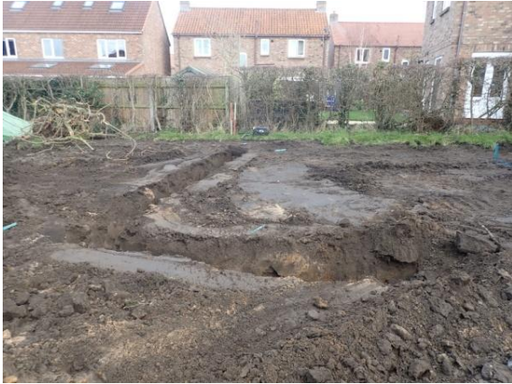
Plate 147: Excavation of the foundations, from the west
