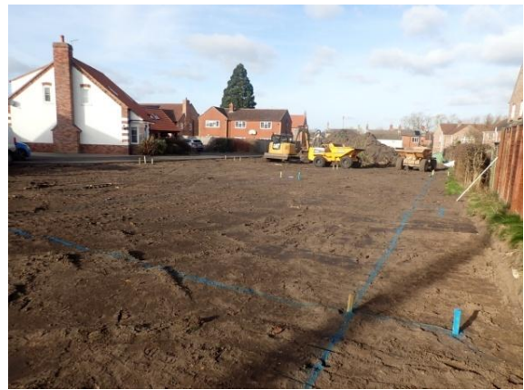
Plate 42: Set out foundations, from the south
