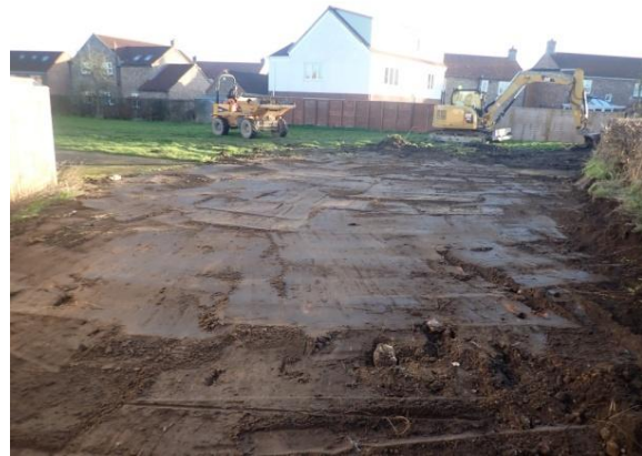
Plate 5: Initial ground reduction, from the west
