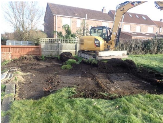
Plate 20: Initial ground reduction, from the west
