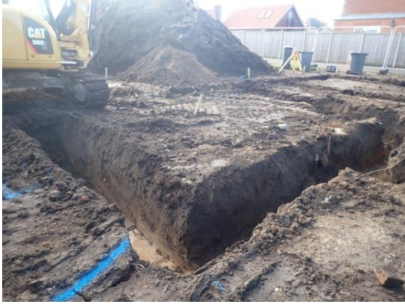
Plate 136: Excavation of the foundations, from the north-east
