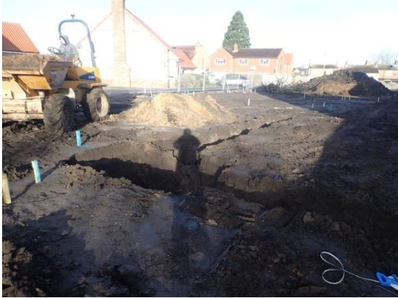
Plate 67: Excavation of the foundations, from the south
