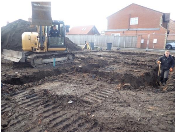
Plate 131: Excavation of the foundations, from the east
