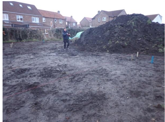
Plate 106: Set out foundations, from the north-west
