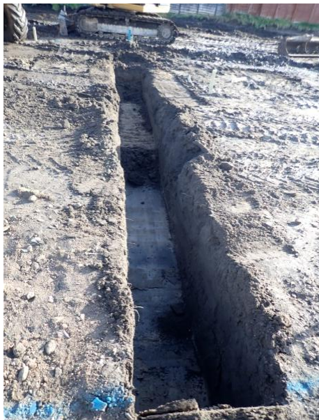
Plate 75: Excavation of the foundations, from the west
