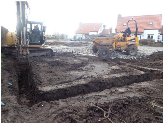
Plate 148: Excavation of the foundations, from the north
