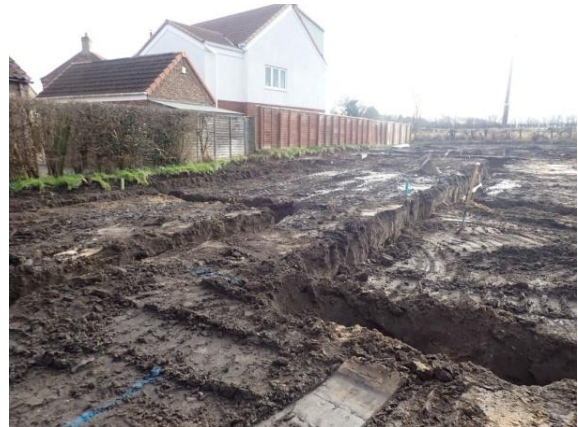
Plate 89: Excavation of the foundations, from the north
