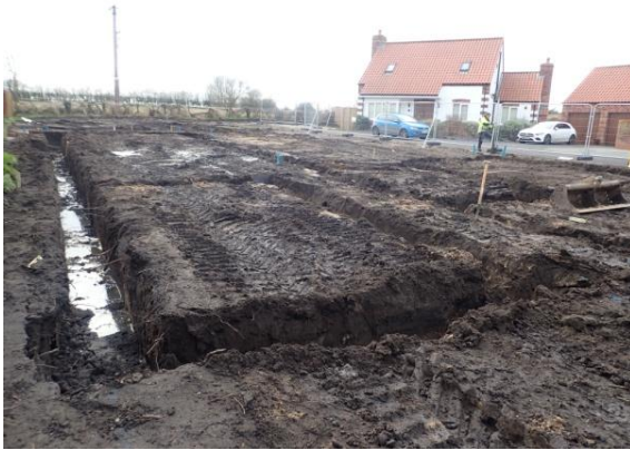
Plate 97: Excavation of the foundations, from the north
