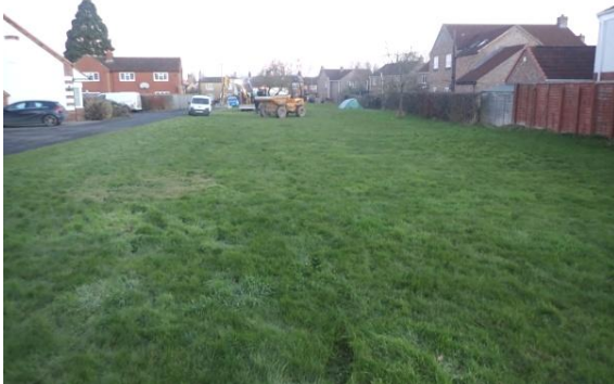
Plate 2: Pre- groundworks, from the south
