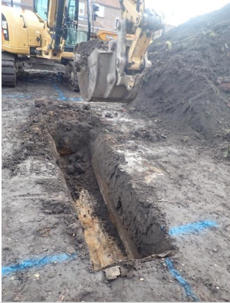
Plate 107: Excavation of the foundations, from the west
