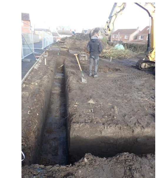
Plate 81: Excavation of the foundations, from the south
