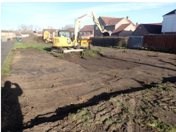
Plate 15: Initial ground reduction, from the south
