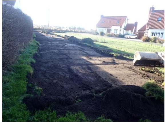
Plate 10: Initial ground reduction, from the north
