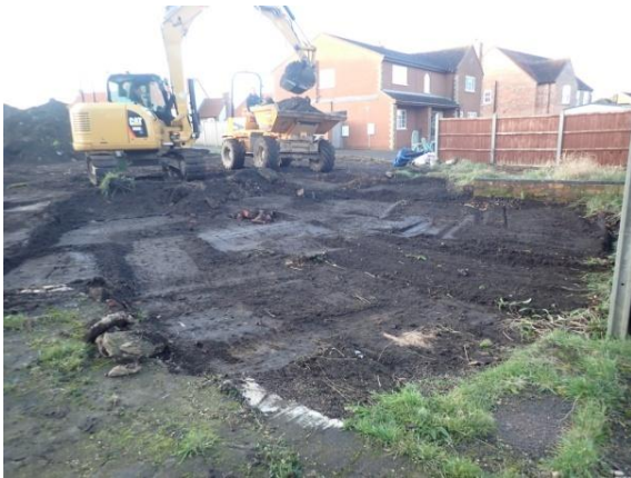
Plate 32: Initial ground reduction, from the south-east
