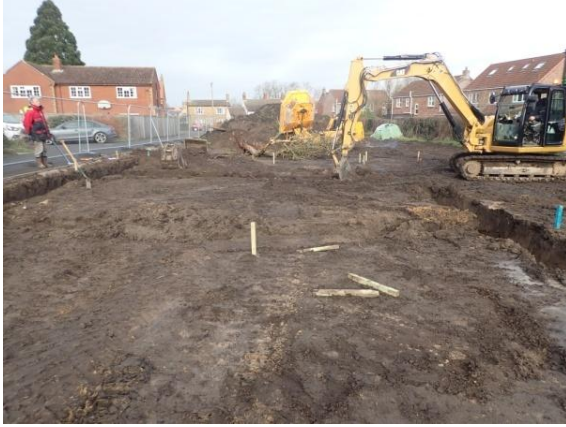
Plate 85: Excavation of the foundations, from the south
