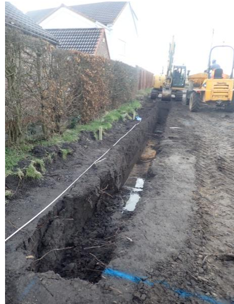
Plate 50: Excavation of the foundations, from the north
