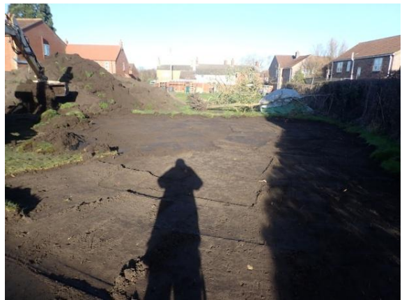
Plate 11: Initial ground reduction, from the south
