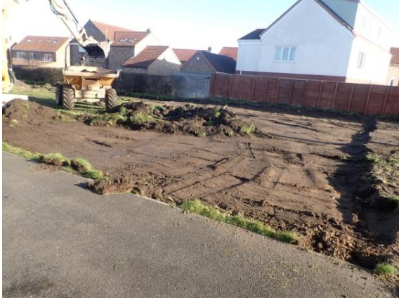
Plate 13: Initial ground reduction, from the west
