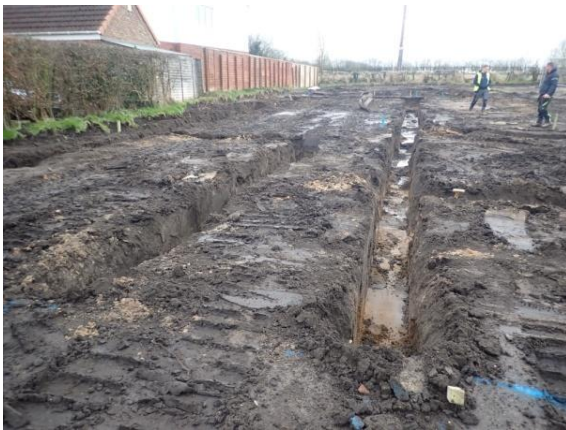
Plate 92: Excavation of the foundations, from the north
