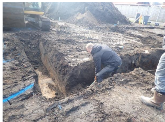
Plate 135: Excavation of the foundations, from the north
