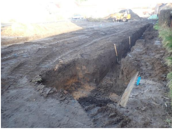
Plate 61: Excavation of the foundations, from the south
