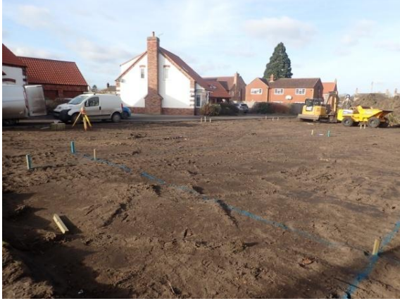
Plate 43: Set out foundations, from the south-east
