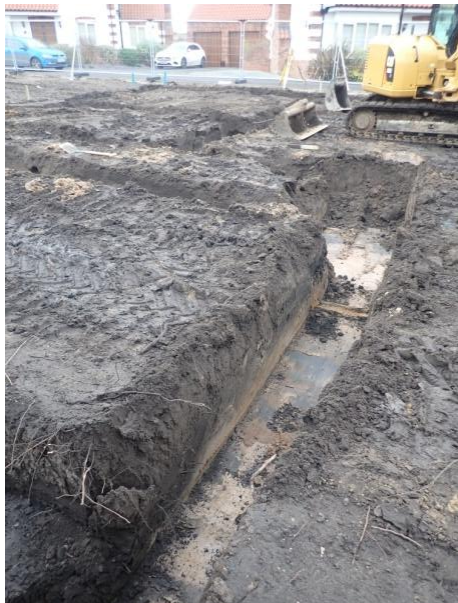
Plate 98: Excavation of the foundations, from the north
