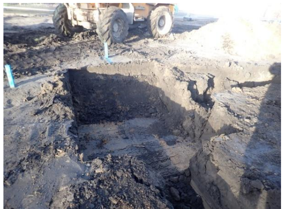
Plate 66: Excavation of the foundations, from the east
