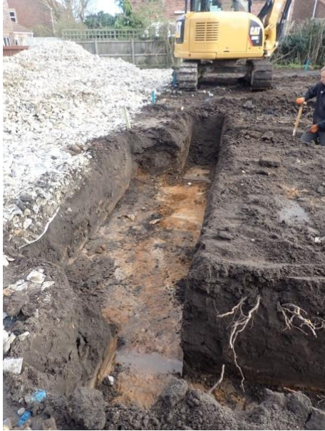
Plate 125: Excavation of the foundations, from the west
