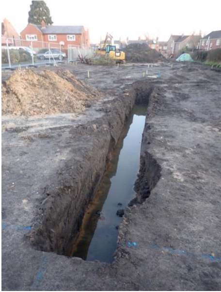
Plate 47: Excavation of the foundations, from the south
