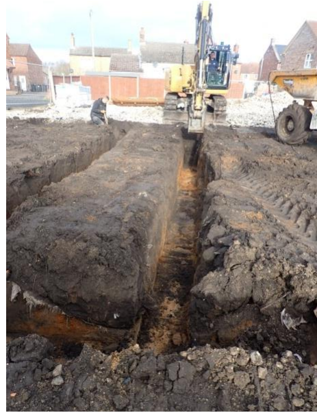
Plate 123: Excavation of the foundations, from the south
