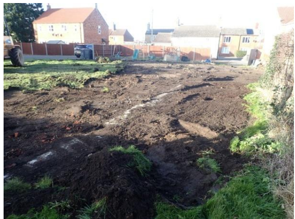
Plate 24: Initial ground reduction, from the south
