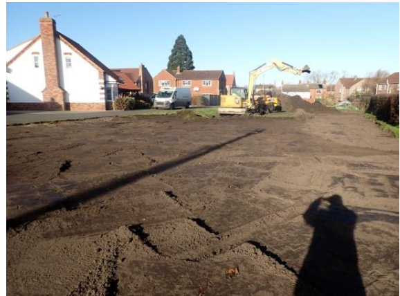
Plate 17: Initial ground reduction, from the south
