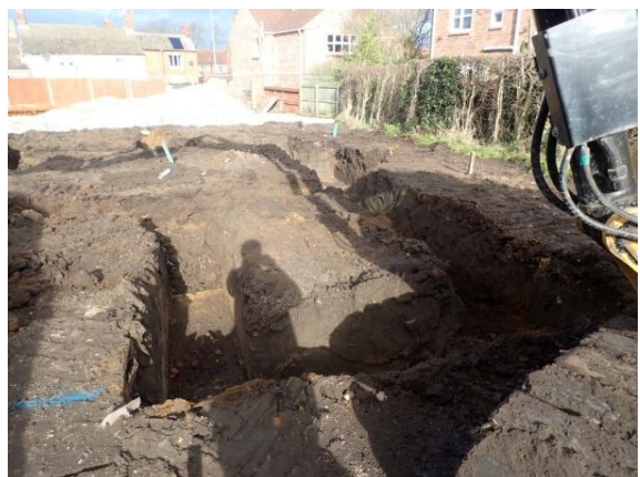
Plate 141: Excavation of the foundations, from the south
