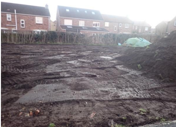
Plate 27: Initial ground reduction, from the west
