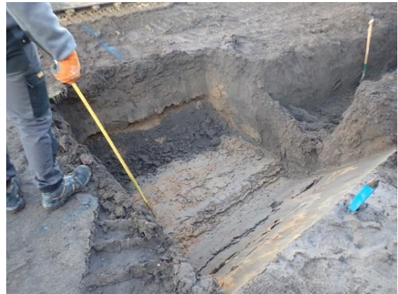
Plate 59: Excavation of the foundations, from the east
