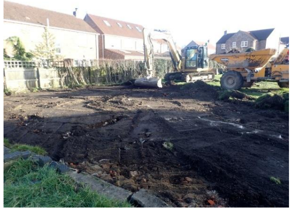
Plate 22: Initial ground reduction, from the north-west
