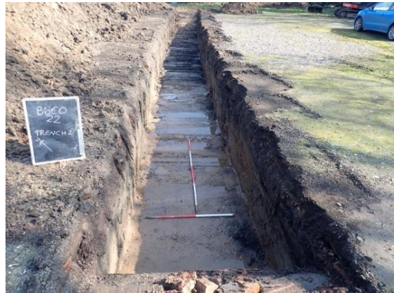
Plate 14: Trench 2, from the south-west
