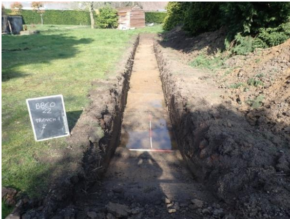
Plate 8: Trench 1, from the south-east
