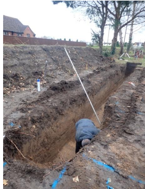
Plate 46: Excavation of the foundations, from the north
