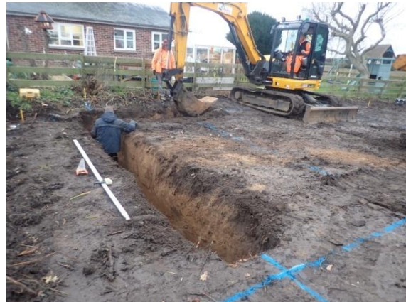
Plate 10: Excavation of the foundations, from the north
