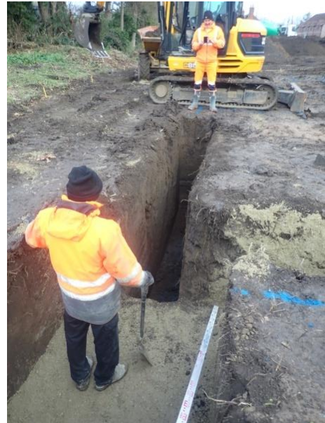
Plate 120: Excavation of the foundations, from the south
