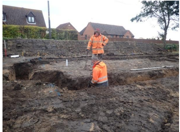
Plate 85: Excavation of the foundations, from the west
