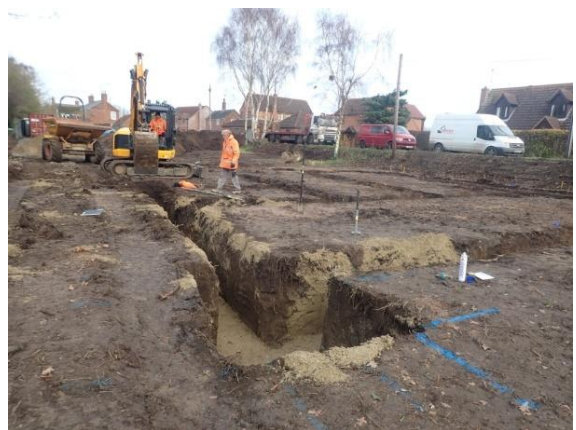
Plate 137: Excavation of the foundations, from the south
