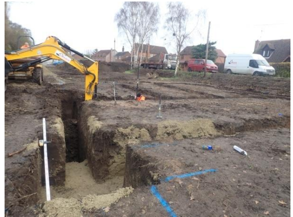
Plate 125: Excavation of the foundations, from the south
