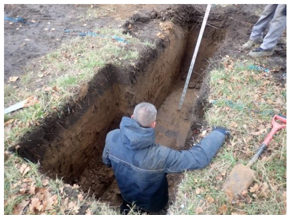
Plate 38: Excavation of the foundations, from the south
