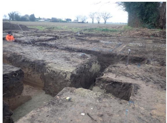
Plate 148: Excavation of the foundations, from the east
