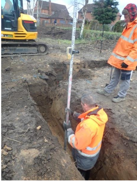
Plate 86: Excavation of the foundations, from the north
