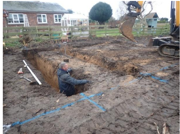
Plate 19: Excavation of the foundations, from the north
