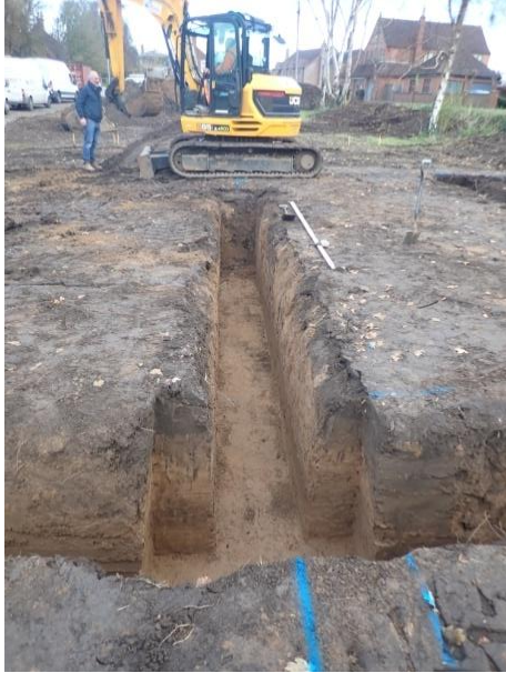
Plate 76: Excavation of the foundations, from the south
