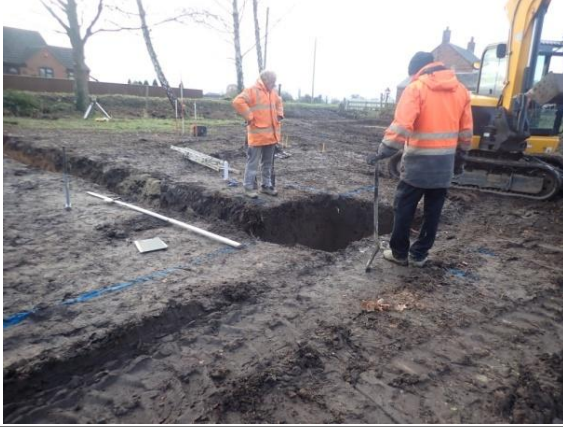
Plate 113: Excavation of the foundations, from the north-west
