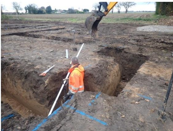
Plate 83: Excavation of the foundations, from the east
