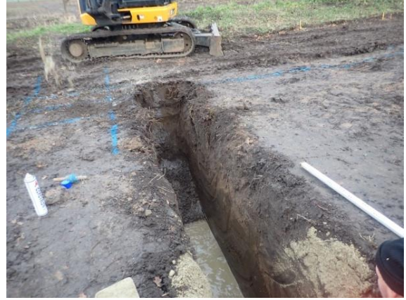
Plate 101: Excavation of the foundations, from the east
