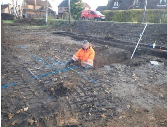
Plate 59: Excavation of the foundations, from the south
