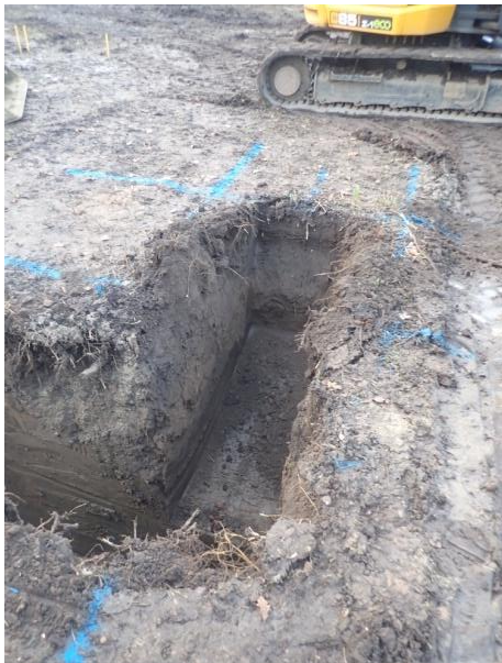
Plate 108: Excavation of the foundations, from the west
