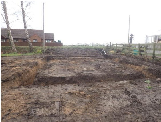
Plate 34: Excavation of the foundations, from the west
