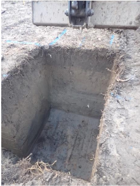
Plate 114: Excavation of the foundations, from the north
