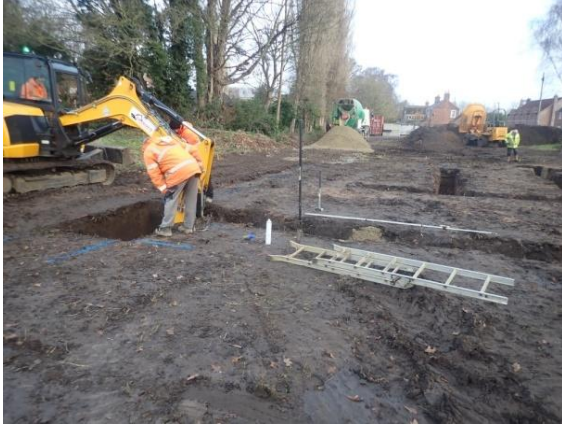
Plate 117: Excavation of the foundations, from the south
