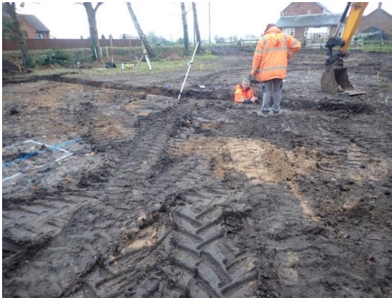
Plate 54: Excavation of the foundations, from the north
