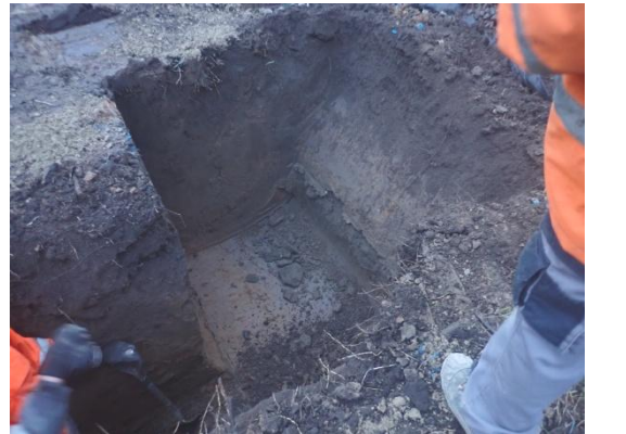
Plate 159: Excavation of the foundations, from the north
