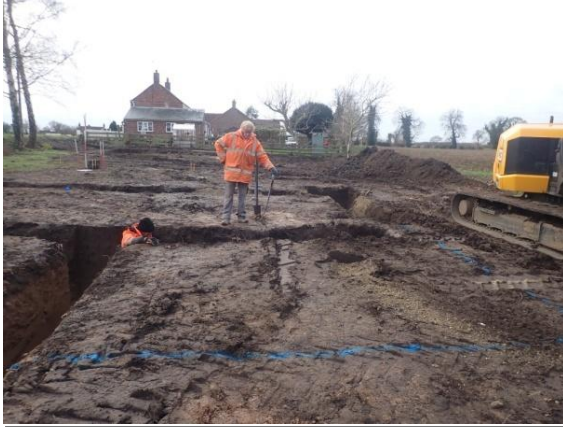
Plate 121: Excavation of the foundations, from the north
