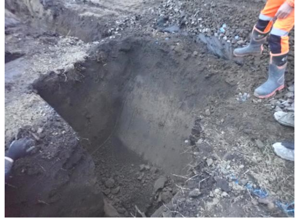
Plate 158: Excavation of the foundations, from the north-east
