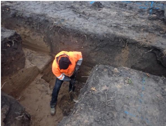
Plate 93: Excavation of the foundations, from the east
