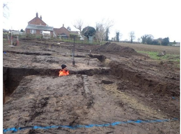
Plate 126: Excavation of the foundations, from the north
