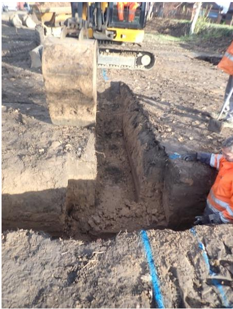
Plate 72: Excavation of the foundations, from the south
