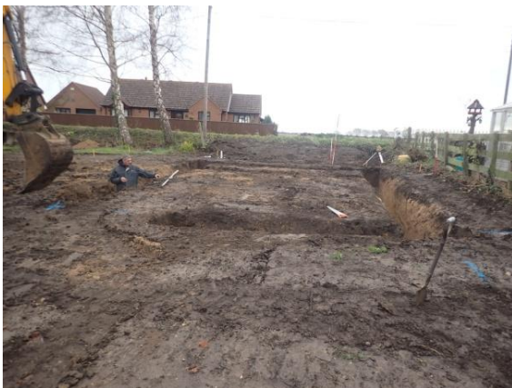
Plate 29: Excavation of the foundations, from the west
