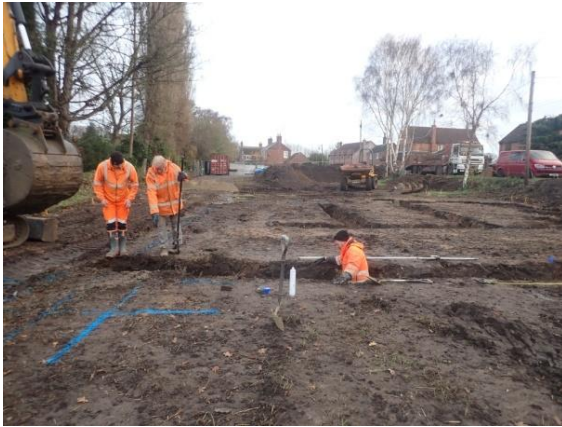
Plate 104: Excavation of the foundations, from the south
