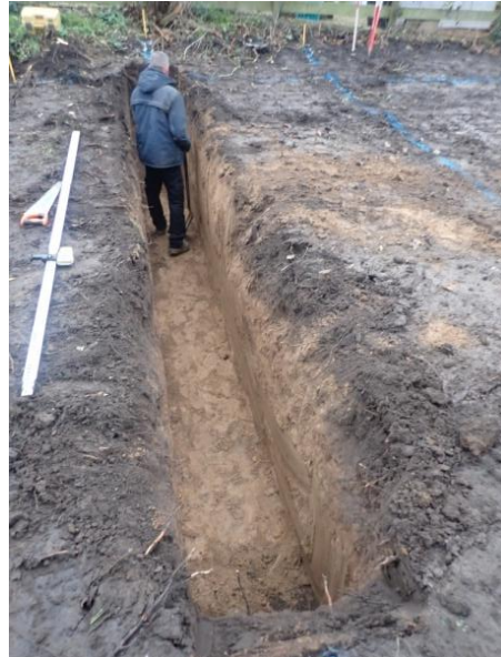
Plate 9: Excavation of the foundations, from the north
