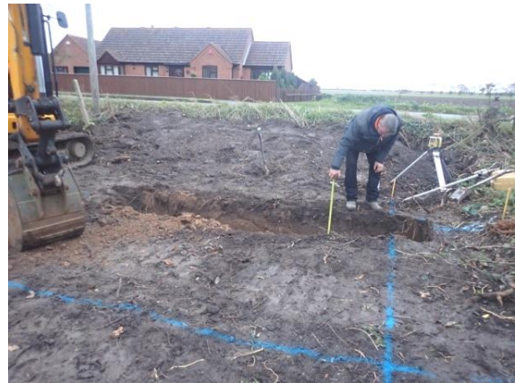
Plate 5: Excavation of the foundations, from the west
