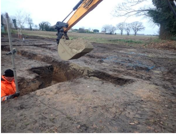
Plate 98: Excavation of the foundations, from the north-east
