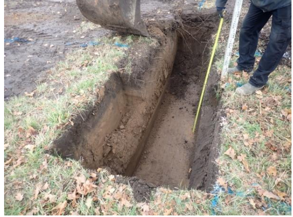
Plate 36: Excavation of the foundations, from the south
