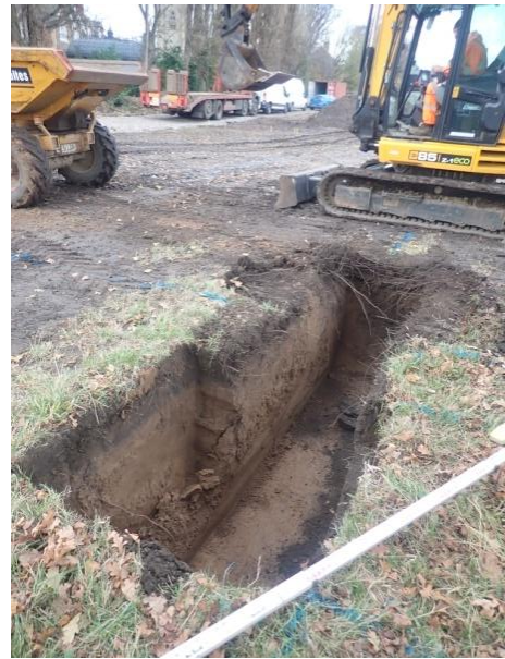
Plate 37: Excavation of the foundations, from the south
