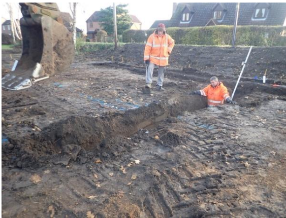
Plate 60: Excavation of the foundations, from the south-west
