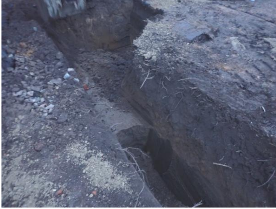
Plate 161: Excavation of the foundations, from the south
