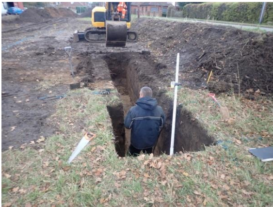
Plate 40: Excavation of the foundations, from the south
