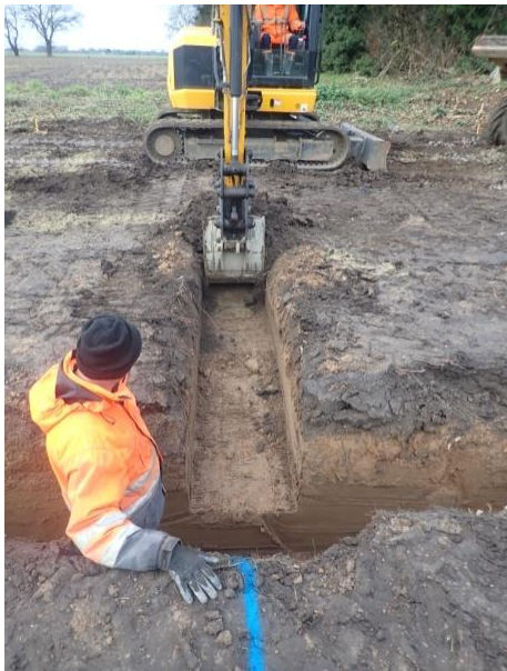
Plate 128 Excavation of the foundations, from the east
