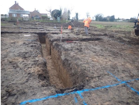
Plate 133: Excavation of the foundations, from the north
