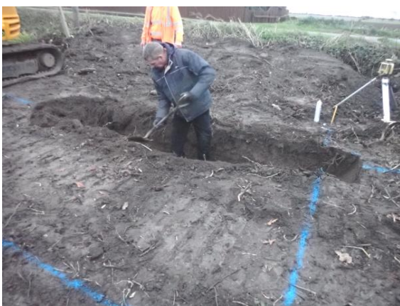
Plate 3: Excavation of the foundations, from the west
