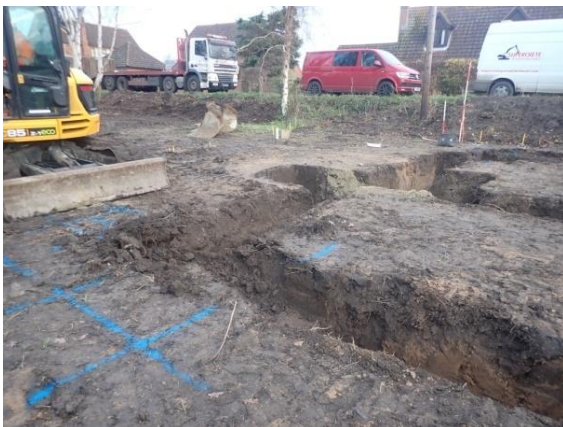
Plate 145: Excavation of the foundations, from the south-east
