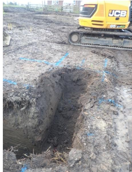
Plate 106: Excavation of the foundations, from the north
