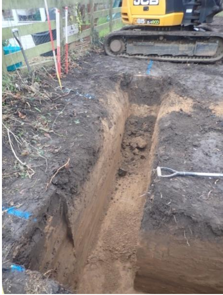
Plate 11: Excavation of the foundations, from the north
