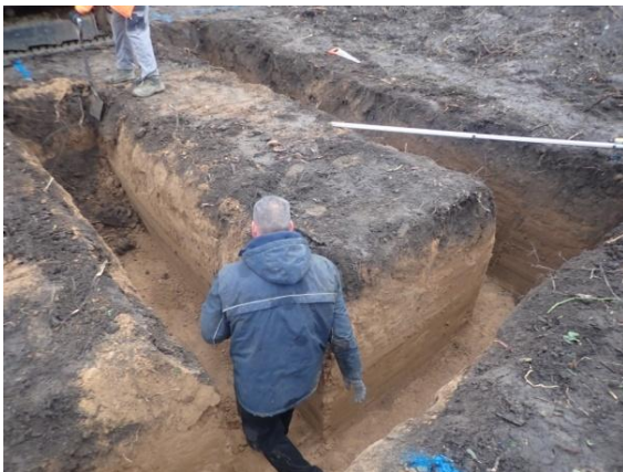
Plate 17: Excavation of the foundations, from the south-west
