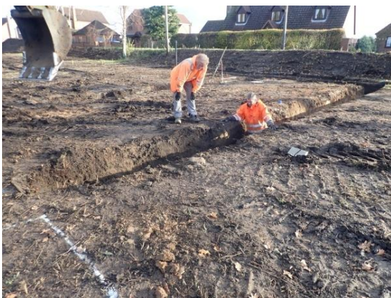
Plate 67: Excavation of the foundations, from the south-west
