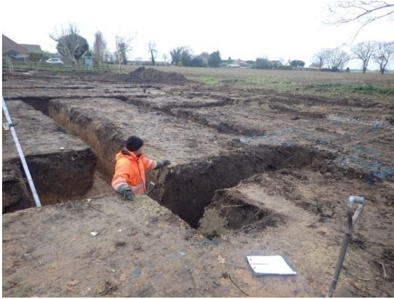
Plate 144: Excavation of the foundations, from the north-east
