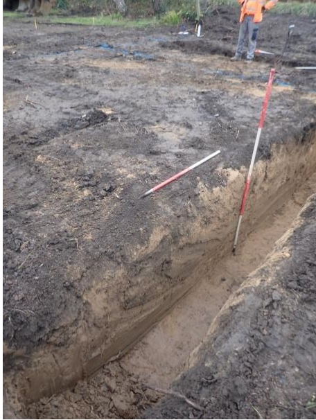
Plate 15: Representative Section 2, from the south-west
