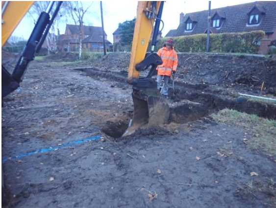
Plate 48: Excavation of the foundations, from the south
