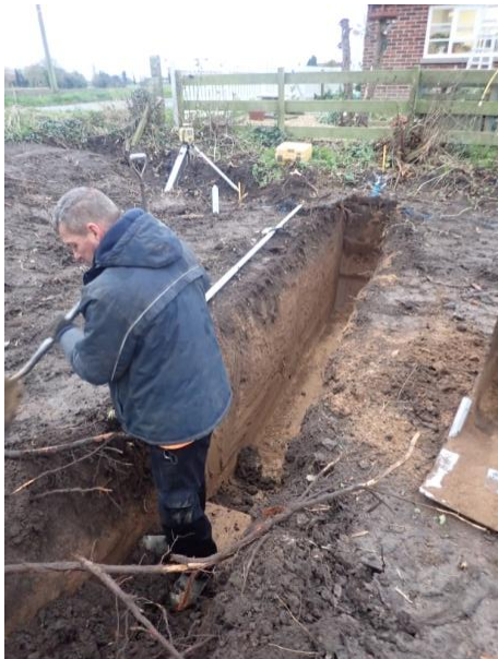
Plate 8: Excavation of the foundations, from the north
