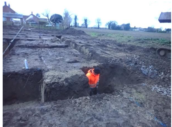
Plate 160: Excavation of the foundations, from the north
