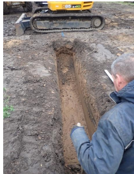
Plate 26: Excavation of the foundations, from the south
