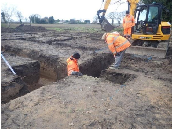
Plate 143: Excavation of the foundations, from the north-east
