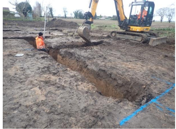
Plate 129: Excavation of the foundations, from the north-east
