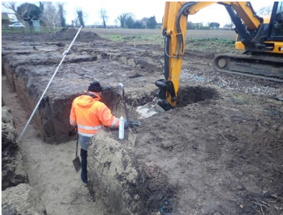
Plate 156: Excavation of the foundations, from the north
