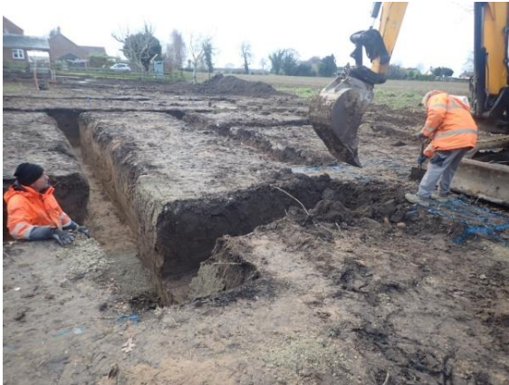
Plate 139: Excavation of the foundations, from the north
