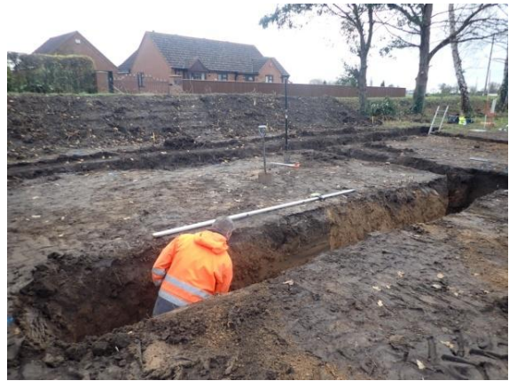
Plate 75: Excavation of the foundations, from the north-west
