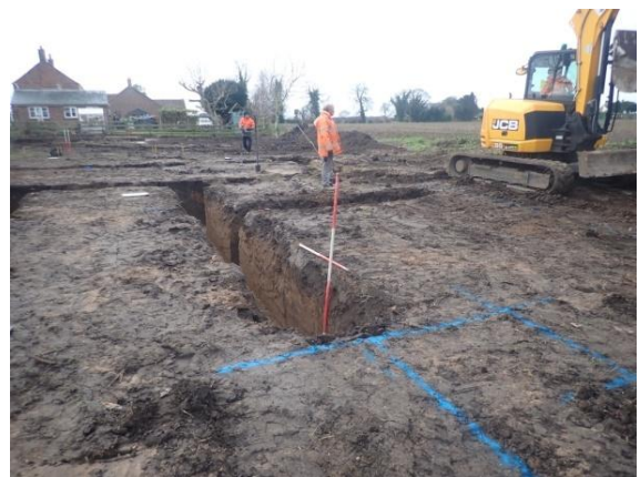
Plate 131: Excavation of the foundations, from the north
