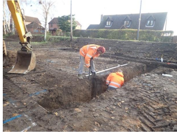
Plate 62: Excavation of the foundations, from the south-west
