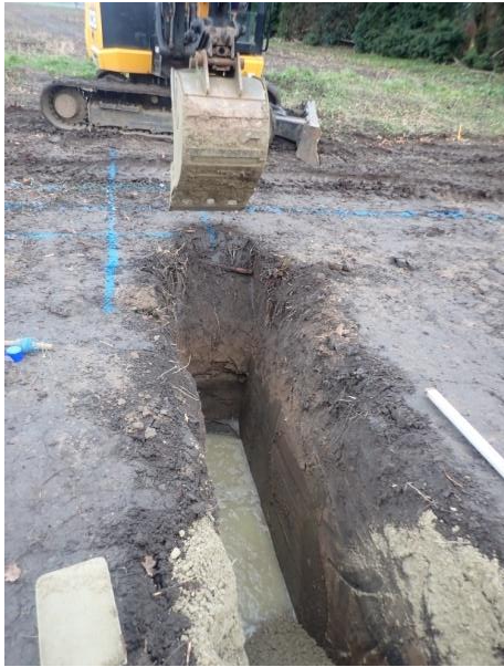
Plate 99: Excavation of the foundations, from the east
