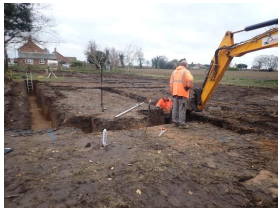
Plate 91: Excavation of the foundations, from the north
