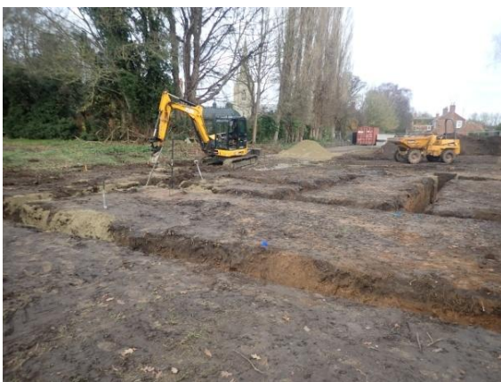
Plate 134: Excavation of the foundations, from the south
