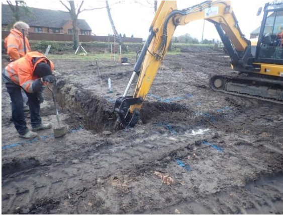
Plate 107: Excavation of the foundations, from the west
