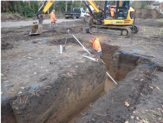
Plate 82: Excavation of the foundations, from the north-east
