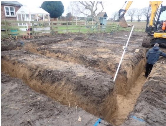
Plate 22: Excavation of the foundations, from the east
