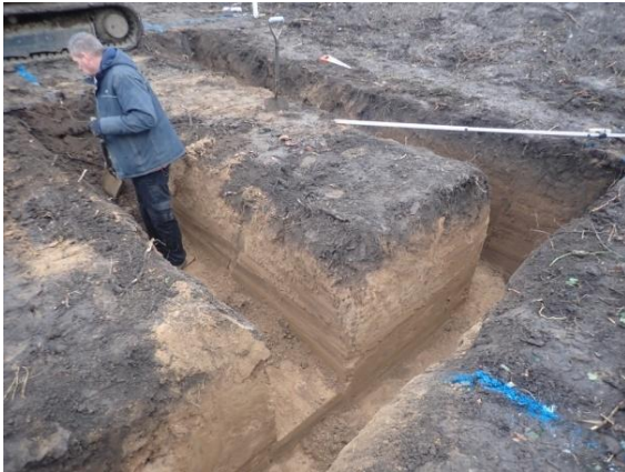
Plate 16: Excavation of the foundations, from the south-west
