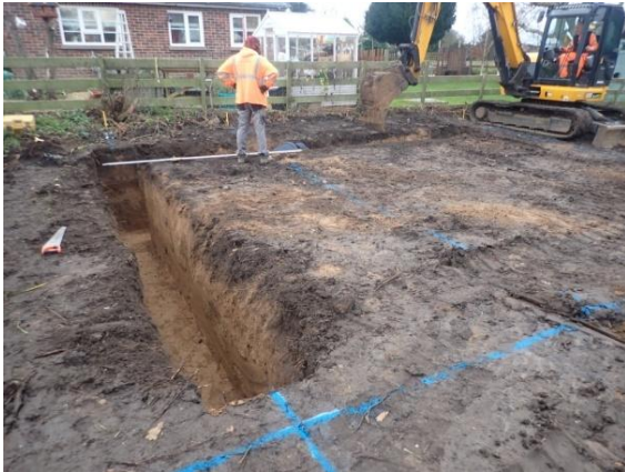
Plate 12: Excavation of the foundations, from the north
