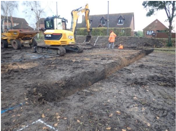
Plate 58: Excavation of the foundations, from the south-west
