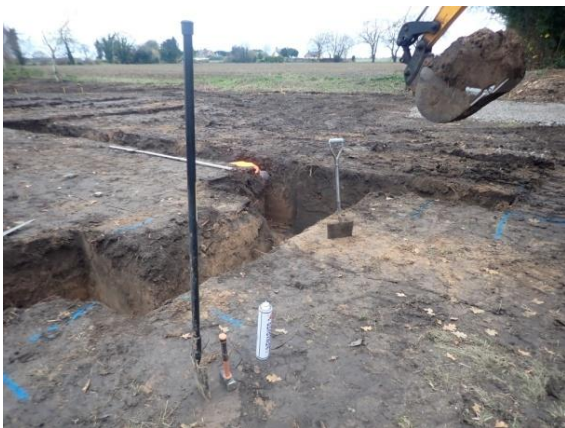
Plate 88: Excavation of the foundations, from the north-east
