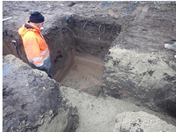
Plate 153: Excavation of the foundations, from the east
