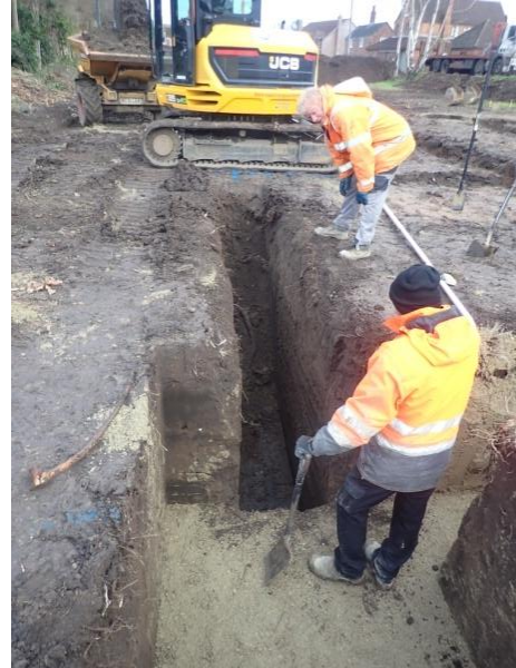
Plate 119: Excavation of the foundations, from the south
