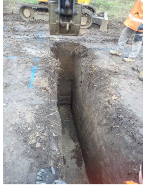
Plate 105: Excavation of the foundations, from the east
