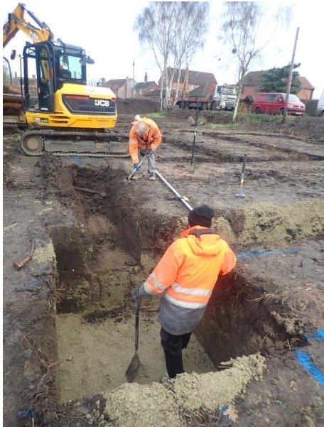
Plate 118: Excavation of the foundations, from the south
