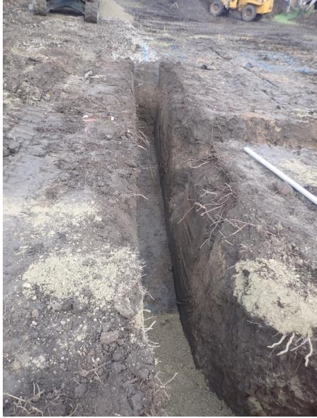
Plate 138: Excavation of the foundations, from the south
