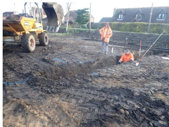
Plate 64: Excavation of the foundations, from the south-west
