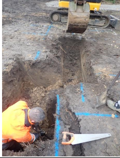
Plate 78: Excavation of the foundations, from the east
