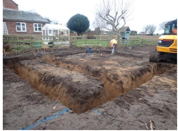
Plate 24: Excavation of the foundations, from the north-east
