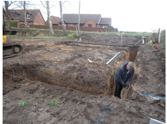
Plate 25: Excavation of the foundations, from the west
