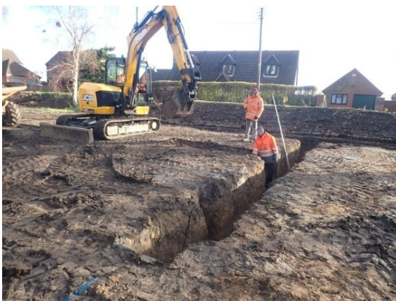
Plate 73: Excavation of the foundations, from the west
