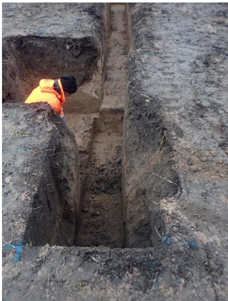
Plate 94: Excavation of the foundations, from the north
