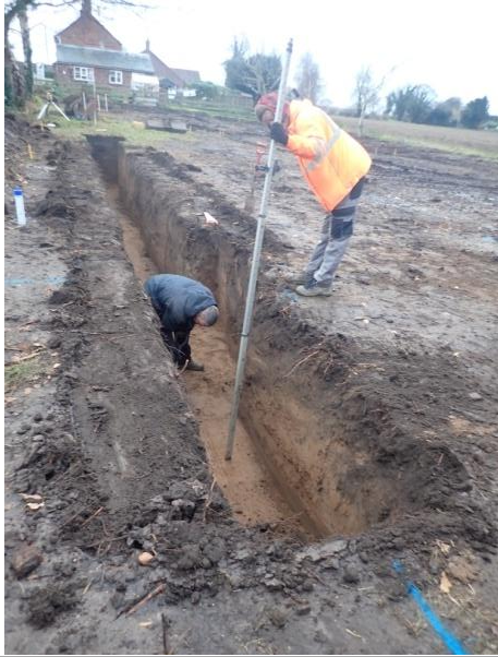
Plate 47: Excavation of the foundations, from the north
