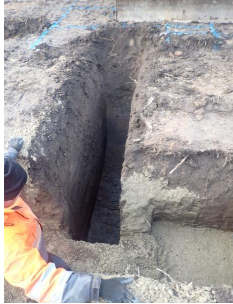
Plate 141: Excavation of the foundations, from the east
