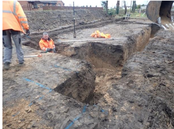
Plate 90: Excavation of the foundations, from the north
