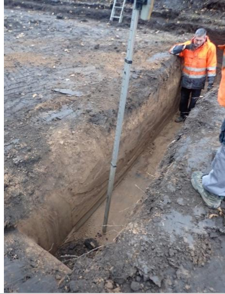
Plate 50: Excavation of the foundations, from the west
