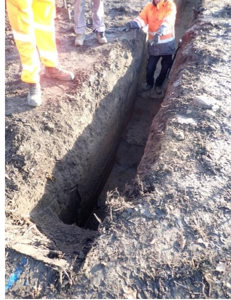
Plate 68: Excavation of the foundations, from the west
