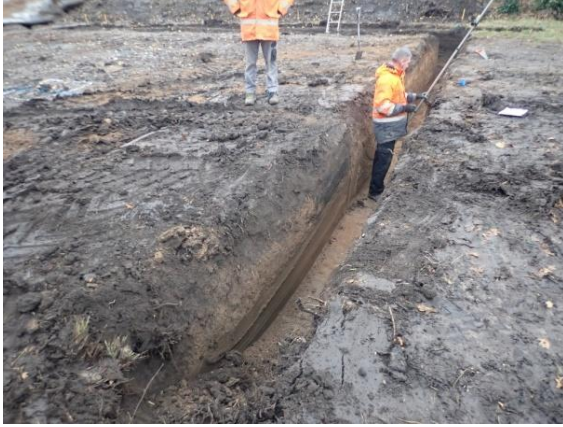
Plate 53: Excavation of the foundations, from the west
