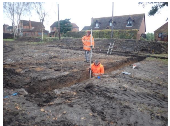
Plate 52: Excavation of the foundations, from the south-west
