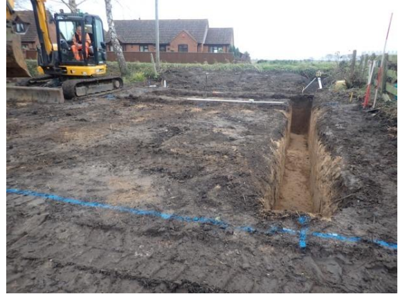
Plate 18: Excavation of the foundations, from the west
