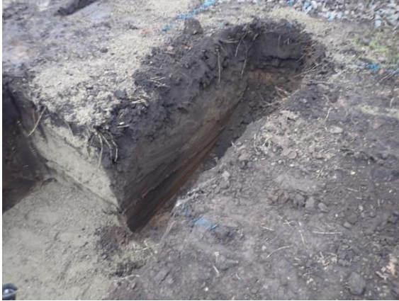
Plate 155: Excavation of the foundations, from the north-east
