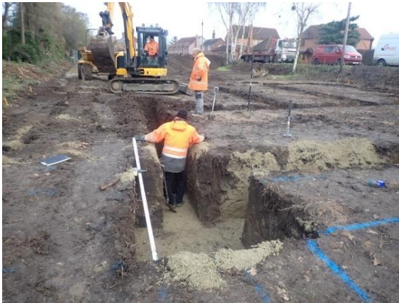
Plate 122: Excavation of the foundations, from the south
