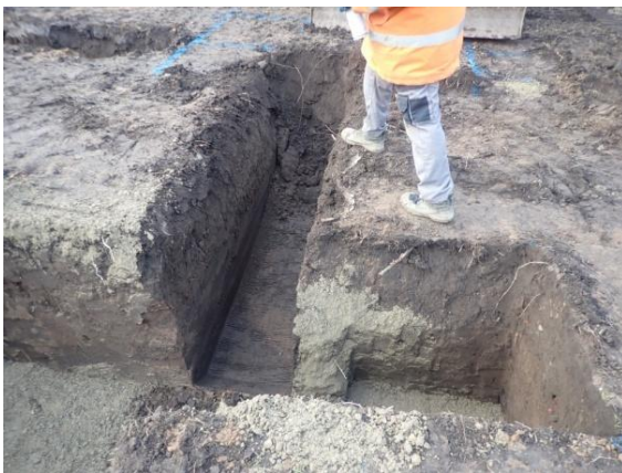
Plate 140: Excavation of the foundations, from the east
