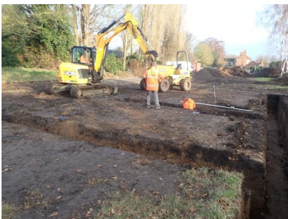
Plate 61: Excavation of the foundations, from the south
