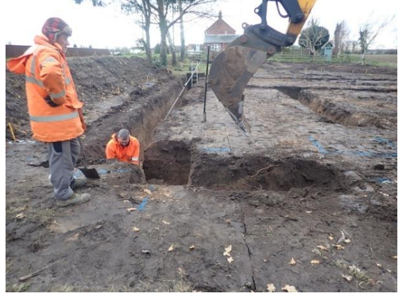
Plate 79: Excavation of the foundations, from the north
