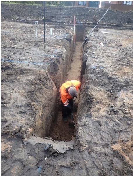
Plate 66: Excavation of the foundations, from the west
