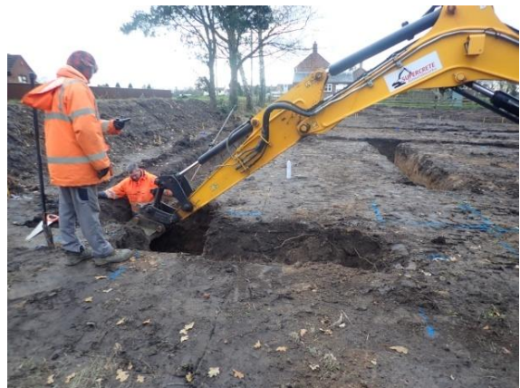
Plate 80: Excavation of the foundations, from the north
