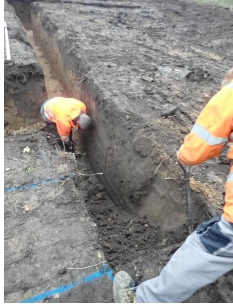
Plate 89: Excavation of the foundations, from the north
