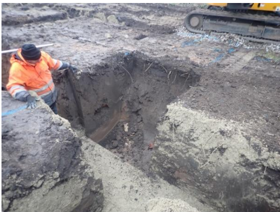
Plate 151: Excavation of the foundations, from the north-east
