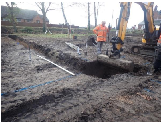
Plate 109: Excavation of the foundations, from the west
