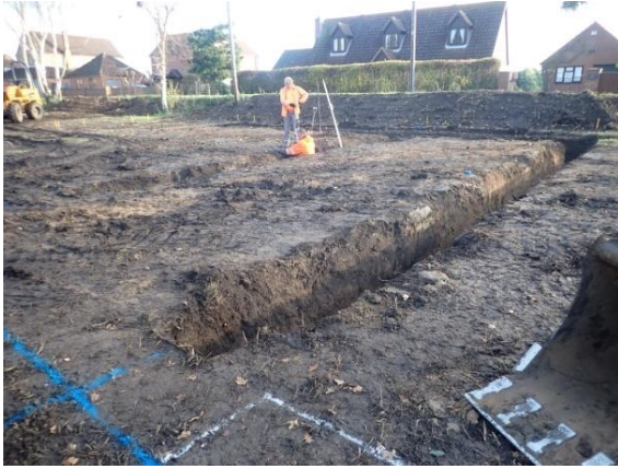
Plate 71: Representative Section 10, from the south-west
