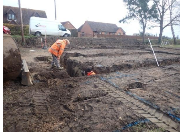
Plate 146: Excavation of the foundations, from the west
