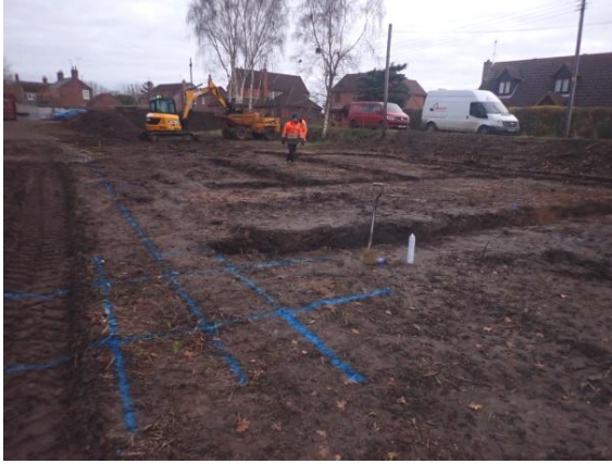
Plate 92: Excavation of the foundations, from the south
