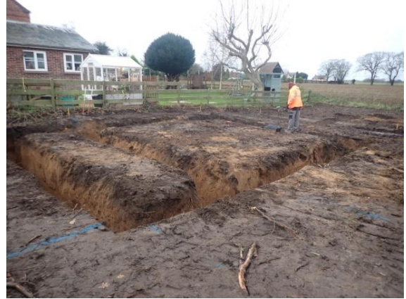
Plate 30: Excavation of the foundations, from the north-east
