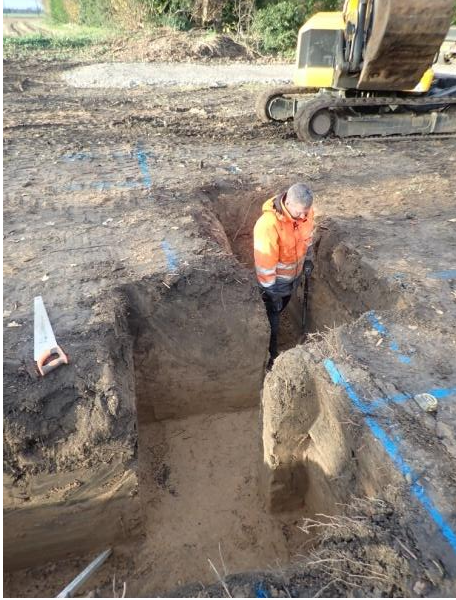
Plate 81: Excavation of the foundations, from the east
