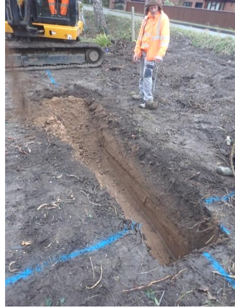
Plate 4: Excavation of the foundations, from the south
