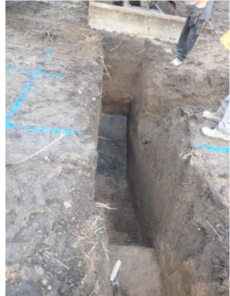
Plate 147: Excavation of the foundations, from the south
