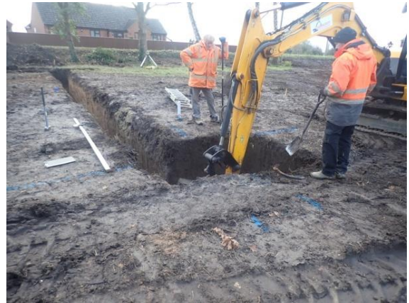
Plate 111: Excavation of the foundations, from the west
