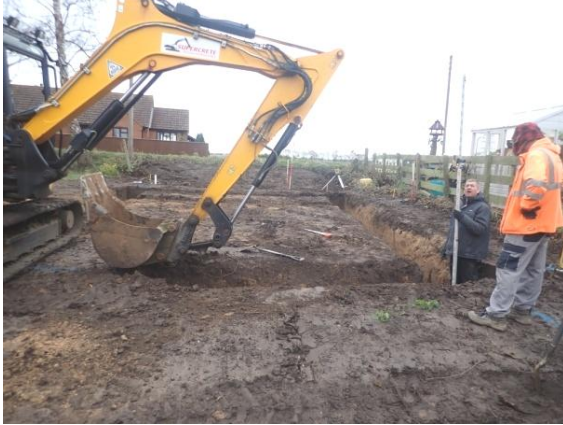
Plate 27: Excavation of the foundations, from the west
