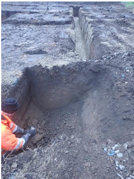
Plate 157: Excavation of the foundations, from the north
