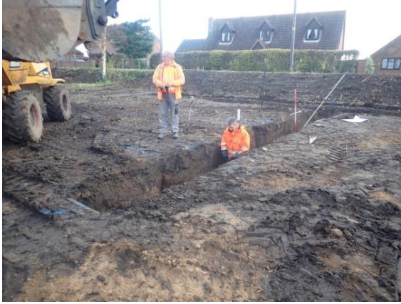
Plate 65: Excavation of the foundations, from the south-west
