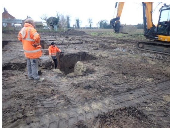
Plate 154: Excavation of the foundations, from the north
