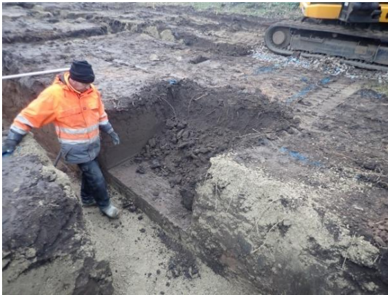
Plate 150: Excavation of the foundations, from the north-east
