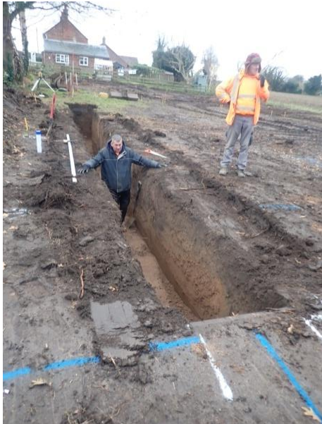
Plate 44: Excavation of the foundations, from the north
