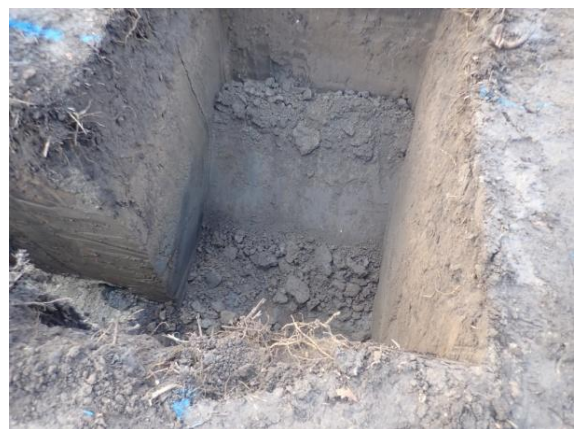
Plate 112: Excavation of the foundations, from the north
