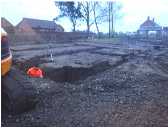
Plate 163: Excavation of the foundations, from the north-west
