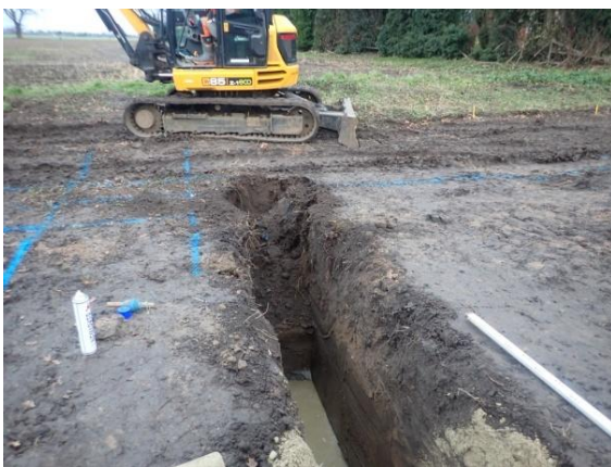
Plate 100: Excavation of the foundations, from the east
