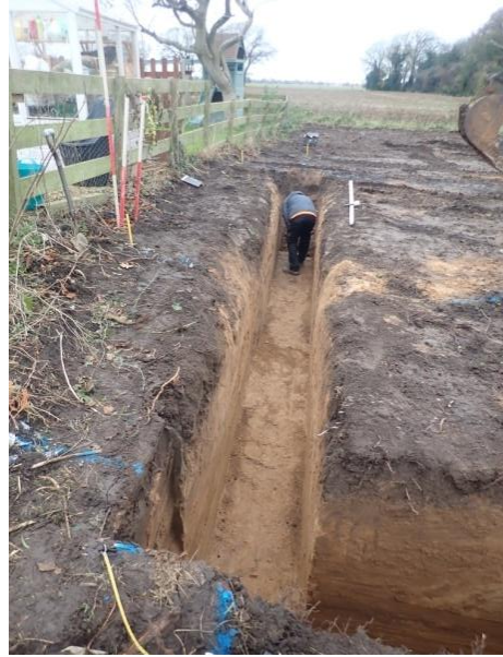
Plate 13: Excavation of the foundations, from the east
