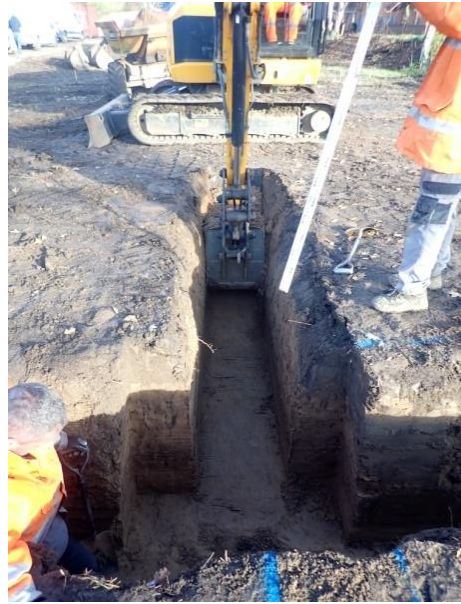
Plate 74: Excavation of the foundations, from the south
