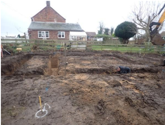
Plate 28: Excavation of the foundations, from the north
