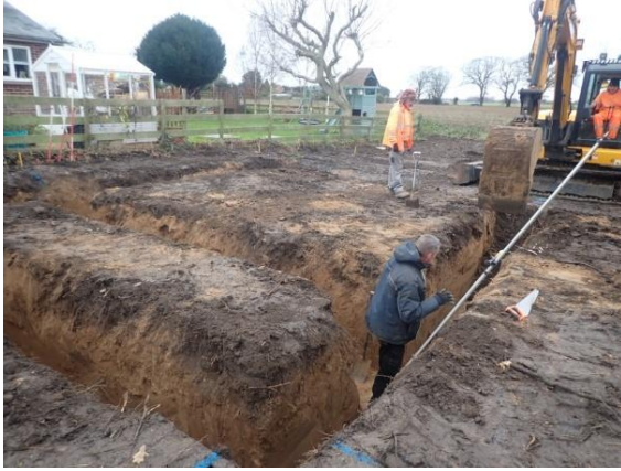
Plate 21: Excavation of the foundations, from the east
