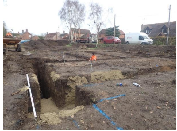
Plate 124: Excavation of the foundations, from the south
