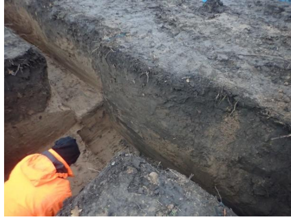
Plate 95: Excavation of the foundations, from the north-east
