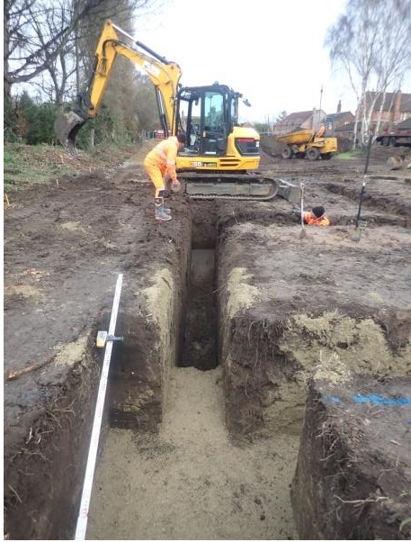
Plate 127: Excavation of the foundations, from the south
