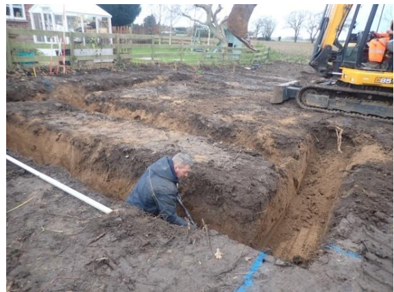
Plate 20: Excavation of the foundations, from the east
