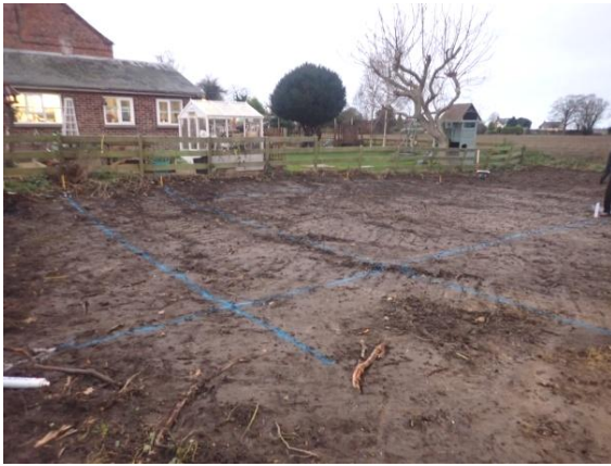
Plate 1: Pre-groundworks, from the north-east
