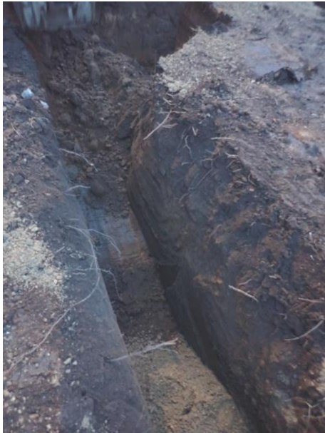
Plate 162: Excavation of the foundations, from the south
