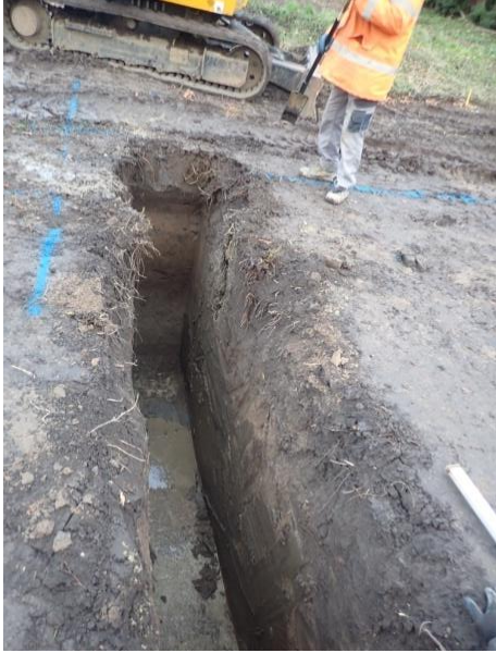
Plate 103: Excavation of the foundations, from the east
