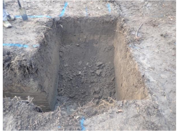
Plate 110: Excavation of the foundations, from the north
