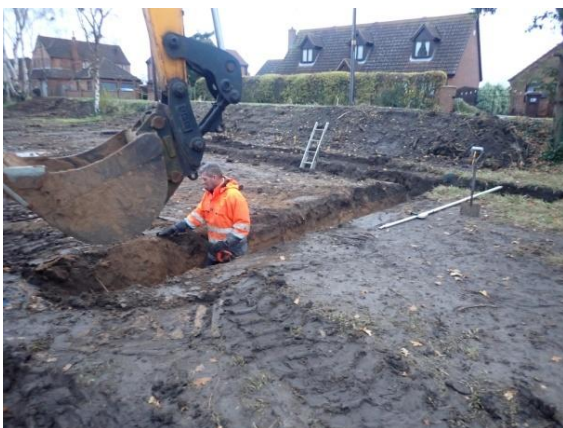
Plate 49: Excavation of the foundations, from the south-west
