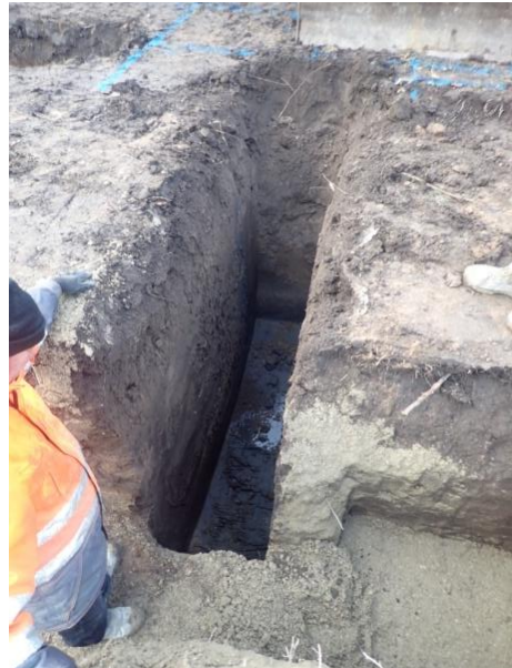
Plate 142: Excavation of the foundations, from the east
