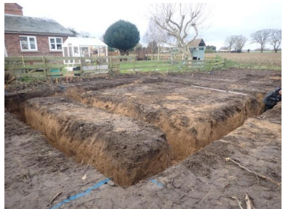
Plate 32: Excavation of the foundations, from the north-east
