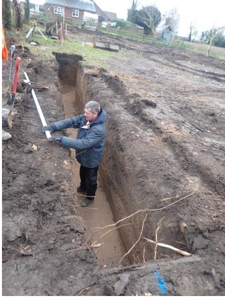
Plate 43: Excavation of the foundations, from the north
