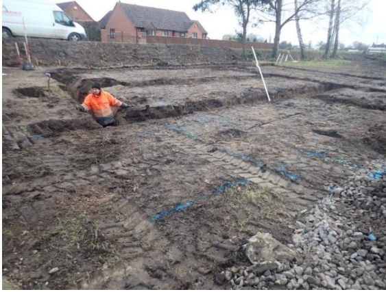
Plate 149: Excavation of the foundations, from the west
