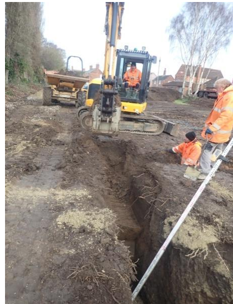
Plate 136: Excavation of the foundations, from the south
