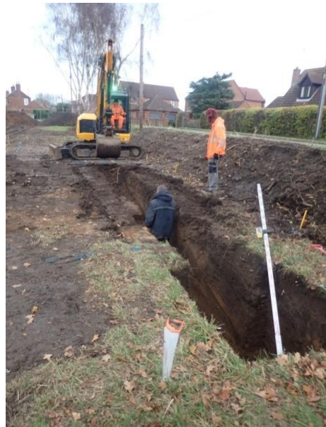
Plate 42: Excavation of the foundations, from the south
