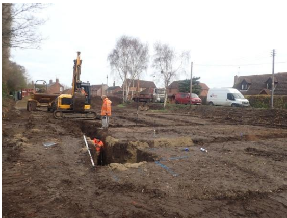
Plate 123: Excavation of the foundations, from the south
