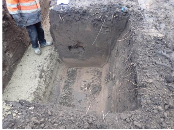
Plate 152: Excavation of the foundations, from the north
