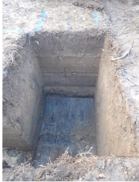
Plate 115: Excavation of the foundations, from the north
