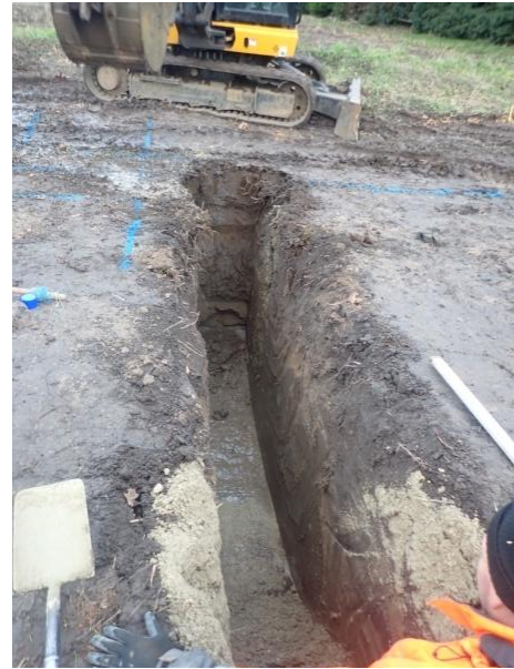
Plate 102: Excavation of the foundations, from the east
