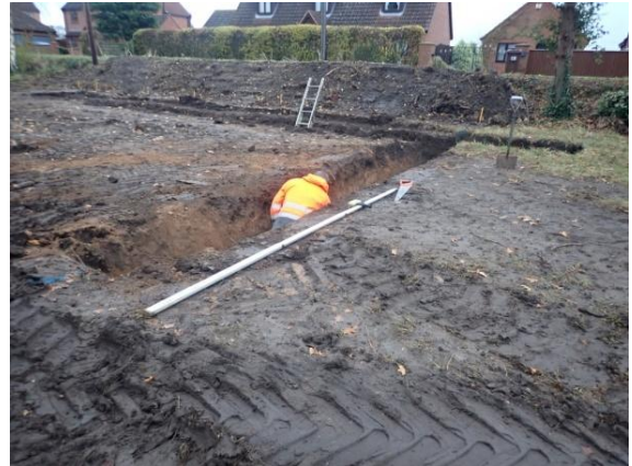
Plate 51: Excavation of the foundations, from the west
