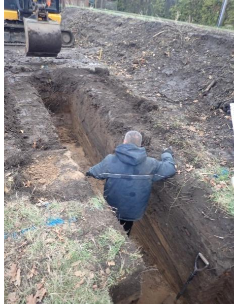
Plate 41: Excavation of the foundations, from the south
