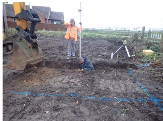
Plate 6: Excavation of the foundations, from the west
