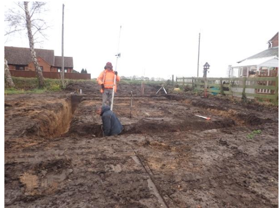
Plate 31: Excavation of the foundations, from the west
