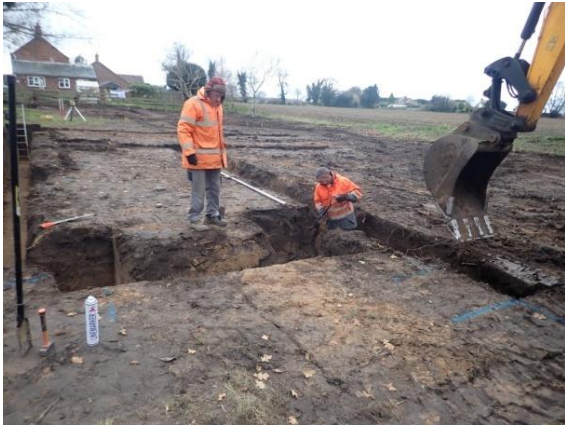
Plate 87: Excavation of the foundations, from the north
