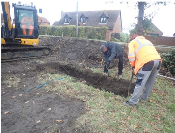
Plate 35: Excavation of the foundations, from the west
