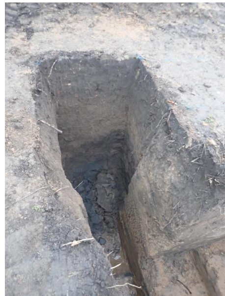
Plate 97: Excavation of the foundations, from the south
