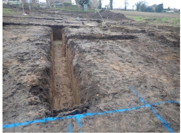
Plate 135: Excavation of the foundations, from the north
