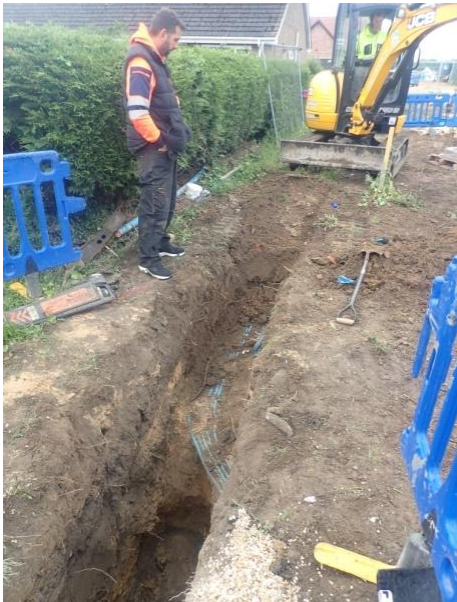
Plate 159: Excavation of the service trench, from the north
