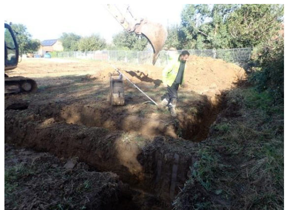
Plate 80: Excavation of the foundations, from the south
