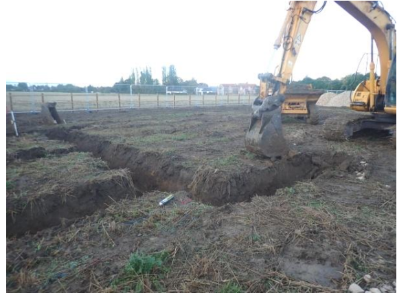
Plate 57: Excavation of the foundations, from the north-east
