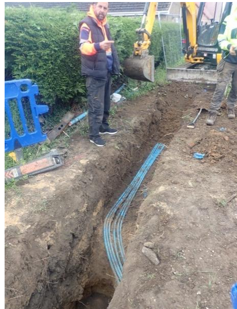
Plate 161: Excavation of the service trench, from the north
