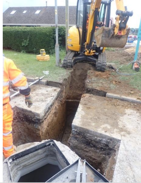
Plate 143: Excavation of the service trench, from the north
