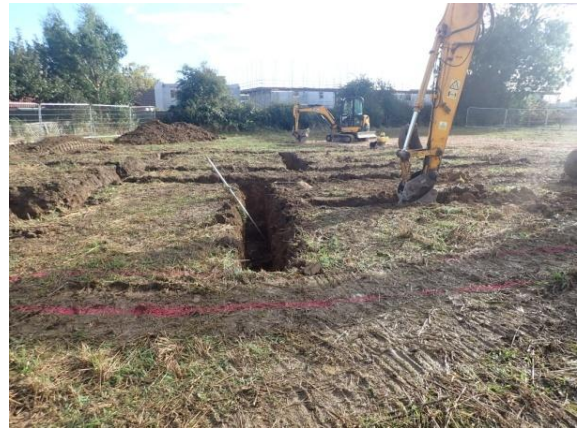
Plate 28: Excavation of the foundations, from the west
