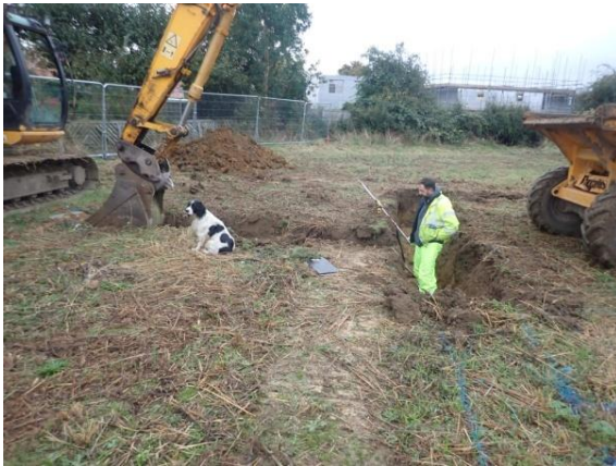
Plate 13: Excavation of the foundations, from the west
