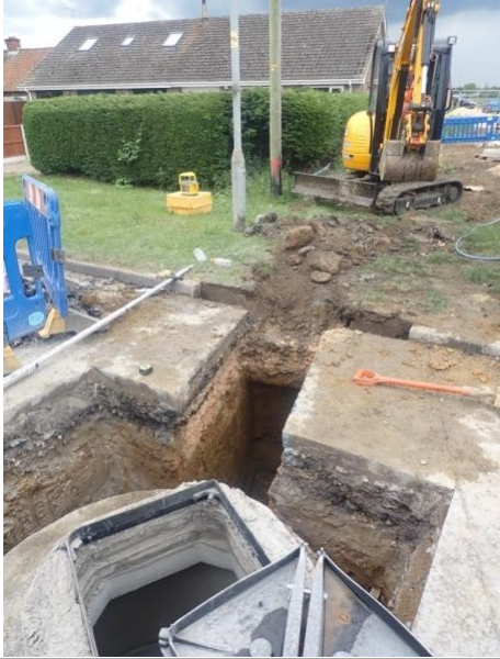
Plate 141: Excavation of the service trench, from the north
