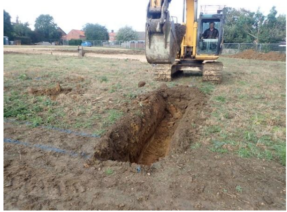
Plate 39: Excavation of the foundations, from the south
