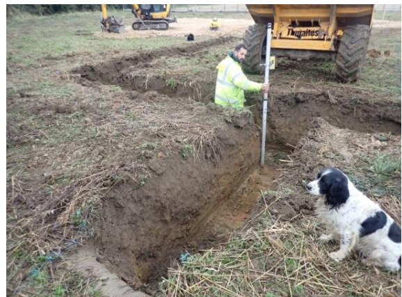
Plate 11: Excavation of the foundations, from the north
