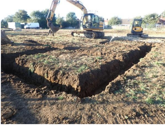
Plate 54: Excavation of the foundations, from the south-east
