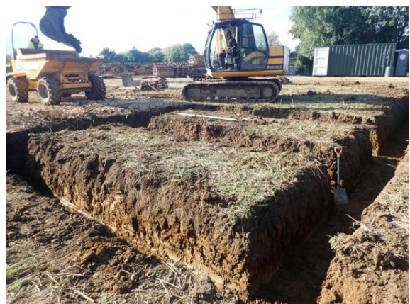
Plate 110: Excavation of the foundations, from the north-east
