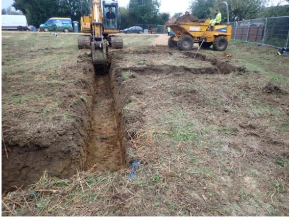
Plate 18: Excavation of the foundations, from the east
