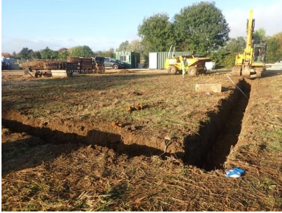
Plate 93: Excavation of the foundations, from the east
