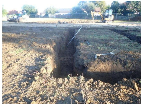
Plate 64: Excavation of the foundations, from the south
