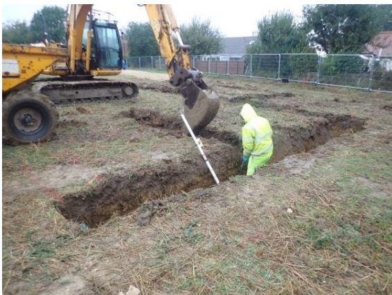
Plate 20: Excavation of the foundations, from the south-east
