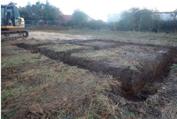
Plate 56: Excavation of the foundations, from the south-west
