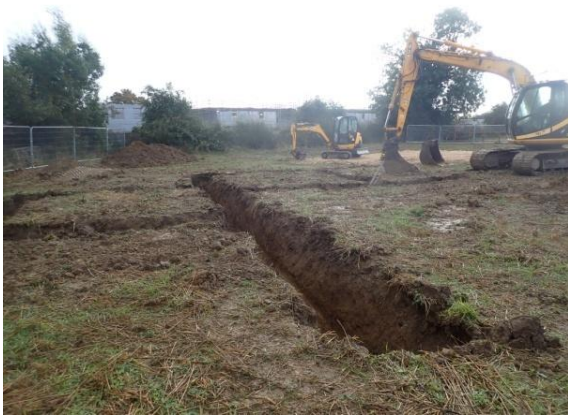
Plate 25: Excavation of the foundations, from the west
