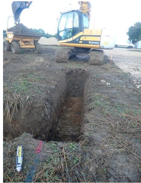
Plate 58: Excavation of the foundations, from the east
