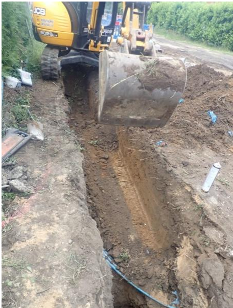
Plate 163: Excavation of the service trench, from the north
