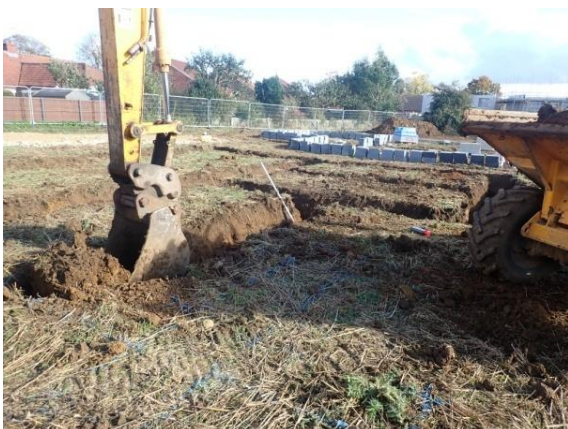
Plate 113: Excavation of the foundations, from the west
