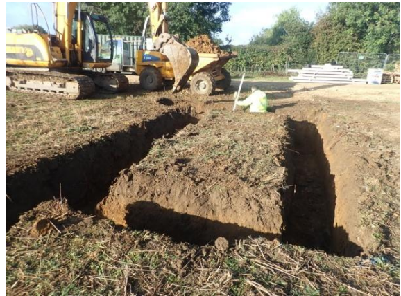
Plate 97: Excavation of the foundations, from the east
