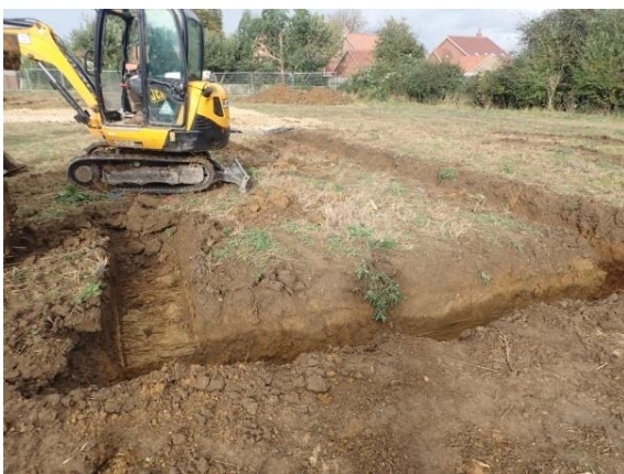
Plate 44: Excavation of the foundations, from the south
