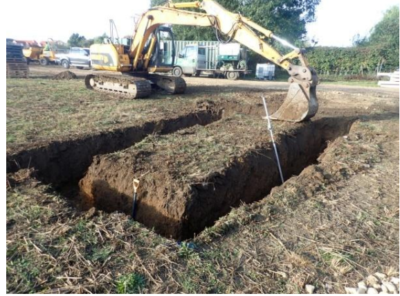
Plate 96: Excavation of the foundations, from the north-east
