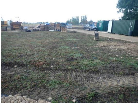
Plate 87: Excavation of the foundations, from the north
