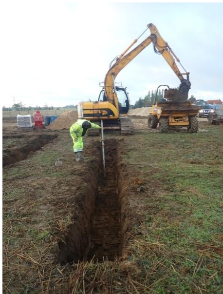
Plate 89: Excavation of the foundations, from the north
