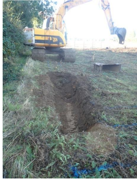
Plate 68: Excavation of the foundations, from the north
