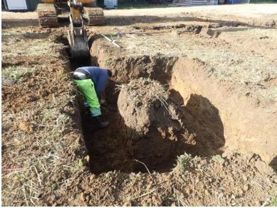
Plate 117: Excavation of the foundations, from the north
