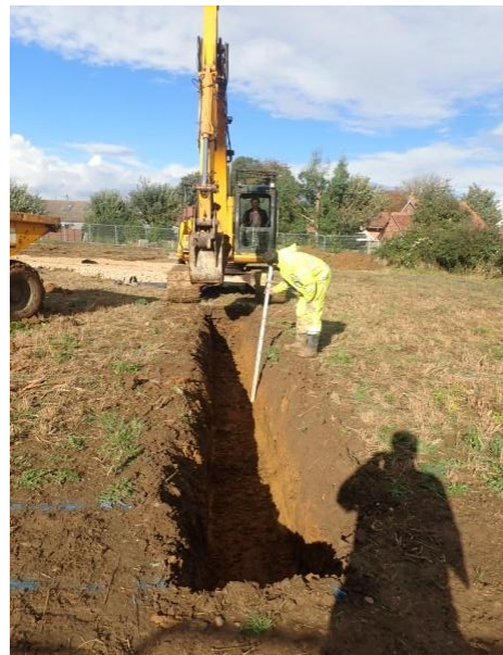
Plate 41: Excavation of the foundations, from the south
