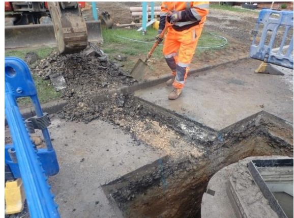
Plate 131: Excavation of the service trench, from the north-east
