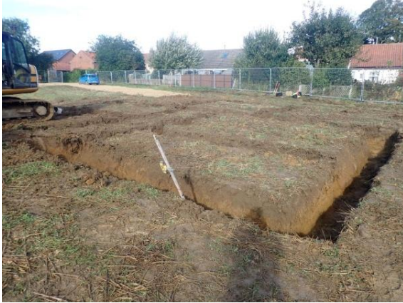
Plate 30: Excavation of the foundations, from the south-east
