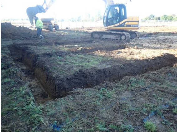
Plate 75: Excavation of the foundations, from the north
