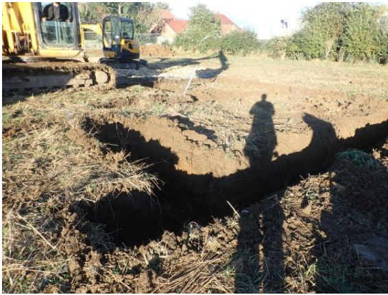
Plate 55: Excavation of the foundations, from the south-east
