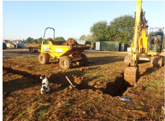
Plate 91: Excavation of the foundations, from the east
