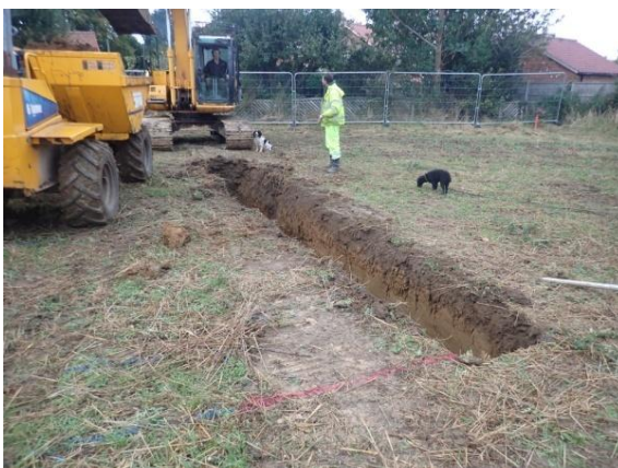
Plate 8: Excavation of the foundations, from the south
