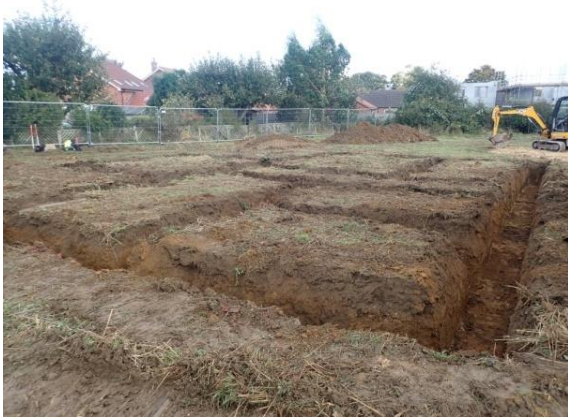
Plate 37: Excavation of the foundations, from the west
