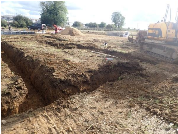
Plate 118: Excavation of the foundations, from the west
