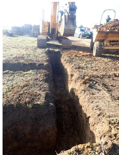
Plate 98: Excavation of the foundations, from the north
