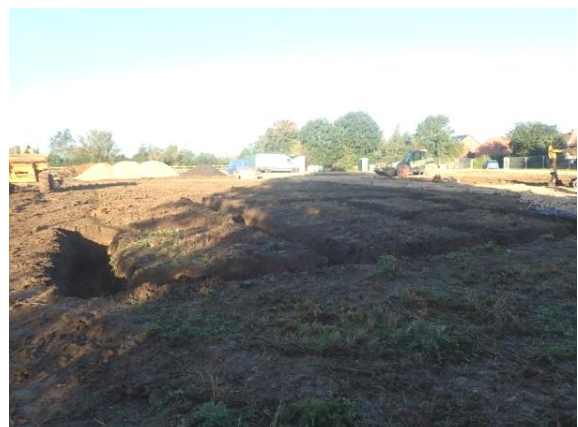
Plate 65: Excavation of the foundations, from the east
