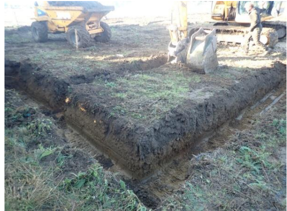
Plate 73: Excavation of the foundations, from the north-east
