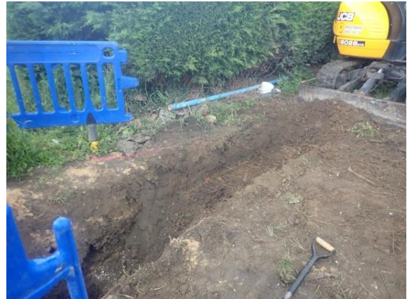
Plate 156: Excavation of the service trench, from the north-west
