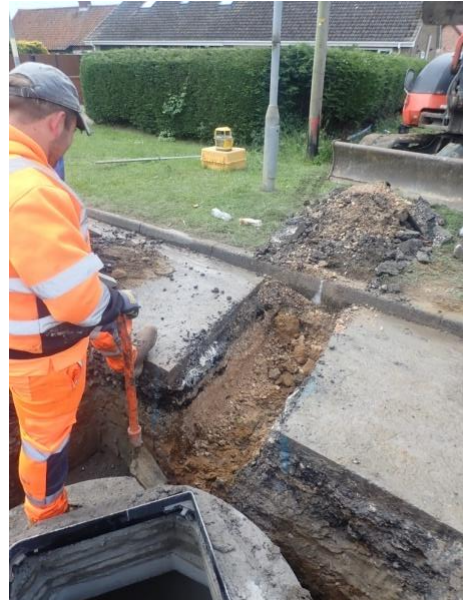
Plate 135: Excavation of the service trench, from the north
