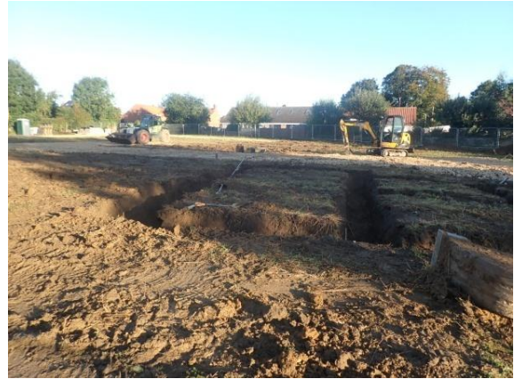
Plate 63: Excavation of the foundations, from the south
