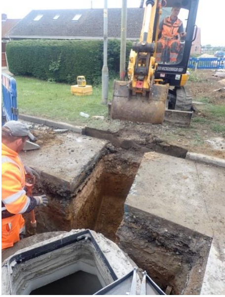
Plate 137: Excavation of the service trench, from the north
