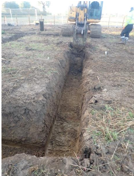
Plate 61: Excavation of the foundations, from the north
