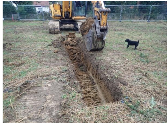
Plate 5: Excavation of the foundations, from the south
