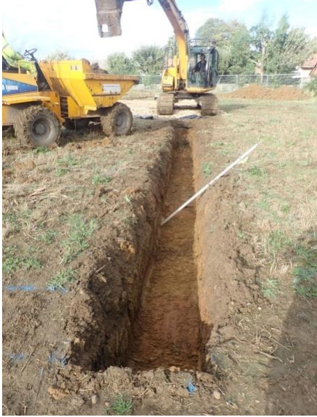
Plate 42: Excavation of the foundations, from the south
