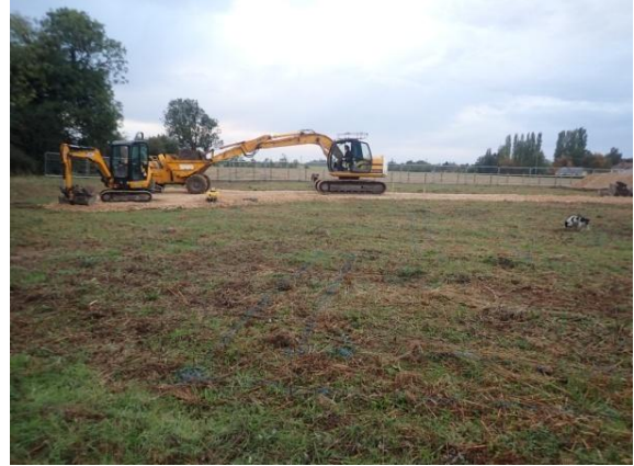
Plate 4: Pre-groundworks, from the north-west
