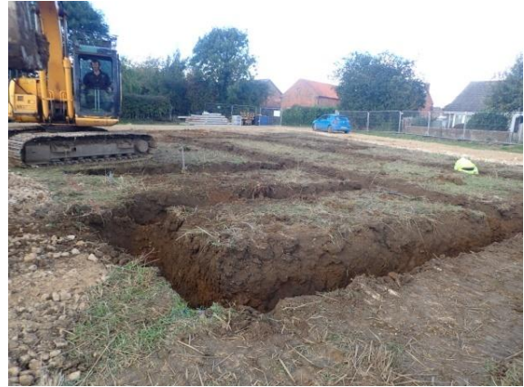
Plate 108: Excavation of the foundations, from the east
