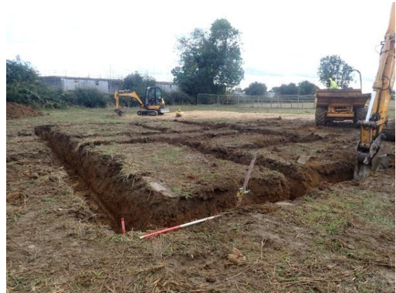
Plate 34: Excavation of the foundations, from the west
