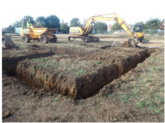
Plate 52: Excavation of the foundations, from the south-east
