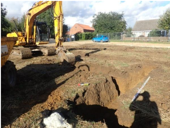
Plate 112: Excavation of the foundations, from the south
