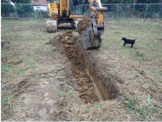
Plate 1: Pre-groundworks, from the north-west
