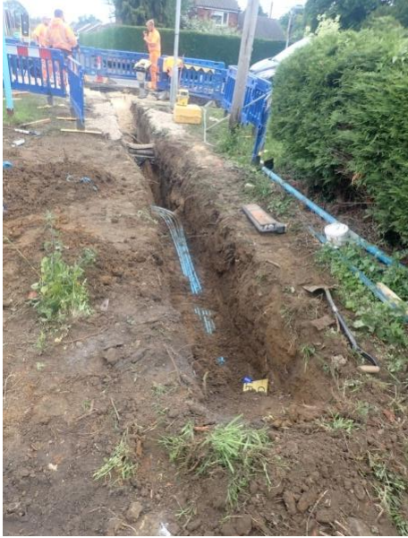
Plate 162: Excavation of the service trench, from the south
