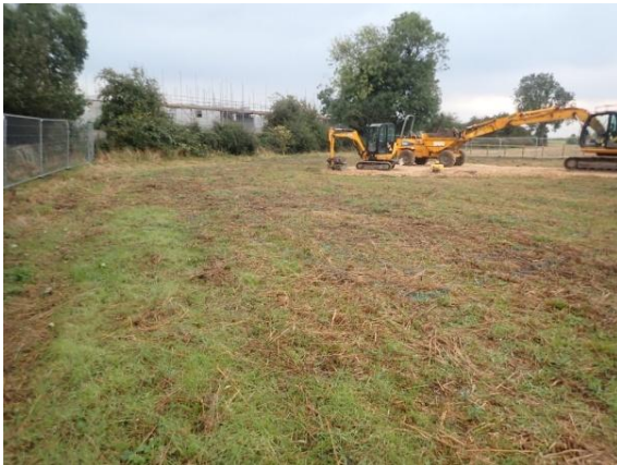
Plate 2: Pre-groundworks, from the west
