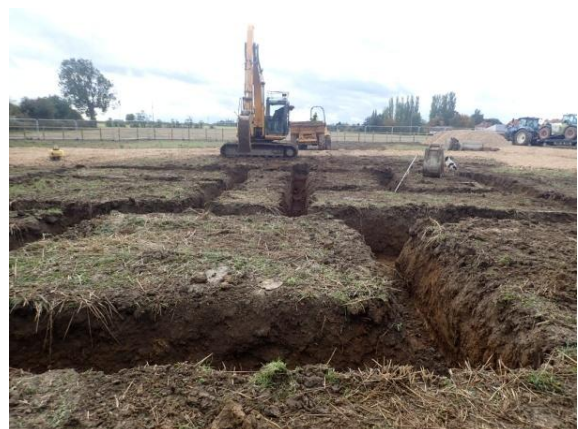
Plate 35: Excavation of the foundations, from the north
