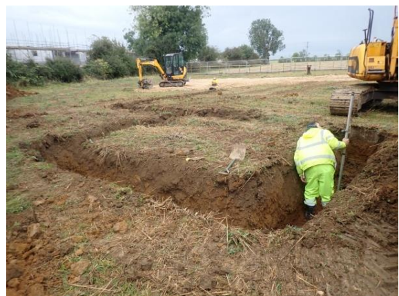
Plate 17: Excavation of the foundations, from the north
