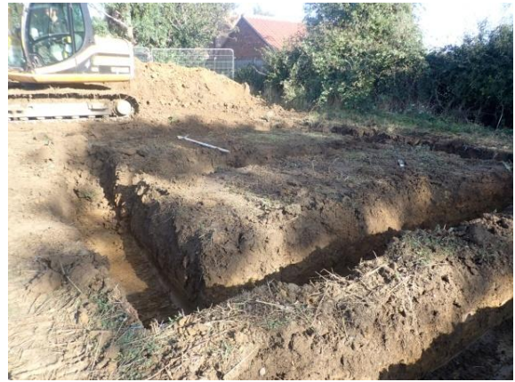
Plate 85: Excavation of the foundations, from the south
