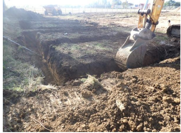
Plate 84: Excavation of the foundations, from the north
