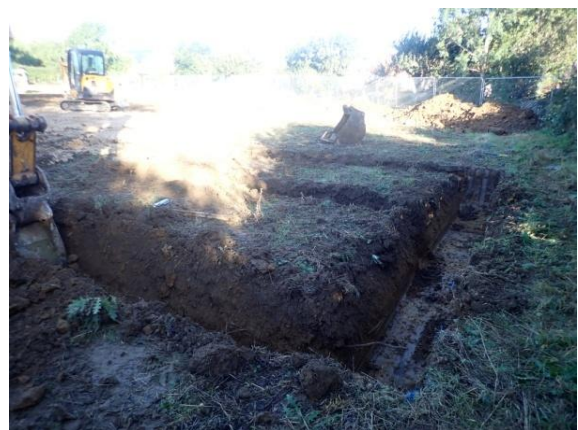
Plate 74: Excavation of the foundations, from the west
