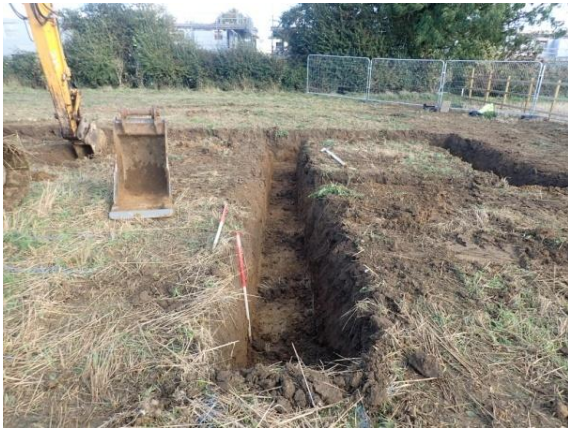
Plate 49: Excavation of the foundations, from the south
