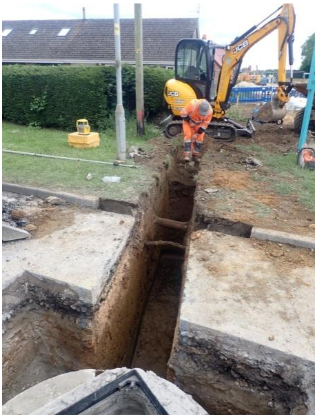
Plate 146: Excavation of the service trench, from the north
