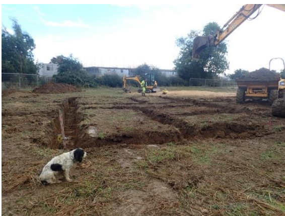
Plate 32: Excavation of the foundations, from the west
