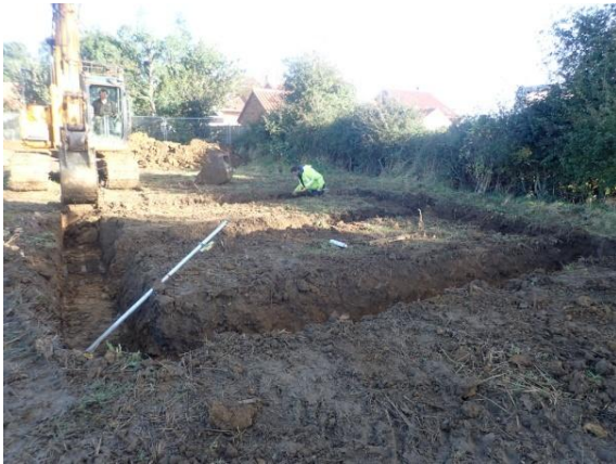
Plate 76: Excavation of the foundations, from the south
