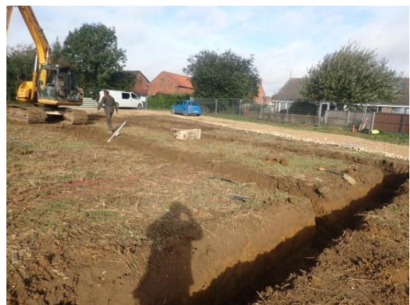
Plate 104: Excavation of the foundations, from the south-east
