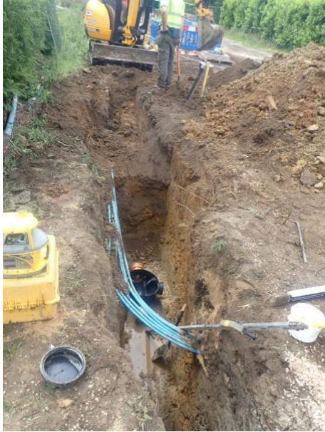
Plate 166: Excavation of the service trench, from the north
