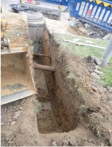
Plate 145: Excavation of the service trench, from the south
