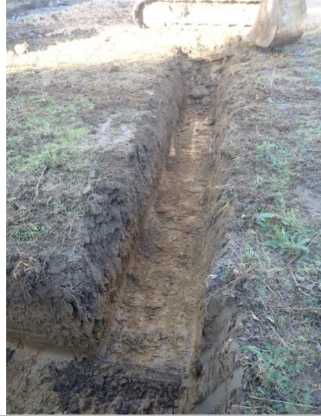
Plate 72: Excavation of the foundations, from the east
