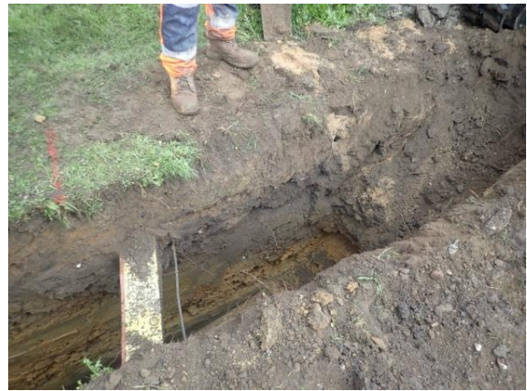
Plate 152: Excavation of the service trench, from the west
