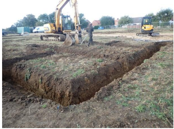
Plate 51: Excavation of the foundations, from the south-east
