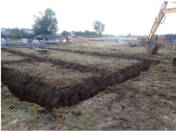
Plate 105: Excavation of the foundations, from the north-west
