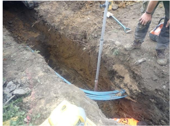
Plate 165: Excavation of the service trench, from the north-east
