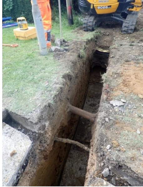
Plate 147: Excavation of the service trench, from the north
