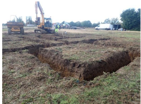
Plate 29: Excavation of the foundations, from the north-east
