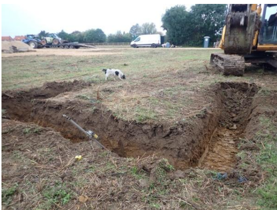
Plate 14: Excavation of the foundations, from the east
