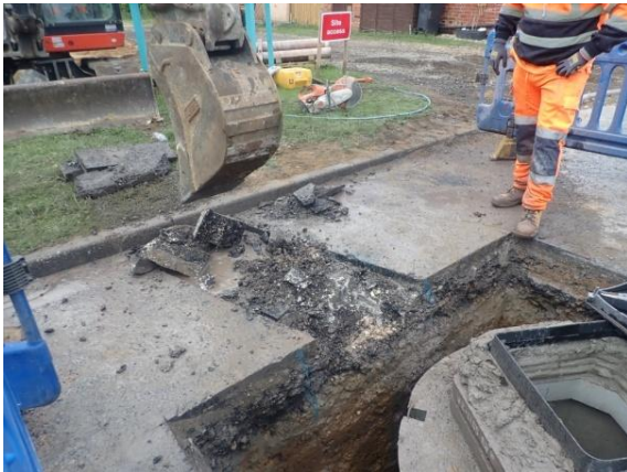
Plate 128: Excavation of the service trench, from the north-east
