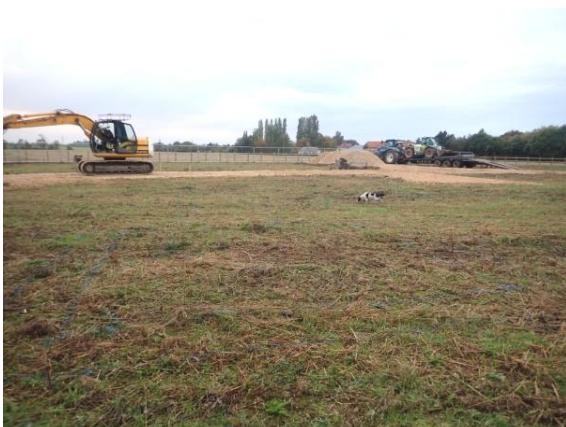
Plate 3: Pre-groundworks, from the north-east
