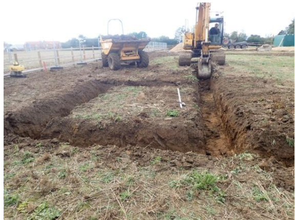
Plate 46: Excavation of the foundations, from the east
