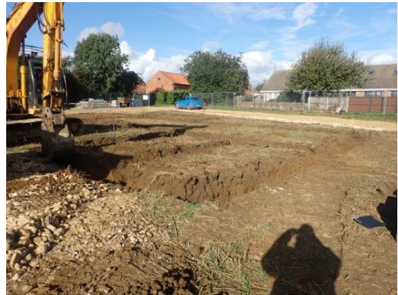
Plate 109: Excavation of the foundations, from the south-east
