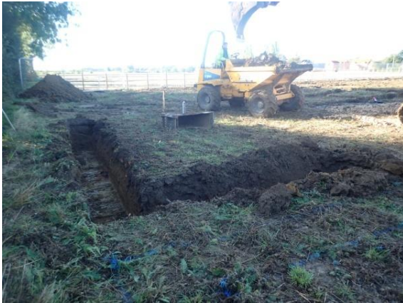
Plate 71: Excavation of the foundations, from the north
