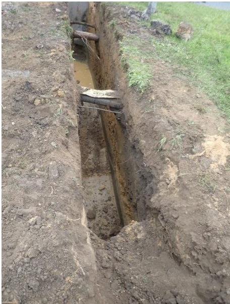
Plate 154: Excavation of the service trench, from the south
