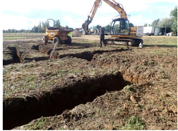
Plate 27: Excavation of the foundations, from the north-east
