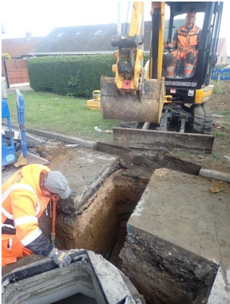
Plate 138: Excavation of the service trench, from the north
