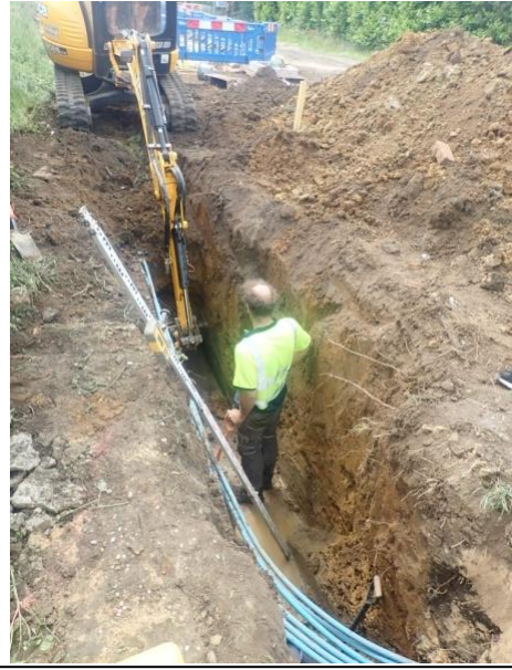
Plate 168: Excavation of the service trench, from the north
