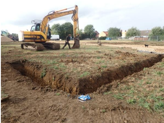
Plate 43: Excavation of the foundations, from the south
