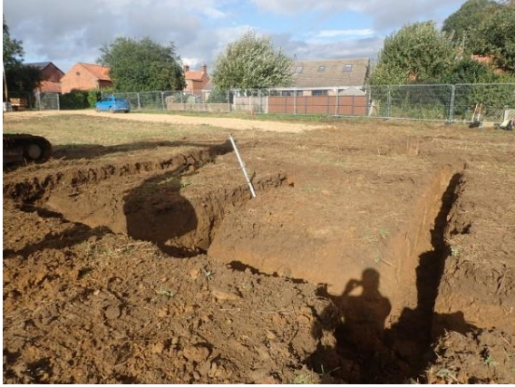
Plate 36: Excavation of the foundations, from the south-east
