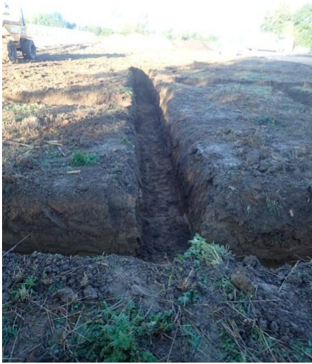
Plate 66: Excavation of the foundations, from the east
