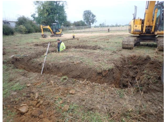
Plate 16: Excavation of the foundations, from the north
