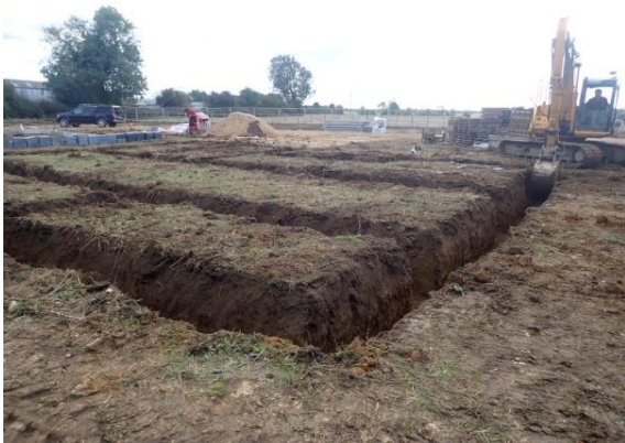
Plate 119: Excavation of the foundations, from the north-east
