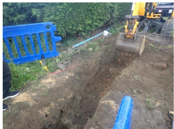
Plate 157: Excavation of the service trench, from the north-west
