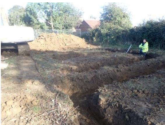
Plate 83: Excavation of the foundations, from the south
