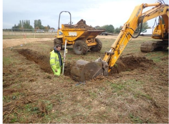
Plate 9: Excavation of the foundations, from the north-west
