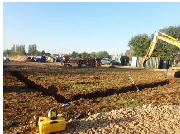
Plate 92: Excavation of the foundations, from the north
