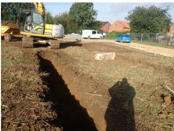
Plate 101: Excavation of the foundations, from the east
