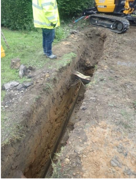
Plate 153: Excavation of the service trench, from the north
