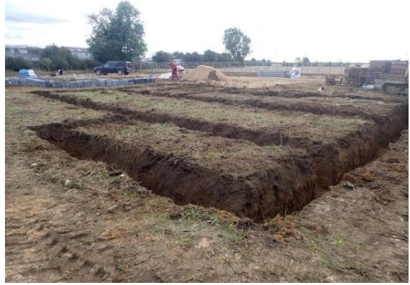
Plate 120: Excavation of the foundations, from the north-east
