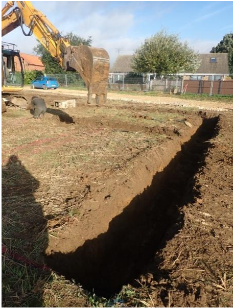
Plate 100: Excavation of the foundations, from the south
