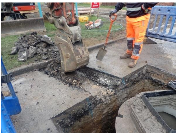
Plate 129: Excavation of the service trench, from the north-east
