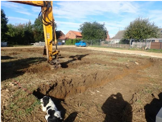
Plate 106: Excavation of the foundations, from the south-east
