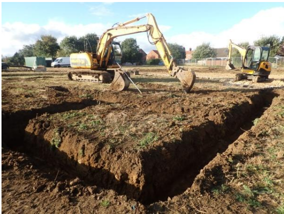
Plate 50: Excavation of the foundations, from the south-east
