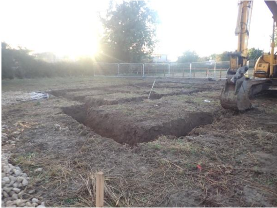
Plate 60: Excavation of the foundations, from the north-west
