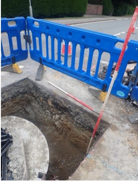
Plate 122: Section 14 through Tillbridge Lane, from the south-west
