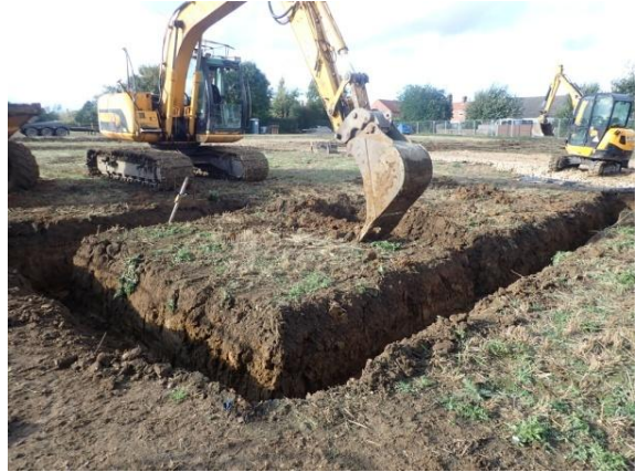
Plate 45: Excavation of the foundations, from the south-east
