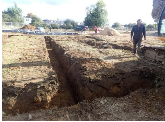
Plate 114: Excavation of the foundations, from the north
