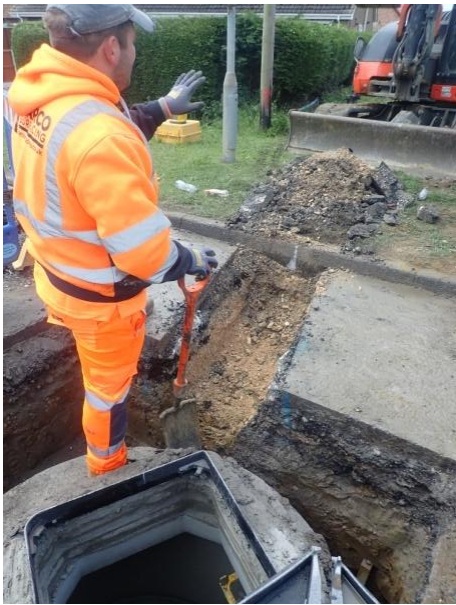
Plate 134: Excavation of the service trench, from the north
