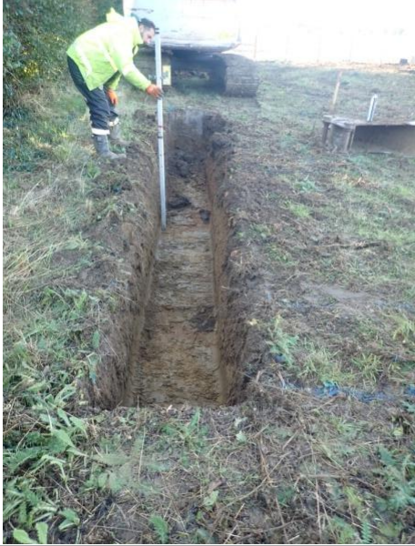
Plate 70: Excavation of the foundations, from the north
