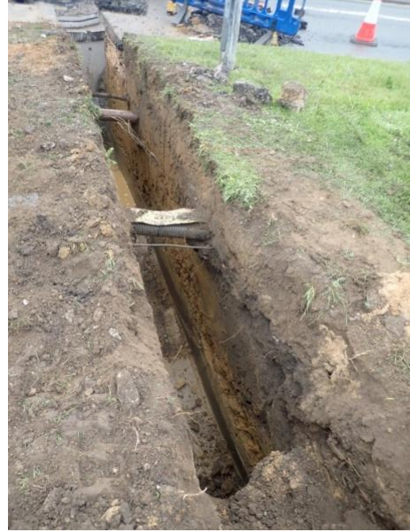
Plate 155: Excavation of the service trench, from the south
