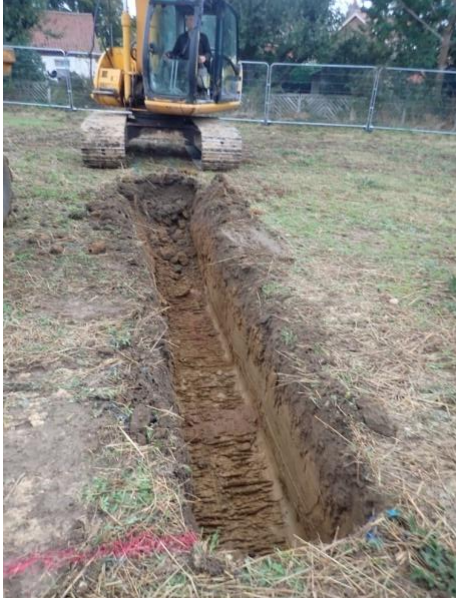
Plate 6: Excavation of the foundations, from the south
