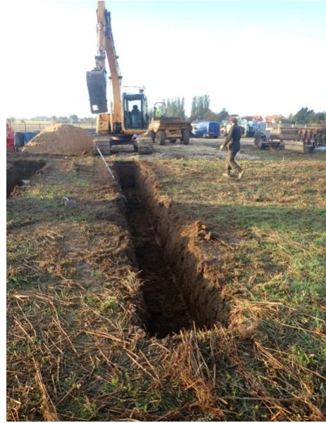
Plate 90: Excavation of the foundations, from the north
