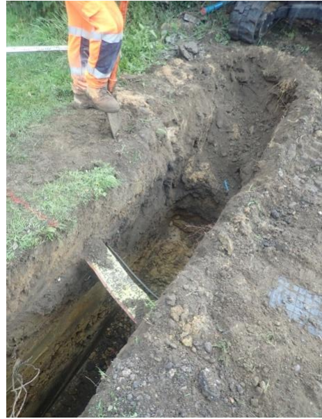
Plate 151: Excavation of the service trench, from the north
