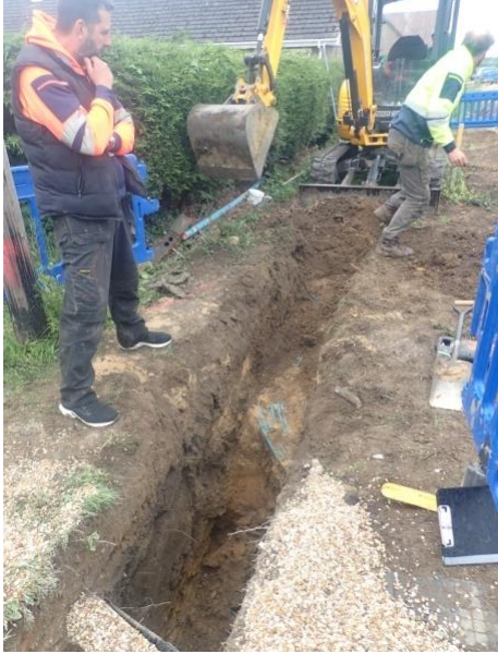
Plate 158: Excavation of the service trench, from the north
