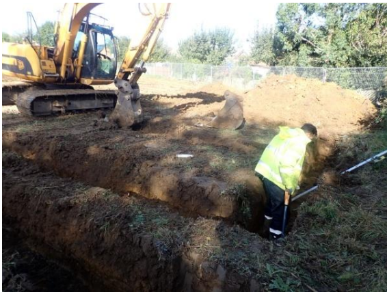
Plate 82: Excavation of the foundations, from the south
