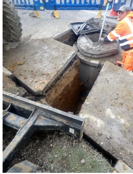
Plate 139: Excavation of the service trench, from the north
