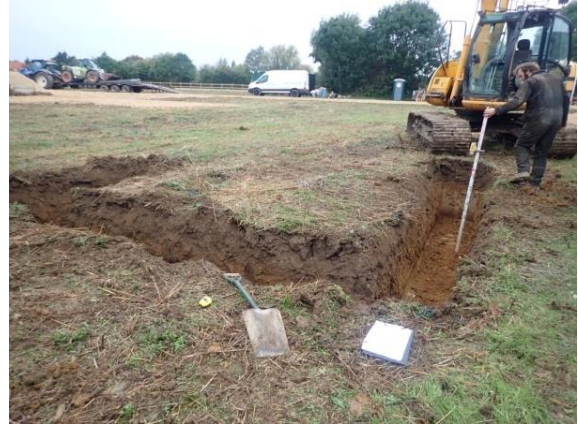
Plate 15: Excavation of the foundations, from the east
