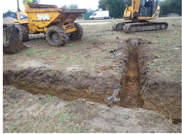
Plate 21: Excavation of the foundations, from the east
