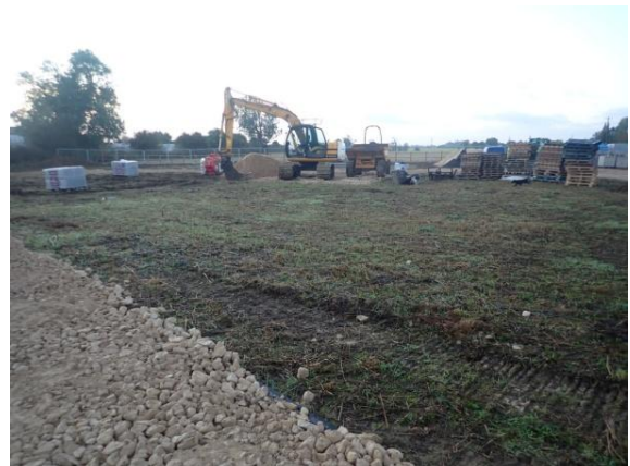
Plate 86: Excavation of the foundations, from the north-west
