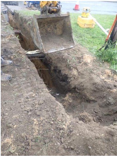
Plate 150: Excavation of the service trench, from the south
