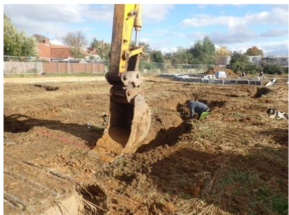
Plate 116: Excavation of the foundations, from the west
