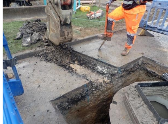
Plate 130: Excavation of the service trench, from the north-east
