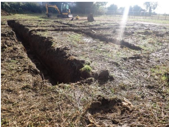
Plate 26: Excavation of the foundations, from the west
