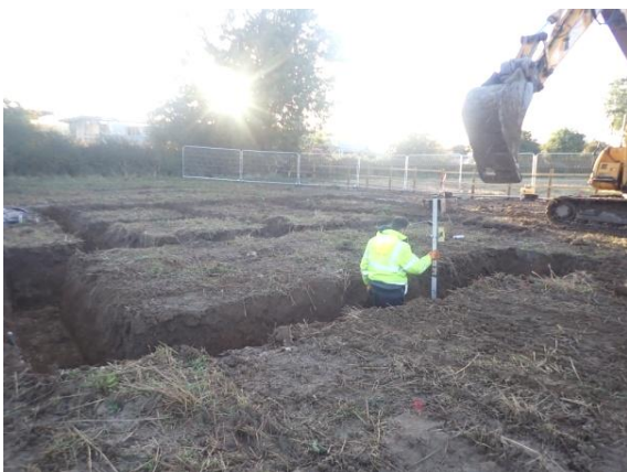
Plate 62: Excavation of the foundations, from the south-west
