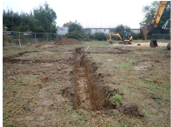
Plate 22: Excavation of the foundations, from the west
