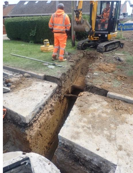
Plate 144: Excavation of the service trench, from the north
