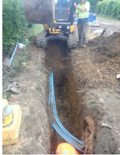
Plate 164: Excavation of the service trench, from the north
