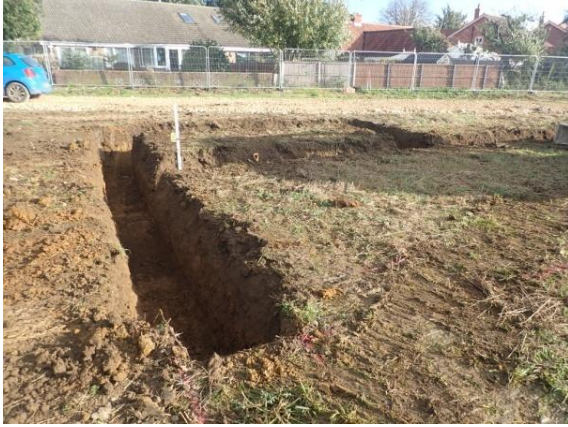
Plate 99: Excavation of the foundations, from the south
