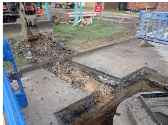
Plate 132: Excavation of the service trench, from the north-east
