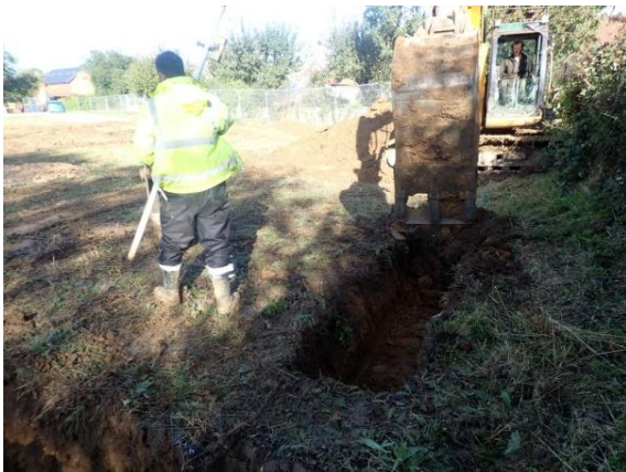
Plate 77: Excavation of the foundations, from the south
