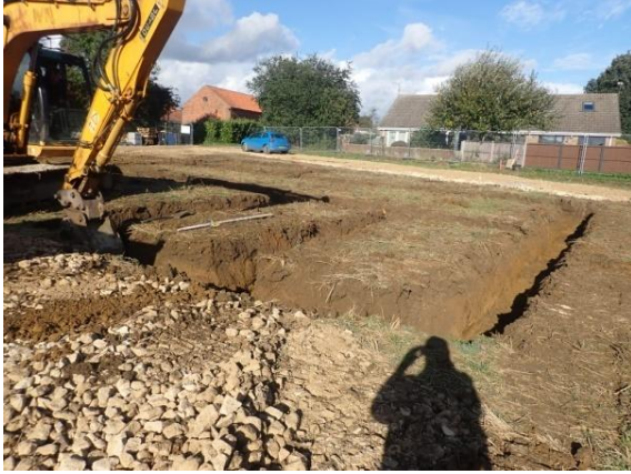
Plate 111: Excavation of the foundations, from the south
