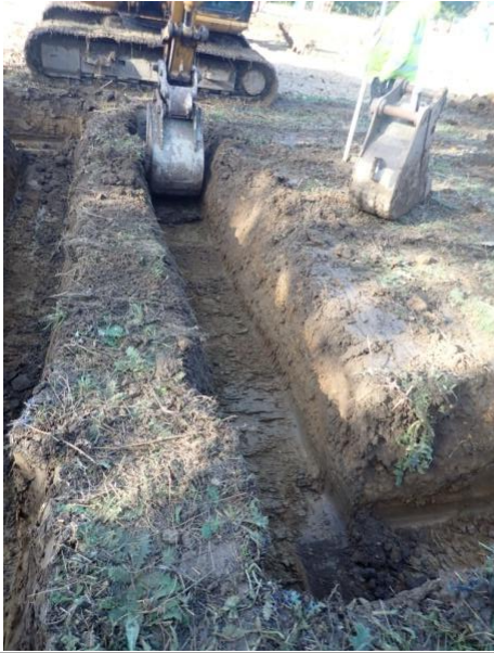
Plate 81: Excavation of the foundations, from the east
