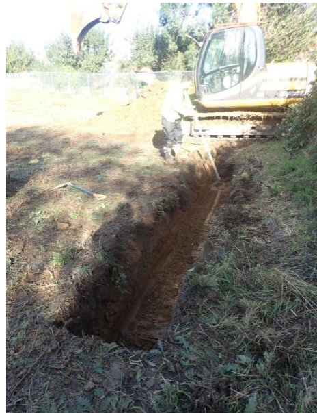
Plate 79: Excavation of the foundations, from the south
