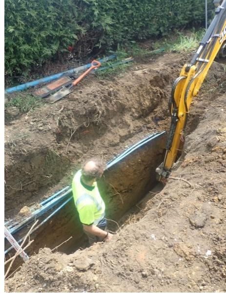
Plate 169: Excavation of the service trench, from the north-west
