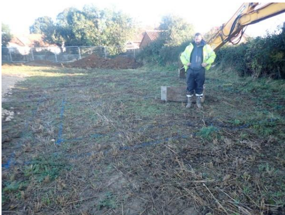
Plate 67: Pre-groundworks, from the south
