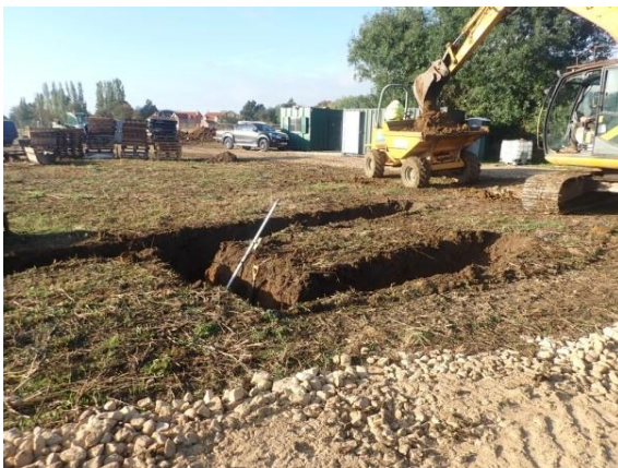
Plate 95: Excavation of the foundations, from the north
