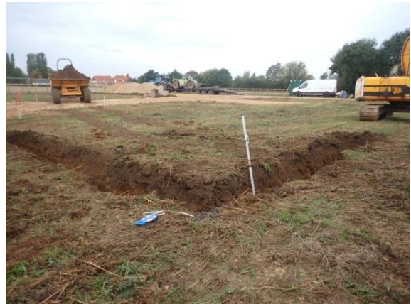
Plate 10: Excavation of the foundations, from the north-east
