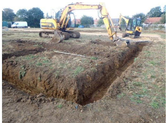
Plate 47: Excavation of the foundations, from the south
