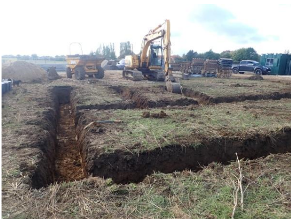
Plate 107: Excavation of the foundations, from the north
