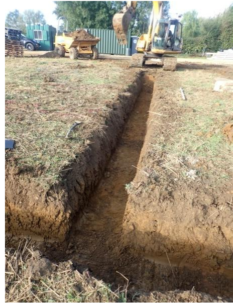
Plate 103: Excavation of the foundations, from the south
