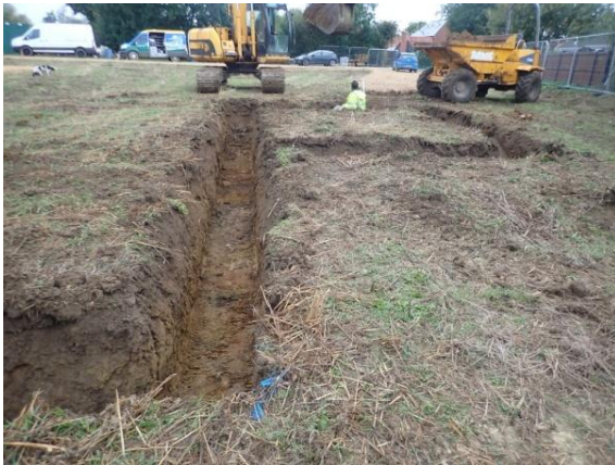
Plate 19: Excavation of the foundations, from the east
