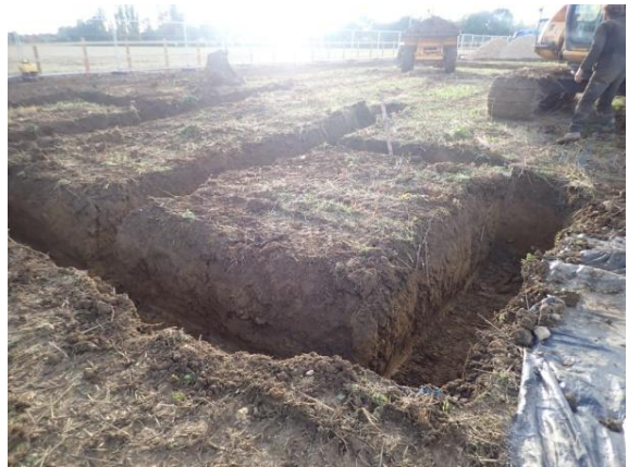
Plate 53: Excavation of the foundations, from the north-east
