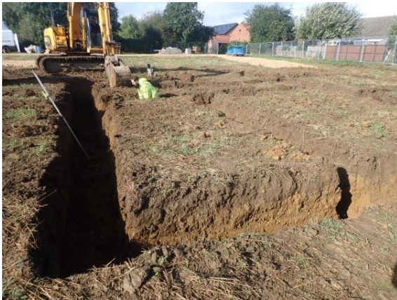
Plate 31: Excavation of the foundations, from the east
