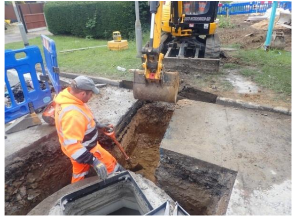
Plate 136: Excavation of the service trench, from the north
