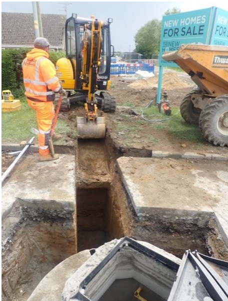
Plate 142: Excavation of the service trench, from the north
