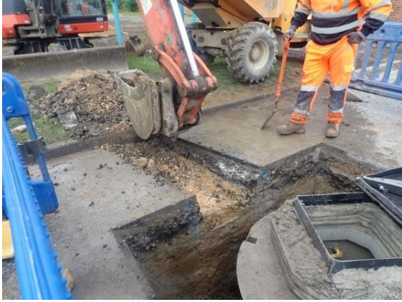
Plate 133: Excavation of the service trench, from the north-east
