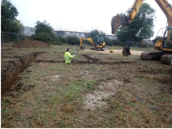
Plate 24: Excavation of the foundations, from the west
