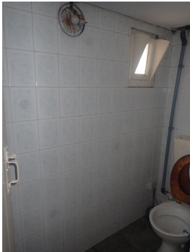
Plate 367: View of the interior of Cell 17, from the north-west
