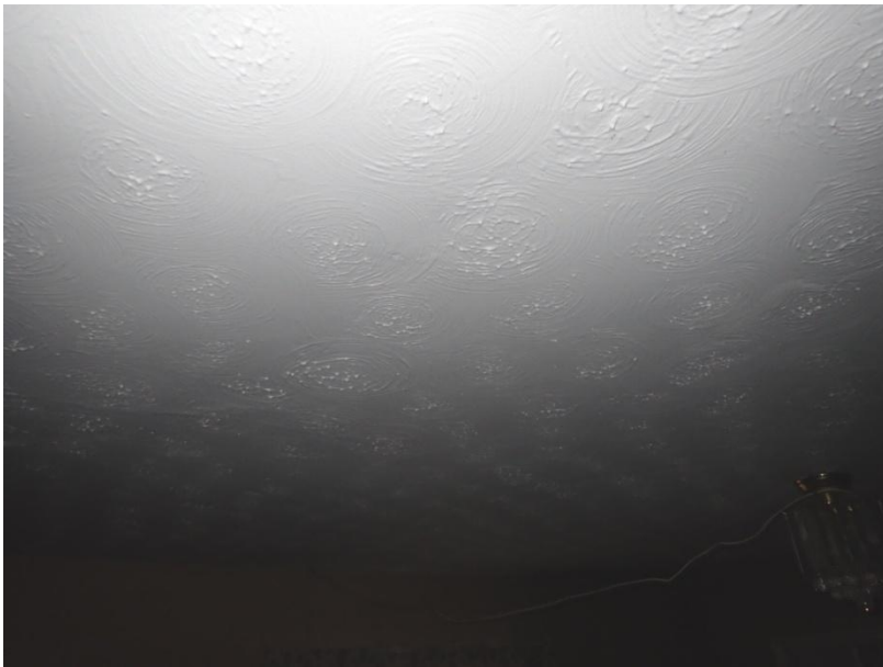
Plate 244: View of the ceiling of Cell 13, from the south
