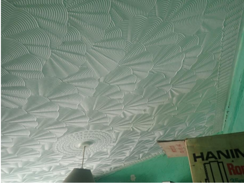
Plate 205: View of the ceiling of Cell 11, from the north-east
