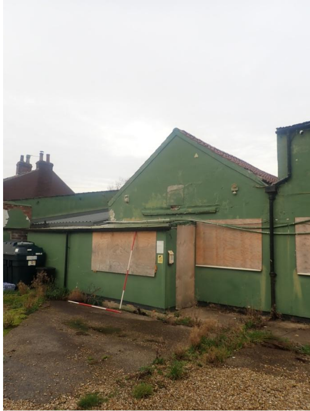
Plate 320: View of the South Elevation of Building 4, from the south-east
