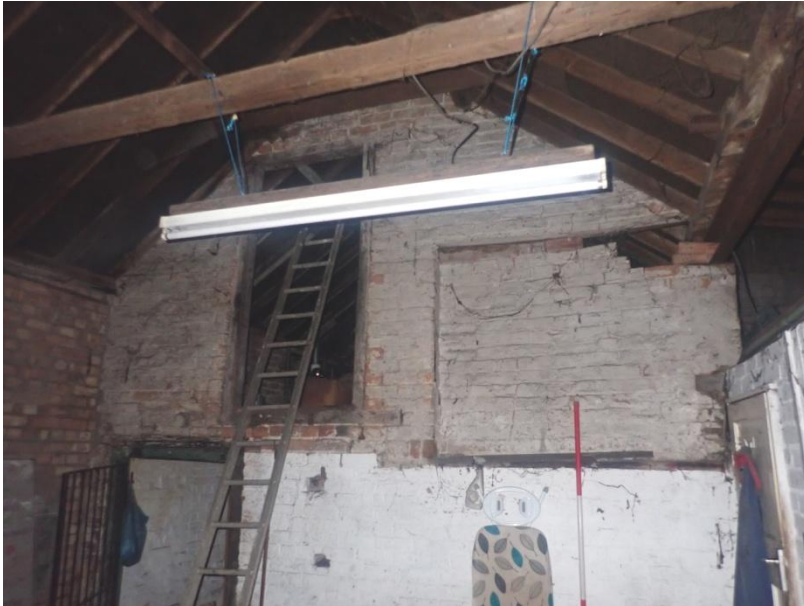
Plate 402: View of the east wall of Cell 19, from the south-west
