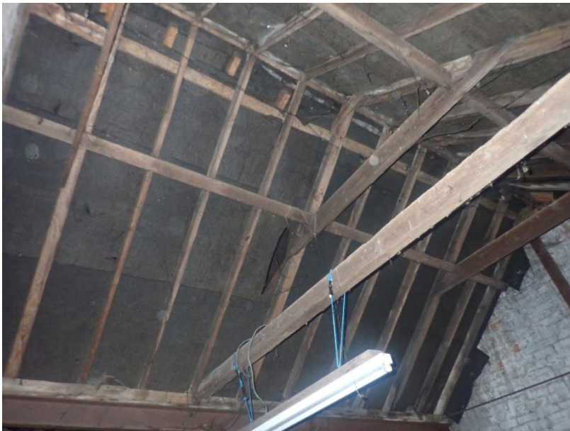
Plate 407: View of the roof supporting structure of Cell 19, from the south-west
