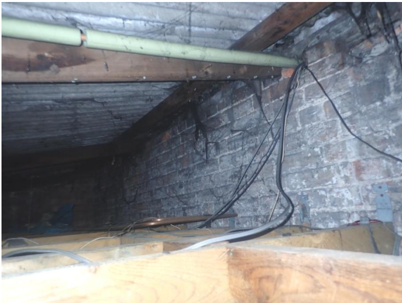
Plate 334: View of the roof space above Cell 16, from the north-east
