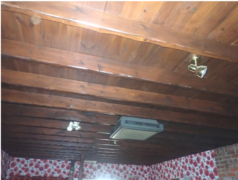
Plate 299: View of the ceiling of Cell 15, from the north-east
