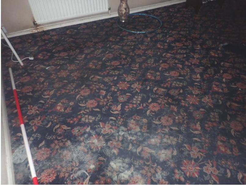
Plate 239: View of the flooring of Cell 13, from the south
