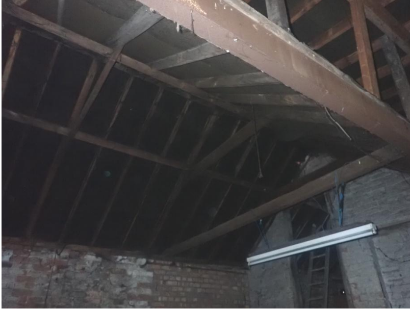
Plate 404: View of the roof supporting structure of Cell 19, from the south-west
