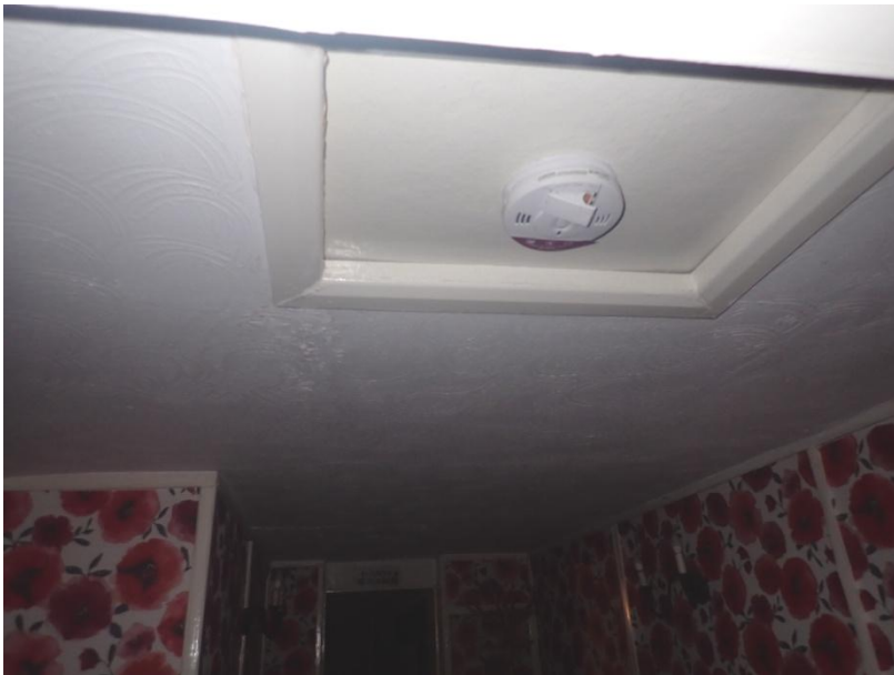
Plate 325: View of the ceiling of Cell 16, from the north-east
