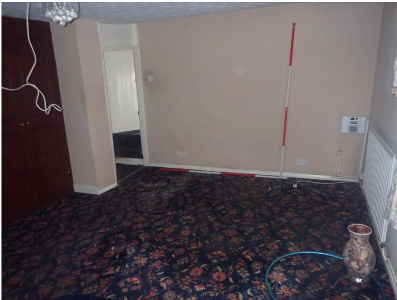
Plate 246: View of the west wall of Cell 13, from the north-east
