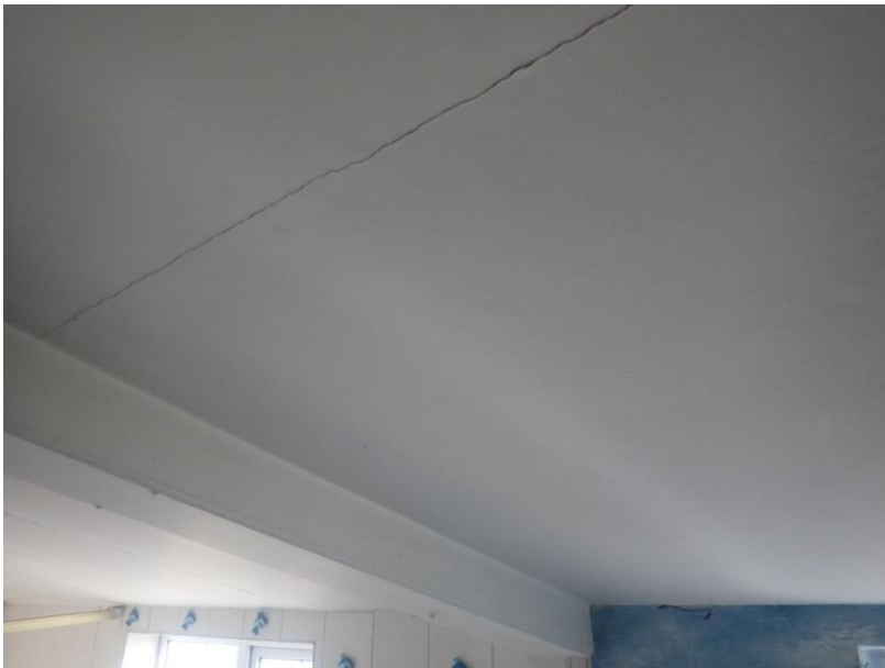
Plate 260: View of the ceiling of Cell 14, from the north-west
