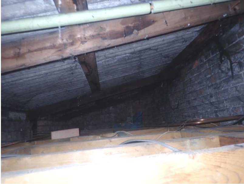
Plate 335: View of the roof space above Cell 16, from the north-east
