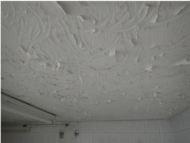
Plate 359: View of the interior of Cell 17, from the north-east
