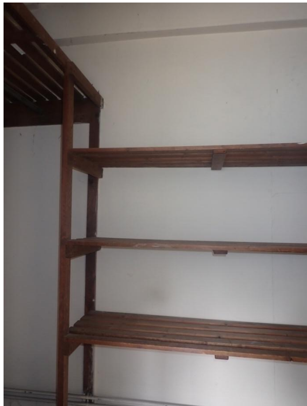
Plate 276: View of the airing cupboard within the north wall of Cell 14, from the south-west
