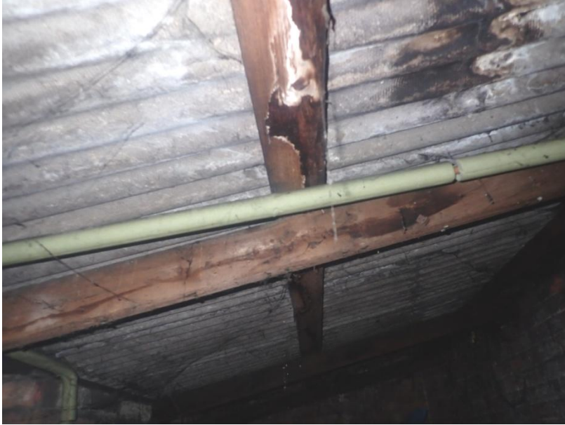
Plate 331: View of the roof space above Cell 16, from the north-east
