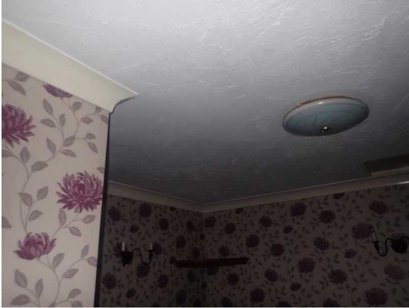
Plate 382: View of the ceiling of Cell 18, from the north-west
