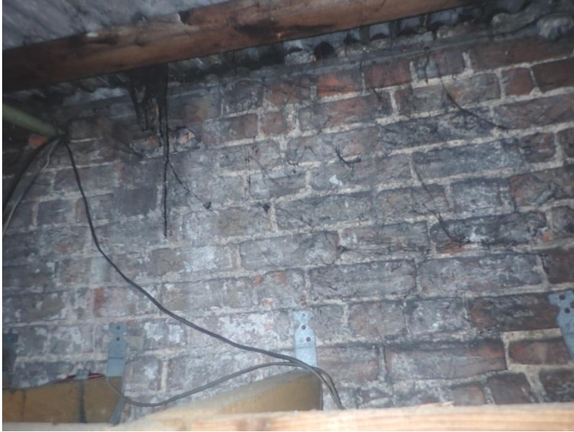
Plate 333: View of the roof space above Cell 16, from the south-east
