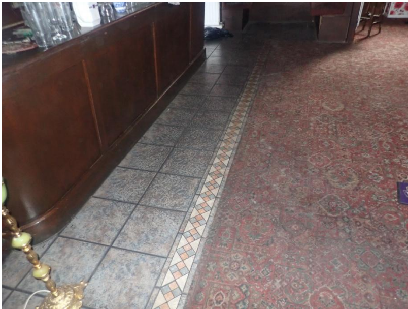
Plate 295: View of the flooring of Cell 15, from the north-west
