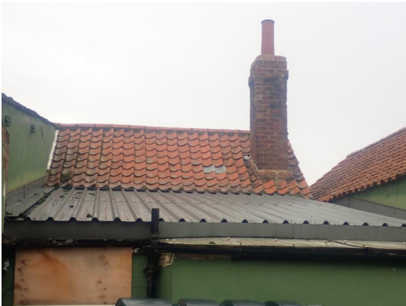
Plate 375: View of the roofing of Building 5, from the south-east
