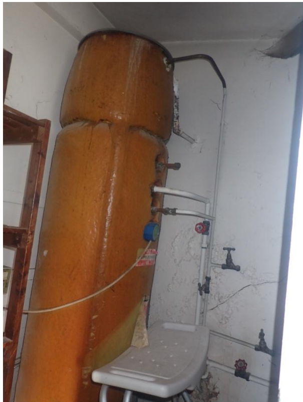
Plate 274: View of the airing cupboard within the north wall of Cell 14, from the south-west
