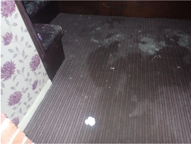
Plate 378: View of the flooring of Cell 18, from the north-east
