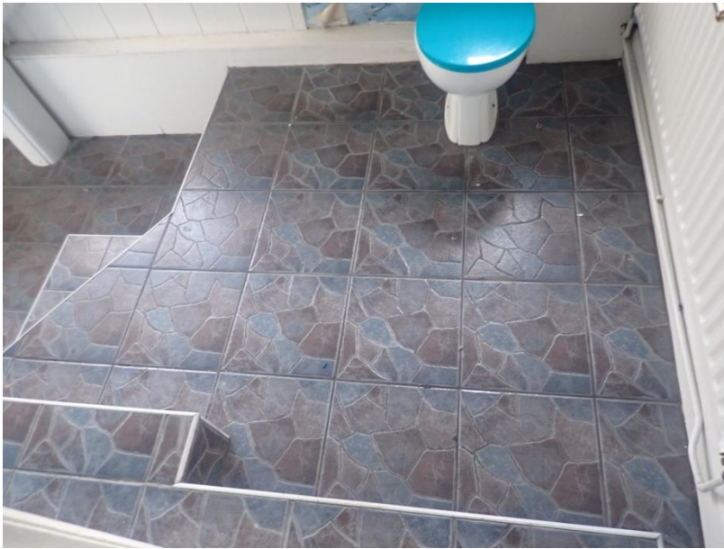
Plate 253: View of the flooring of Cell 14, from the north-west
