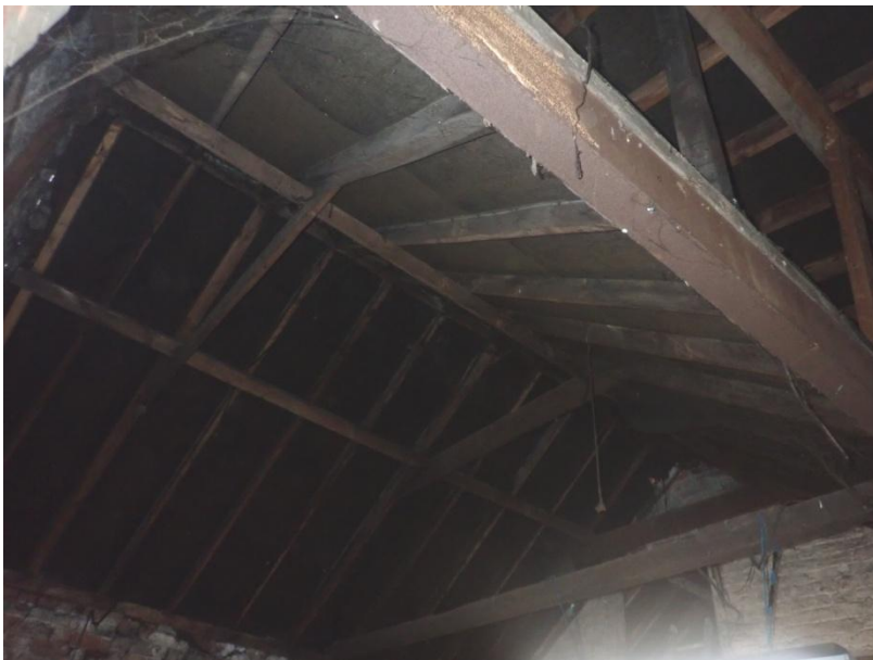
Plate 403: View of the roof supporting structure of Cell 19, from the south-west
