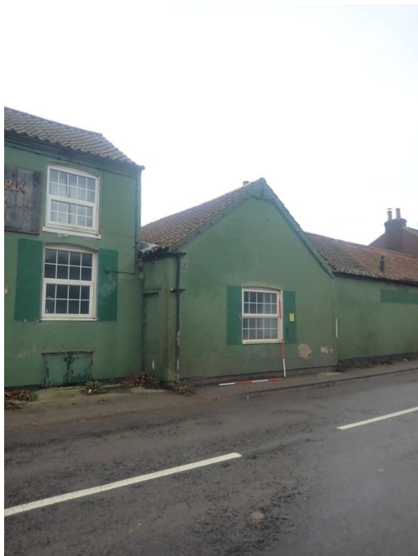
Plate 286: View of the North Elevation of Building 3, from the north-east
