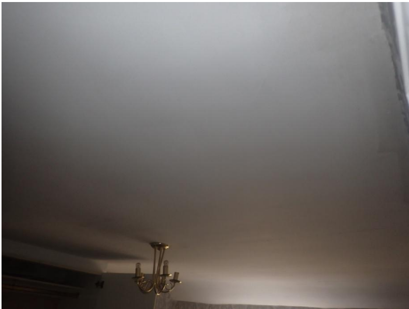
Plate 228: View of the ceiling of Cell 12, from the south
