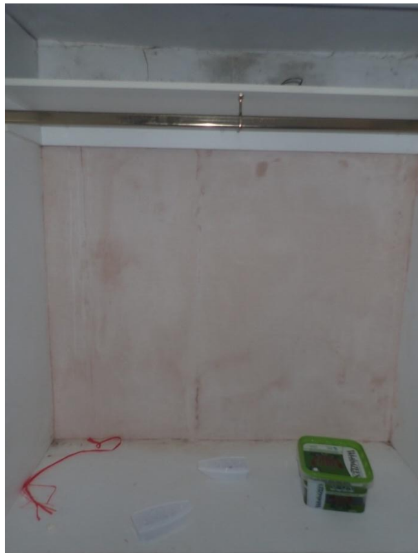
Plate 236: View of the west wall of Cell 12, from the south-east
