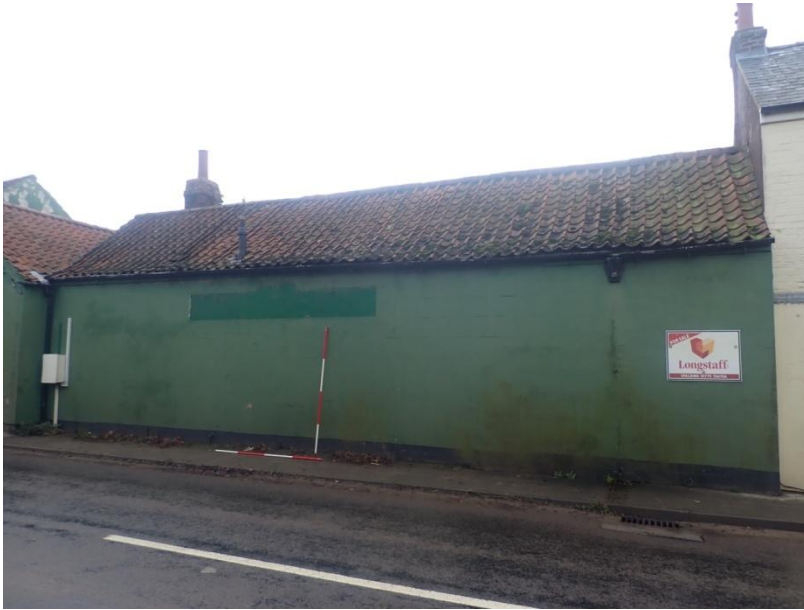
Plate 376: View of the North Elevation of Building 5, from the north-west
