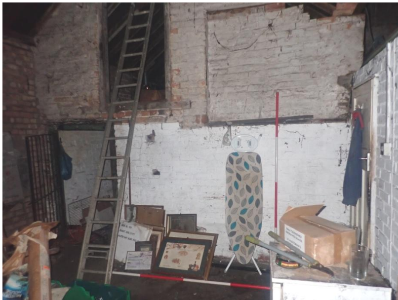
Plate 401: View of the east wall of Cell 19, from the south-west
