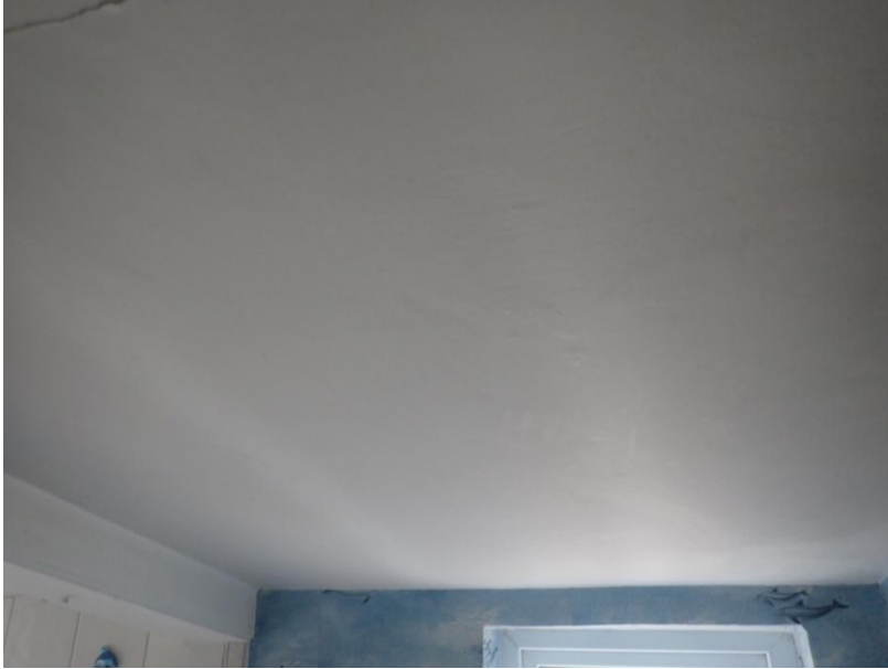
Plate 261: View of the ceiling of Cell 14, from the north
