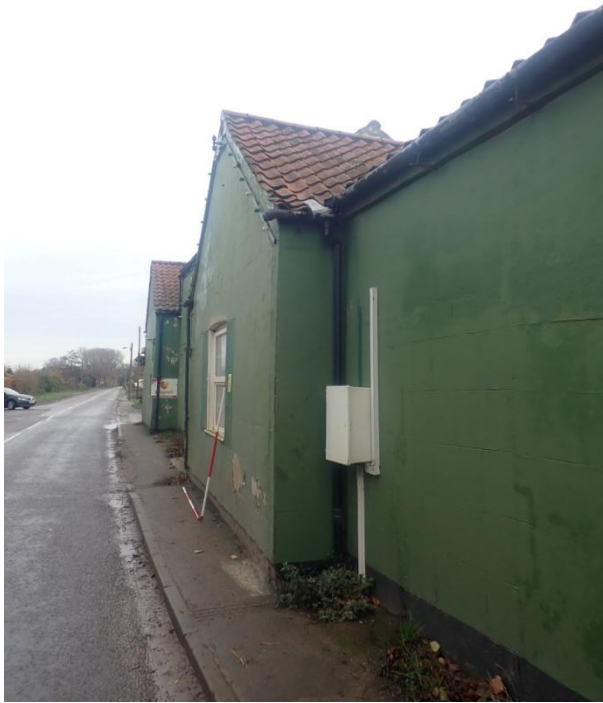
Plate 287: View of the North Elevation of Building 3, from the west
