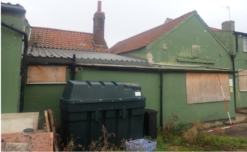
Plate 318: View of the South Elevation of Building 4, from the south-west
