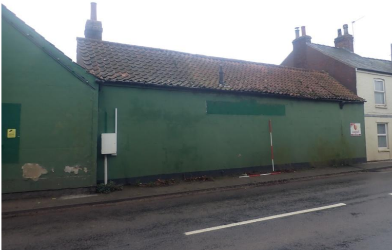
Plate 377: View of the North Elevation of Building 5, from the north-east
