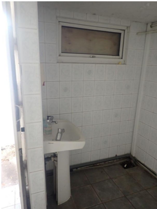
Plate 361: View of the interior of Cell 17, from the north-east
