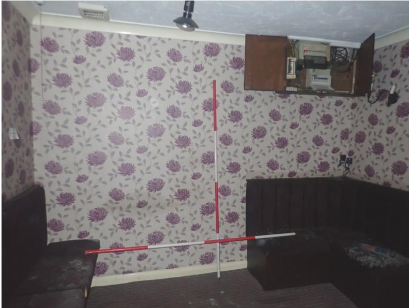
Plate 390: View of the north wall of Cell 18, from the south-east
