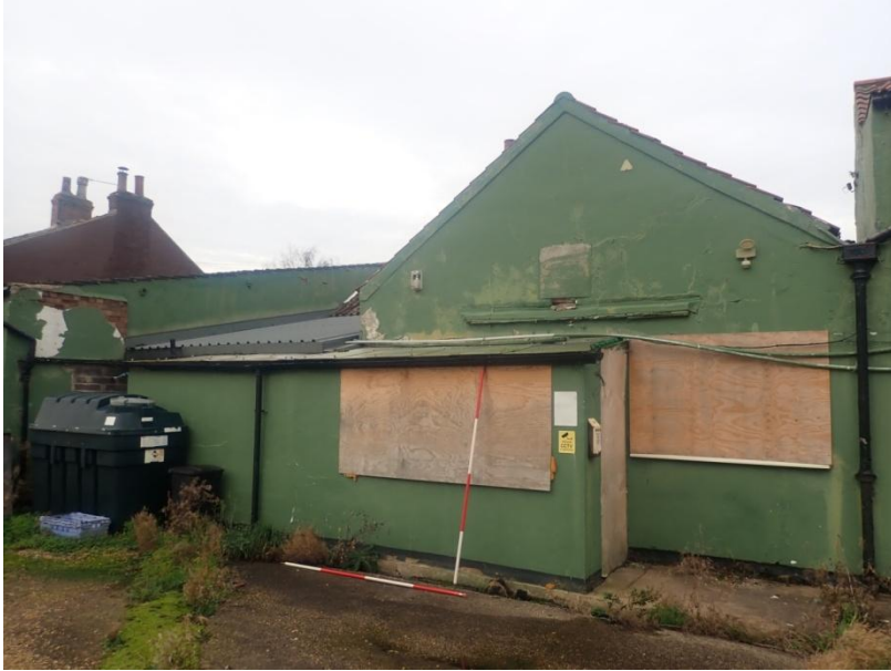
Plate 281: View of the South Elevation of Building 3, from the south-east
