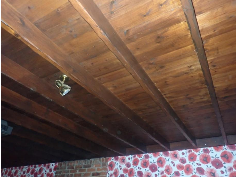
Plate 300: View of the ceiling of Cell 15, from the north-east
