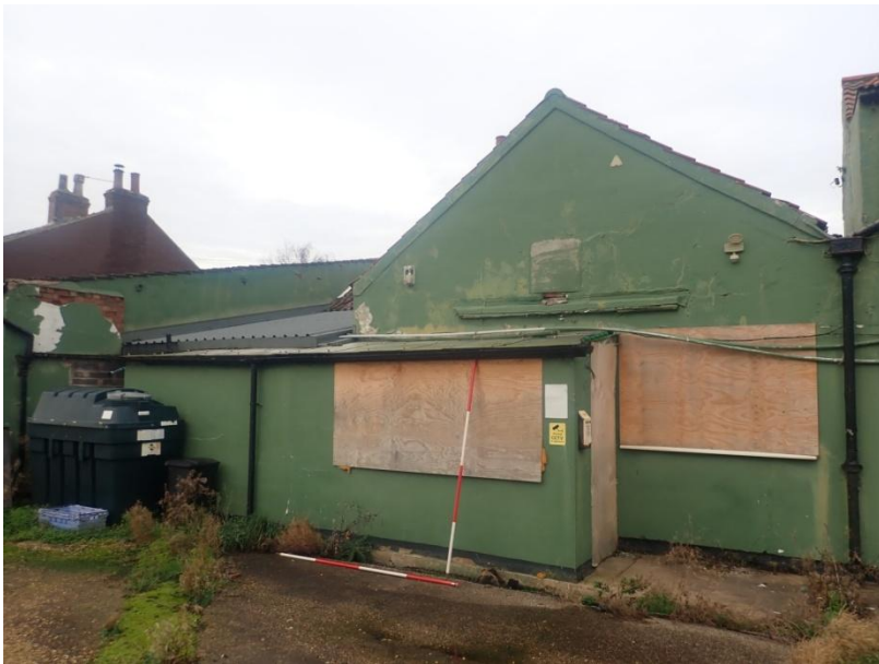
Plate 319: View of the South Elevation of Building 4, from the south-east
