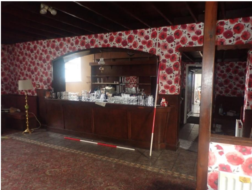
Plate 315: View of the east wall of Cell 15, from the south-west
