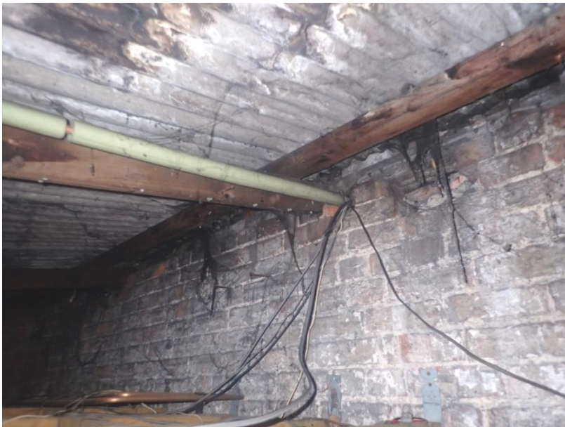
Plate 332: View of the roof space above Cell 16, from the north-east
