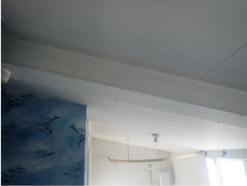
Plate 259: View of the ceiling of Cell 14, from the south-west
