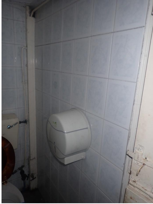
Plate 372: View of the interior of Cell 17, from the north-west
