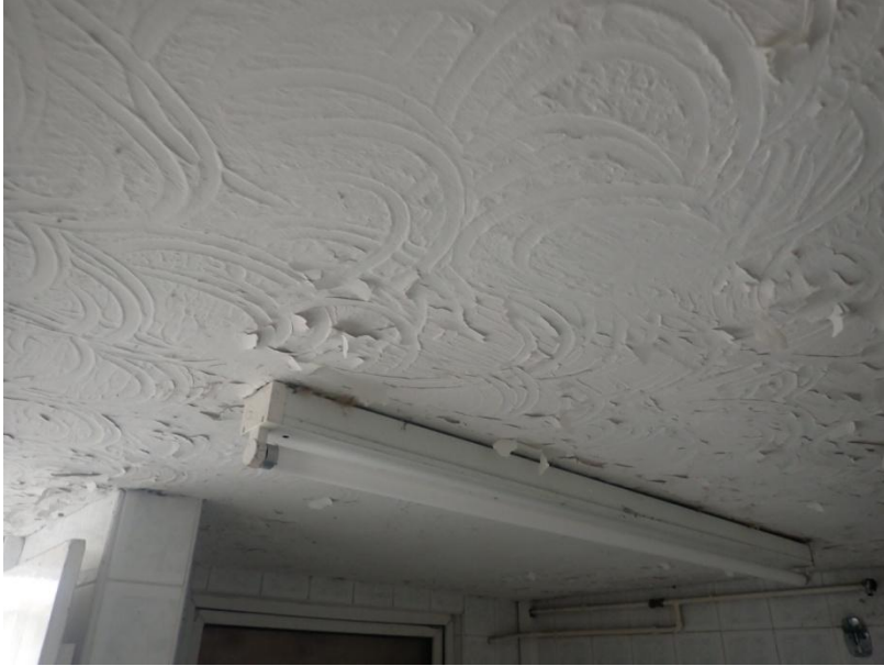
Plate 358: View of the interior of Cell 17, from the north
