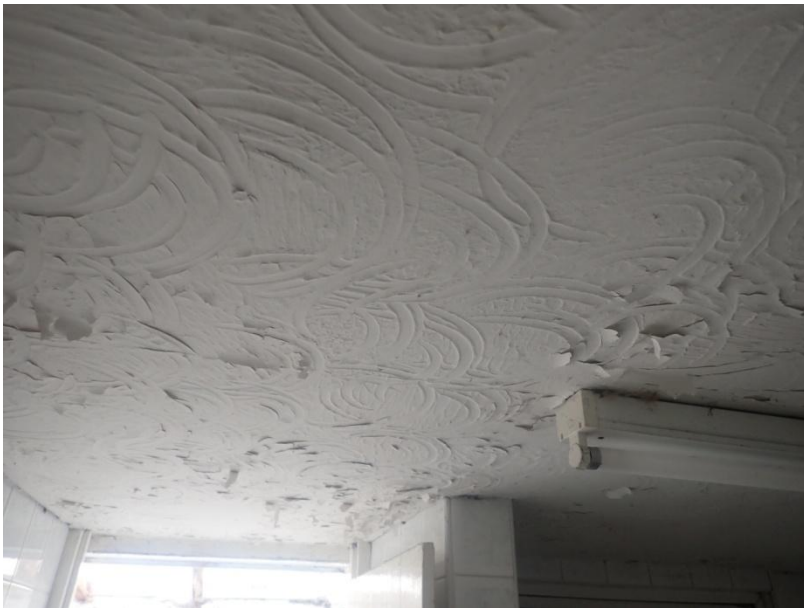
Plate 357: View of the interior of Cell 17, from the north-west
