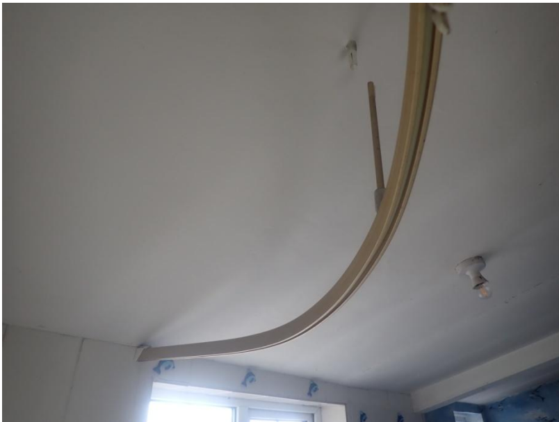
Plate 258: View of the ceiling of Cell 14, from the north
