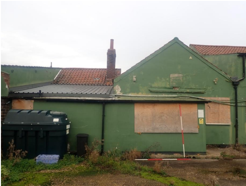
Plate 317: View of the South Elevation of Building 4, from the south-east
