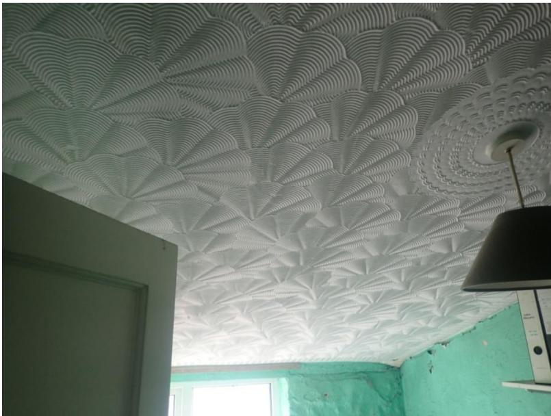
Plate 206: View of the ceiling of Cell 11, from the north
