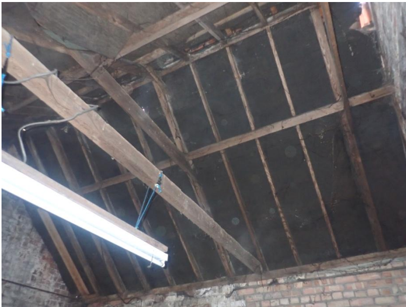
Plate 405: View of the roof supporting structure of Cell 19, from the south-east
