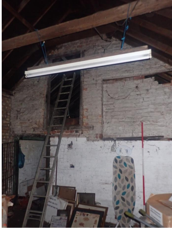
Plate 400: View of the east wall of Cell 19, from the south-west
