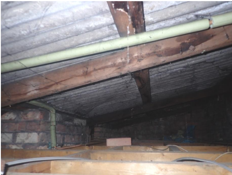
Plate 336: View of the roof space above Cell 16, from the north-east
