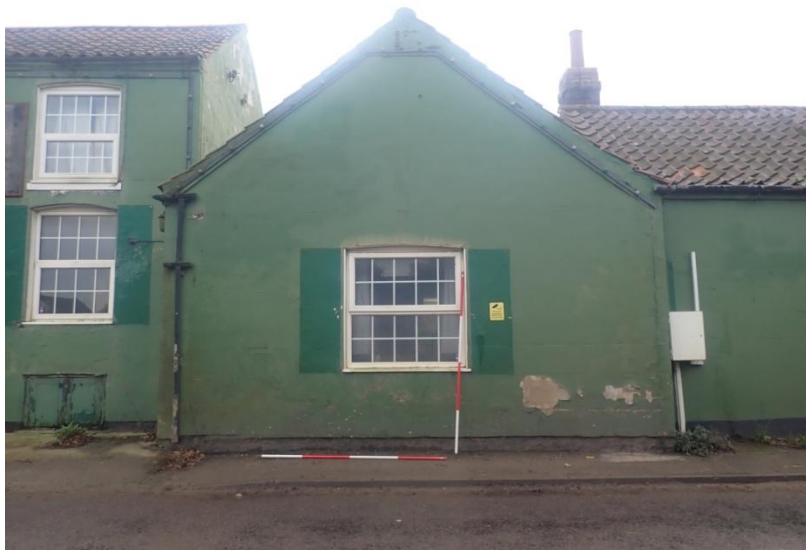
Plate 284: View of the North Elevation of Building 3, from the north-west
