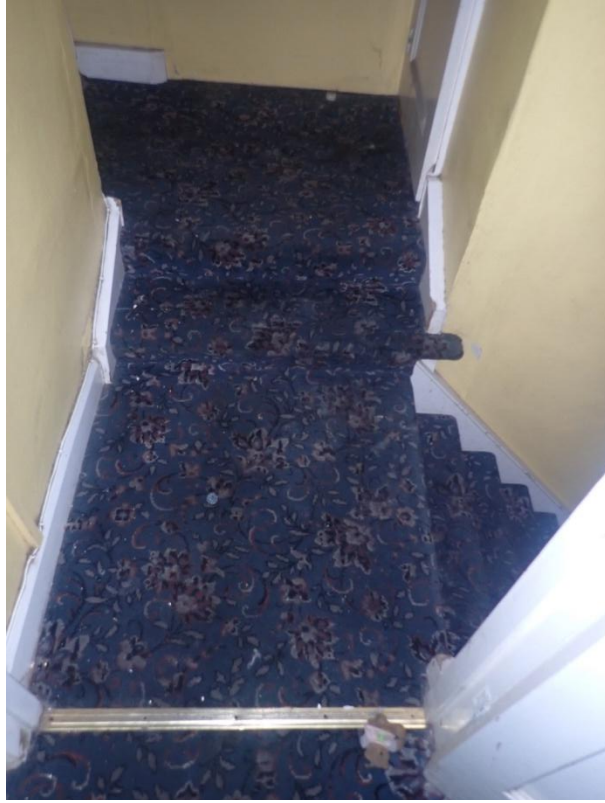
Plate 212: View of the first floor landing of Building 2, from the south-west
