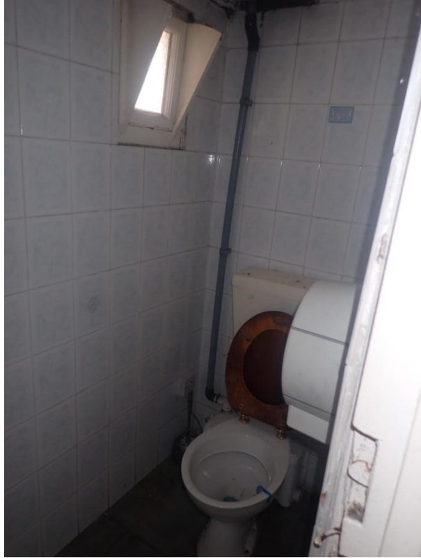
Plate 366: View of the interior of Cell 17, from the north-west
