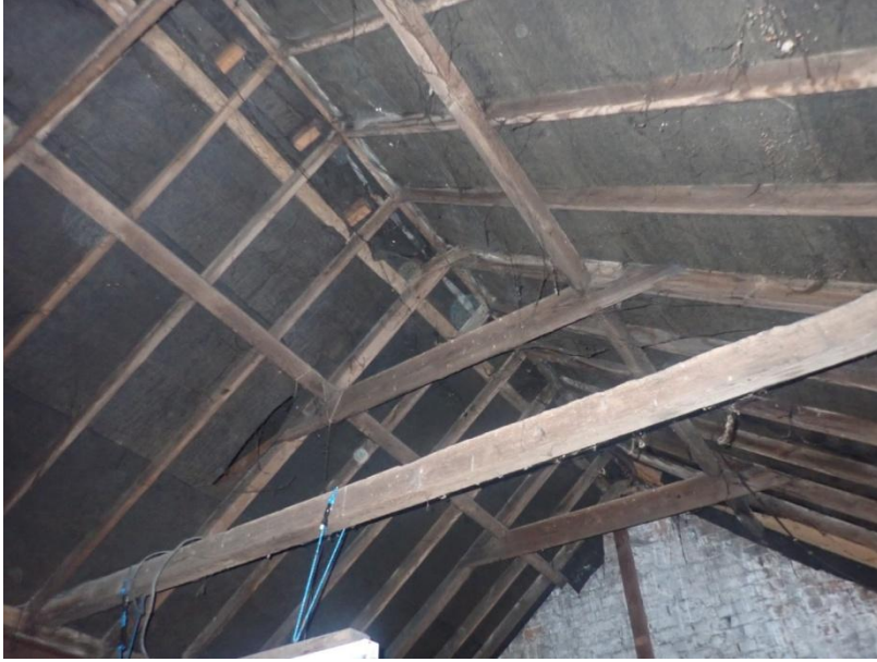
Plate 408: View of the roof supporting structure of Cell 19, from the north-east
