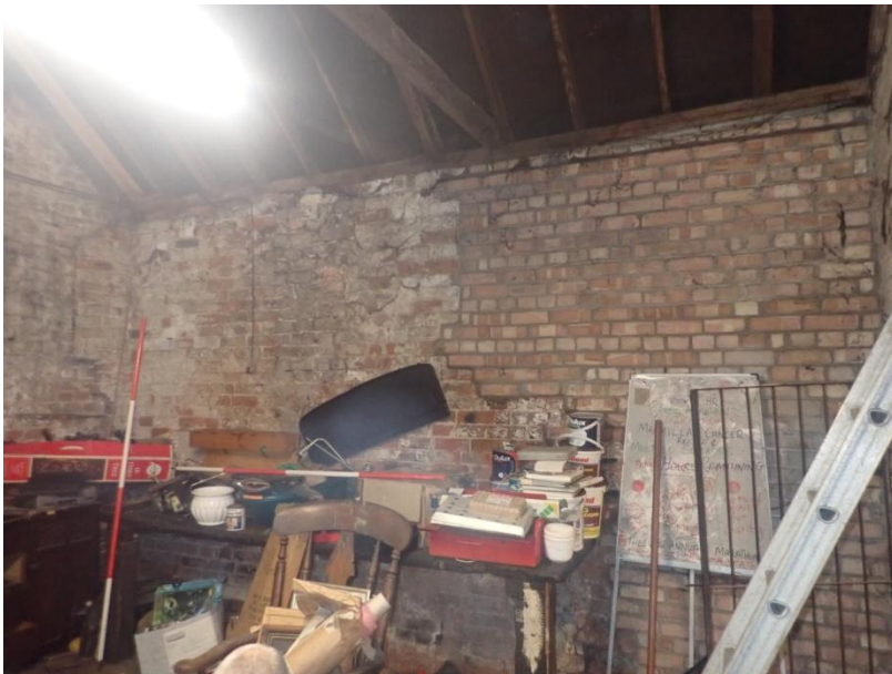
Plate 397: View of the north wall of Cell 19, from the south-east
