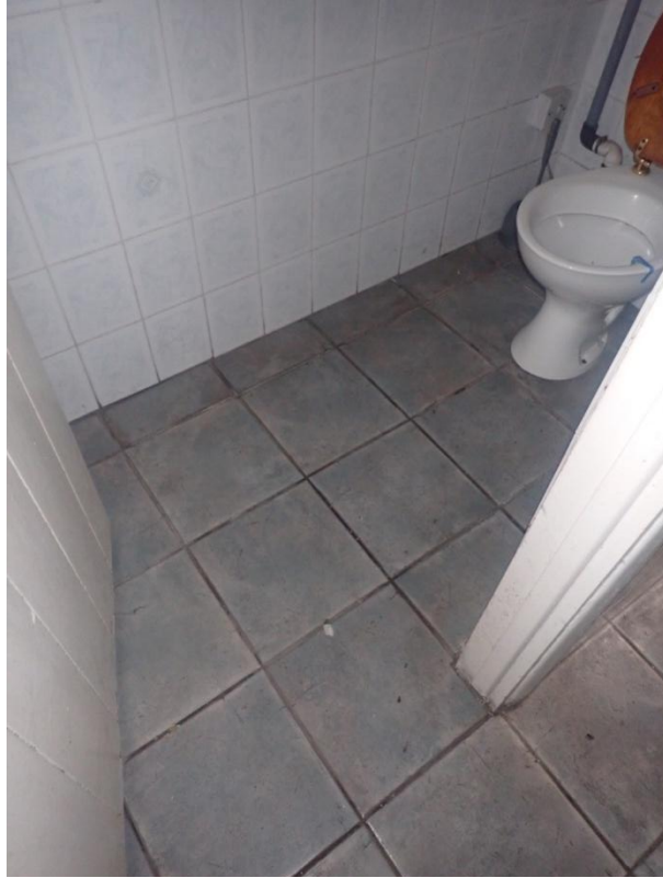
Plate 368: View of the interior of Cell 17, from the north-west
