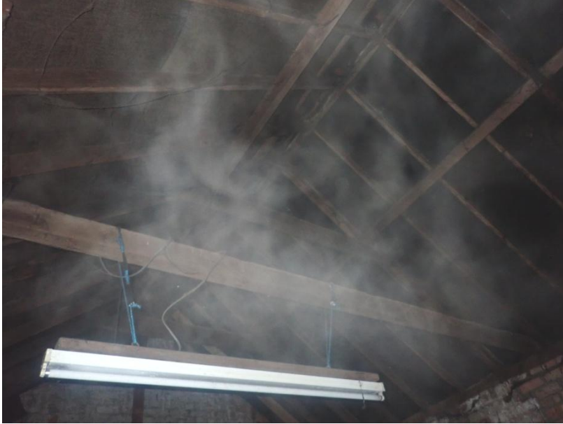
Plate 406: View of the roof supporting structure of Cell 19, from the south-east
