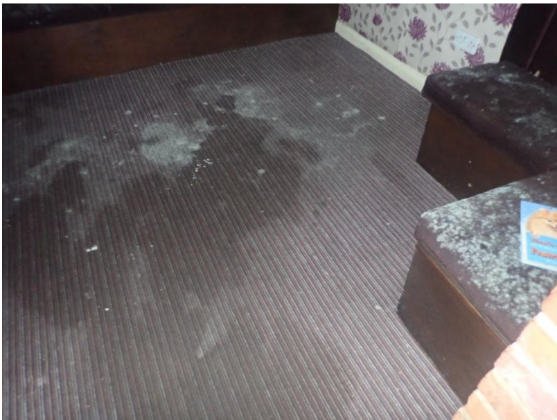
Plate 379: View of the flooring of Cell 18, from the south-east
