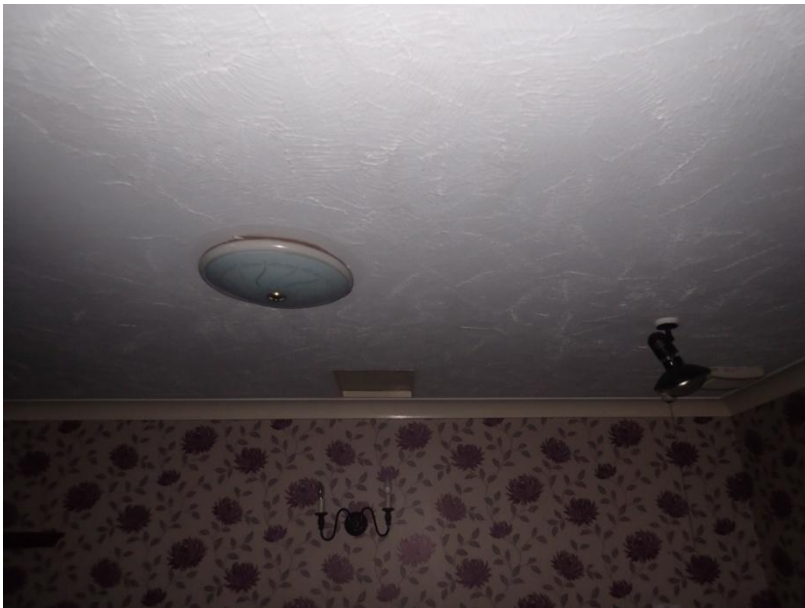
Plate 381: View of the ceiling of Cell 18, from the north-east
