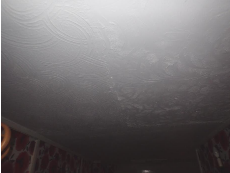
Plate 324: View of the ceiling of Cell 16, from the south-west
