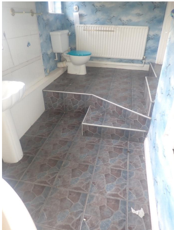
Plate 256: View of the flooring of Cell 14, from the north-east
