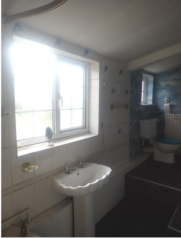
Plate 267: View of the north wall of Cell 14, from the north-east
