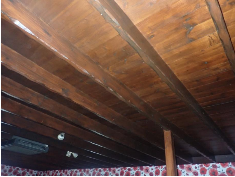
Plate 302: View of the ceiling of Cell 15, from the south-west
