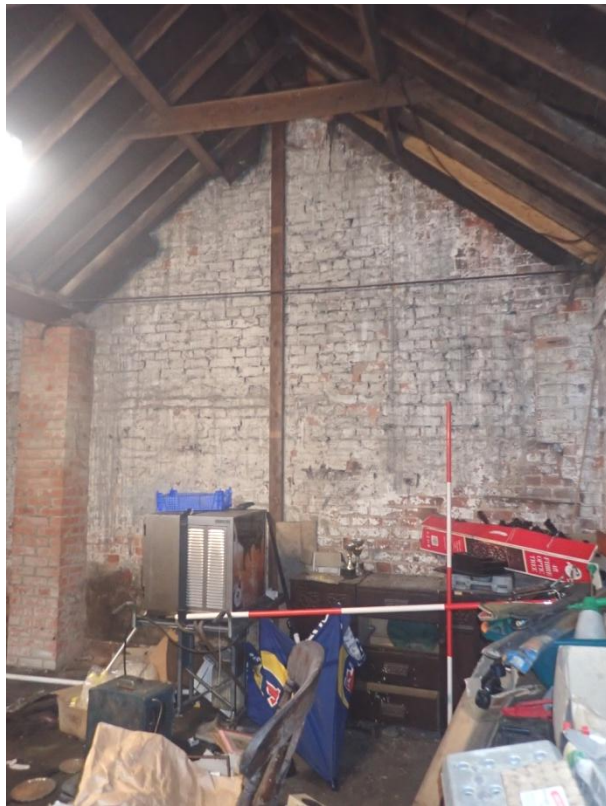
Plate 399: View of the west wall of Cell 19, from the north-east
