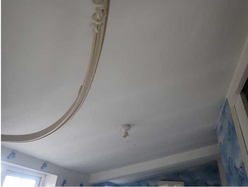
Plate 257: View of the ceiling of Cell 14, from the north-east
