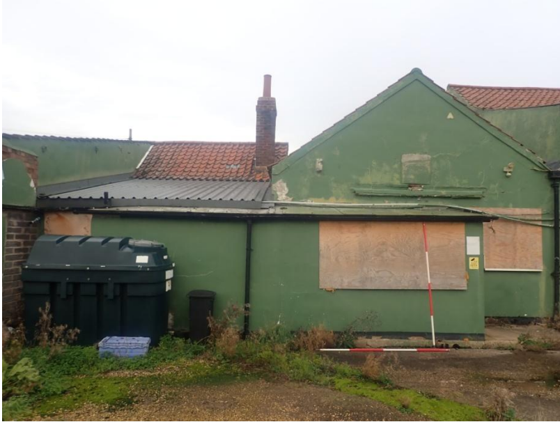
Plate 279: View of the South Elevation of Building 3, from the south-east
