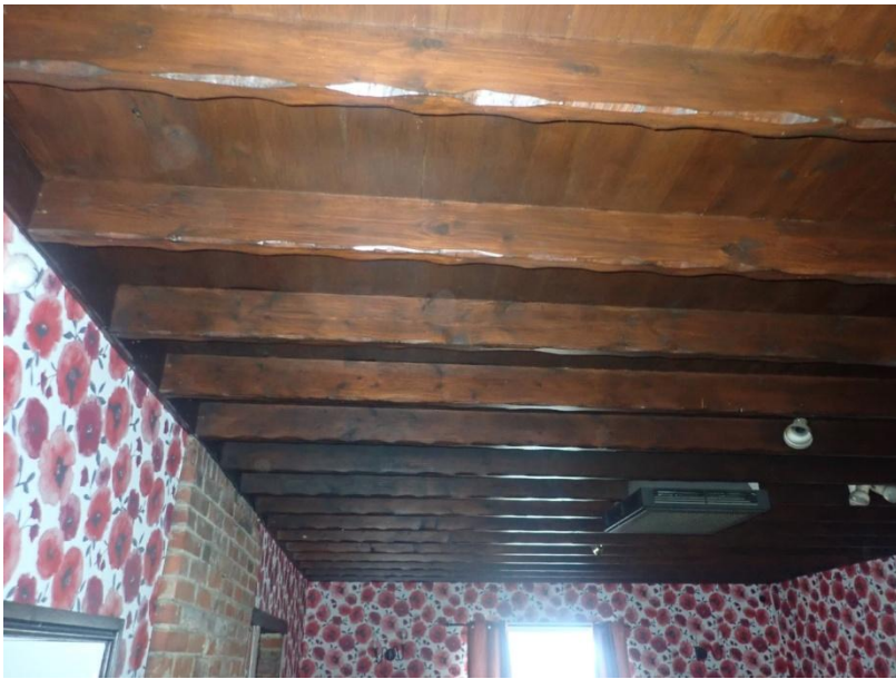
Plate 301: View of the ceiling of Cell 15, from the south
