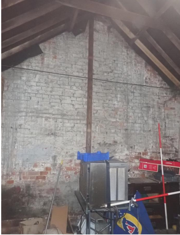
Plate 398: View of the west wall of Cell 19, from the north-east
