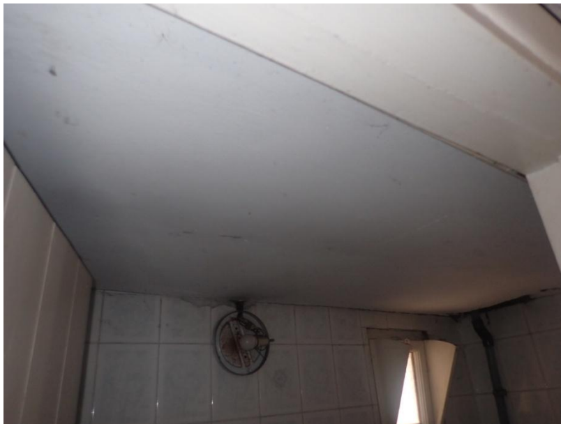
Plate 369: View of the interior of Cell 17, from the north-west
