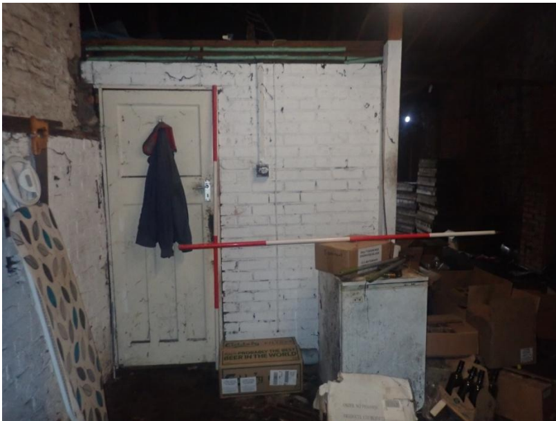
Plate 395: View of the south wall of Cell 19, from the north-west
