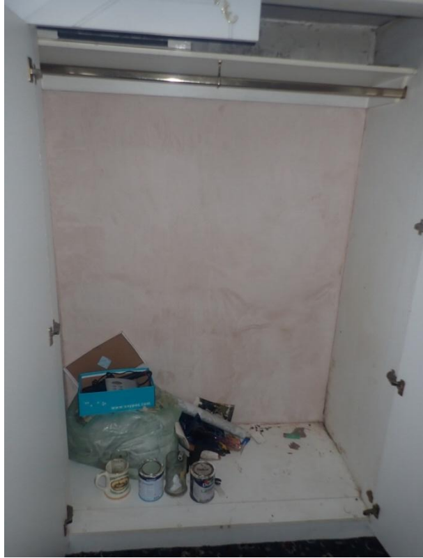
Plate 235: View of the west wall of Cell 12, from the south-east
