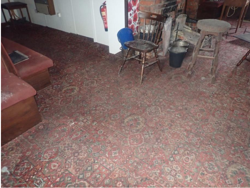
Plate 290: View of the flooring of Cell 15, from the south-east
