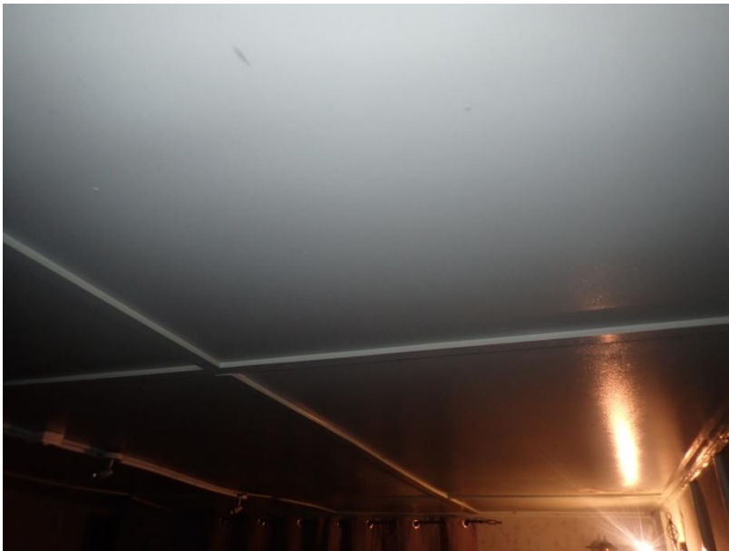
Plate 474: View of the ceiling of Cell 24, from the north-west
