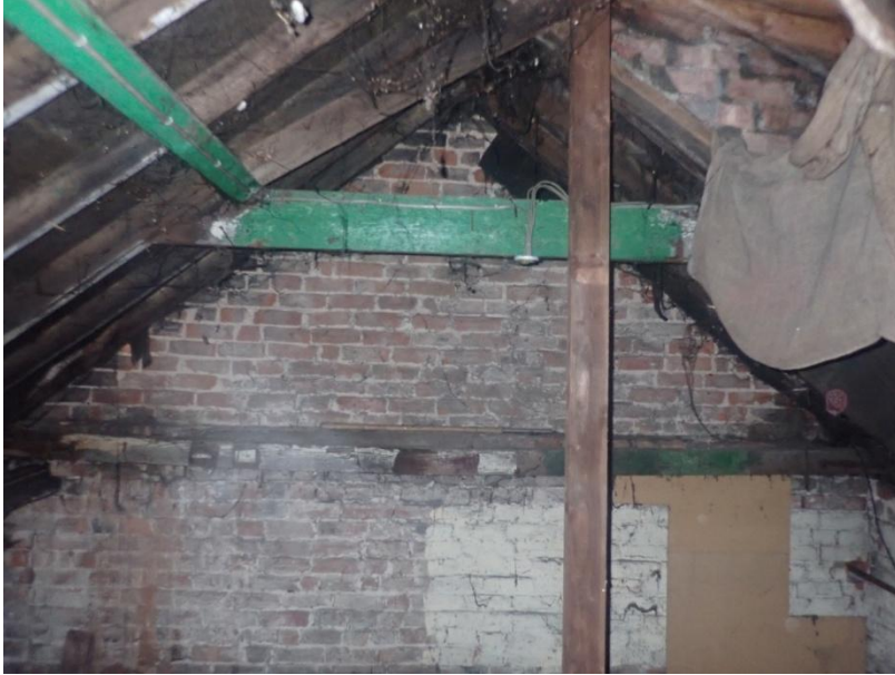
Plate 411: View of the east wall of Cell 20, from the south-west
