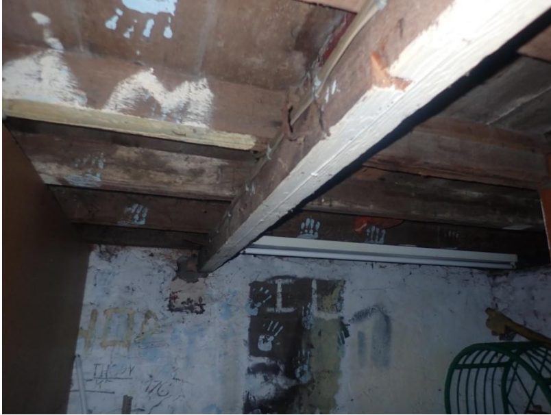
Plate 442: View of the ceiling structure of Cell 22, from the south-west
