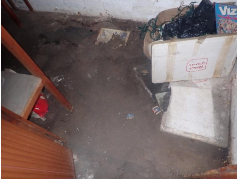
Plate 451: View of the flooring of Cell 23, from the north-west
