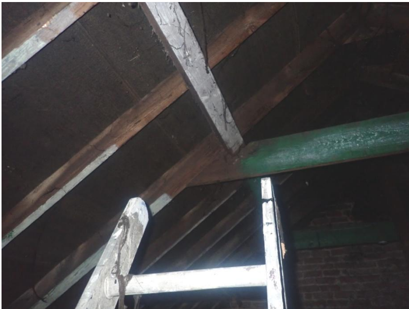
Plate 424: View of the roof supporting structure of Cell 20, from the north-west
