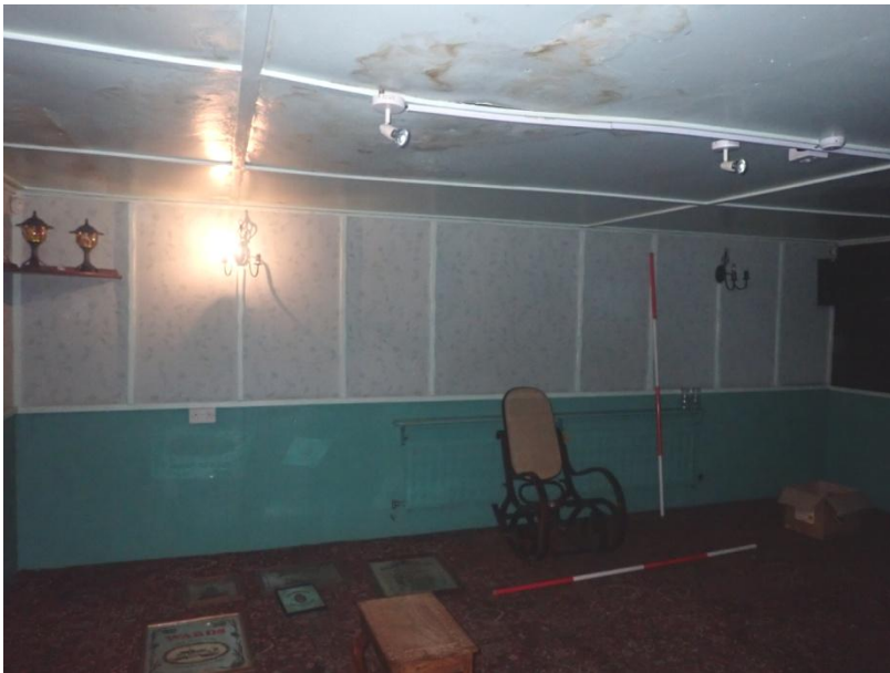
Plate 480: View of the west wall of Cell 24, from the south-east
