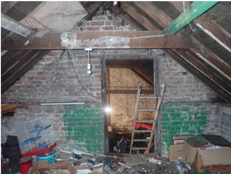
Plate 412: View of the west wall of Cell 20, from the east
