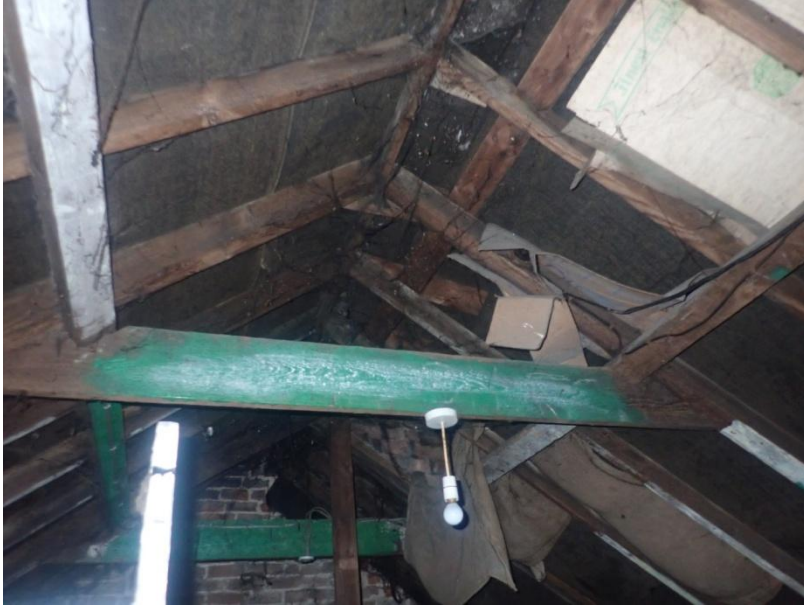
Plate 425: View of the roof supporting structure of Cell 20, from the north-west
