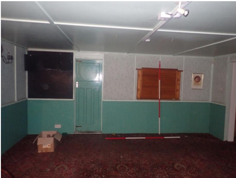
Plate 476: View of the north wall of Cell 24, from the south-east
