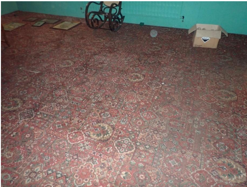
Plate 468: View of the flooring of Cell 24, from the north-east
