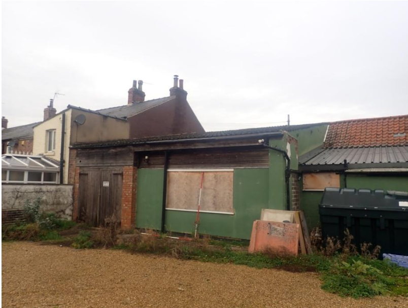
Plate 463: View of the South Elevation of Building 6, from the south-east
