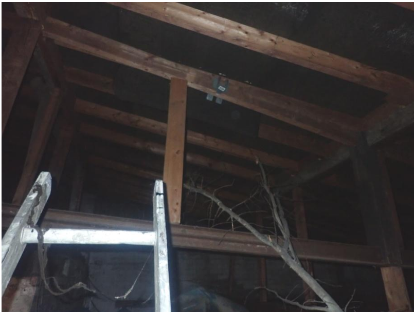
Plate 498: View of the roof supporting structure of Building 6, from the north-west
