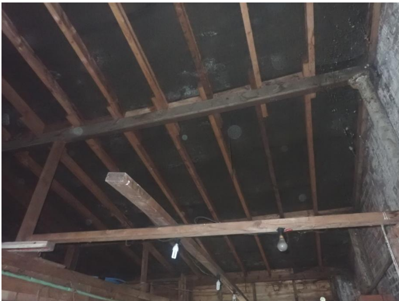
Plate 492: View of the roof supporting structure of Building 6, from the north-west
