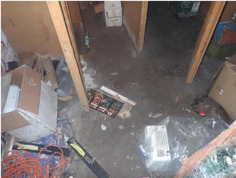
Plate 426: View of the flooring of Cell 21, from the north-west
