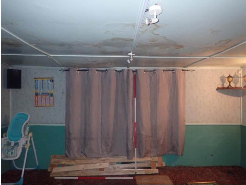
Plate 475: View of the south wall of Cell 24, from the north-west
