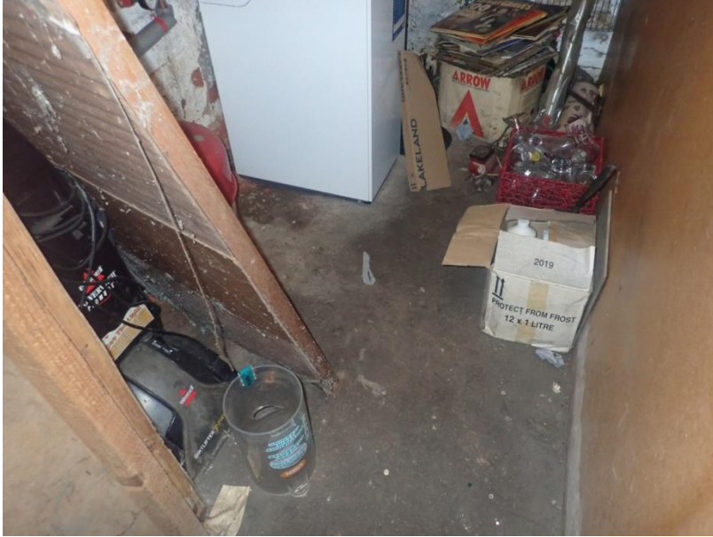
Plate 427: View of the flooring of Cell 21, from the north-west
