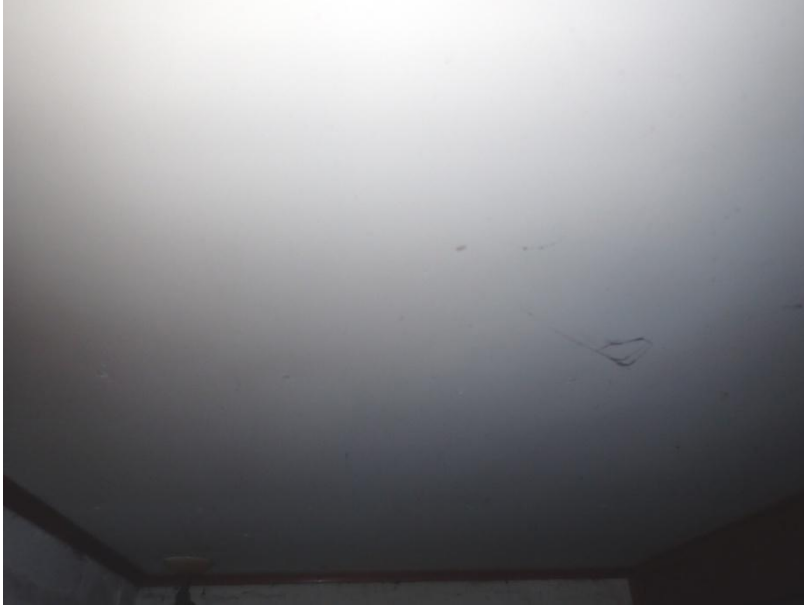
Plate 457: View of the ceiling of Cell 23, from the north-east
