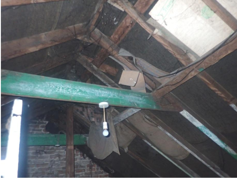
Plate 423: View of the roof supporting structure of Cell 20, from the north-west
