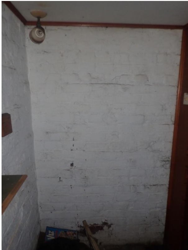
Plate 456: View of the interior of Cell 23, from the north-east
