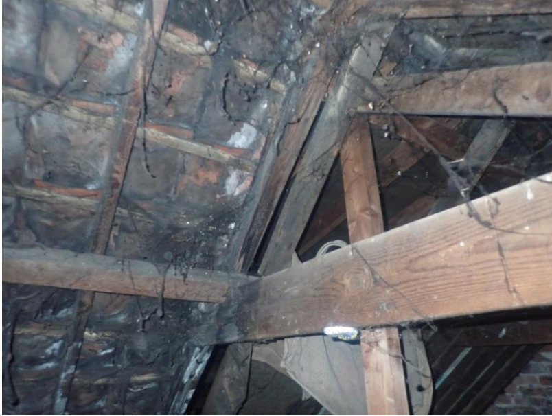
Plate 415: View of the roof supporting structure of Cell 20, from the north-east
