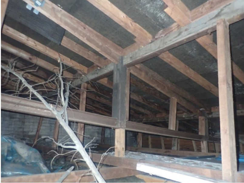
Plate 499: View of the roof supporting structure of Building 6, from the north-west
