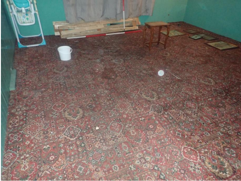
Plate 467: View of the flooring of Cell 24, from the north-east
