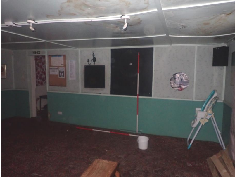
Plate 477: View of the east wall of Cell 24, from the south-west
