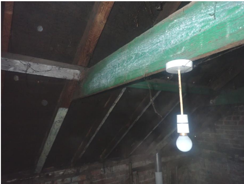
Plate 420: View of the roof supporting structure of Cell 20, from the south-west
