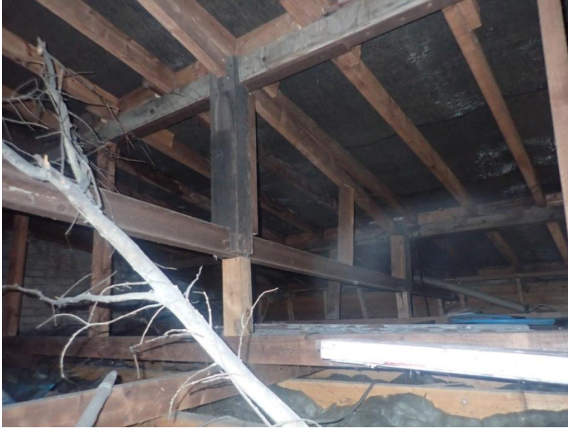
Plate 503: View of the roof supporting structure of Building 6, from the north-west
