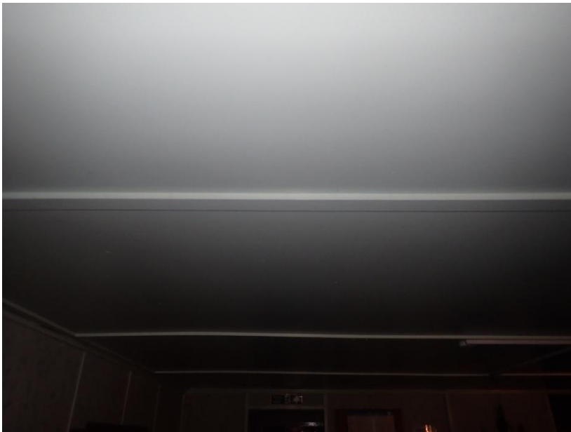
Plate 472: View of the ceiling of Cell 24, from the north-east
