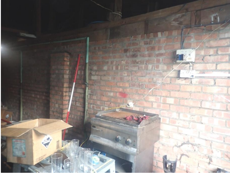
Plate 485: View of the east wall of Cell 25, from the south-west
