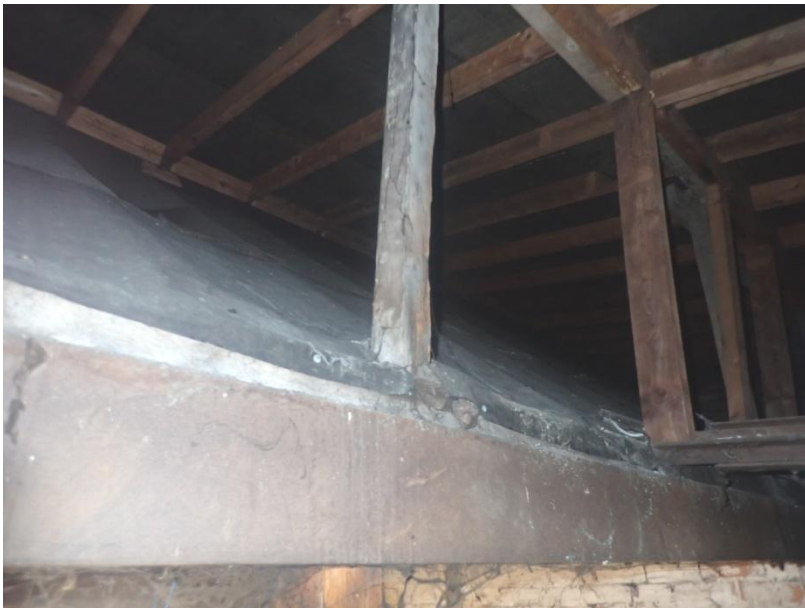
Plate 500: View of the roof supporting structure of Building 6, from the south-west
