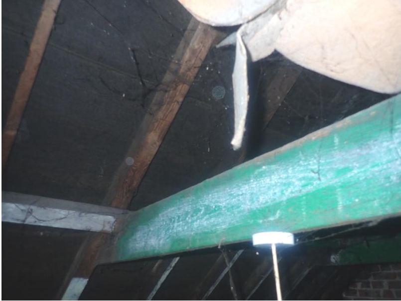
Plate 421: View of the roof supporting structure of Cell 20, from the north
