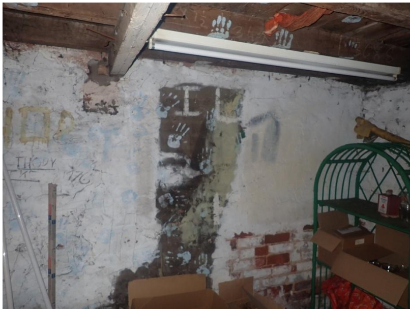
Plate 447: View of the interior of Cell 22, from the north-west
