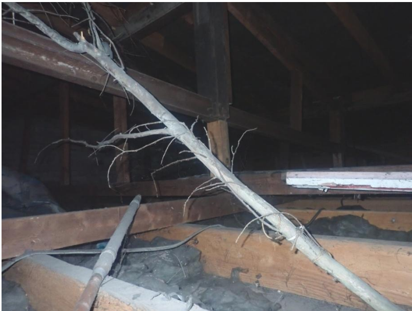
Plate 502: View of the roof supporting structure of Building 6, from the north-west
