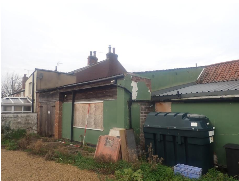
Plate 464: View of the East Elevation of Building 6, from the south-east
