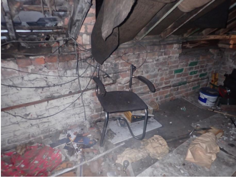
Plate 413: View of the south wall of Cell 20, from the north-east
