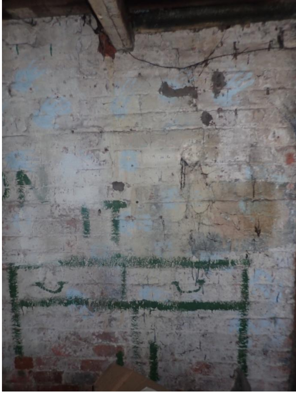
Plate 436: View of the interior of Cell 21, from the east
