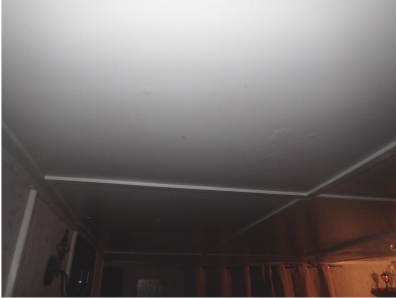
Plate 469: View of the ceiling of Cell 24, from the north-east
