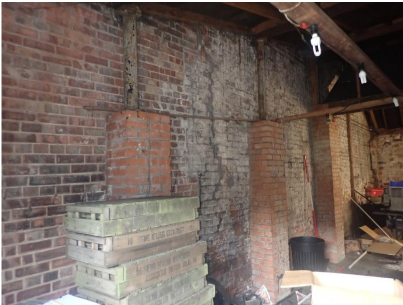
Plate 488: View of the west wall of Cell 25, from the south-east
