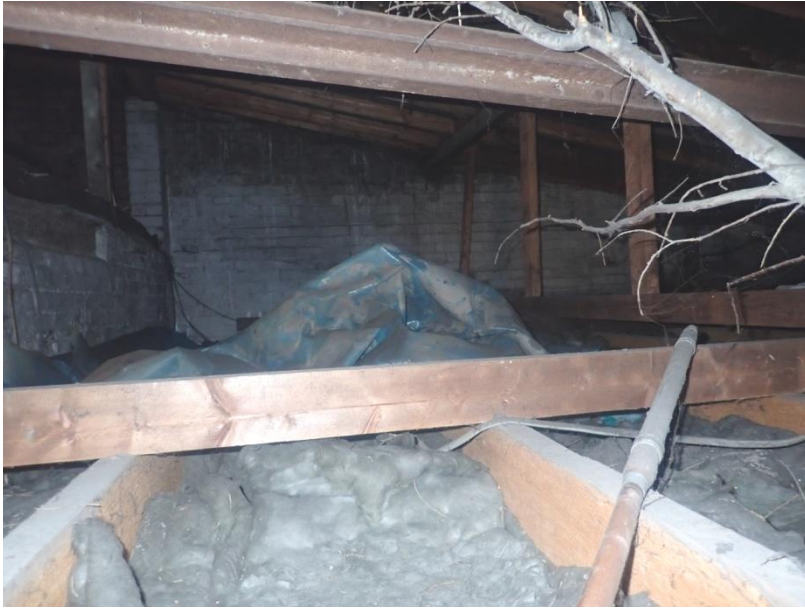
Plate 501: View of the roof supporting structure of Building 6, from the north-west
