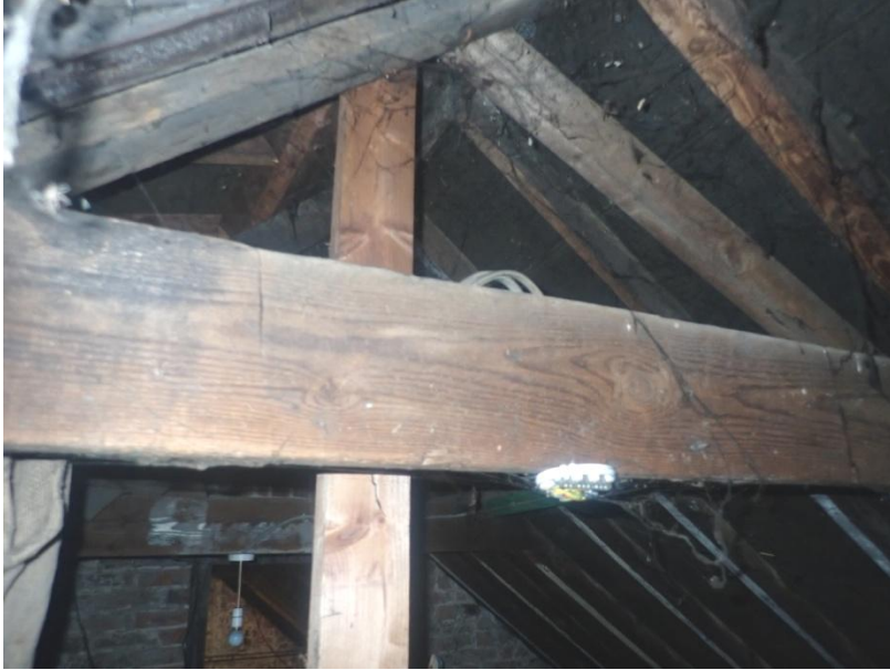
Plate 417: View of the roof supporting structure of Cell 20, from the south-east
