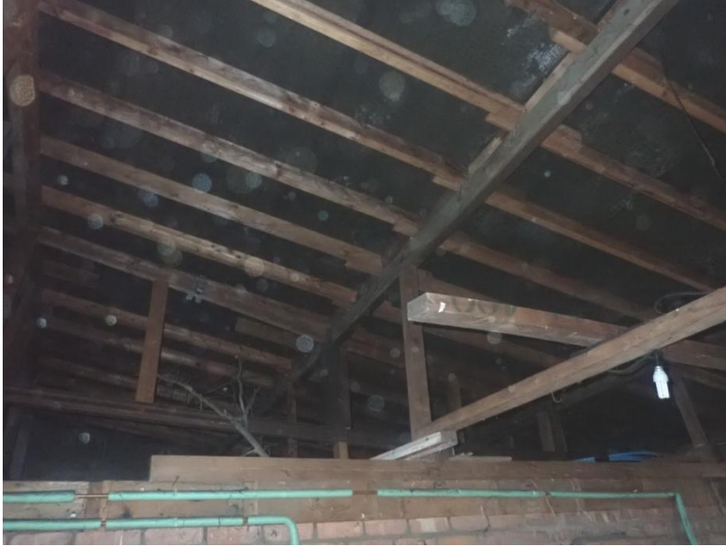
Plate 493: View of the roof supporting structure of Building 6, from the north-west
