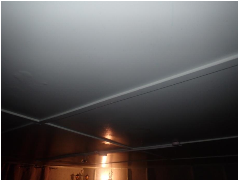
Plate 470: View of the ceiling of Cell 24, from the north-east
