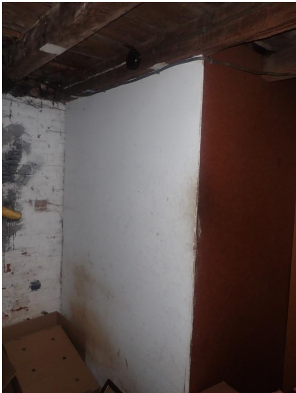
Plate 449: View of the interior of Cell 22, from the north-east
