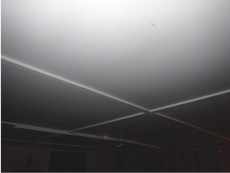
Plate 473: View of the ceiling of Cell 24, from the north-west
