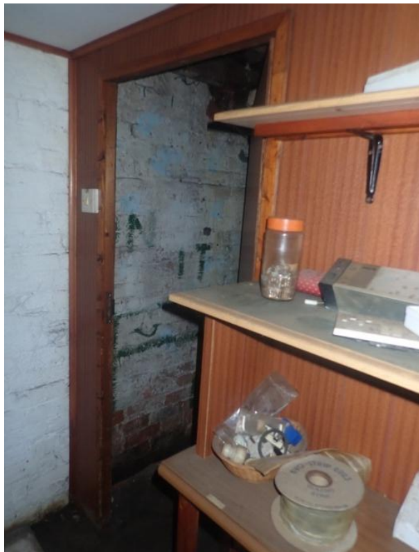
Plate 460 View of the interior of Cell 23, from the north-east
