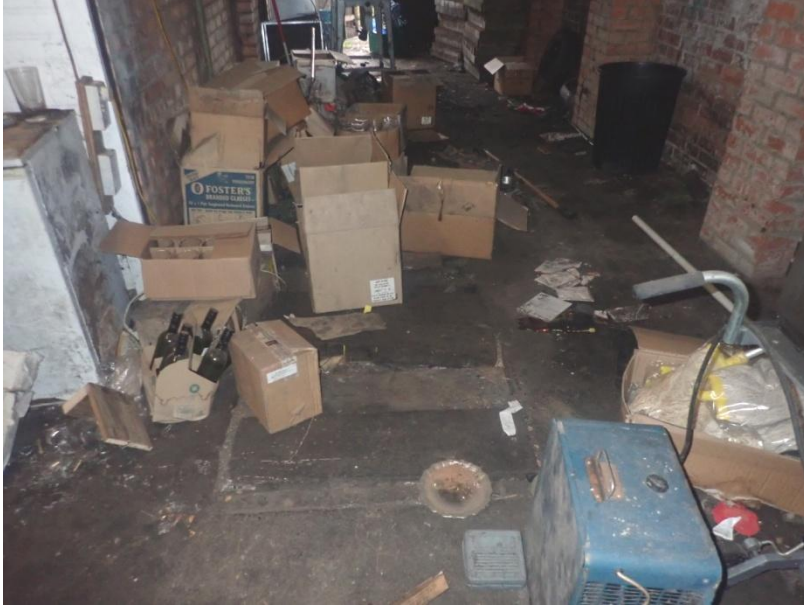
Plate 487 View of the flooring of Cell 25, from the north-west
