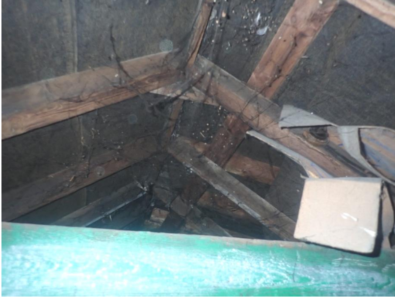
Plate 419: View of the roof supporting structure of Cell 20, from the north-east
