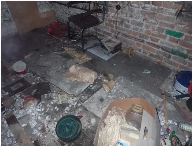
Plate 409: View of the flooring of Cell 20, from the north-west
