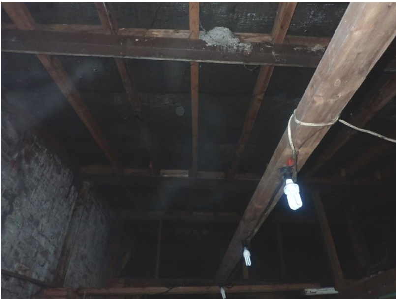
Plate 494: View of the roof supporting structure of Building 6, from the south-west
