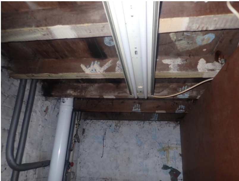
Plate 430: View of the ceiling of Cell 21, from the north-west
