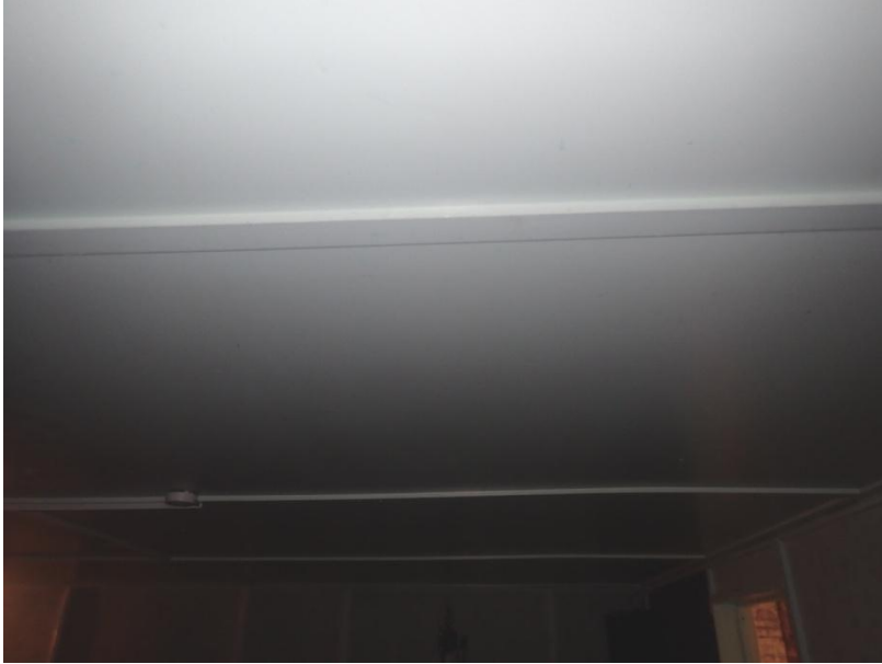
Plate 471: View of the ceiling of Cell 24, from the north-east
