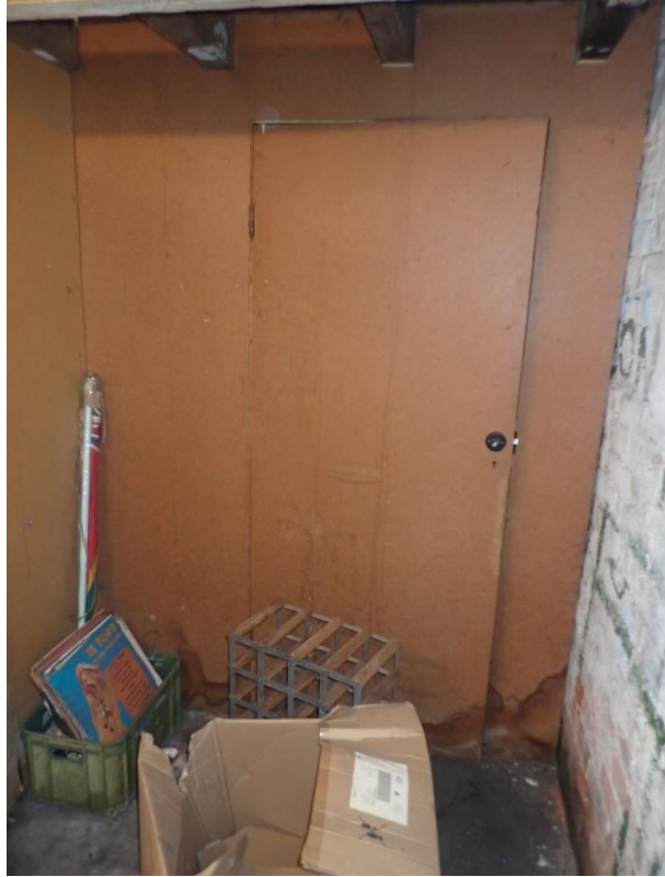
Plate 431: View of the interior of Cell 21, from the north-west
