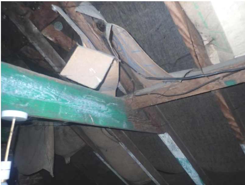
Plate 418: View of the roof supporting structure of Cell 20, from the north-west
