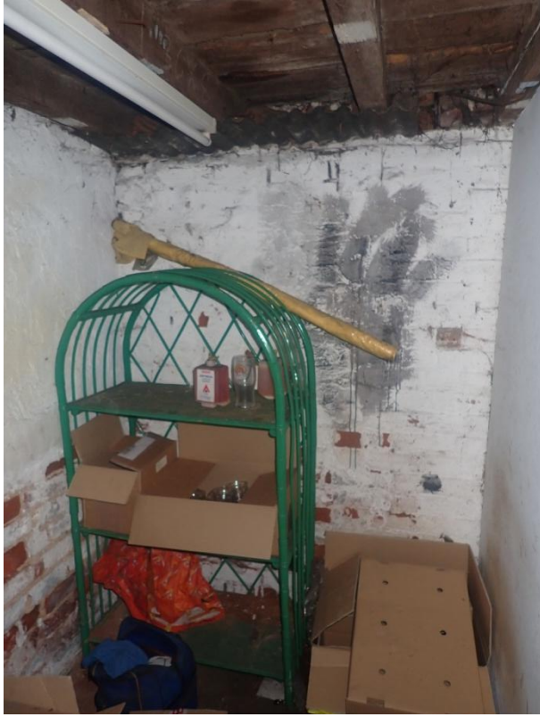
Plate 448: View of the interior of Cell 22, from the north
