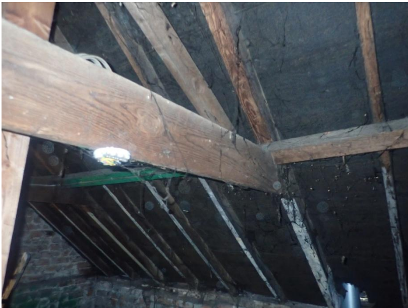
Plate 416: View of the roof supporting structure of Cell 20, from the south-east
