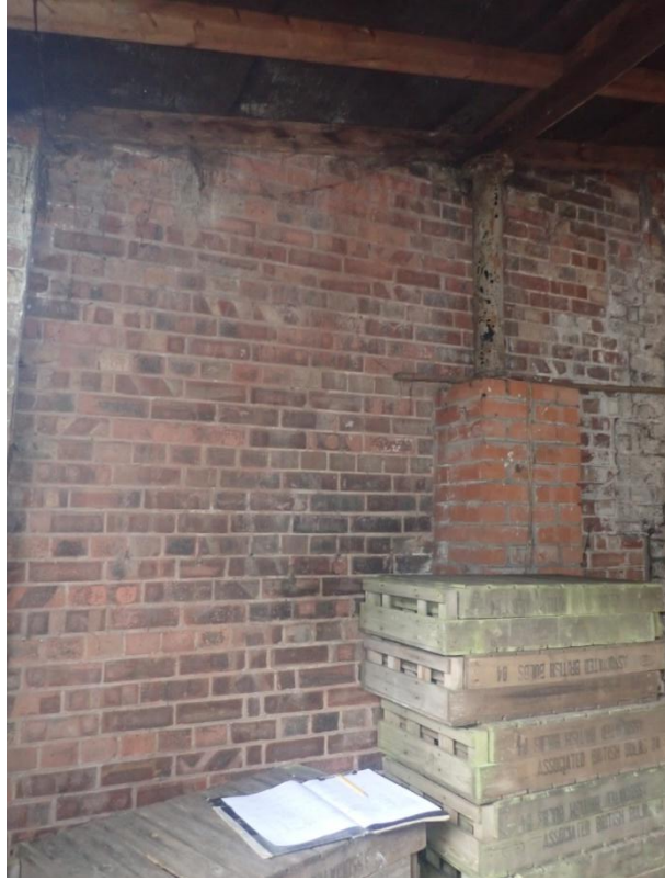
Plate 489: View of the west wall of Cell 25, from the south-east
