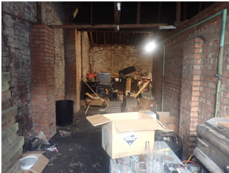
Plate 482: General view of the interior of Cell 25, from the south-east
