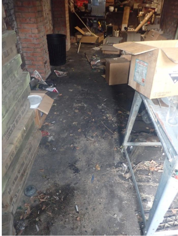
Plate 483: View of the flooring of Cell 25, from the south-east
