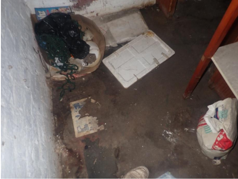
Plate 461: View of the flooring of Cell 23, from the north-east
