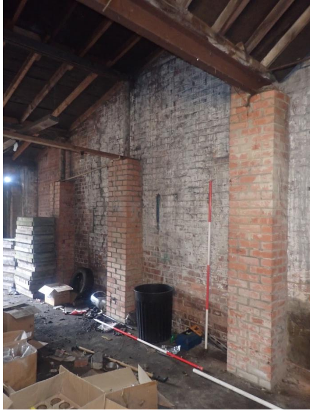
Plate 491: View of the west wall of Cell 25, from the north-east
