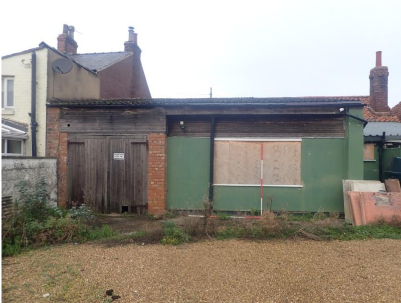
Plate 462: View of the South Elevation of Building 6, from the south-east
