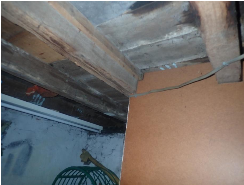
Plate 443: View of the ceiling structure of Cell 22, from the north-west
