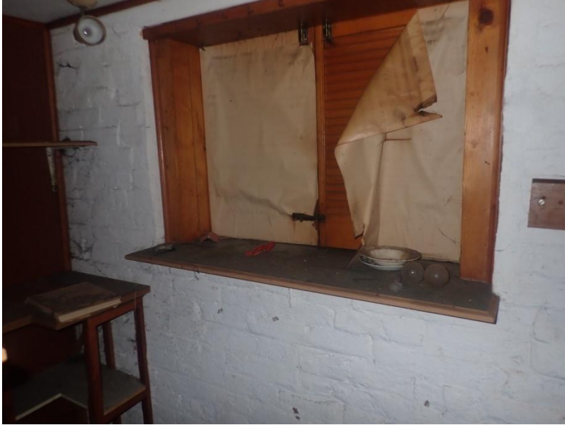
Plate 455: View of the interior of Cell 23, from the north-west
