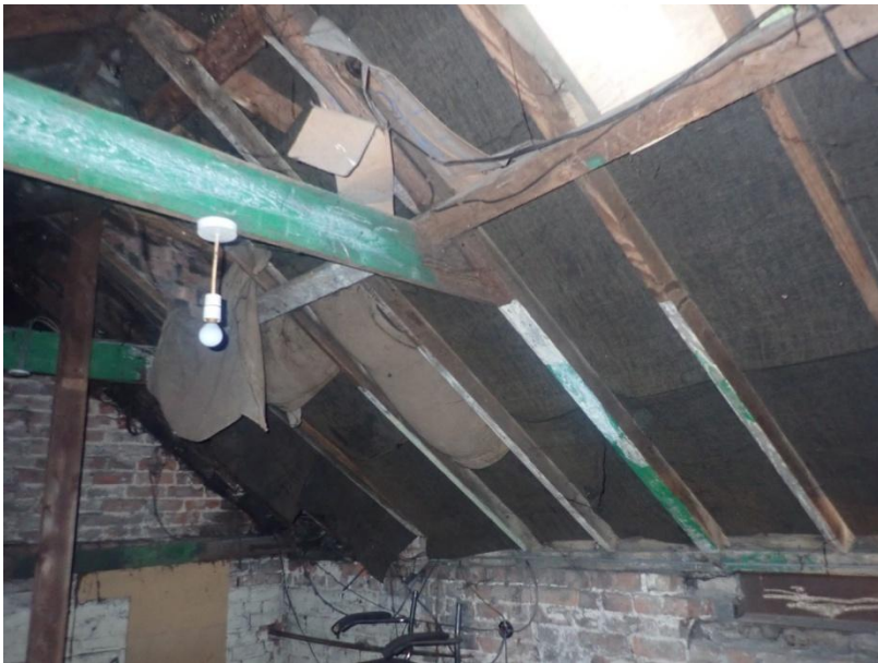
Plate 422: View of the roof supporting structure of Cell 20, from the north-west
