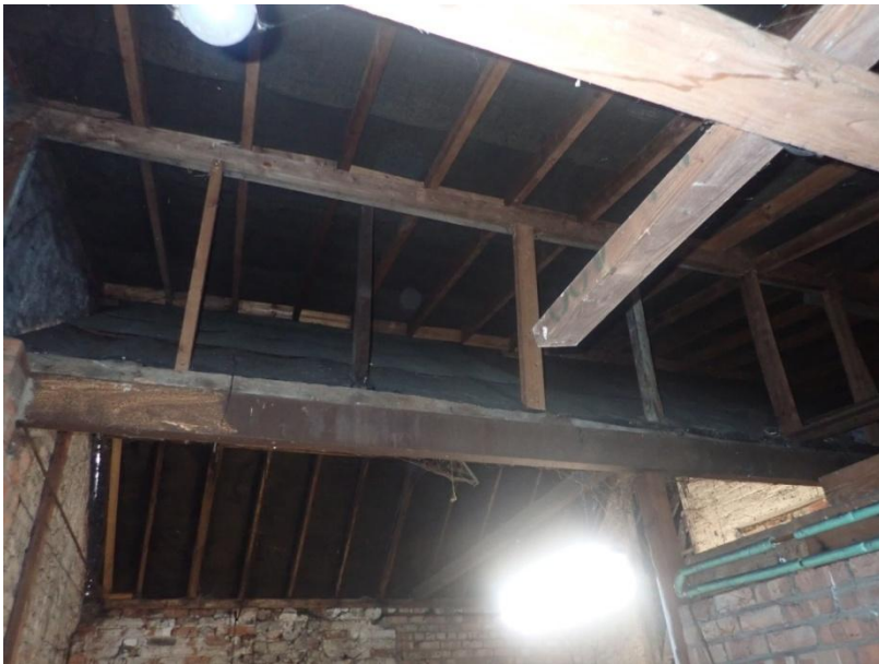
Plate 496: View of the roof supporting structure of Building 6, from the south-west
