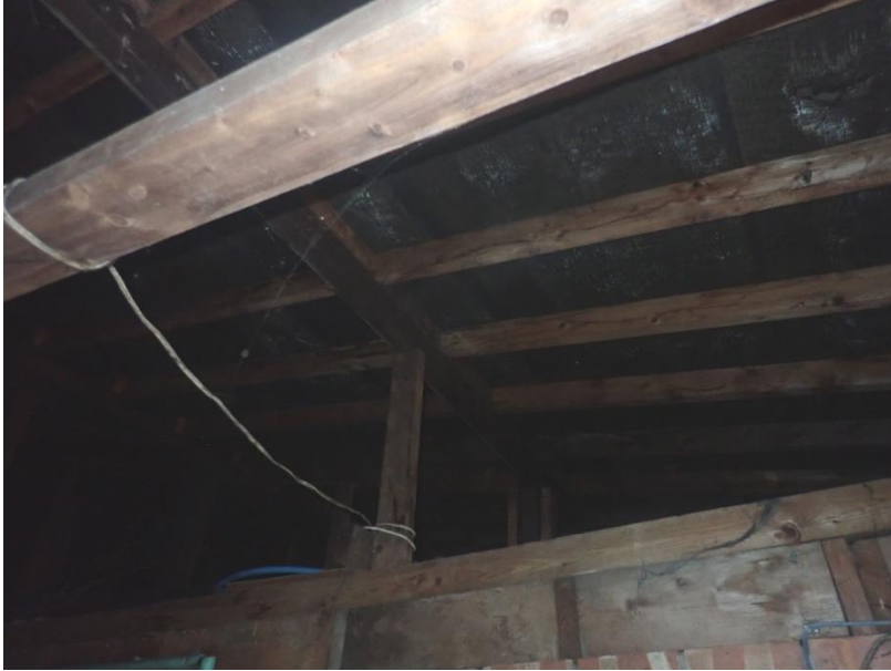
Plate 495: View of the roof supporting structure of Building 6, from the south-west
