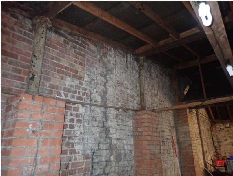
Plate 490: View of the west wall of Cell 25, from the south-east
