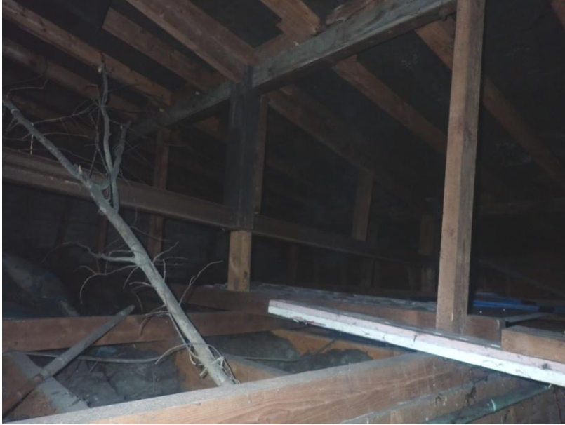
Plate 497: View of the roof supporting structure of Building 6, from the north-west
