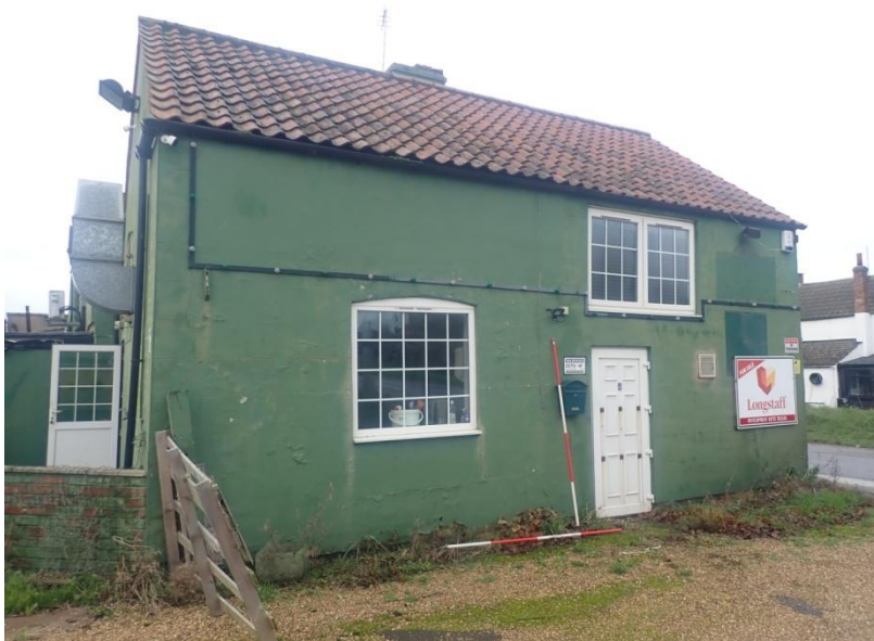
Plate 16: View of the East Elevation of Building 1, from the north-east
