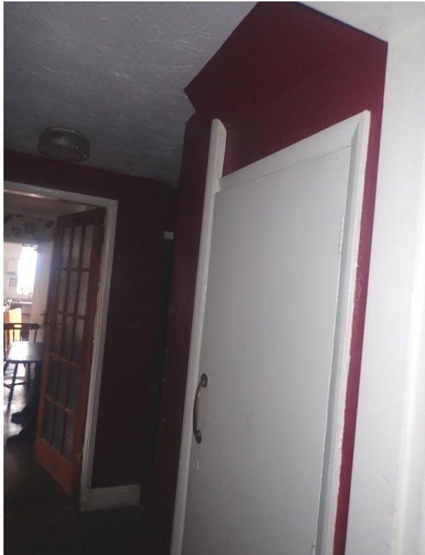
Plate 150: View of the western portion of the south wall of Cell 6, from the south-west
