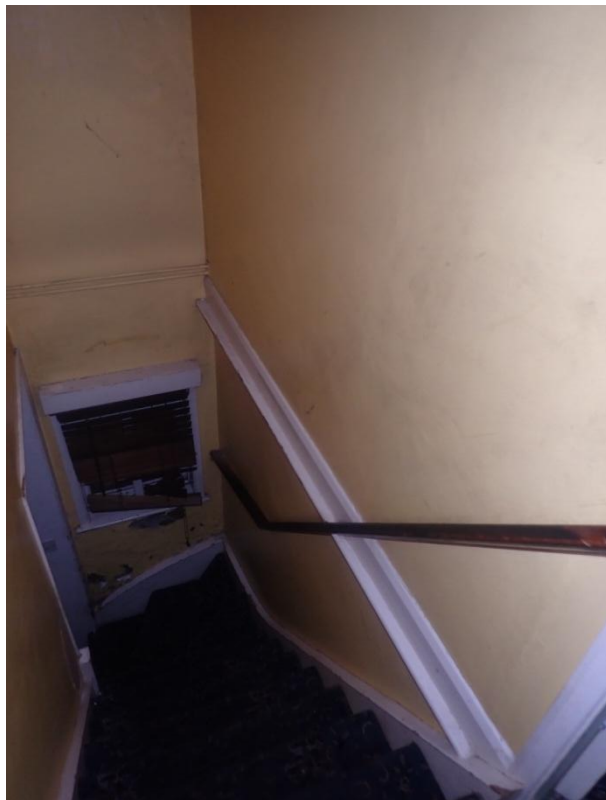
Plate 196: View of the west wall of Cell 10, from the north-west
