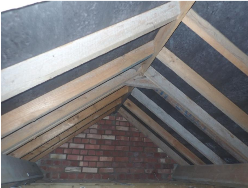
Plate 87: View of the roof supporting structure of Cell 4, from the north-east
