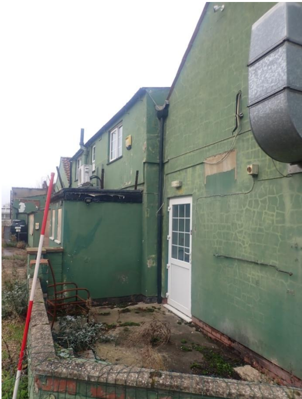
Plate 95: View of the South Elevation of Building 2, from the north-east
