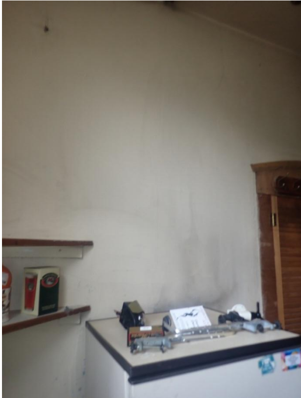
Plate 135: View of the east wall of Cell 6, from the north-west
