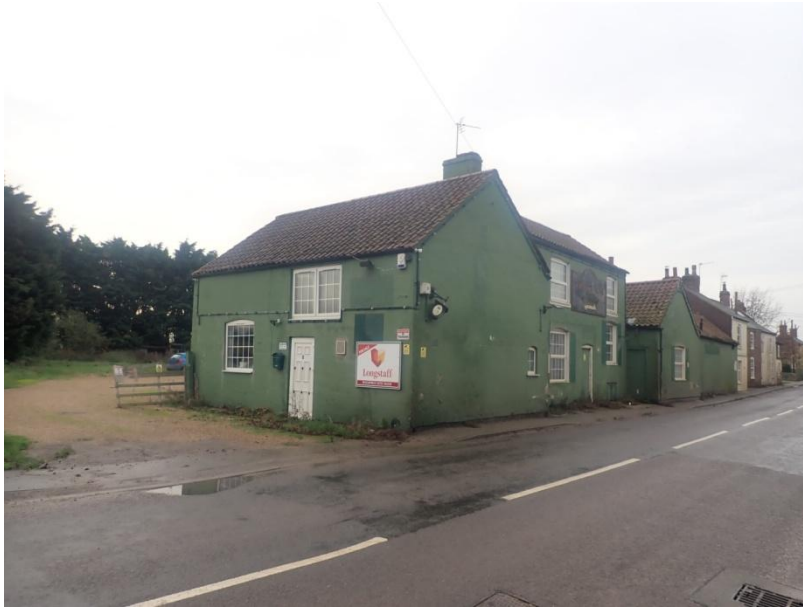
Plate 6: General view of the Duke of York public house complex, from the north-east
