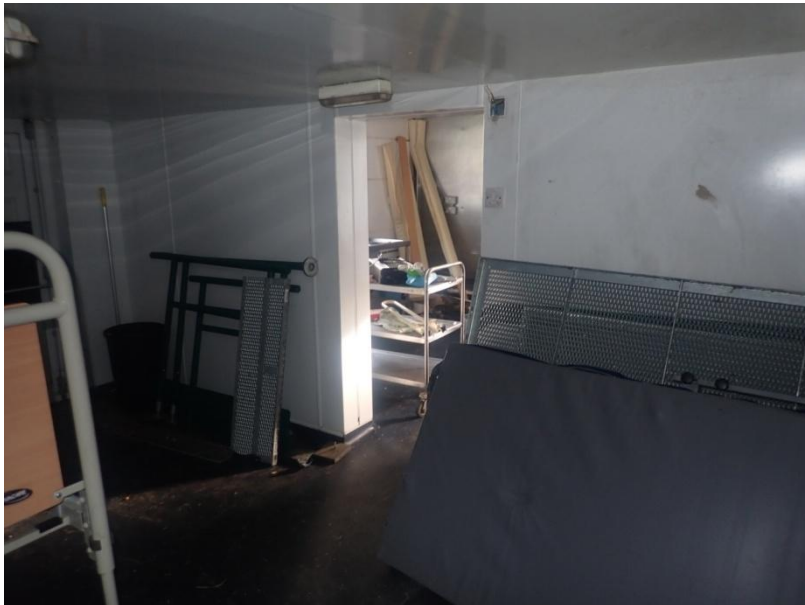
Plate 46: View of the south wall of Cell 2, from the north-west
