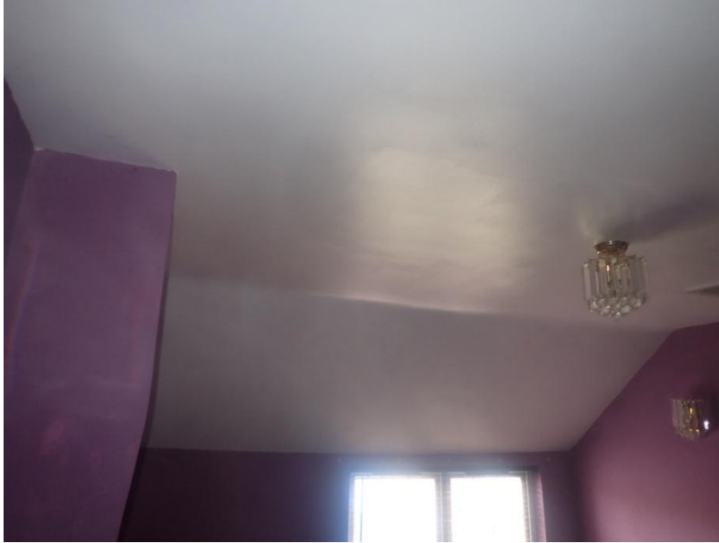
Plate 55: View of the ceiling of Cell 3, from the north-west
