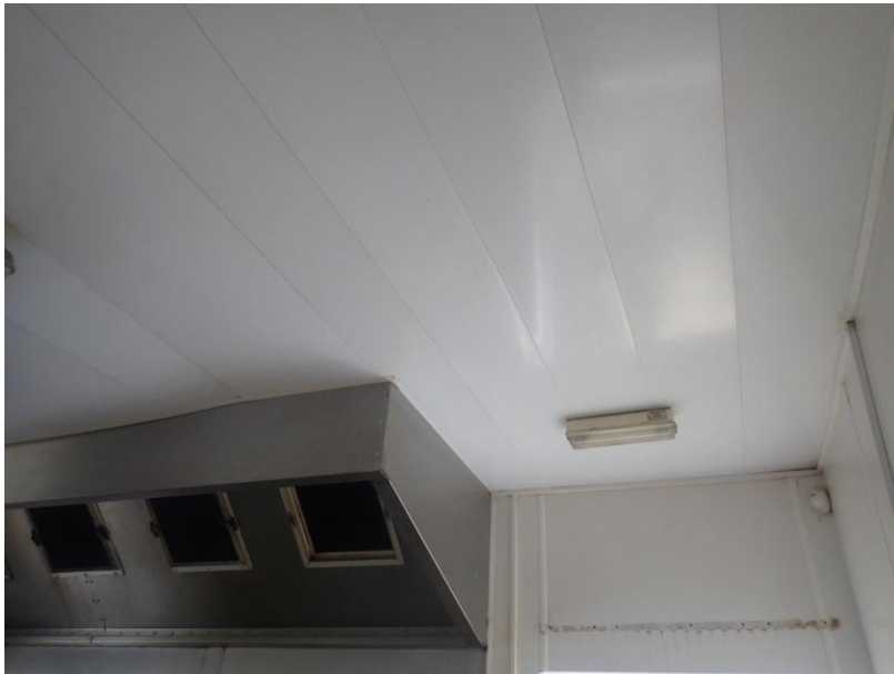
Plate 28: View of the ceiling of Cell 1, from the north
