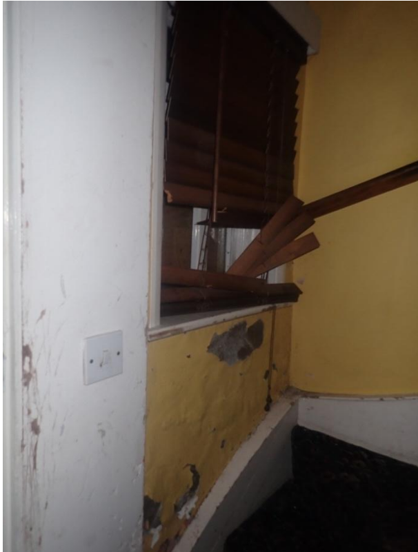
Plate 187: View of the south wall of Cell 10, from the north-east
