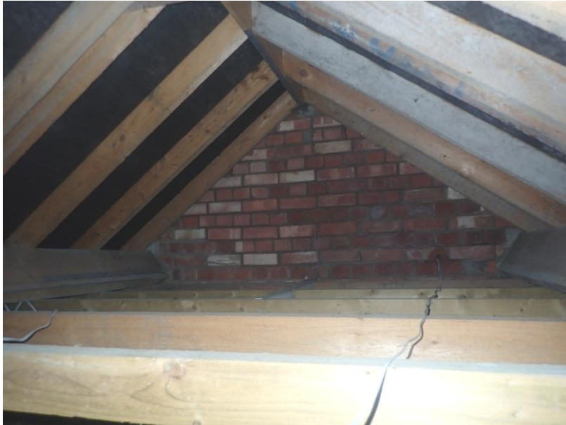
Plate 84: View of the roof supporting structure of Cell 4, from the north-west
