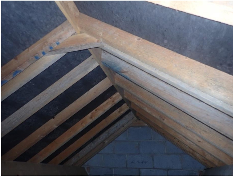
Plate 77: View of the roof supporting structure of Cell 4, from the south-east
