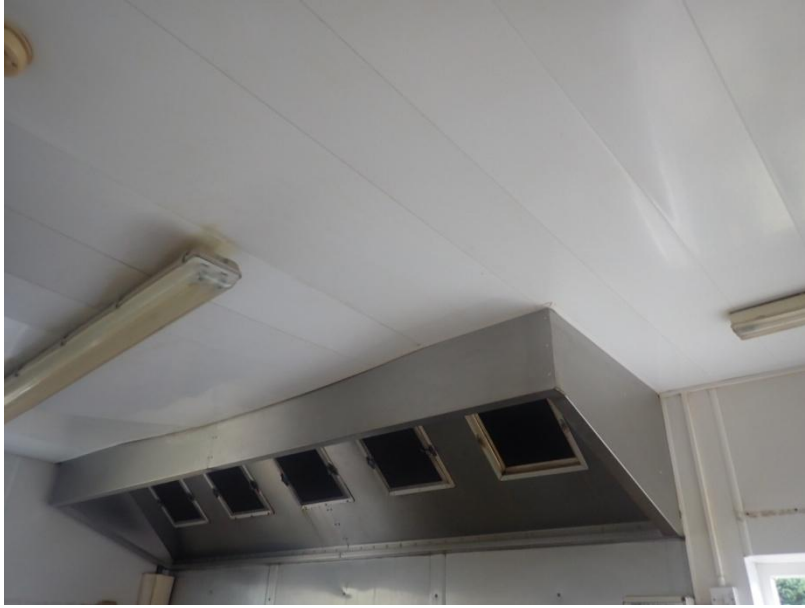
Plate 27: View of the ceiling of Cell 1, from the north-west
