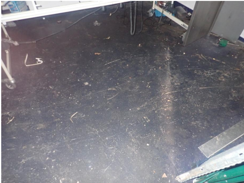
Plate 36: View of the flooring of Cell 1, from the south-west
