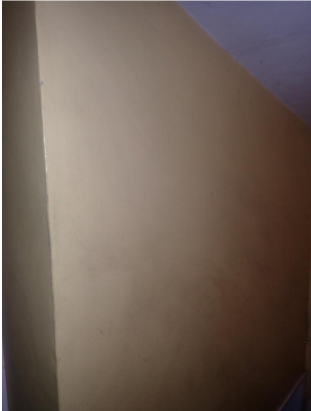
Plate 195: View of the east wall of Cell 10, from the north-west
