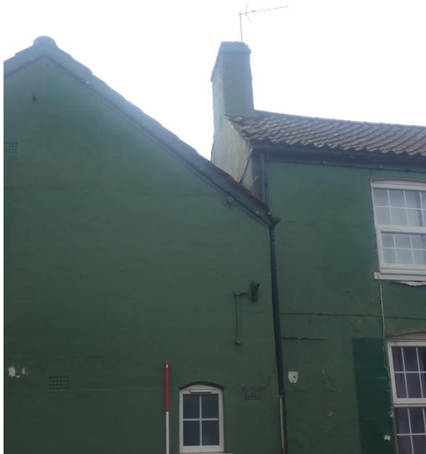
Plate 96: View of the North Elevation of Building 2, from the north-west
