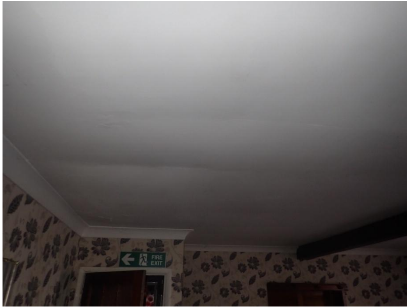
Plate 163: View of the ceiling of Cell 8, from the north-east
