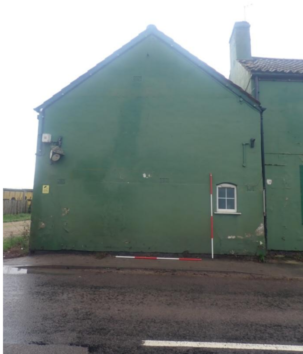
Plate 18: View of the North Elevation of Building 1, from the north-west
