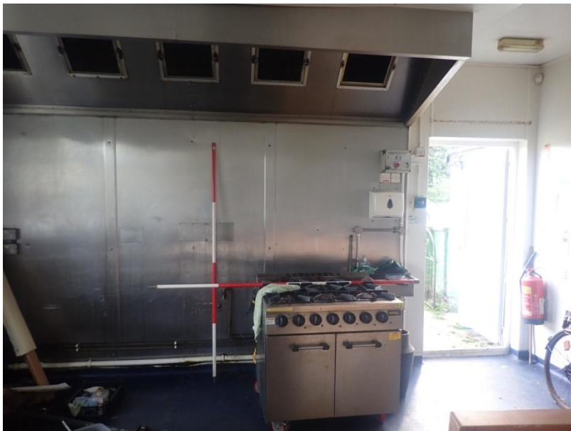
Plate 34: View of the south wall of Cell 1, from the north-west
