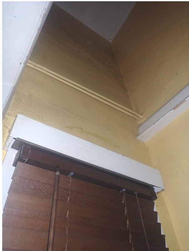
Plate 188: View of the south wall of Cell 10, from the north-east
