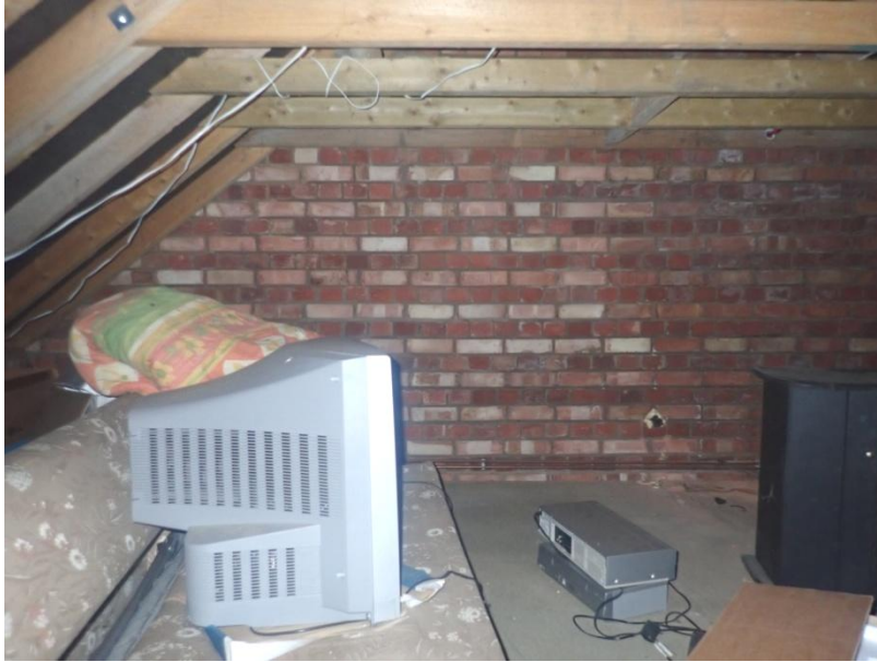
Plate 71: View of the south wall of Cell 4, from the north-east
