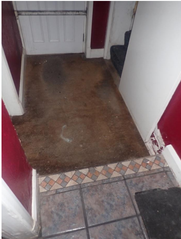
Plate 141: View of the flooring of Cell 7, from the north-east
