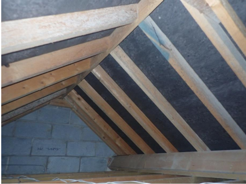
Plate 75: View of the roof supporting structure of Cell 4, from the south-west
