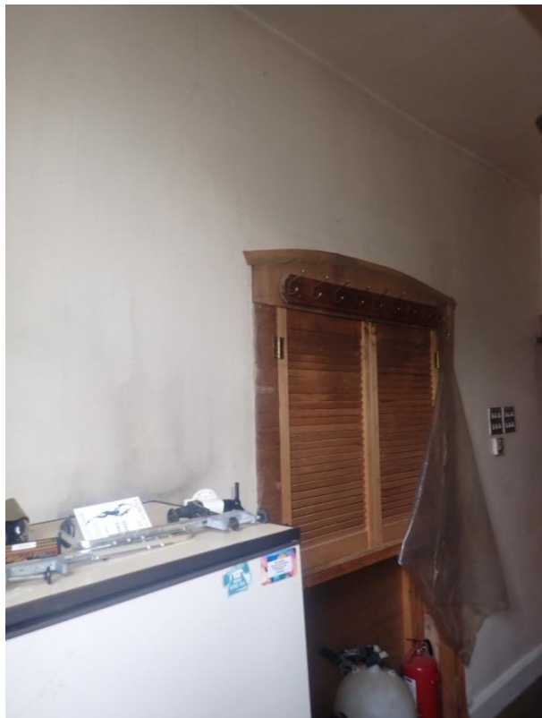
Plate 134: View of the east wall of Cell 6, from the north-west
