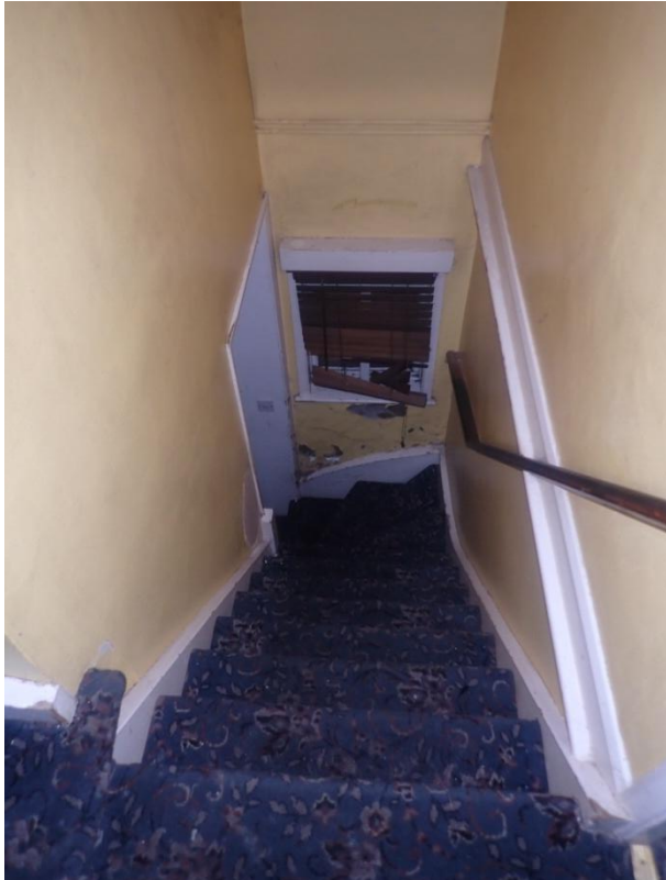
Plate 191: View of the stairwell of Cell 10, from the north-west
