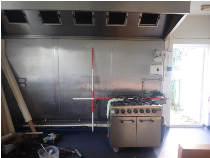
Plate 32: View of the south wall of Cell 1, from the north-west
