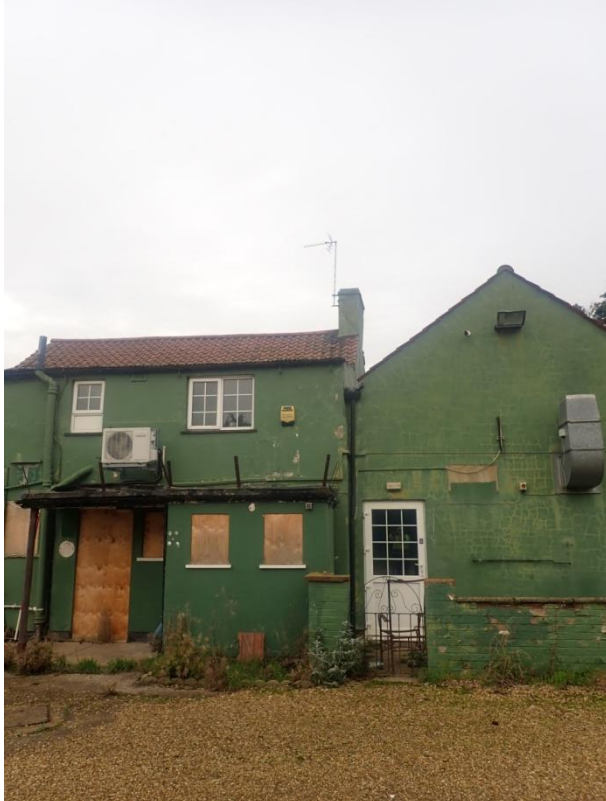
Plate 94: View of the South Elevation of Building 2, from the south-east
