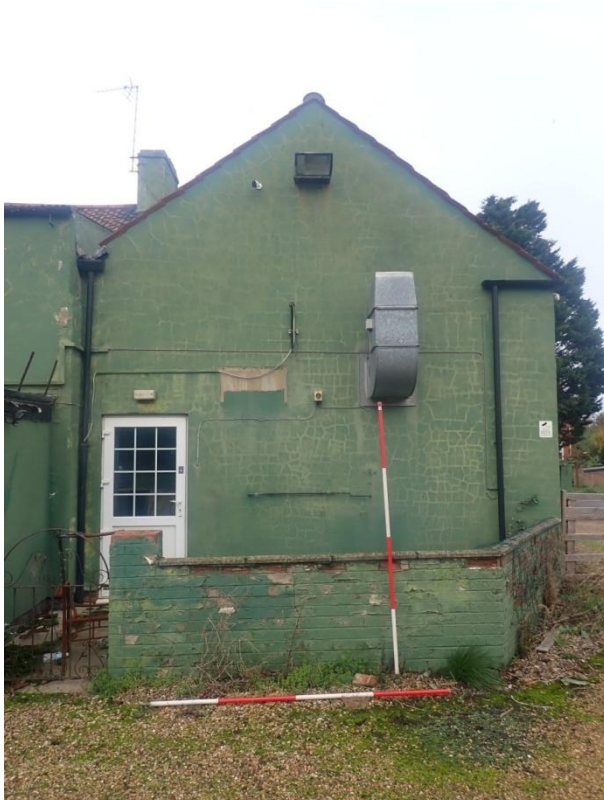
Plate 11: View of the South Elevation of Building 1, from the south-east
