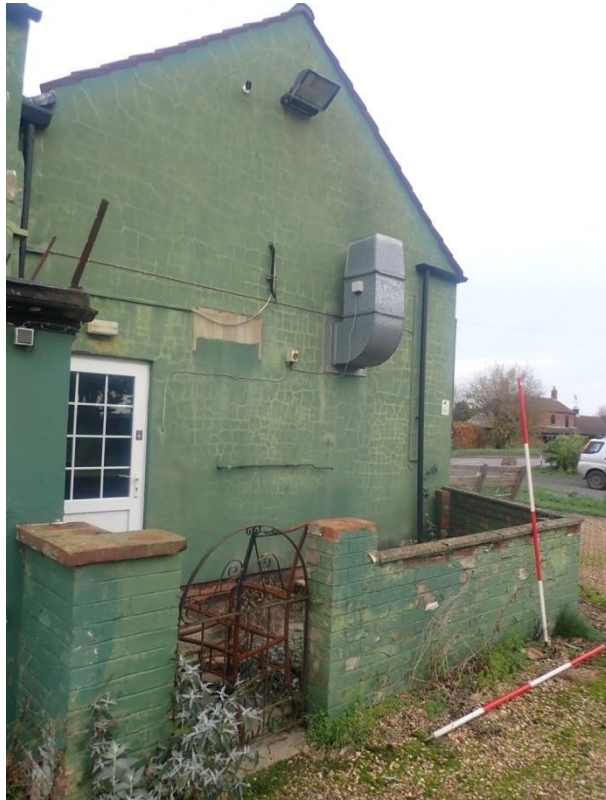
Plate 12: View of the South Elevation of Building 1, from the south-west
