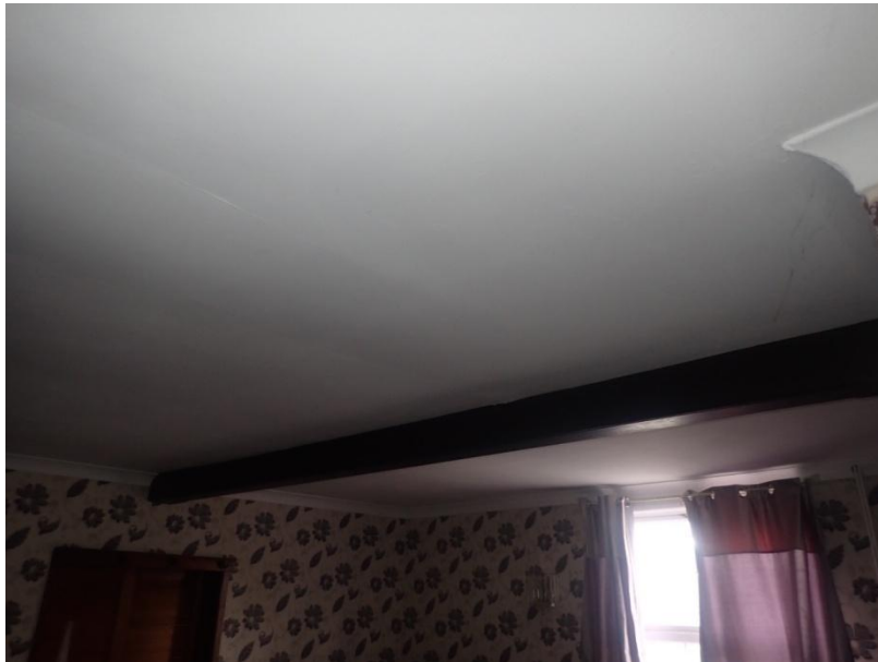
Plate 164: View of the ceiling of Cell 8, from the south-east
