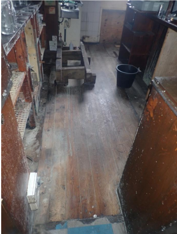
Plate 111: View of the flooring of Cell 6, from the south-east
