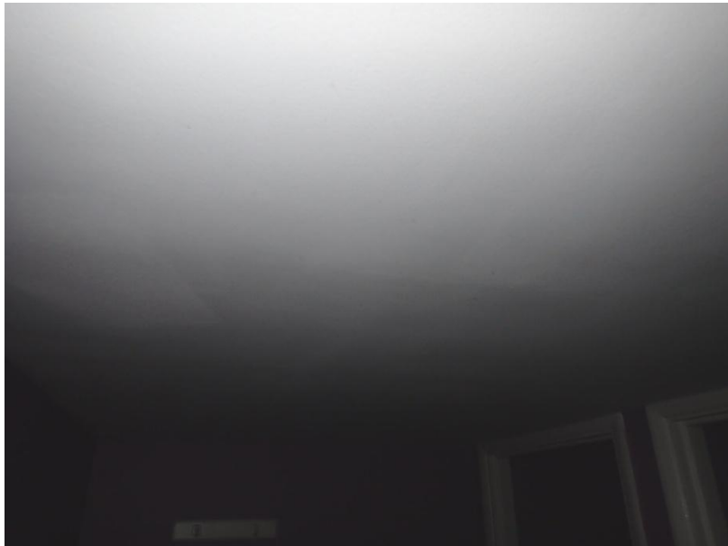
Plate 172: View of the ceiling of Cell 9, from the south-west
