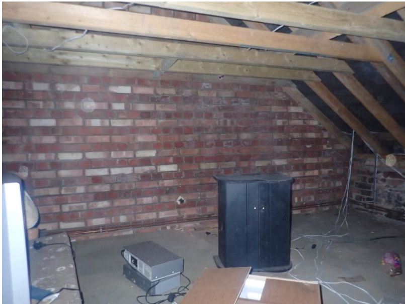
Plate 70: View of the south wall of Cell 4, from the north-east
