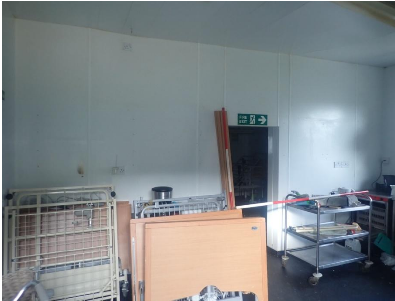
Plate 31: View of the north wall of Cell 1, from the south-west
