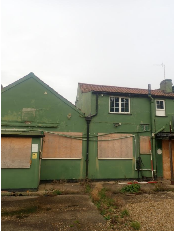
Plate 93: View of the South Elevation of Building 2, from the south-west
