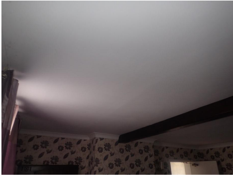
Plate 159: View of the ceiling of Cell 8, from the north-west
