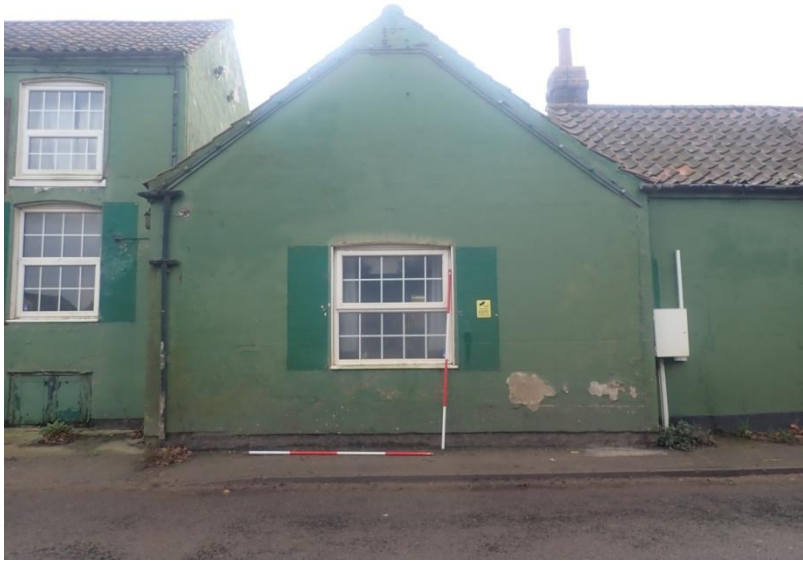
Plate 100: View of the West Elevation of Building 2, from the north-west
