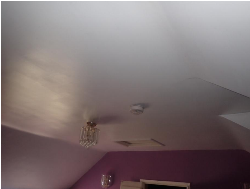
Plate 56: View of the ceiling of Cell 3, from the north-west
