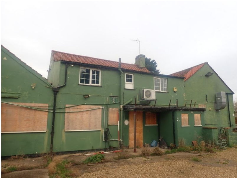
Plate 90: View of the South Elevation of Building 2, from the south-west
