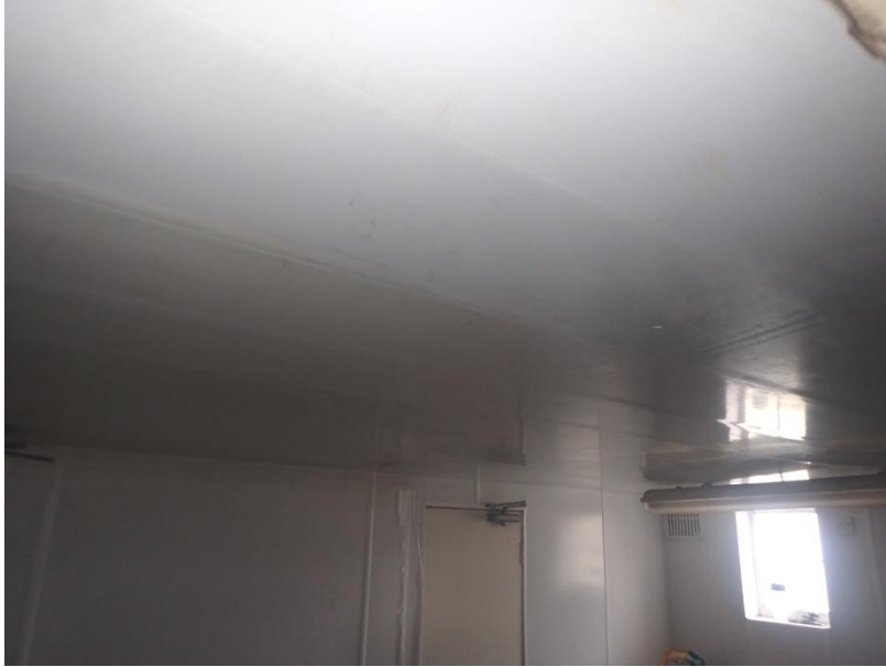
Plate 39: View of the ceiling of Cell 2, from the south-east
