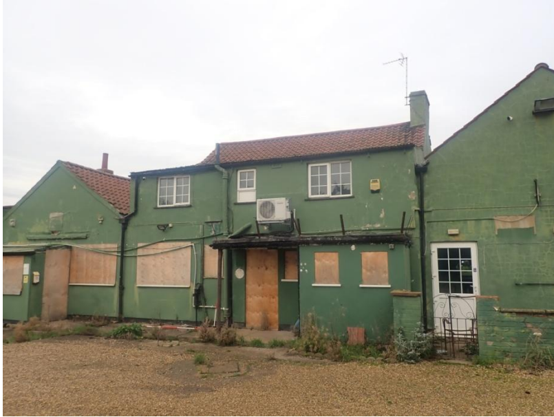
Plate 91: View of the South Elevation of Building 2, from the south-east
