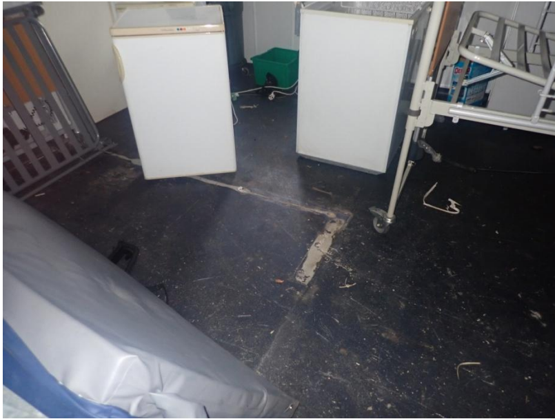
Plate 35: View of the flooring of Cell 1, from the south-east
