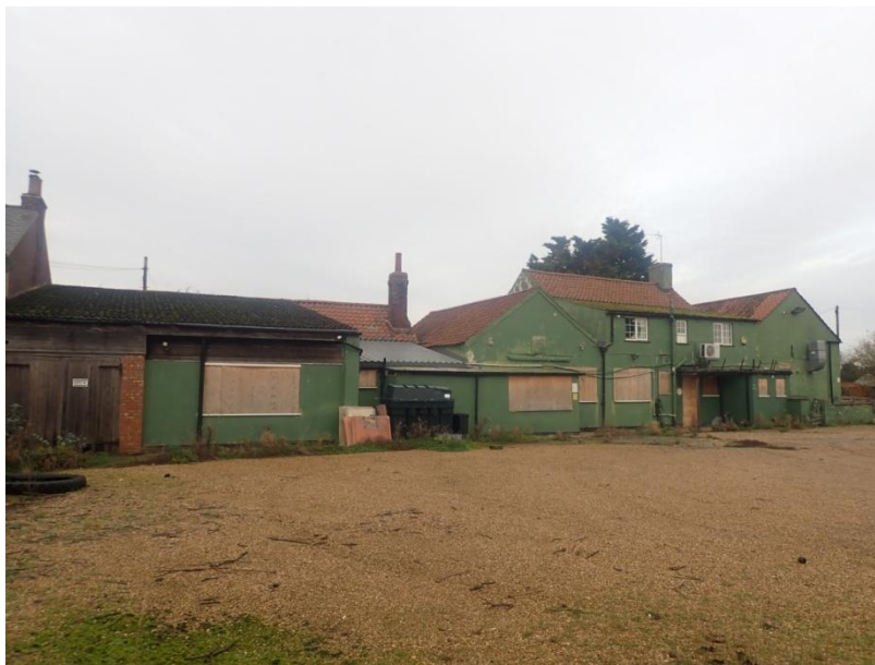
Plate 1: General view of the Duke of York public house complex, from the south-west
