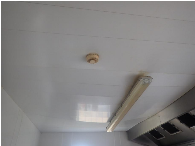
Plate 26: View of the ceiling of Cell 1, from the south-west
