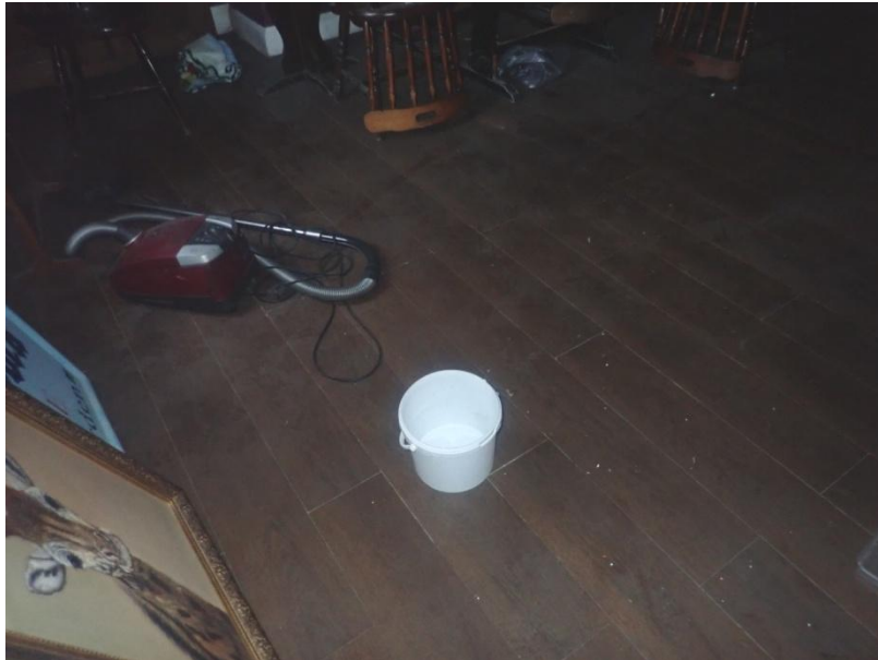
Plate 155: View of the flooring of Cell 8, from the south
