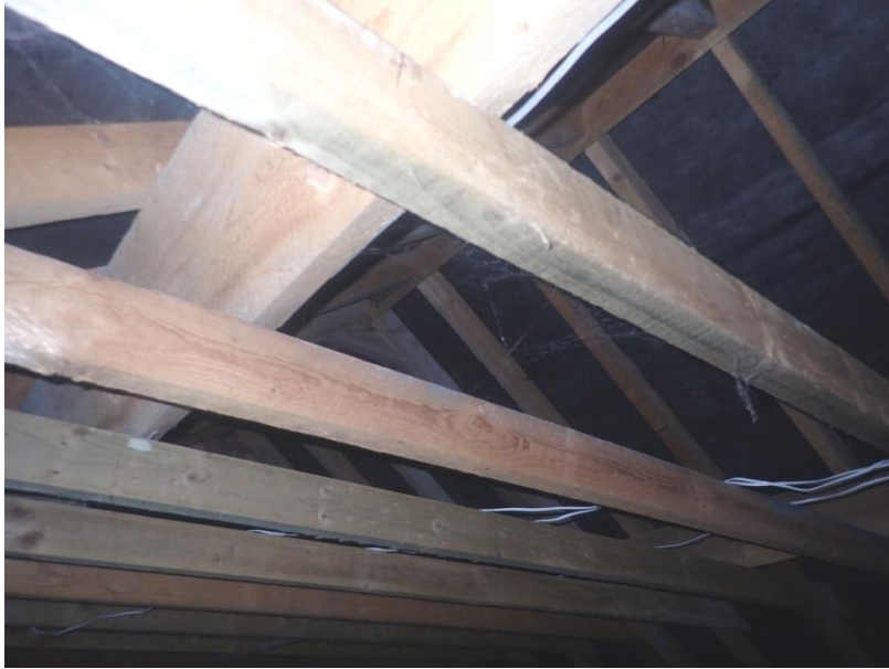
Plate 69: View of the roof supporting structure of Cell 4, from the north
