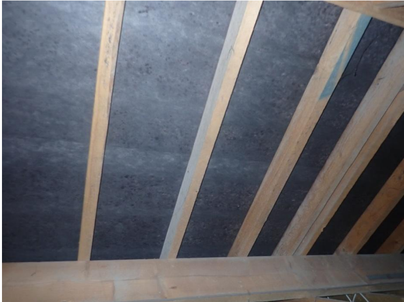
Plate 86: View of the roof supporting structure of Cell 4, from the west
