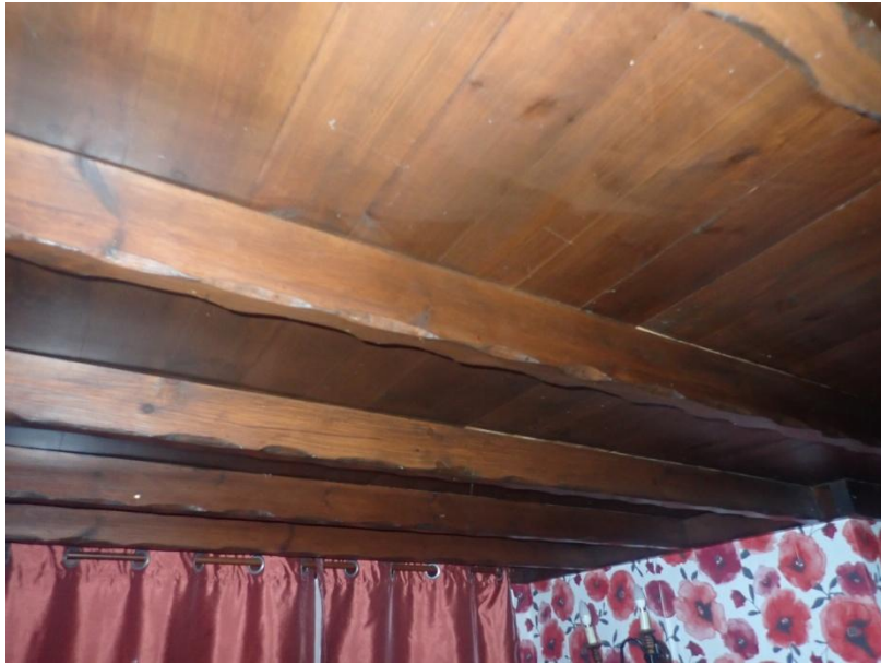
Plate 106: View of the ceiling of Cell 5, from the north-west
