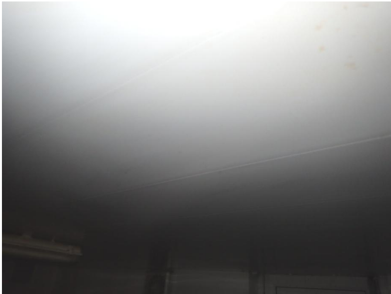
Plate 40: View of the ceiling of Cell 2, from the south-west
