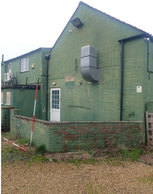
Plate 13: View of the South Elevation of Building 1, from the south-east
