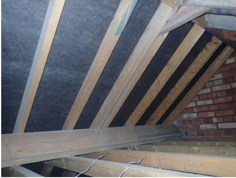
Plate 85: View of the roof supporting structure of Cell 4, from the north-west
