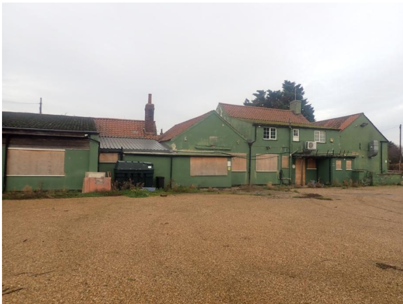
Plate 3: General view of the Duke of York public house complex, from the south-west
