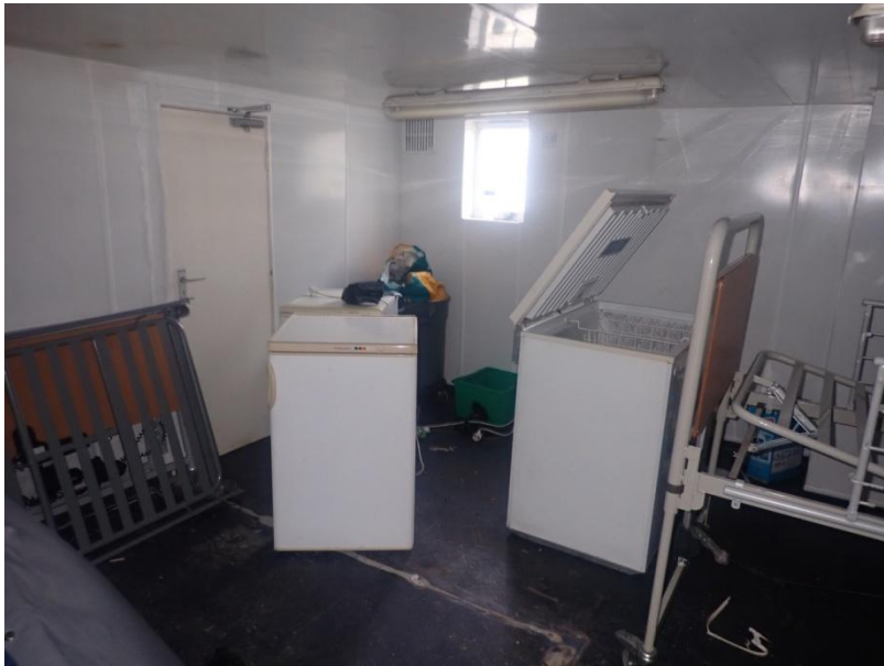
Plate 38: General view of the interior of Cell 2, from the south-east
