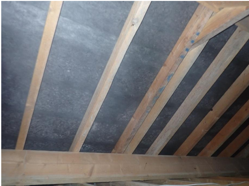
Plate 78: View of the roof supporting structure of Cell 4, from the south-east
