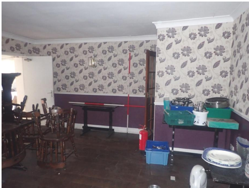
Plate 166: View of the south wall of Cell 8, from the north-west
