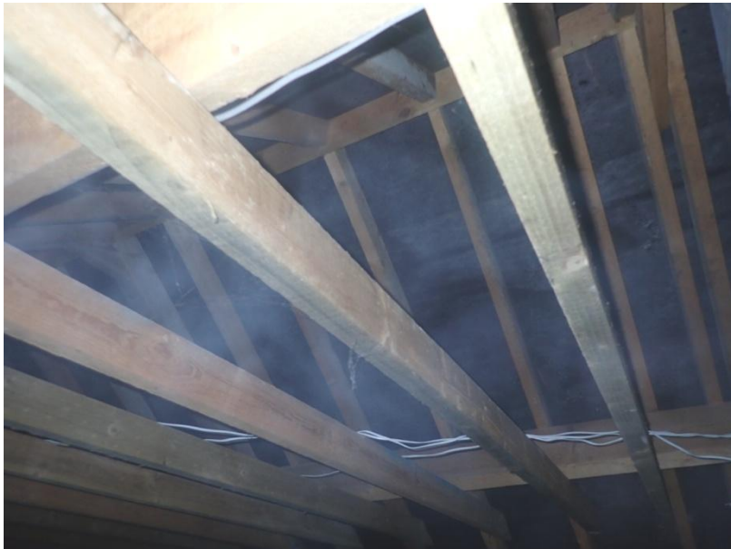
Plate 68: View of the roof supporting structure of Cell 4, from the north-east
