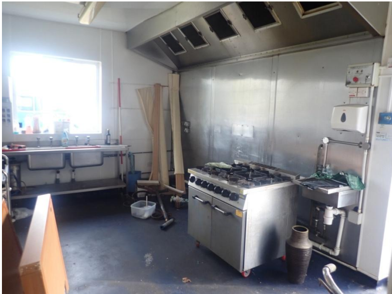
Plate 20: General view of the interior of Cell 1, from the north-west
