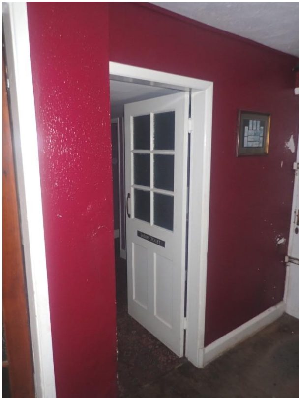
Plate 153: View of the east wall of Cell 7, from the north-west
