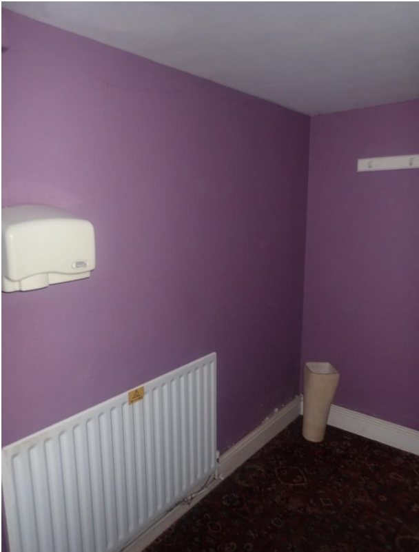
Plate 177: View of the north wall of Cell 9, from the south-west
