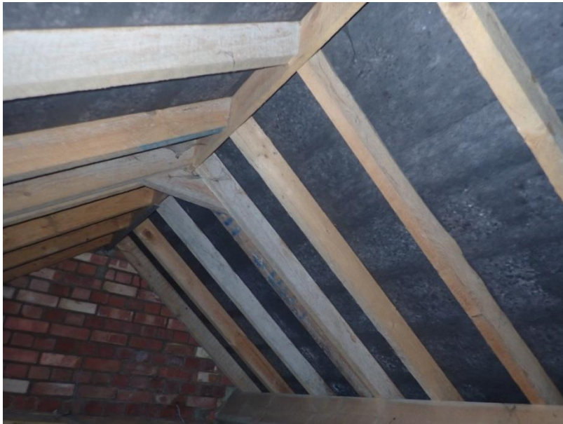
Plate 88: View of the roof supporting structure of Cell 4, from the north-east
