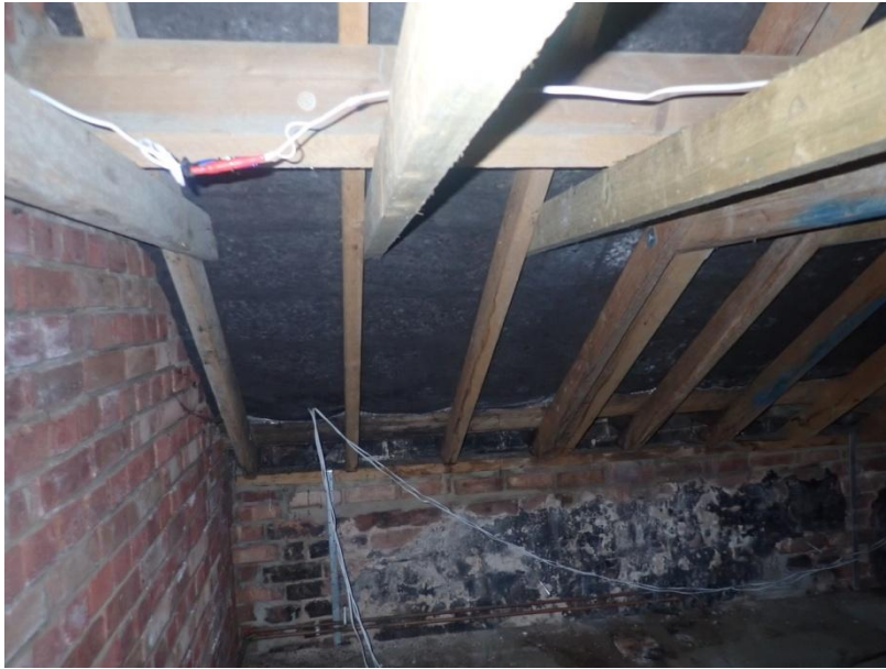
Plate 81: View of the west wall of Cell 4, from the east
