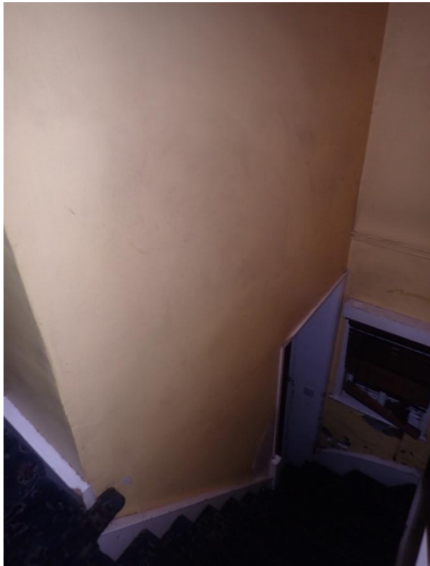
Plate 194: View of the east wall of Cell 10, from the north-west
