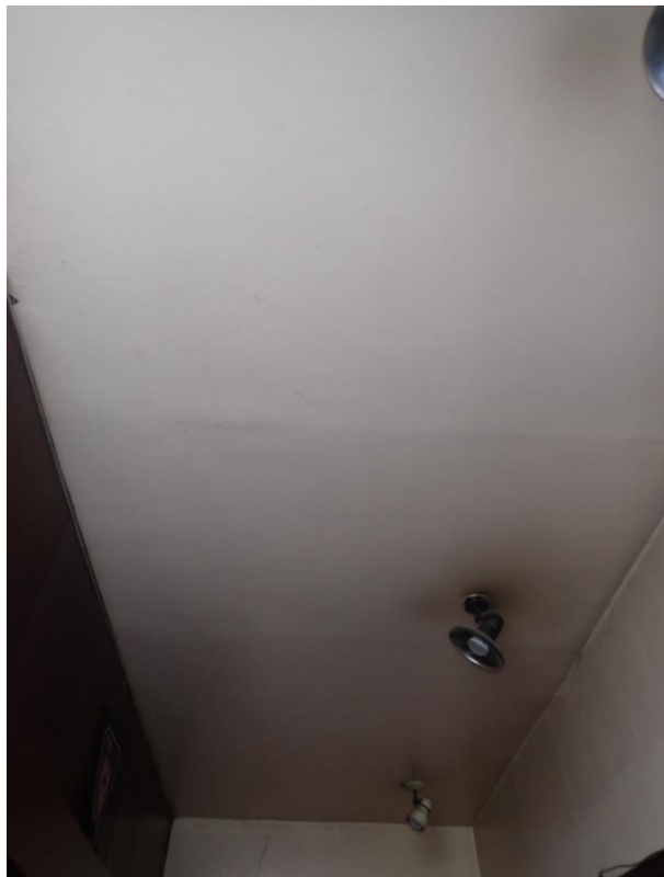
Plate 114: View of the ceiling of Cell 6, from the north-west
