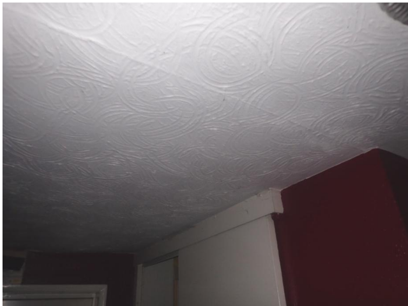
Plate 145: View of the ceiling of Cell 7, from the north
