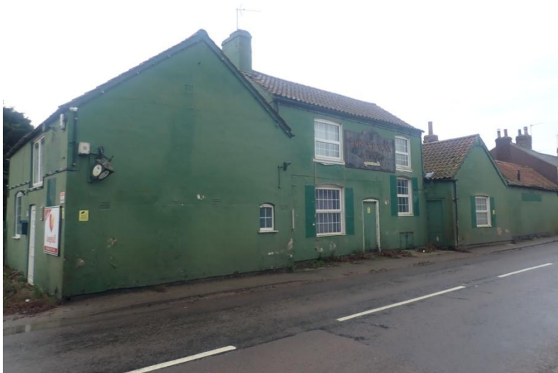
Plate 7: General view of the Duke of York public house complex, from the north-east
