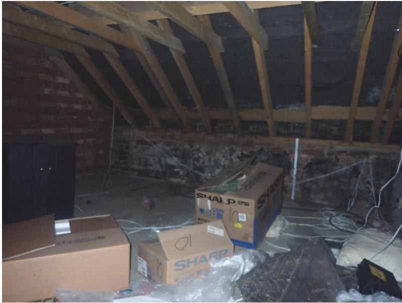
Plate 67: View of the roof supporting structure of Cell 4, from the north-east
