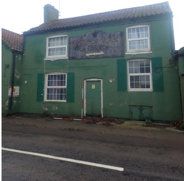
Plate 98: View of the North Elevation of Building 2, from the north-west
