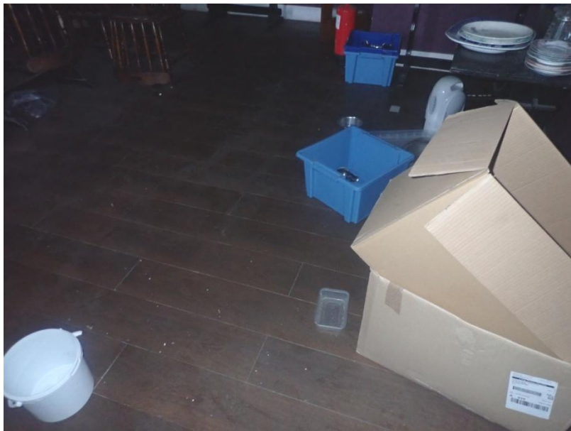
Plate 156: View of the flooring of Cell 8, from the south-west
