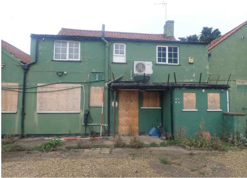
Plate 89: View of the South Elevation of Building 2, from the south-west
