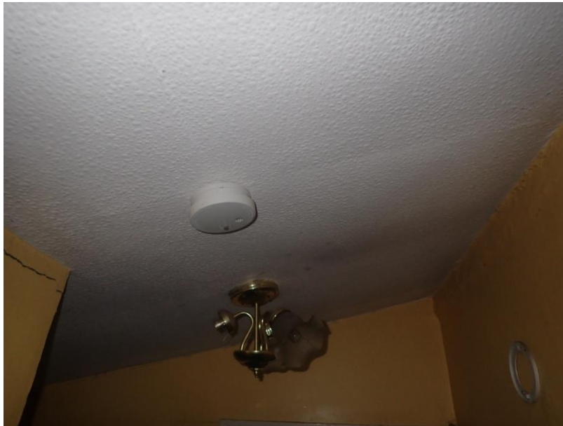
Plate 200: View of the ceiling of Cell 10, from the north-east
