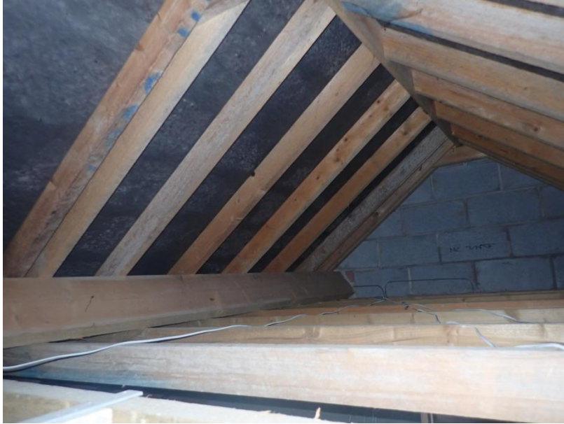
Plate 79: View of the roof supporting structure of Cell 4, from the south-east
