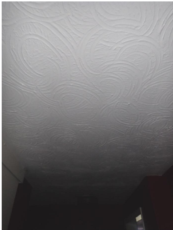
Plate 143: View of the ceiling of Cell 7, from the south-east
