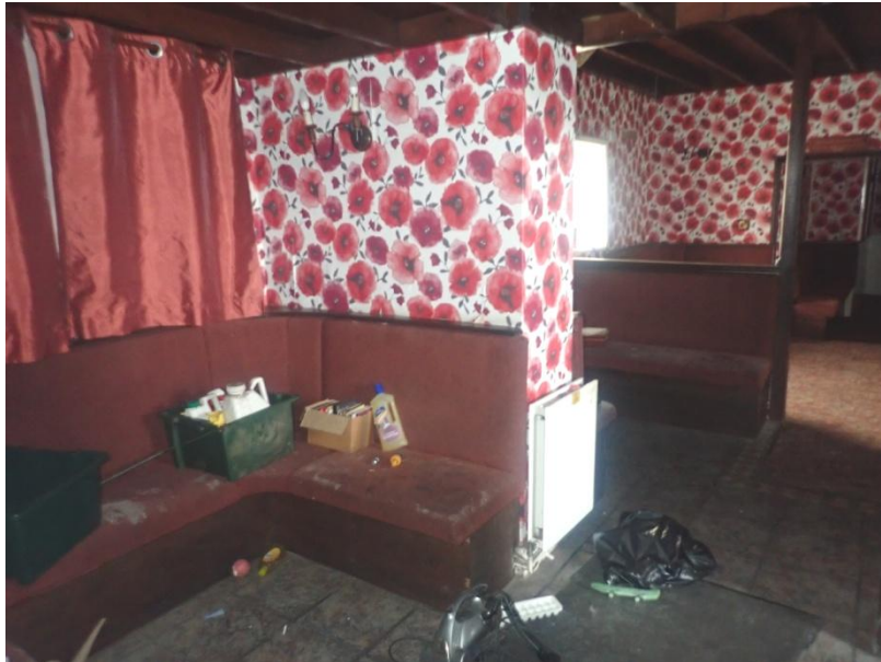
Plate 104: General view of the interior of Cell 5, from the north-east
