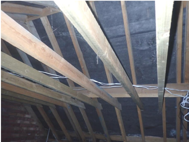
Plate 66: View of the roof supporting structure of Cell 4, from the north-east
