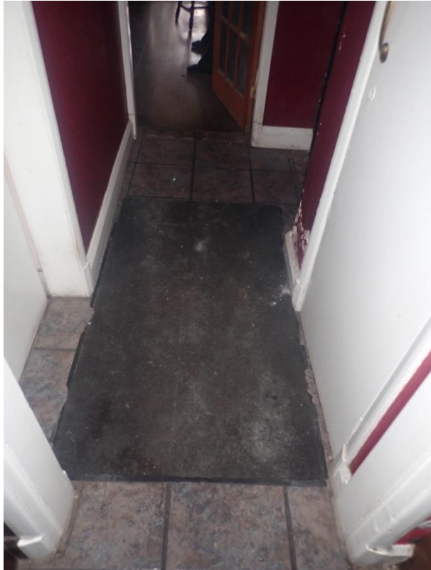
Plate 139: View of the flooring of Cell 7, from the south-west
