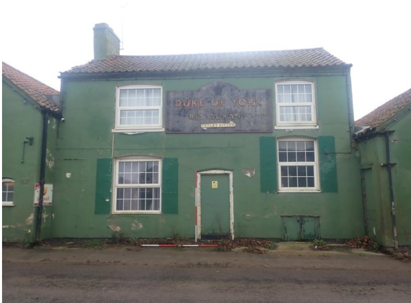
Plate 97: View of the North Elevation of Building 2, from the north-west
