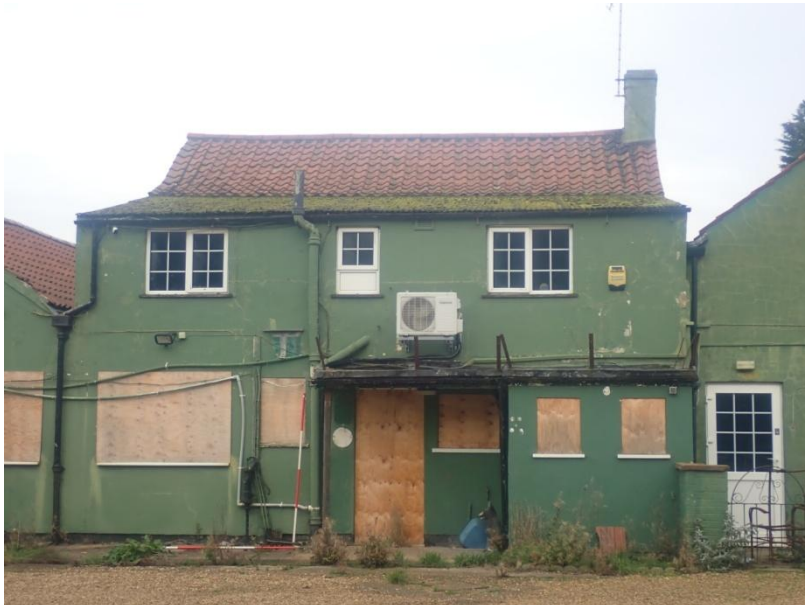
Plate 92: View of the South Elevation of Building 2, from the south-west
