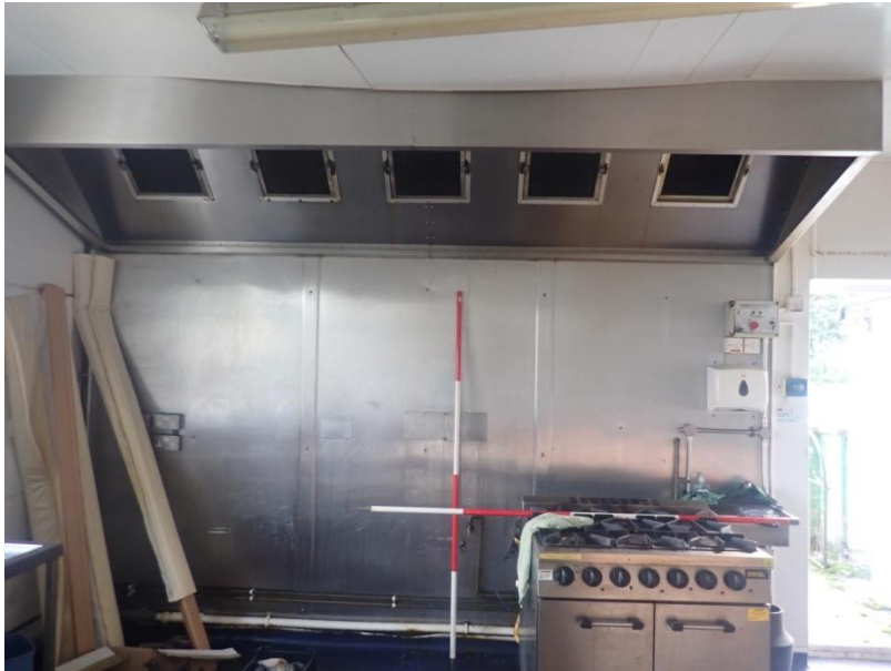
Plate 33: View of the south wall of Cell 1, from the north-west
