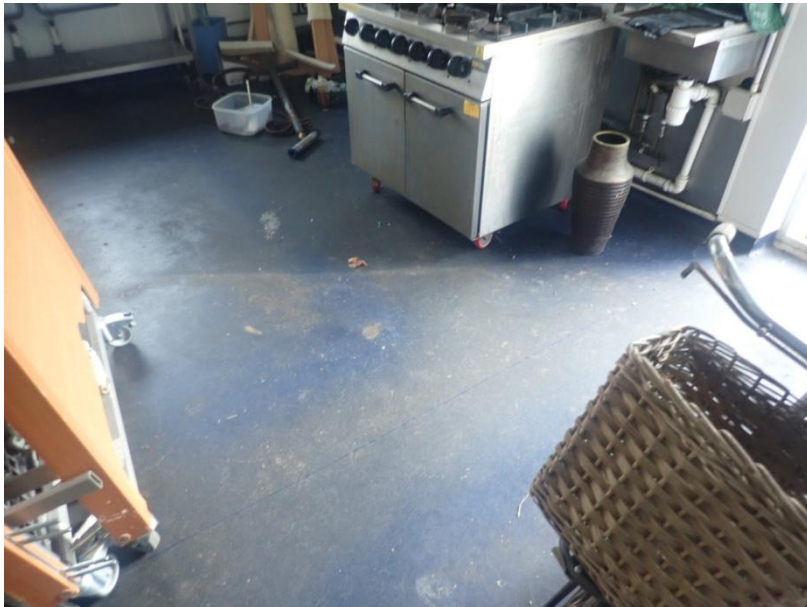
Plate 22: View of the flooring of Cell 1, from the south-west
