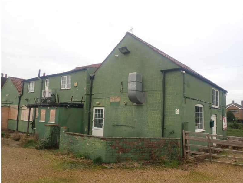
Plate 5: General view of the Duke of York public house complex, from the south-east
