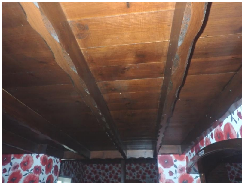
Plate 105: View of the ceiling of Cell 5, from the north-east
