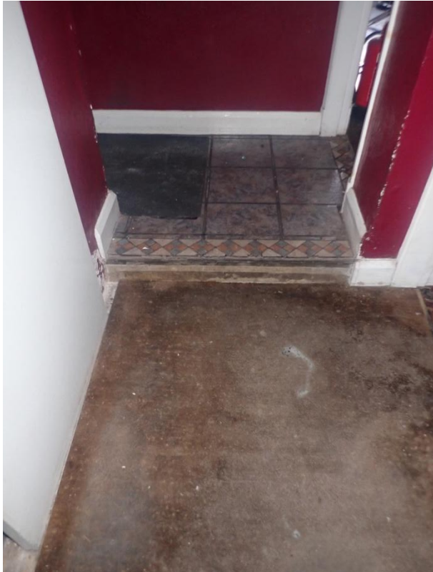
Plate 142: View of the flooring of Cell 7, from the south-east
