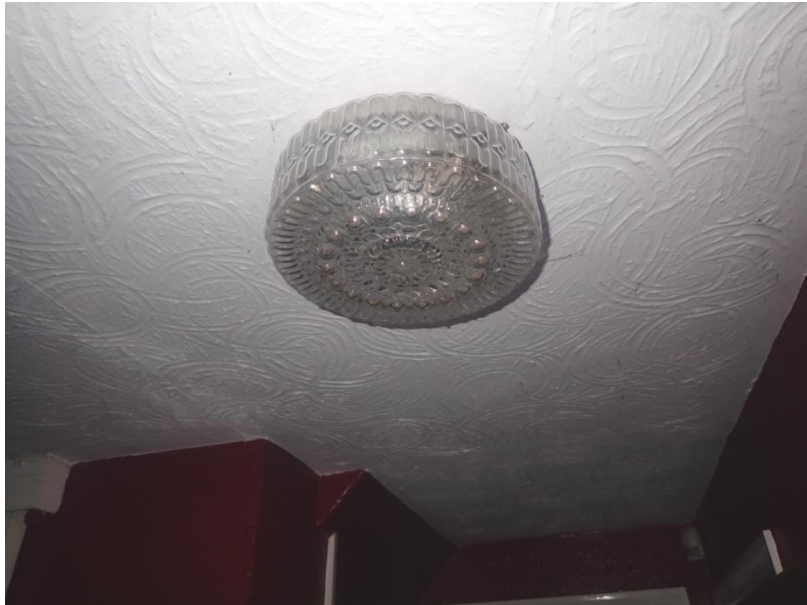
Plate 144: View of the ceiling of Cell 7, from the north-east
