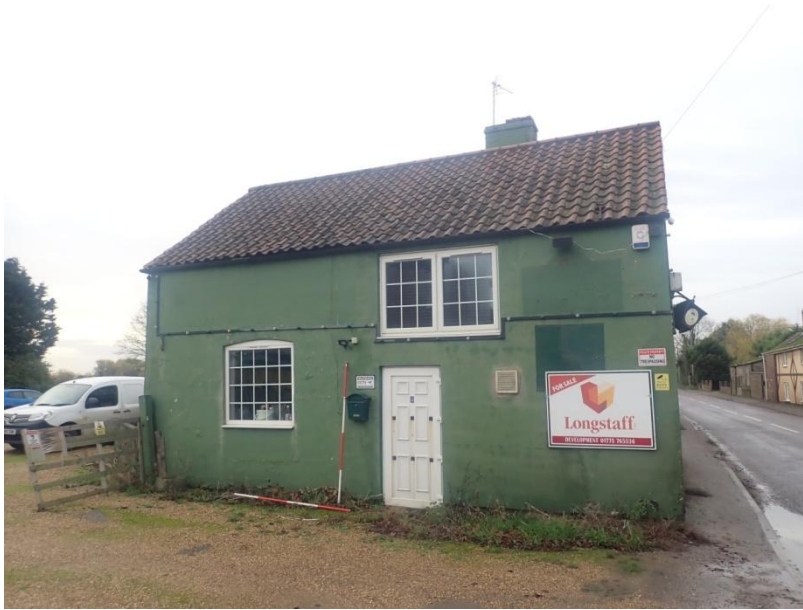
Plate 17: View of the East Elevation of Building 1, from the north-east
