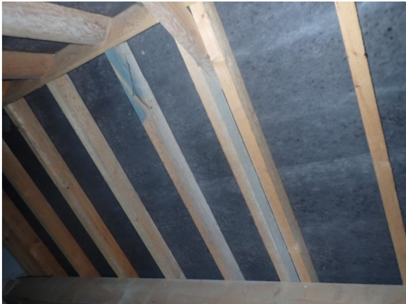
Plate 76: View of the roof supporting structure of Cell 4, from the south-west
