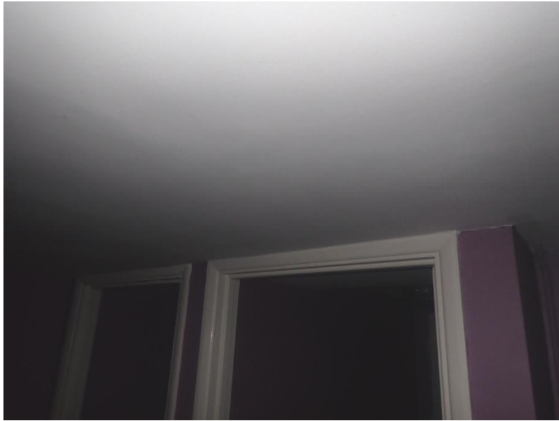
Plate 173: View of the ceiling of Cell 9, from the north-west
