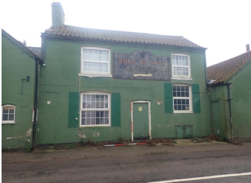
Plate 99: View of the North Elevation of Building 2, from the north-west
