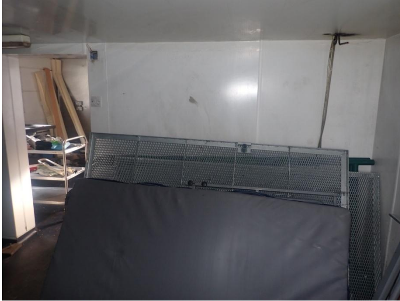
Plate 45: View of the south wall of Cell 2, from the north-west
