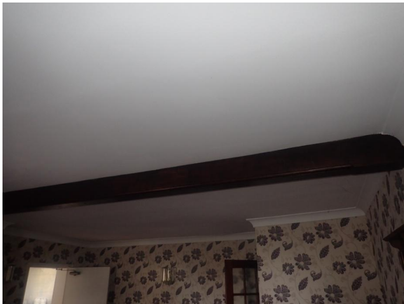
Plate 160: View of the ceiling of Cell 8, from the north
