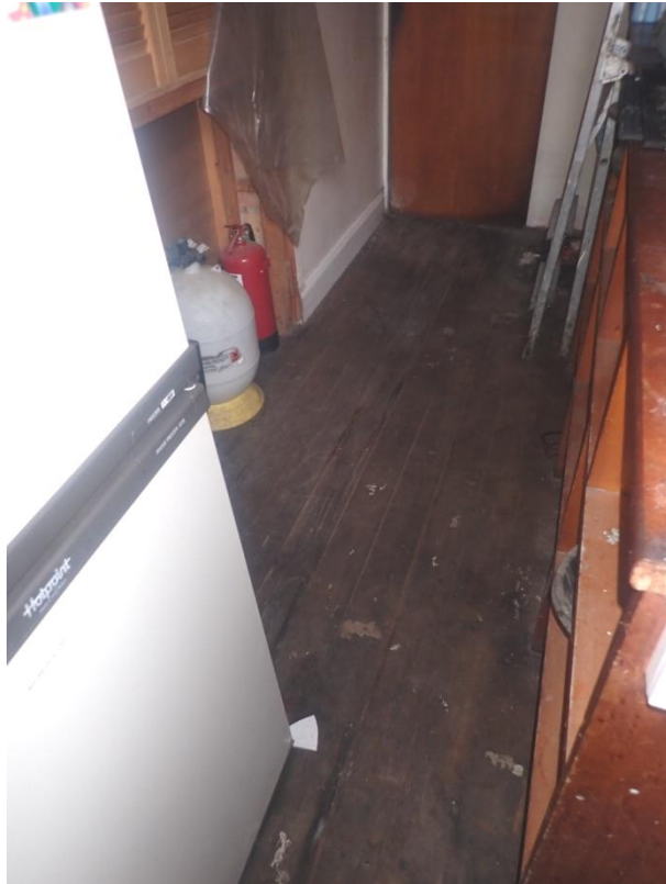
Plate 122: View of the flooring at the rear of Cell 6, from the north-west
