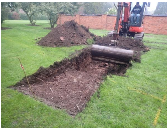
Plate 3: Excavation of the trial trench, from the north-east
