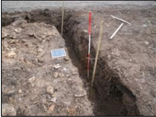
Plate 18: Completed excavation of the internal wall foundation trench, showing Section 3 , from the north
