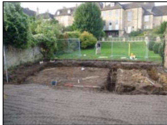
Plate 28: Completed foundation excavations of the new garage/garden store , from the south
