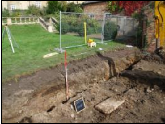
Plate 13: Section 1 & excavated foundation trench, from the south-west
