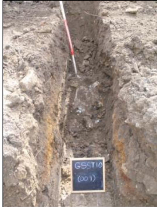
Plate 16: Excavation of the internal dividing wall foundation trench between the garage & garden store showing the pit fill (009), from the north
