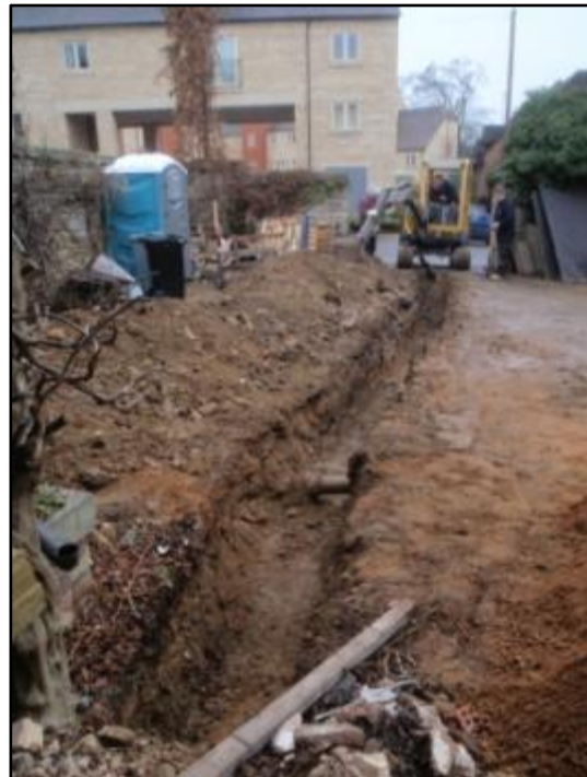
Plate 36: Completed excavation of the second service trench, from the north
