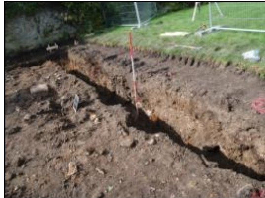
Plate 11: Section 1 & excavated foundation trench, from the south-east
