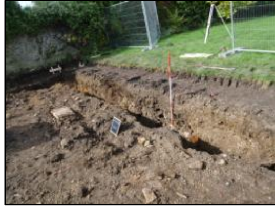
Plate 10: Section 1 & excavated foundation trench, from the south-east
