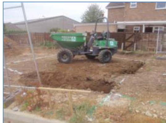
Plate 22: Excavation of the garage foundations, from the east
