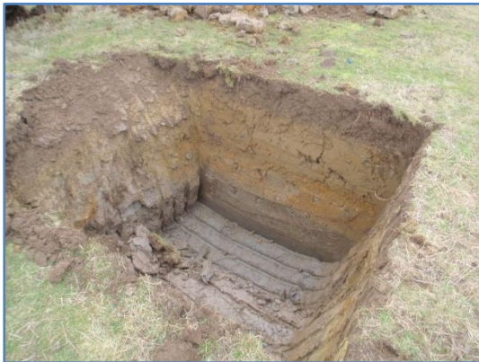
Plate 2: Work in progress,excavation of the soakaway, from the south-west
