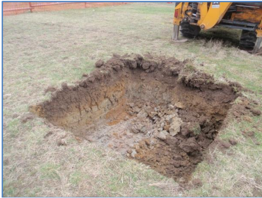
Plate 1: Work in progress,excavation of the soakaway, from the south
