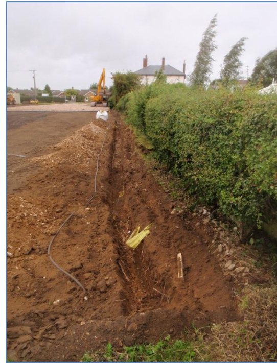
Plate 28: Service trench along the northern site boundary, from the east
