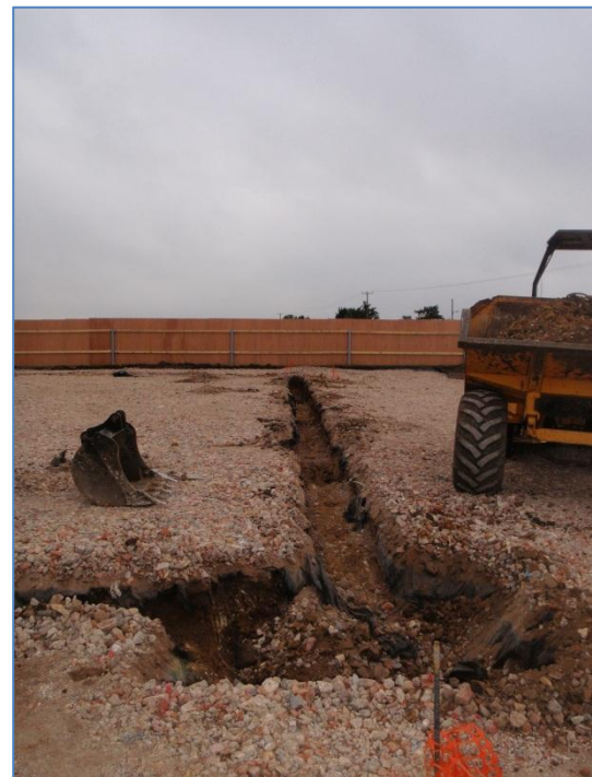
Plate 42: Excavation of Stanchion Bases 20-23 & linking foundation trenches, from the north
