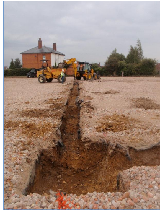
Plate 41: Excavation of Stanchion Bases 20-22 & linking foundation trenches, from the south
