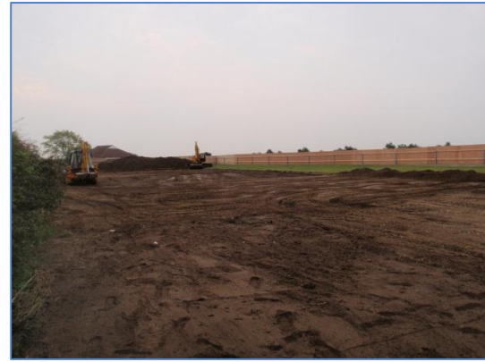
Plate 17: Initial ground reduction, from the west
