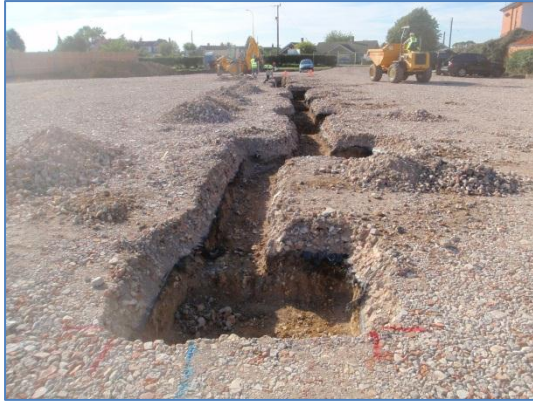
Plate 34: Excavation of Stanchion Bases 13-18 & linking foundation trenches, from the east
