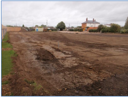
Plate 25: Completed initial ground reduction, from the south-east
