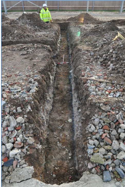
Plate 48: Excavation of the internal foundation trenches, from the north
