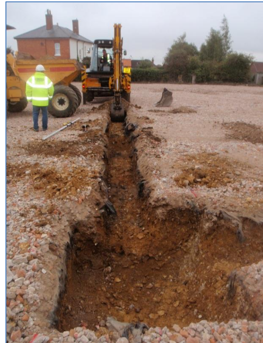
Plate 38: Excavation of Stanchion Base 20 & linking foundation trenches, from the south
