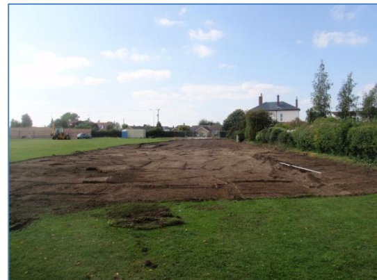
Plate 13: Initial ground reduction, from the east
