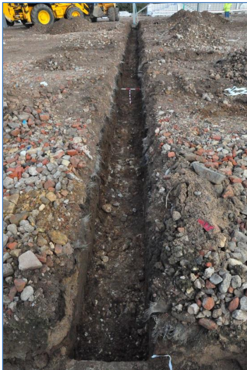
Plate 52: Excavation of the internal foundation trenches, from the south
