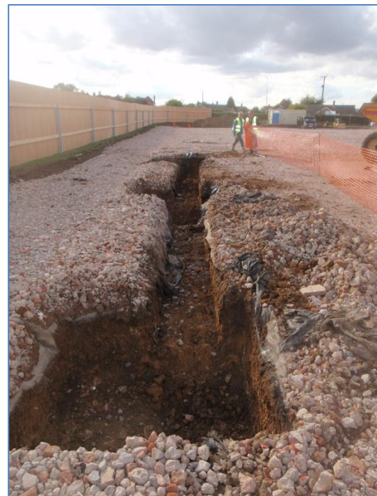
Plate 33: Excavation of Stanchion Bases 1-3 & linking foundation trenches, from the east
