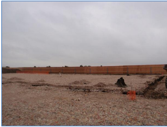
Plate 43: Excavation of Stanchion Bases 19 & 20-23 & linking foundation trenches, from the north
