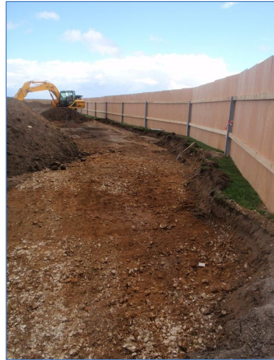
Plate 23: Initial ground reduction, from the west, showing the exposed natural horizon (002)
