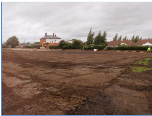
Plate 26: Completed initial ground reduction, from the south-east
