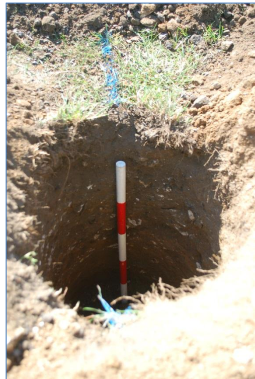
Plate 8: Fence hole 18, from the south
