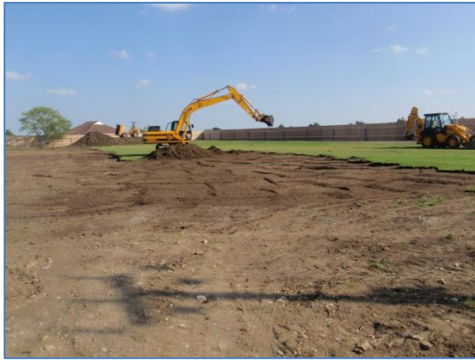
Plate 14: Initial ground reduction, from the west
