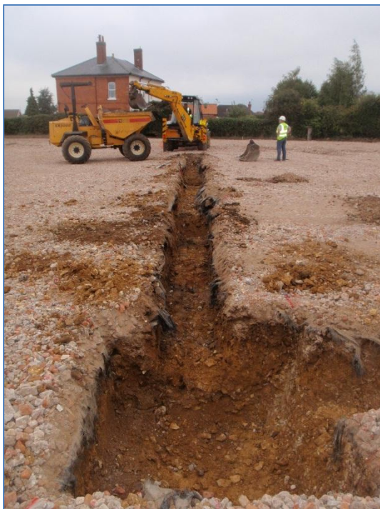
Plate 40: Excavation of Stanchion Bases 20-21 & linking foundation trenches, from the south
