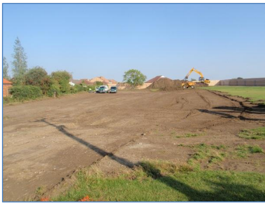
Plate 15: Initial ground reduction, from the west
