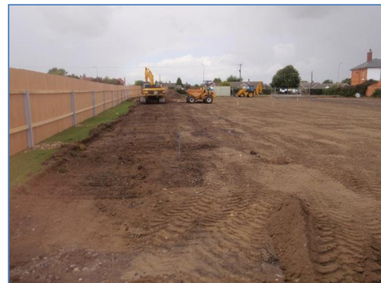
Plate 24: Initial ground reduction, from the east
