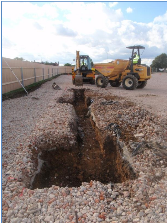
Plate 31: Excavation of Stanchion Bases 1 & 2 & linking foundation trenches, from the east
