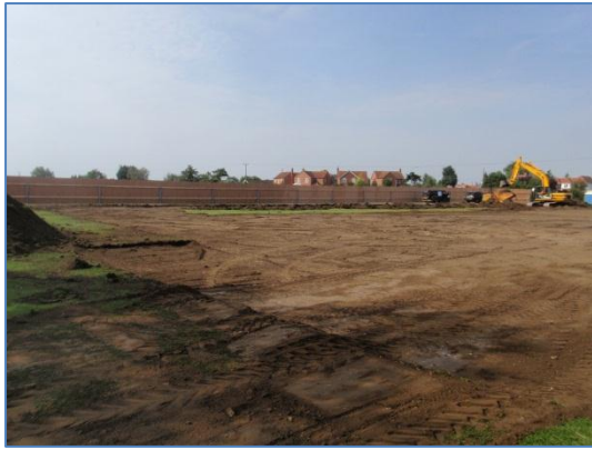
Plate 20: Initial ground reduction, from the north-east
