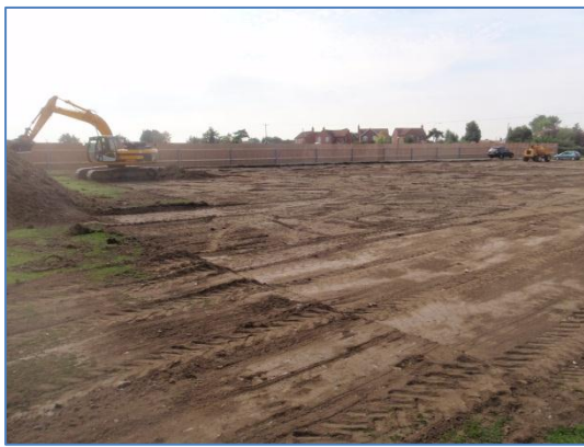
Plate 21: Initial ground reduction, from the north-east
