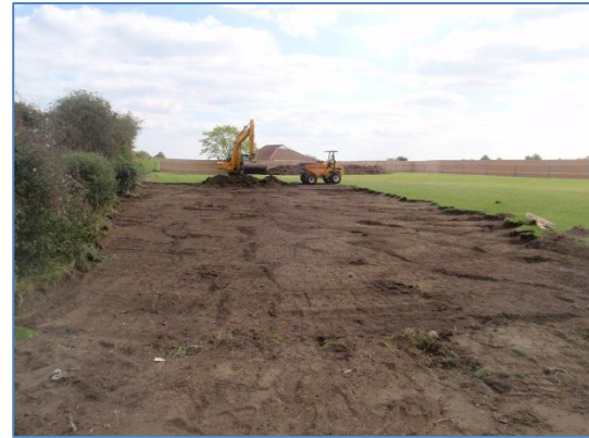
Plate 11: Initial ground reduction, from the west
