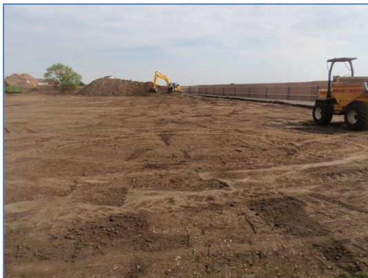
Plate 22: Initial ground reduction, from the west
