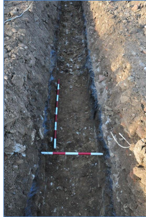
Plate 53: Excavation of the internal foundation trenches, from the south
