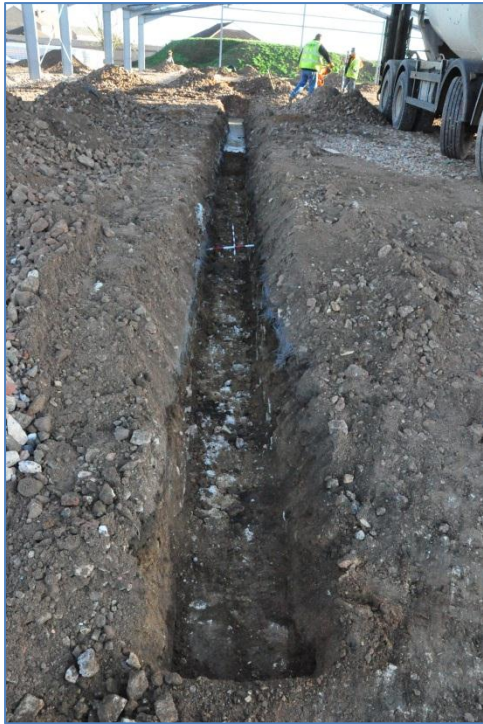
Plate 55: Excavation of the internal foundation trenches, from the west
