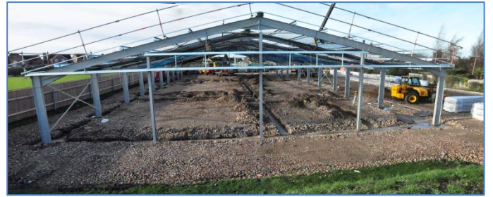
Plate 56: View of the completed internal foundation excavations, from the east
