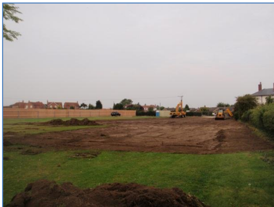
Plate 16: Initial ground reduction, from the east
