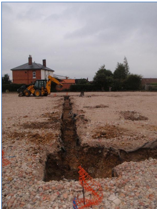
Plate 44: Excavation of Stanchion Bases 19 & 20-23 & linking foundation trenches, from the south
