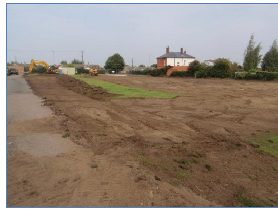
Plate 18: Initial ground reduction, from the south-east
