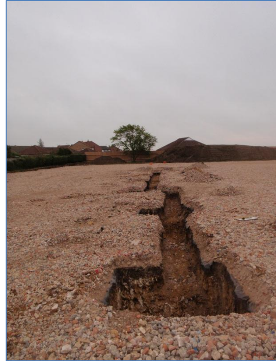
Plate 37: Excavation of Stanchion Bases 13-18 & linking foundation trenches, from the west
