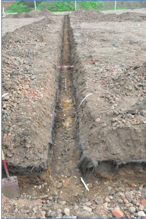
Plate 51: Excavation of the internal foundation trenches, from the west
