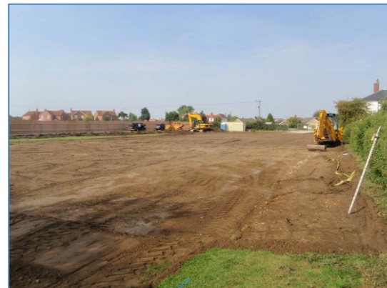
Plate 19: Initial ground reduction, from the east
