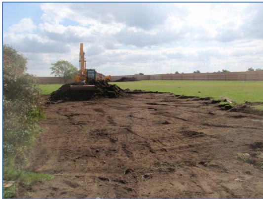
Plate 10: Initial ground reduction, from the west
