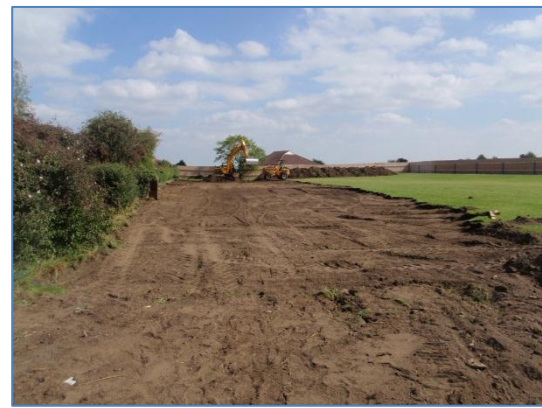
Plate 12: Initial ground reduction, from the west
