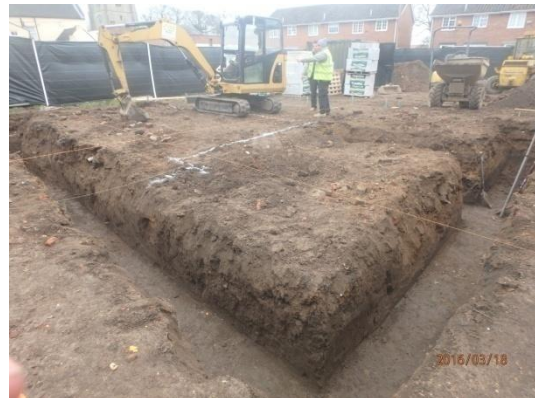
Plate 23: Excavation of the foundations, from the north-west
