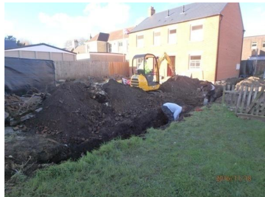
Plate 91: Excavation of the boundary wall trench, from the south-east
