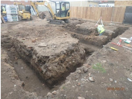
Plate 38: Excavation of the foundations, from the north-east
