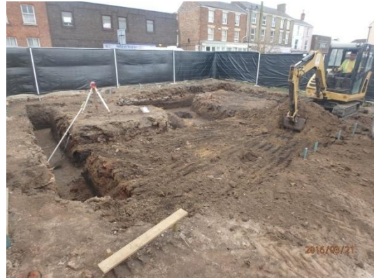
Plate 53: Limited ground reduction, from the south
