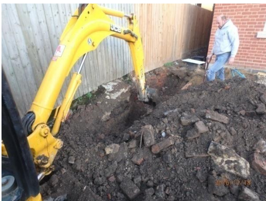
Plate 69: Excavation of the first service trench, from the south
