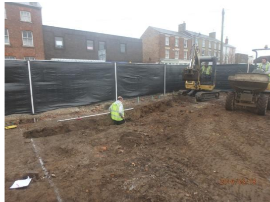
Plate 5: Excavation of the foundations, from the south-west
