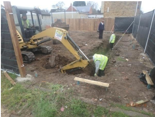
Plate 9: Excavation of the foundations, from the east
