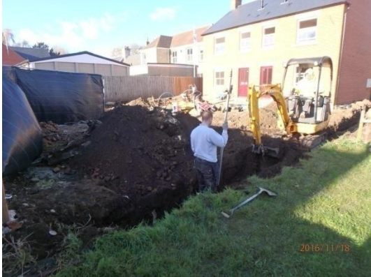
Plate 86: Excavation of the boundary wall trench, from the south-east
