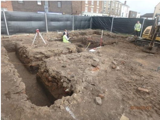
Plate 44: Excavation of the foundations, from the south
