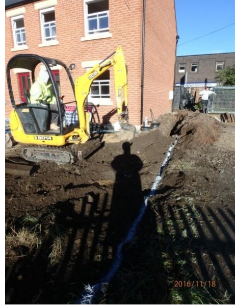
Plate 79: Excavation of the boundary wall trench, from the south
