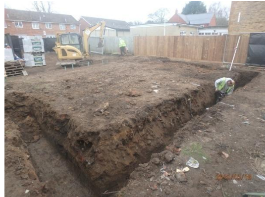
Plate 17: Excavation of the foundations, from the north-east
