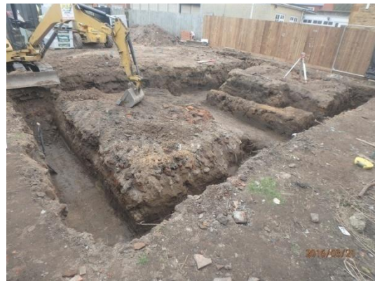
Plate 48: Excavation of the foundations, from the north-east
