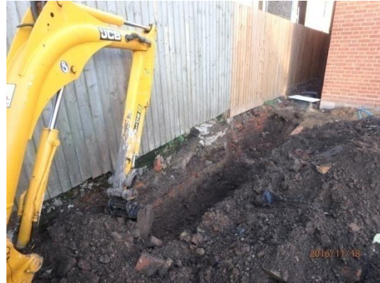
Plate 70: Excavation of the first service trench, from the south
