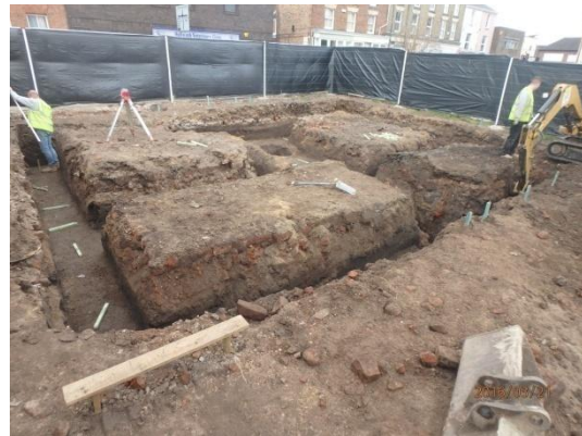
Plate 66: Excavation of the foundations, from the south
