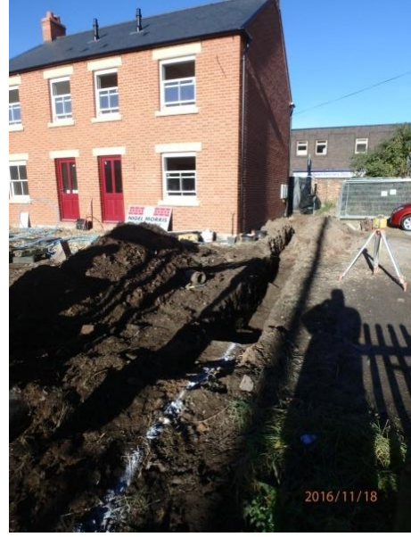
Plate 84: Excavation of the boundary wall trench, from the south
