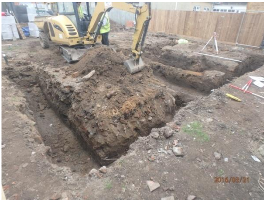
Plate 39: Limited ground reduction, from the north-east
