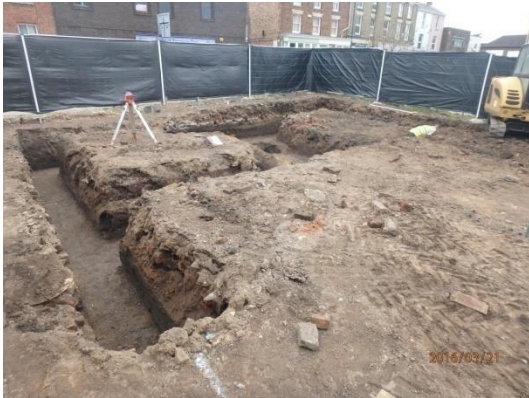
Plate 50: Excavation of the foundations, from the south
