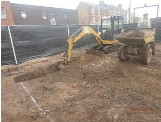
Plate 2: Excavation of the foundations, from the south-west
