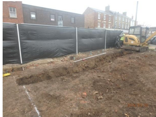
Plate 6: Excavation of the foundations, from the south-west
