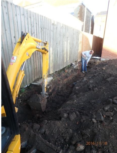
Plate 72: Excavation of the first service trench, from the south
