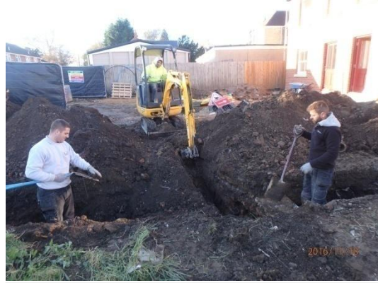
Plate 93: Excavation of the third service trench, from the east
