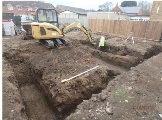
Plate 41: Limited ground reduction and excavation of the foundations, from the north-east
