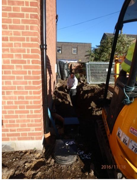
Plate 77: Excavation of the boundary wall trench, from the south
