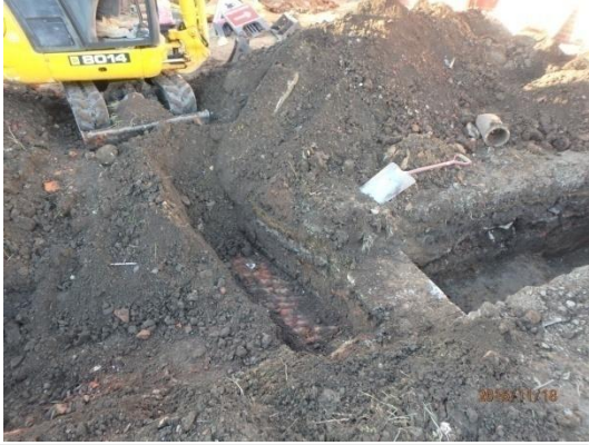
Plate 92: Excavation of the third service trench, from the east
