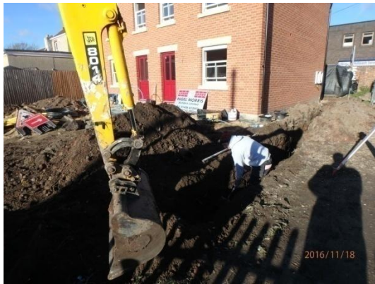
Plate 82: Excavation of the boundary wall trench, from the south
