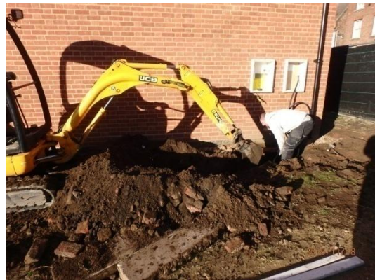
Plate 75: Excavation of the boundary wall trench, from the east
