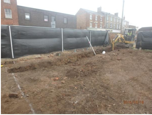
Plate 7: Excavation of the foundations, from the south-west
