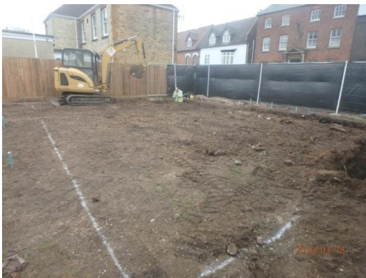
Plate 15: Excavation of the foundations, from the south-east
