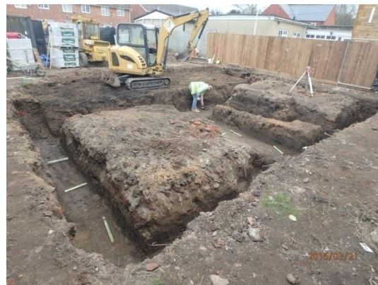
Plate 54: Limited ground reduction, from the north-east
