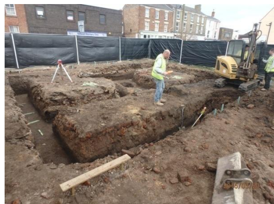
Plate 60: Excavation of the foundations, from the south
