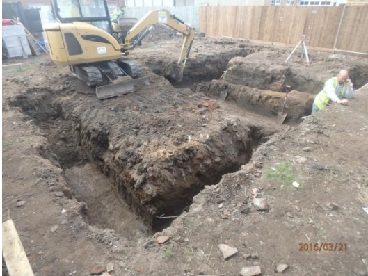
Plate 43: Excavation of the foundations, from the north-east
