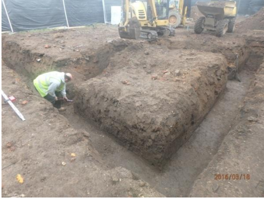
Plate 25: Excavation of the foundations, from the north-west
