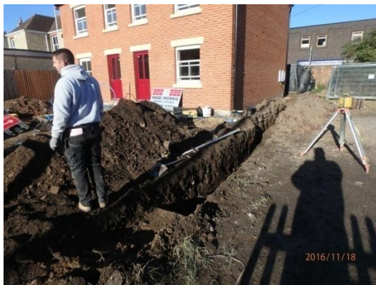
Plate 83: Excavation of the boundary wall trench, from the south
