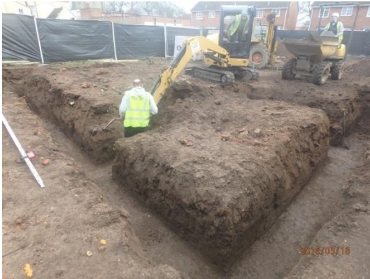
Plate 26: Excavation of the foundations, from the north-west
