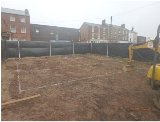
Plate 1: Pre-groundworks, from the south
