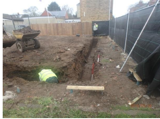
Plate 10: Excavation of the foundations, from the east
