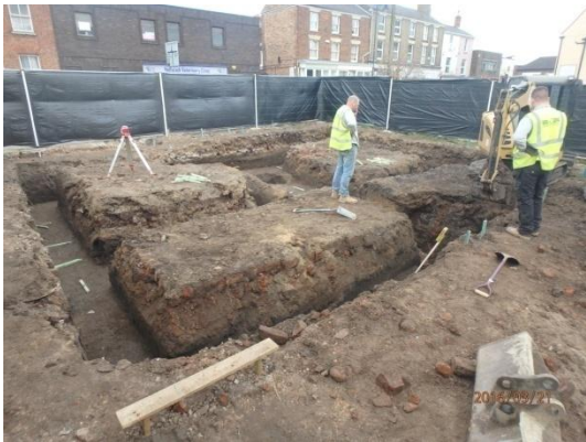
Plate 63: Excavation of the foundations, from the south
