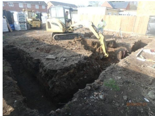
Plate 30: Excavation of the foundations, from the north-east
