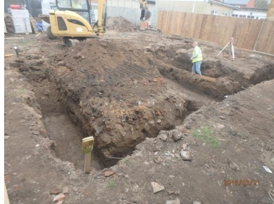
Plate 40: Limited ground reduction, from the north-east
