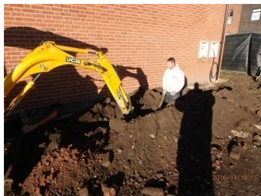
Plate 76: Excavation of the boundary wall trench, from the east
