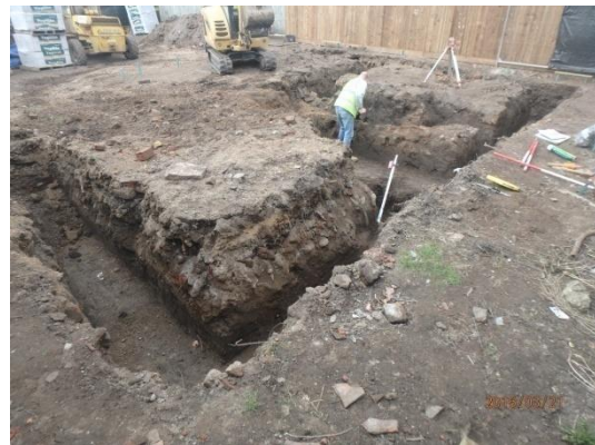
Plate 35: Excavation of the foundations, from the north-east
