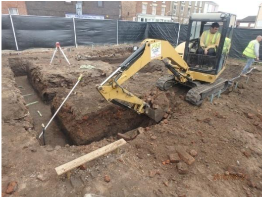
Plate 56: Excavation of the foundations, from the south
