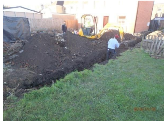
Plate 90: Excavation of the boundary wall trench, from the south-east
