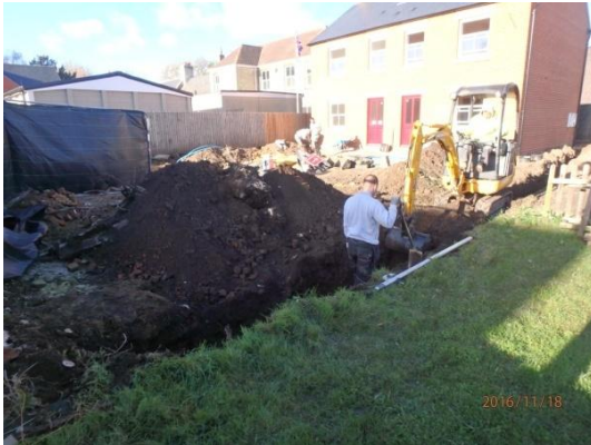
Plate 87: Excavation of the boundary wall trench, from the south-east
