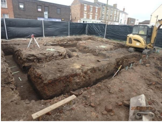
Plate 61: Excavation of the foundations, from the south
