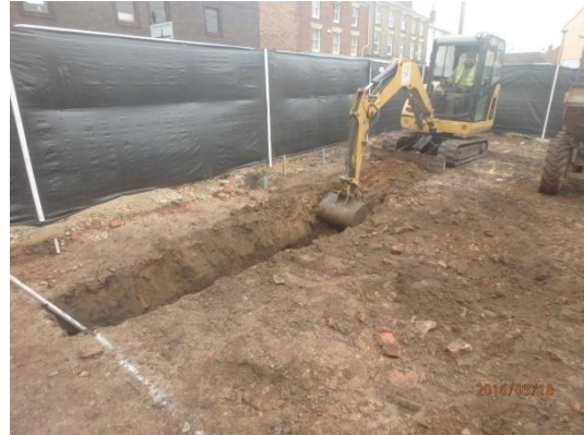
Plate 4: Excavation of the foundations, from the south-west
