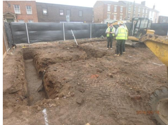
Plate 29: Excavation of the foundations, from the south
