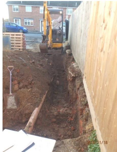
Plate 71: Excavation of the first service trench, from the north
