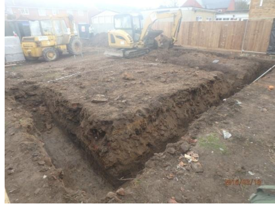
Plate 28: Excavation of the foundations, from the north-east
