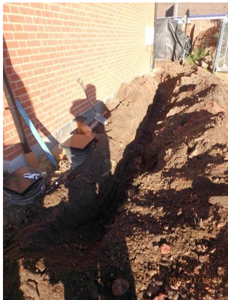
Plate 78: Excavation of the boundary wall trench, from the south
