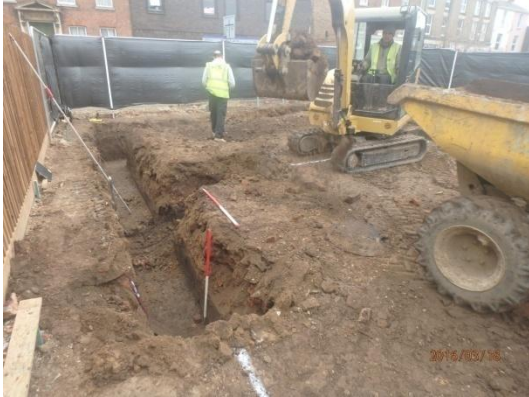
Plate 19: Excavation of the foundations, from the south
