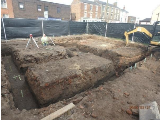
Plate 67: Excavation of the foundations, from the south
