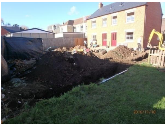
Plate 88: Excavation of the boundary wall trench, from the south-east
