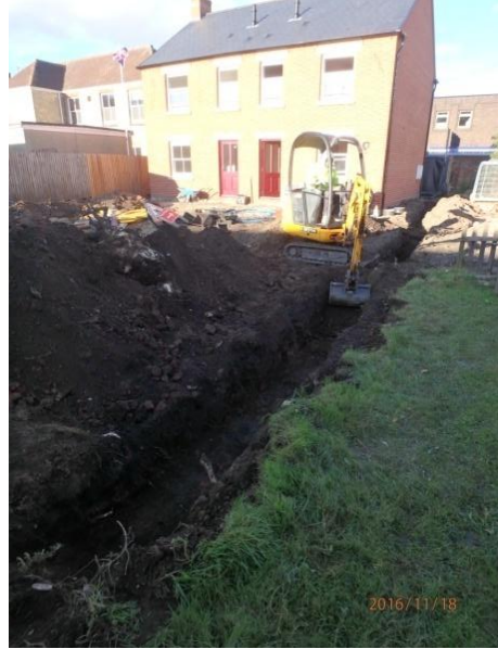
Plate 89: Excavation of the boundary wall trench, from the south
