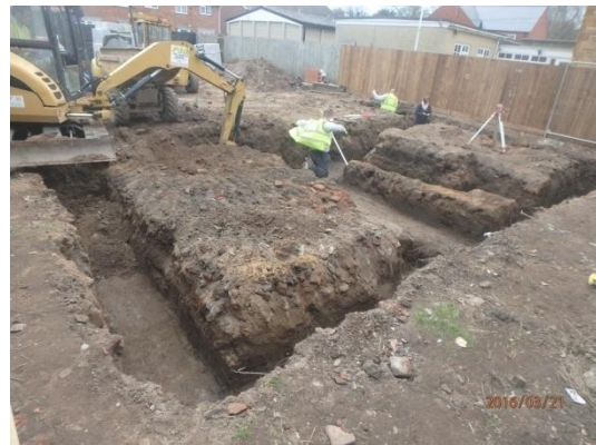
Plate 47: Excavation of the foundations, from the north-east
