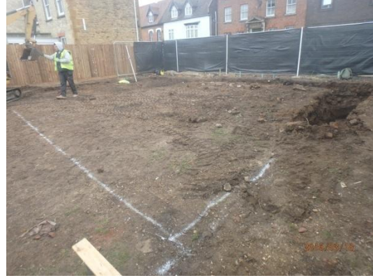
Plate 16: Excavation of the foundations, from the south-east
