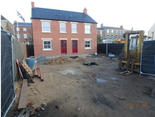
Plate 68: Pre-groundworks, from the south
