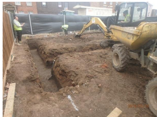
Plate 24: Excavation of the foundations, from the south
