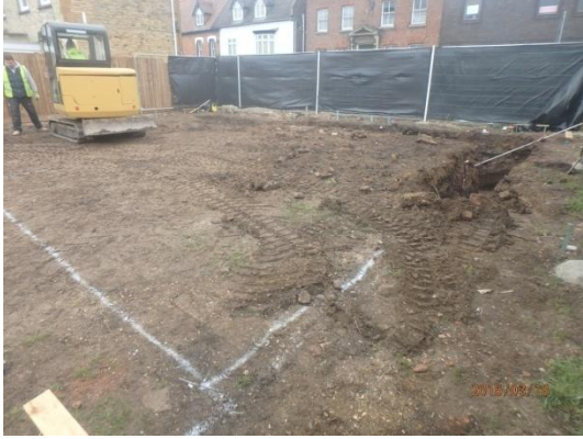
Plate 13: Excavation of the foundations, from the south-east
