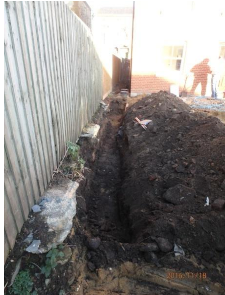
Plate 74: Excavation of the first service trench, from the south
