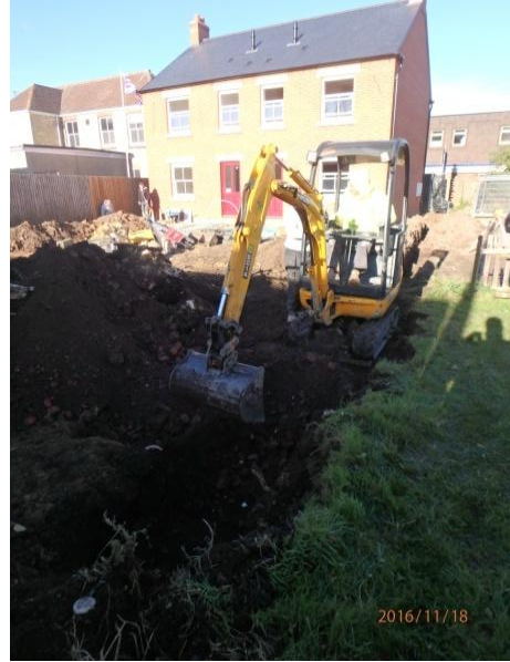
Plate 85: Excavation of the boundary wall trench, from the south
