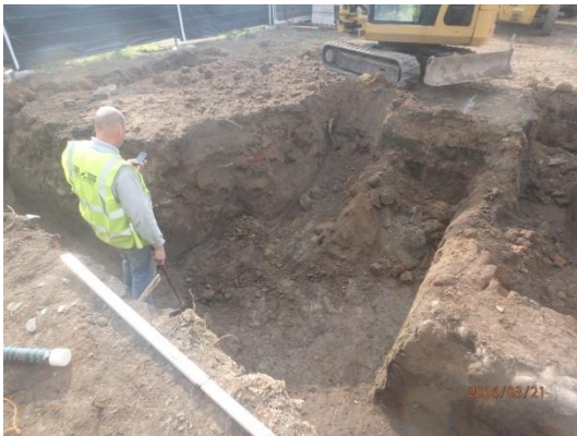
Plate 32: Excavation of the foundations, from the north
