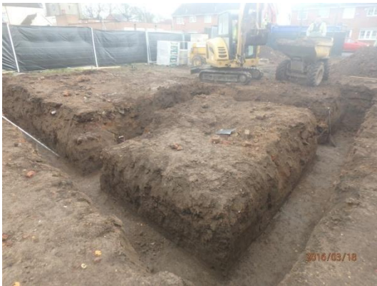
Plate 27: Excavation of the foundations, from the north-west
