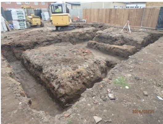
Plate 51: Excavation of the foundations, from the north-east
