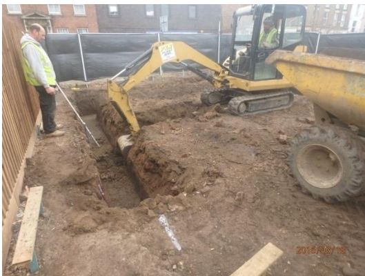
Plate 21: Excavation of the foundations, from the south
