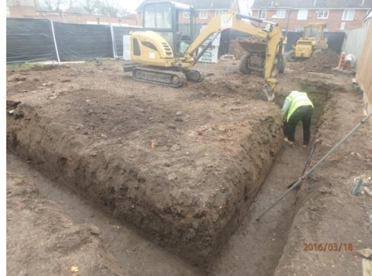
Plate 22: Excavation of the foundations, from the north-west
