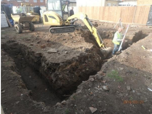
Plate 31: Excavation of the foundations, from the north-east
