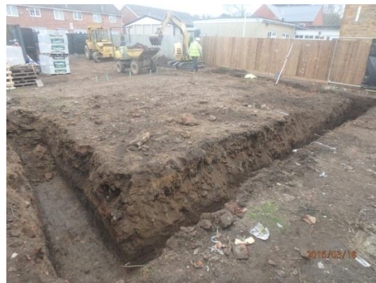
Plate 18: Excavation of the foundations, from the north-east
