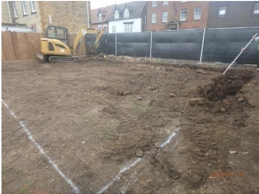
Plate 14: Excavation of the foundations, from the south-east
