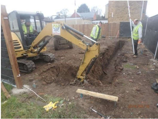
Plate 8: Excavation of the foundations, from the east
