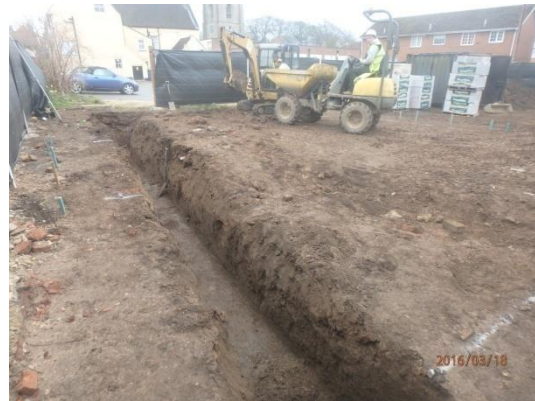
Plate 12: Excavation of the foundations, from the west
