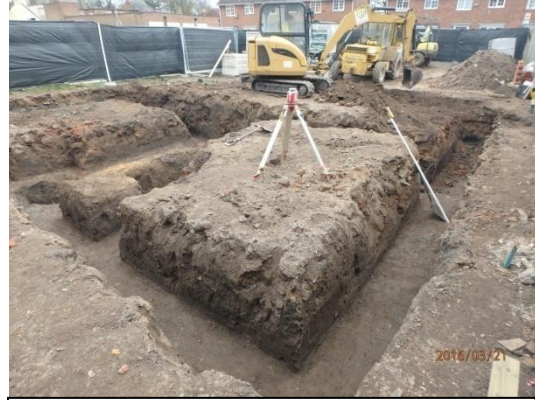
Plate 52: Limited ground reduction, from the north-west
