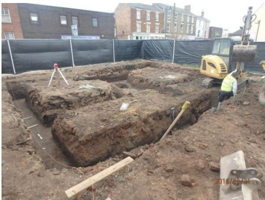
Plate 57: Excavation of the foundations, from the south
