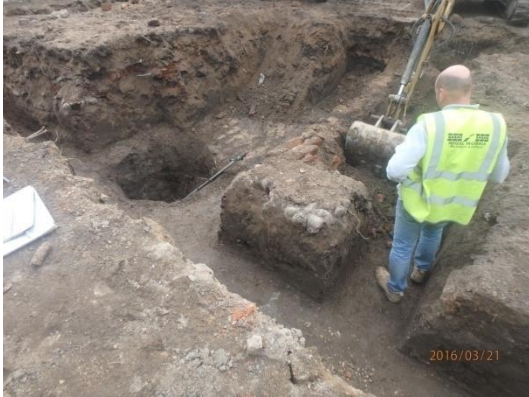
Plate 37: View of the mixed yard surface within (001), from the north
