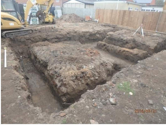
Plate 49: Excavation of the foundations, from the north-east
