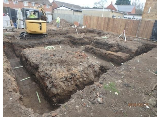
Plate 58: Excavation of the foundations, from the north-east
