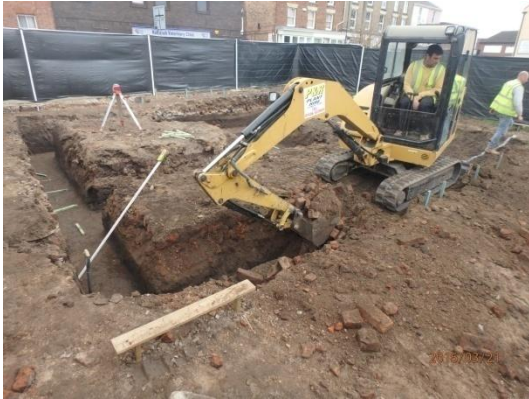
Plate 55: Excavation of the foundations, from the south
