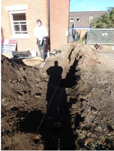
Plate 81: Excavation of the boundary wall trench, from the south
