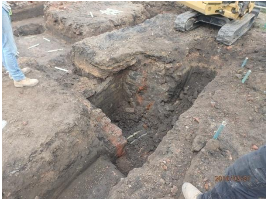
Plate 62: View of the deep cellar walls, from the south-west
