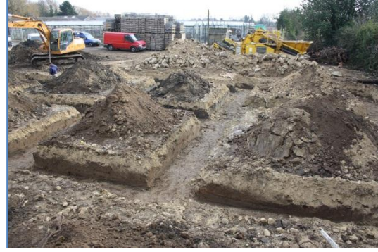
Plate 10: Work in progress, excavation of the foundation trenches, from the north-west
