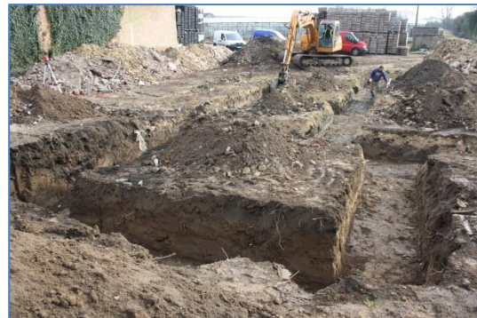
Plate 12: Work in progress, excavation of the foundation trenches, from the north-west
