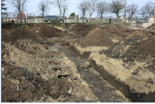
Plate 7: Work in progress, excavation of the foundation trenches, from the east
