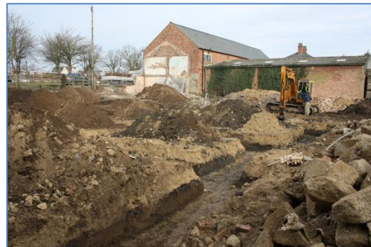
Plate 6: Work in progress, excavation of the foundation trenches, from the south
