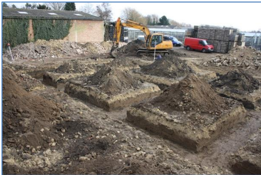
Plate 8: Work in progress, excavation of the foundation trenches, from the west
