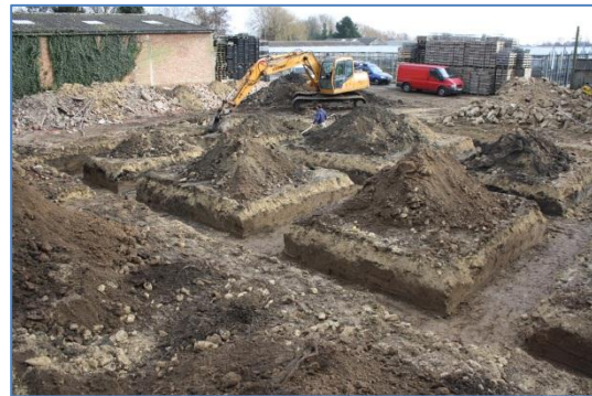
Plate 11: Work in progress, excavation of the foundation trenches, from the west
