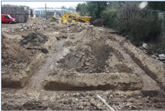
Plate 9: Work in progress, excavation of the foundation trenches, from the north-west
