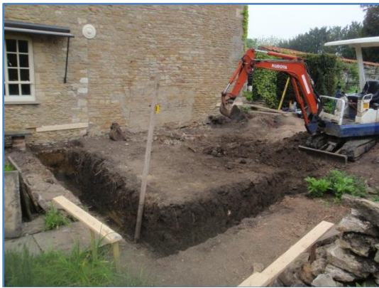
Plate 7: Work in progress, excavation of the foundations, from the south
