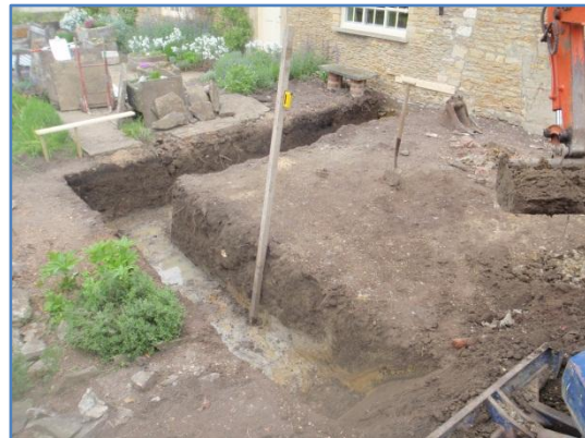
Plate 9: Work in progress, excavation of the foundations, from the east
