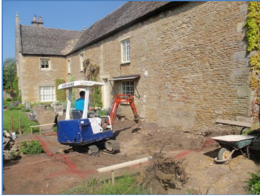
Plate 1: Set out foundations, from the east
