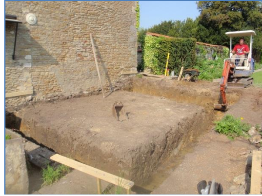
Plate 19: Completed groundworks, from the south-west
