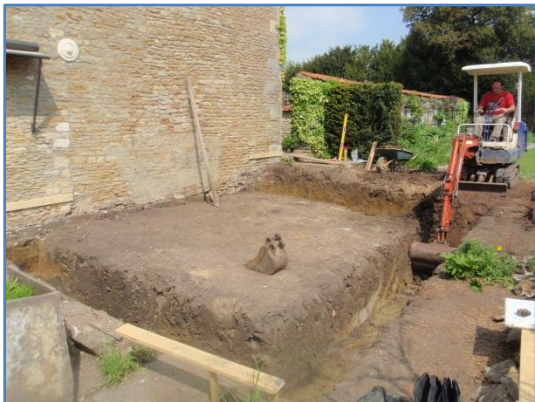
Plate 18: Work in progress, excavation of the foundations, from the south-west
