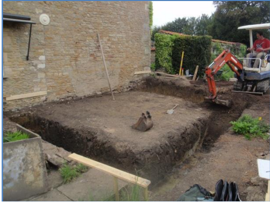
Plate 17: Work in progress, excavation of the foundations, from the south-west
