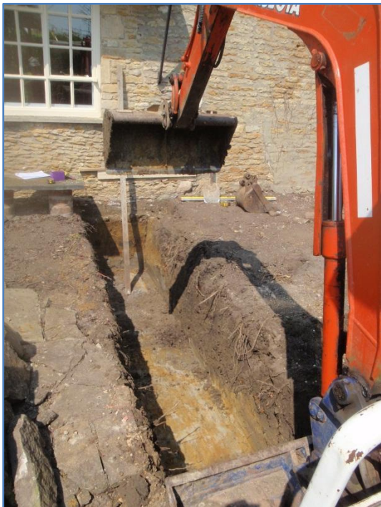
Plate 2: Work in progress, excavation of the foundations, from the south
