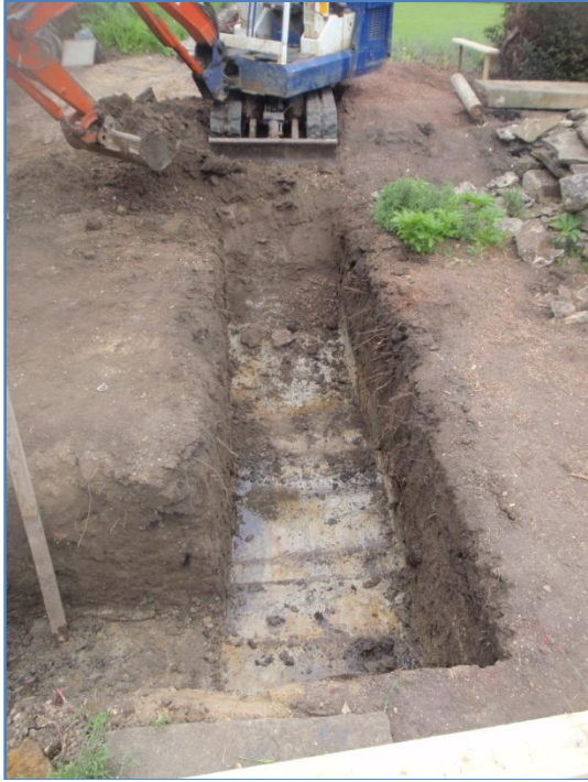
Plate 6: Work in progress, excavation of the foundations, from the west
