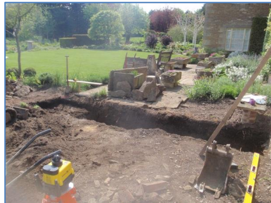
Plate 4: Work in progress, excavation of the foundations, from the east
