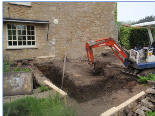
Plate 5: Work in progress, excavation of the foundations, from the south
