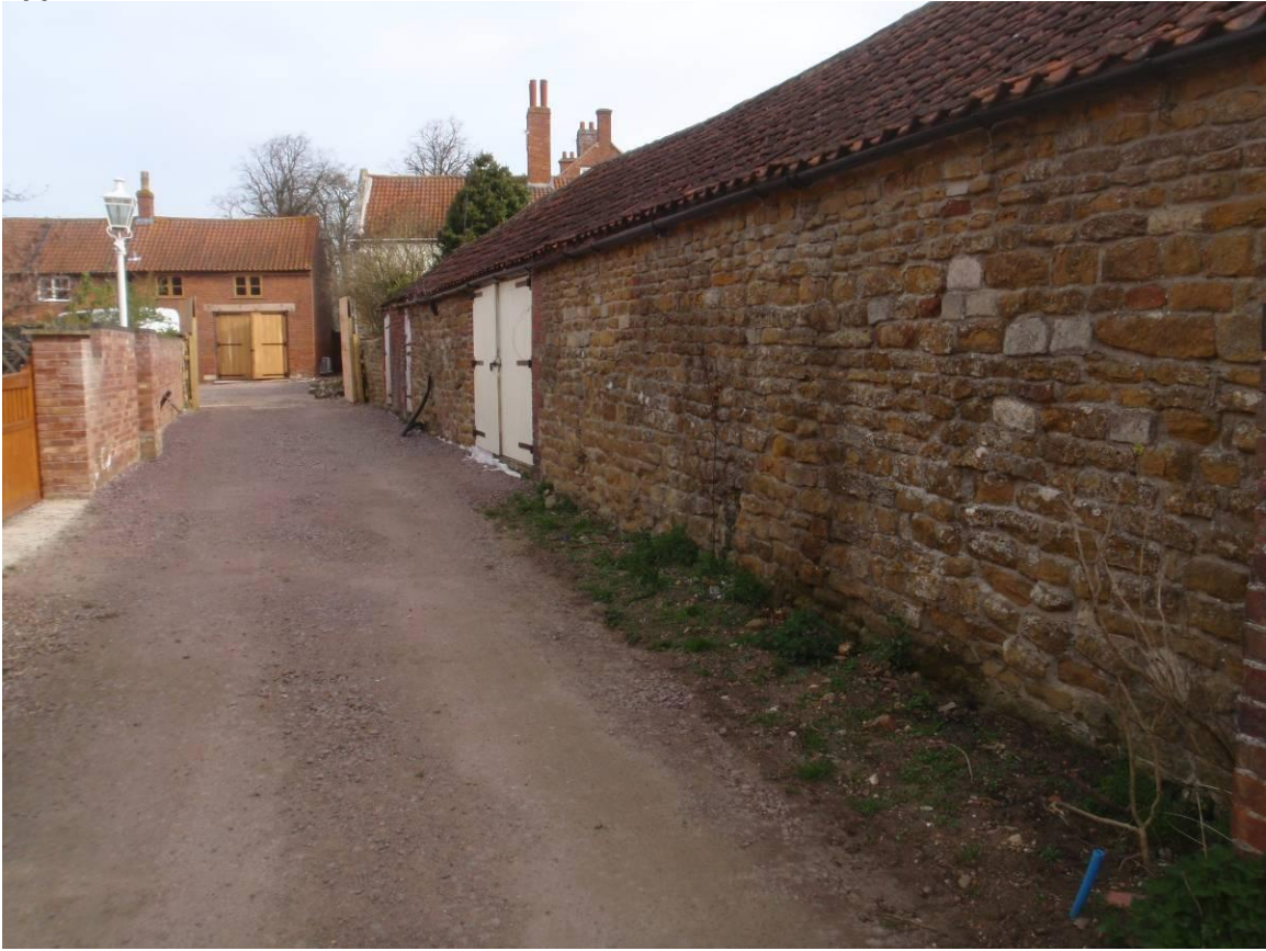
Plate 1: Pre-site works, from the south
