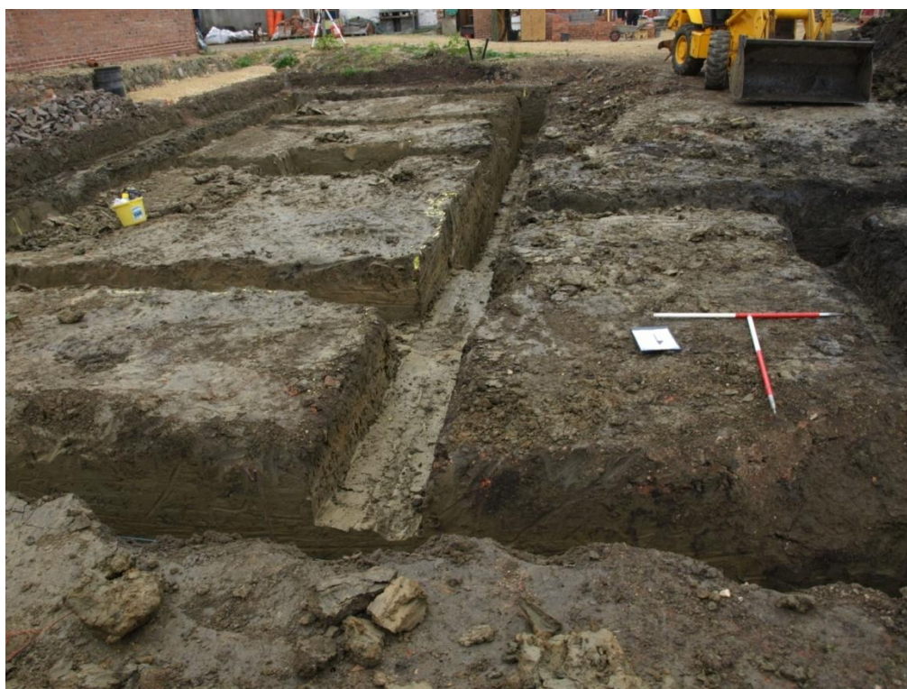
Plate 16: Excavated foundations, from the west
